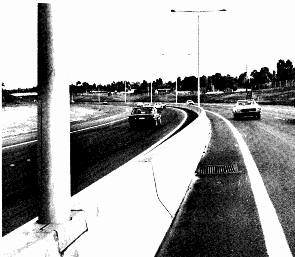
Above: The concrete median barrier on the Eastern Freeway Arterial Road Extension
