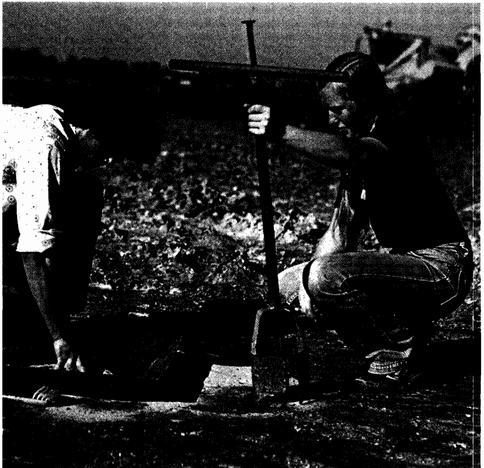
Below: Testing compacted material on the Princes Freeway, bypass of Berwick
