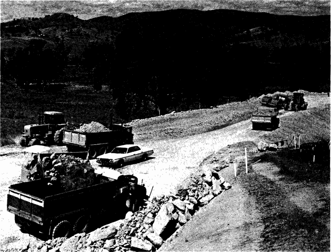
Above: Construction on the Maroondah Highway at Acheron
