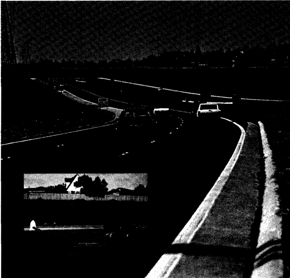
Above: The newly-opened section of the Mulgrave Freeway, looking east, between Warrigal Road and Huntingdale Road
