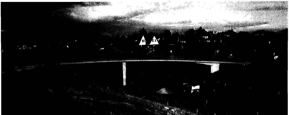
Jacana Street pedestrian overpass spanning an unopened section of the Mulgrave Freeway, Chadstone.
