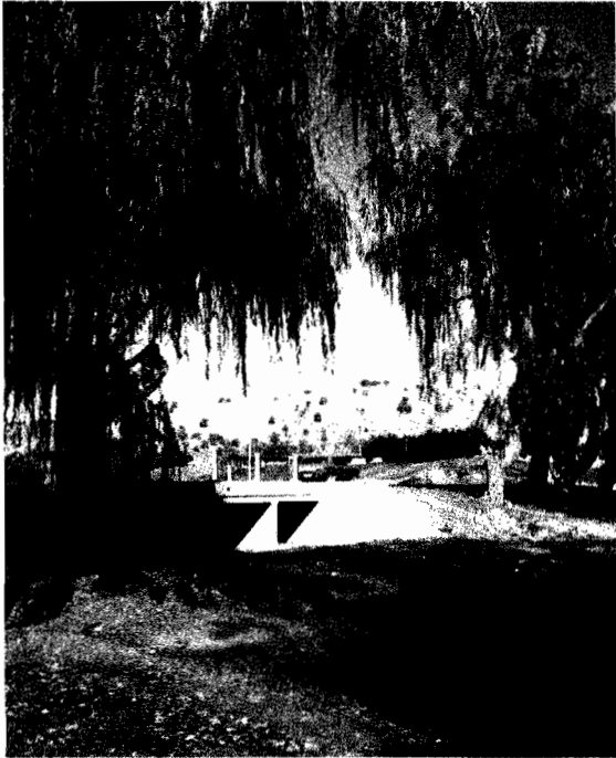
Huon Creek Road — a 4 cell box culvert over House Creek, Wodonga City (Unclassified road).
