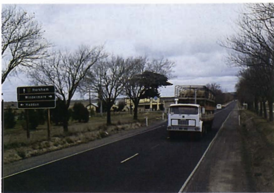
Western Highway reconstruction completed east of the Hadden-Windermere Road.
