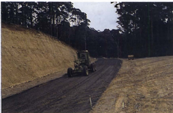
Greendale-Trentham Road, Shire of Ballan — reconstruction north of Barry's Reef.
