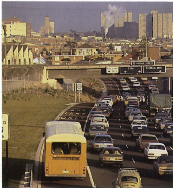
Eastern Freeway — exclusive bus lane and morning peak traffic on exit ramp at Hoddle Street.
