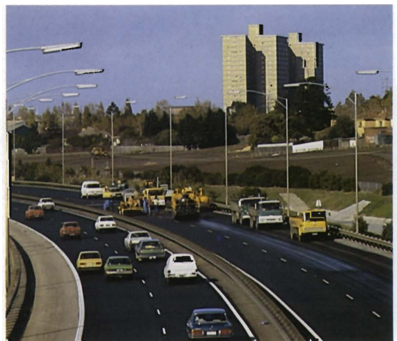
Tullamarine Freeway — asphalt resurfacing south of Brunswick Road.
