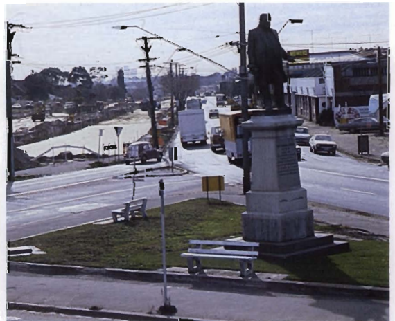
Nepean Highway, at the Hampton Street intersection — construction of divided highway.
