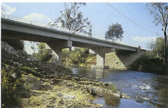
Upper Merriang Road bridge over Buffalo River.
