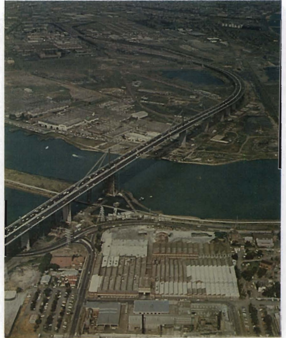
West Gate Bridge across the Yarra River.
