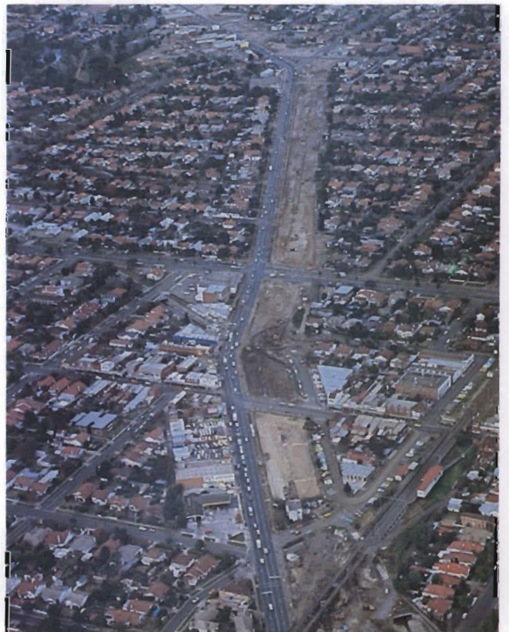
Nepean Highway — widening work south from Gardenvale.
