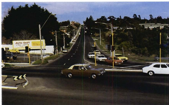
Reconstruction and widening of Princess Street, City of Kew.
