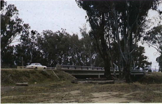
New 2 span bridge on the Violet Town-Dookie Road over the Broken River, Shire of Violet Town.
