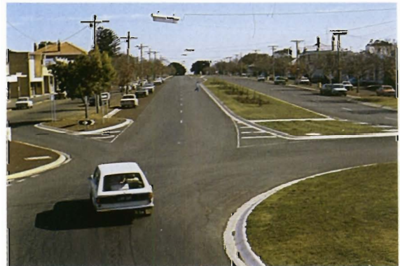
Hamilton Highway — duplication in Mortlake.
