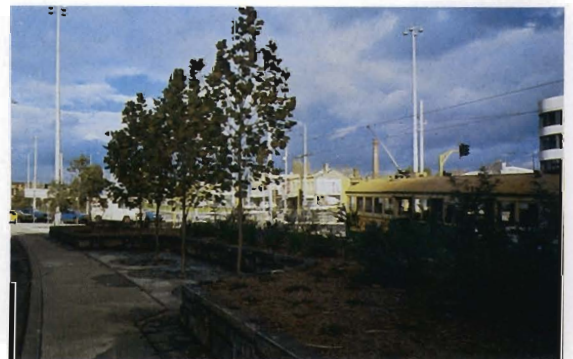
St Kilda Junction — blue stone wall and newly planted trees and shrubs.
