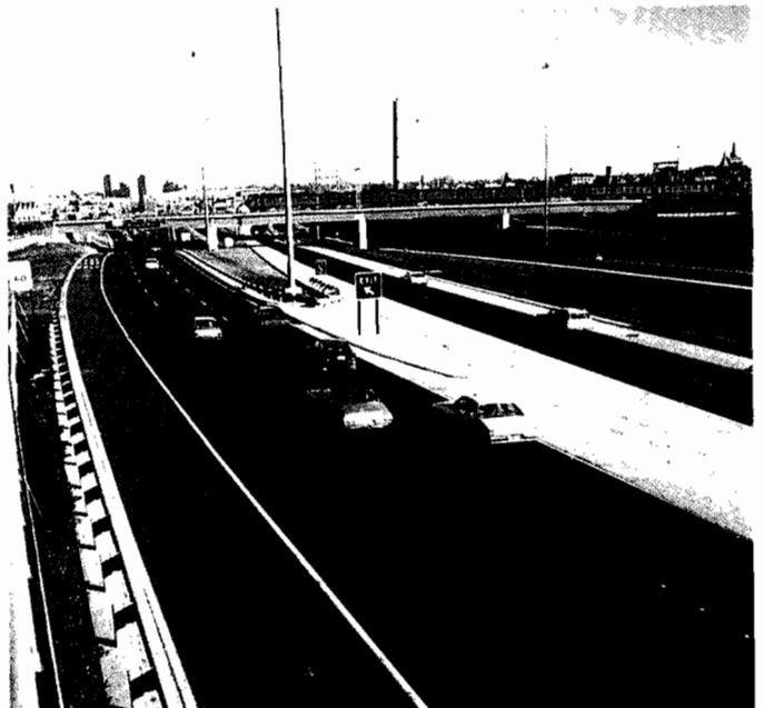
Eastern Freeway — exclusive bus lane on exit ramp at Hoddle Street.
