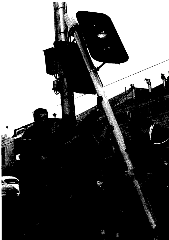
Installation of Advisory Truck Route traffic signals at corner of Clarendon and Grant Streets, South Melbourne.
