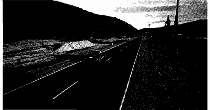
Ovens Highway reconstruction completed between Ovens and Eurobin.
