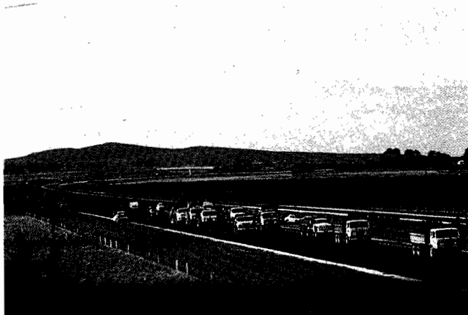
Hume Freeway — asphalt paving south of Wandong.
