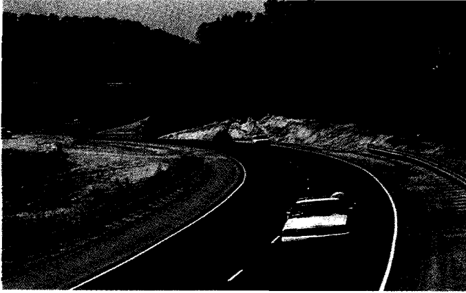
Calder Highway — reconstruction north of Harcourt.
