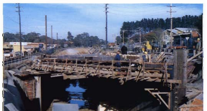
Level crossing elimination, Watsonia, part of the Greensborough Freeway Project.
