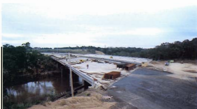
Eastern Freeway-Yarra River Bridge.
