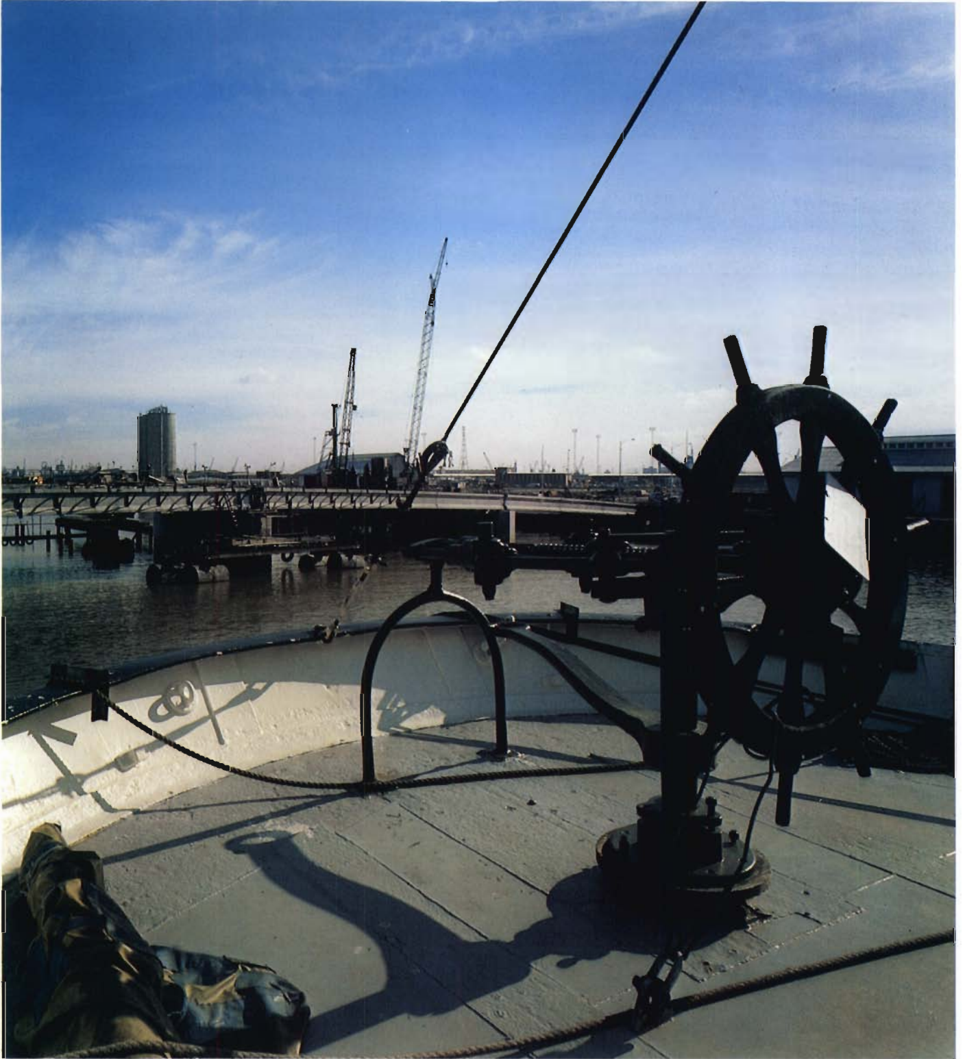
Johnson Street Bridge, South Melbourne
