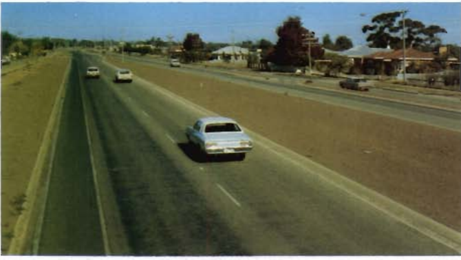
Duplication of the Western Highway, Horsham.
