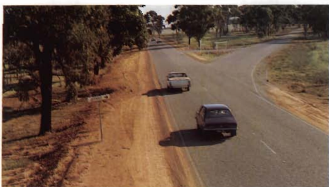
Highways — Western Highway, near Dimboola
