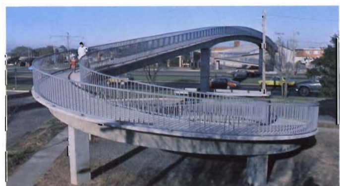
Completed pedestrian overpass, Princes Highway East at Gordon Avenue, Oakleigh.
