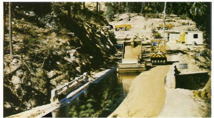
Sprayed bituminous surfacing.
