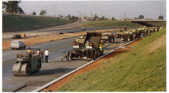
Mulgrave Freeway under construction, west of Blackburn Road.
