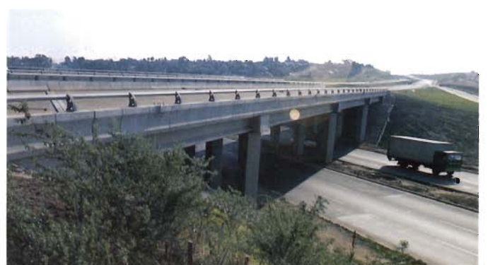
Mulgrave Freeway bridge over Ferntree Gully Road.
