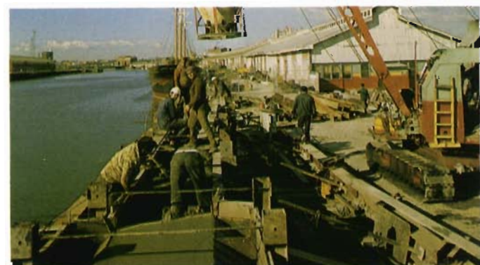
Johnson Street Bridge, South Melbourne.
