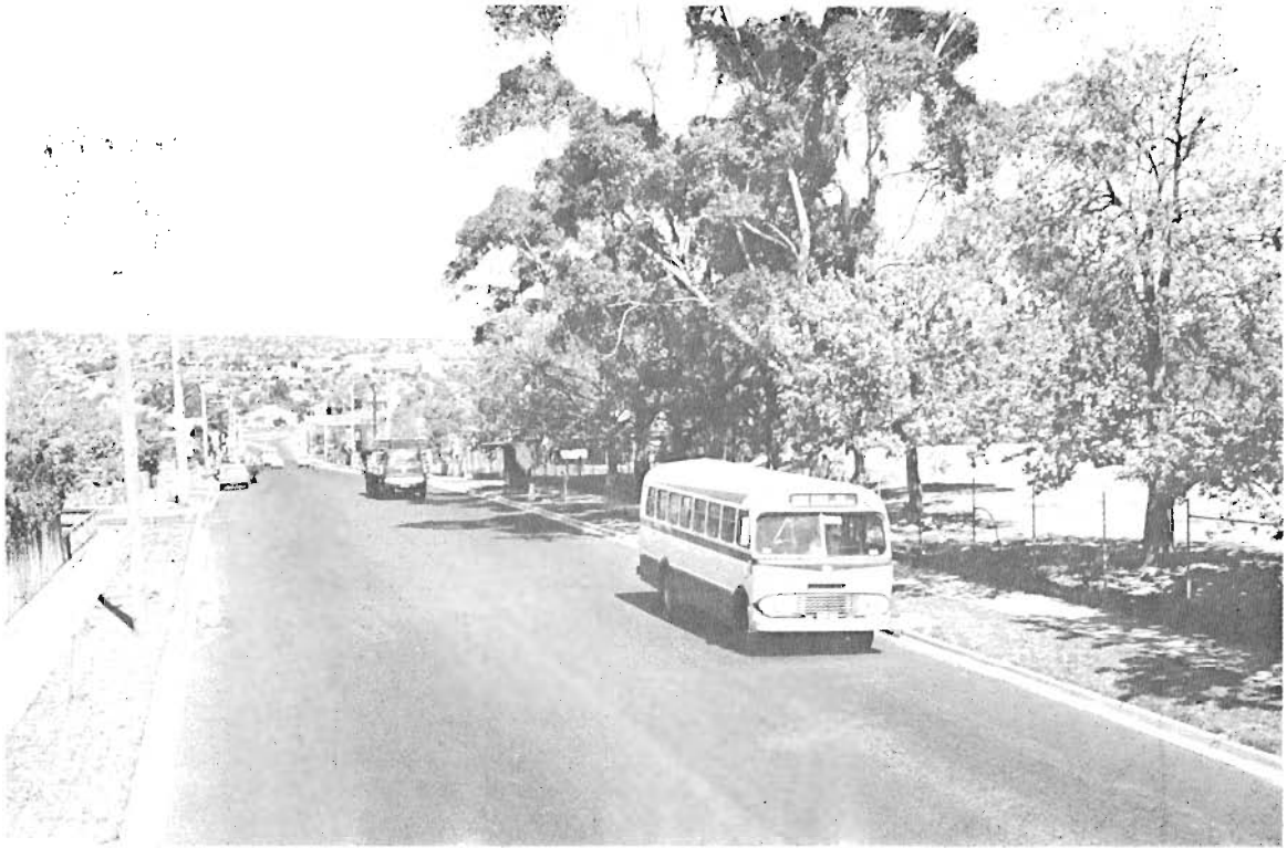
Station Street, Box Hill South, reconstructed by the Box Hill City Council with financial assistance from the Board.
