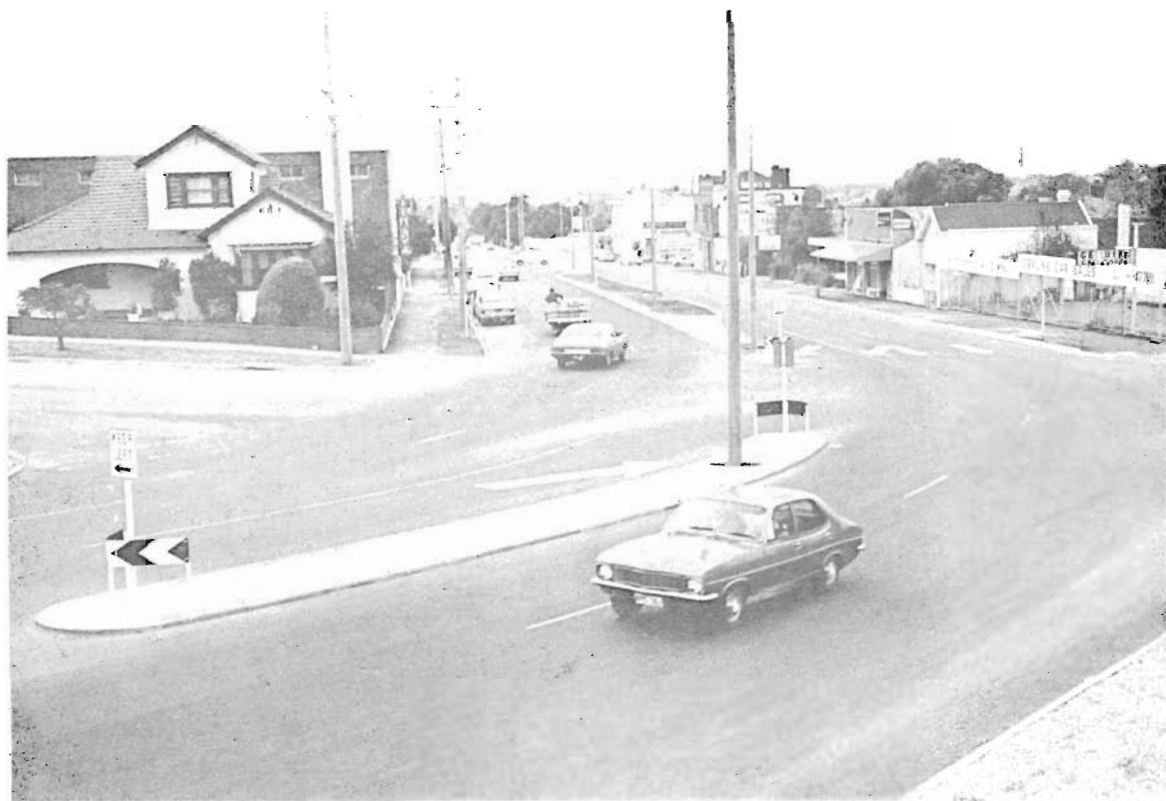
Reconstructed section of the Calder Highway providing dual carriageways in Bendigo City.
