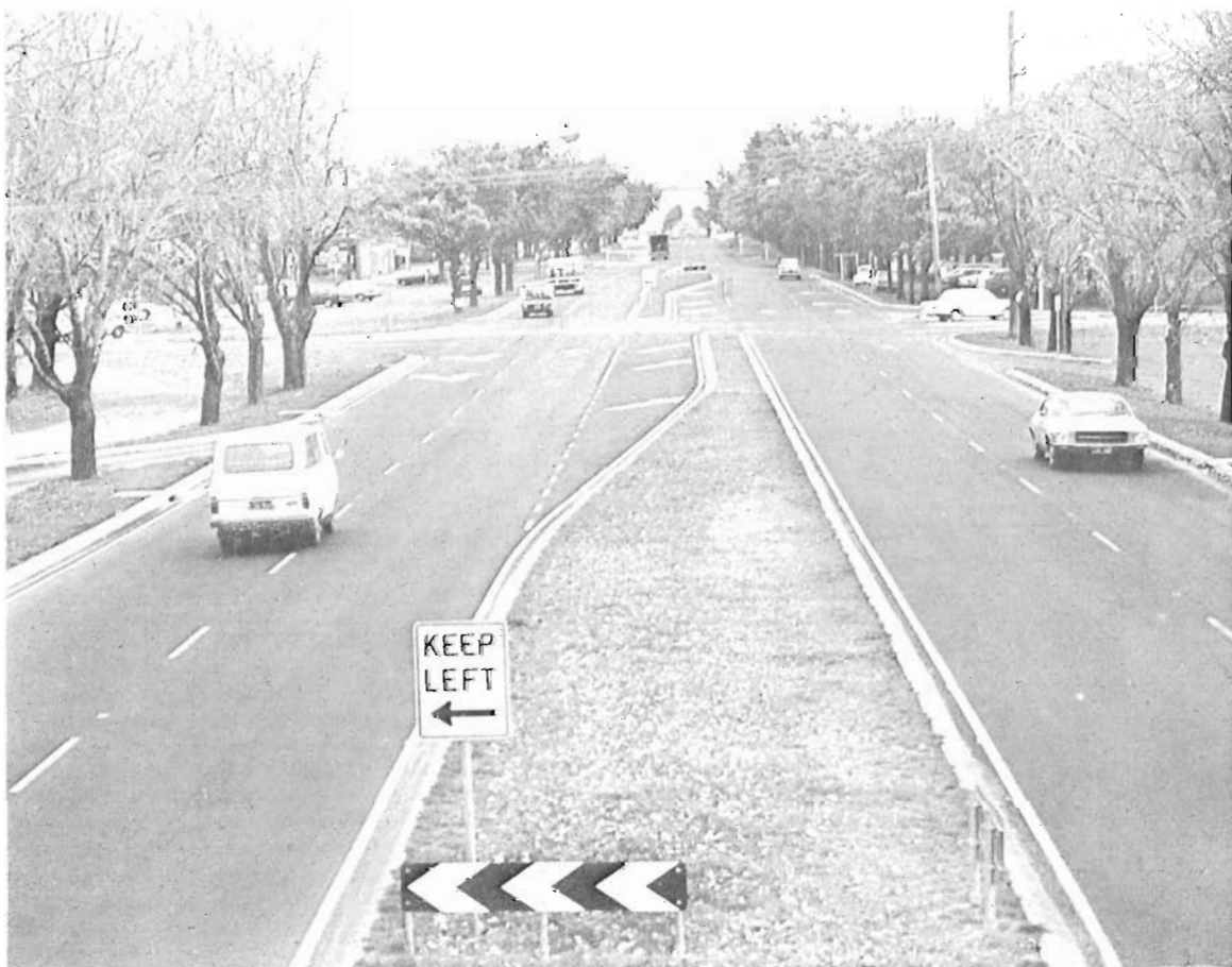
The Western Highway, reconstructed to provide dual carriageways at Ballarat West.
