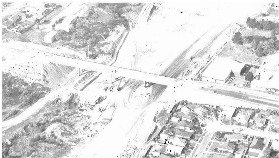
Bridge over the Mulgrave Freeway at Stephenson's Road.
