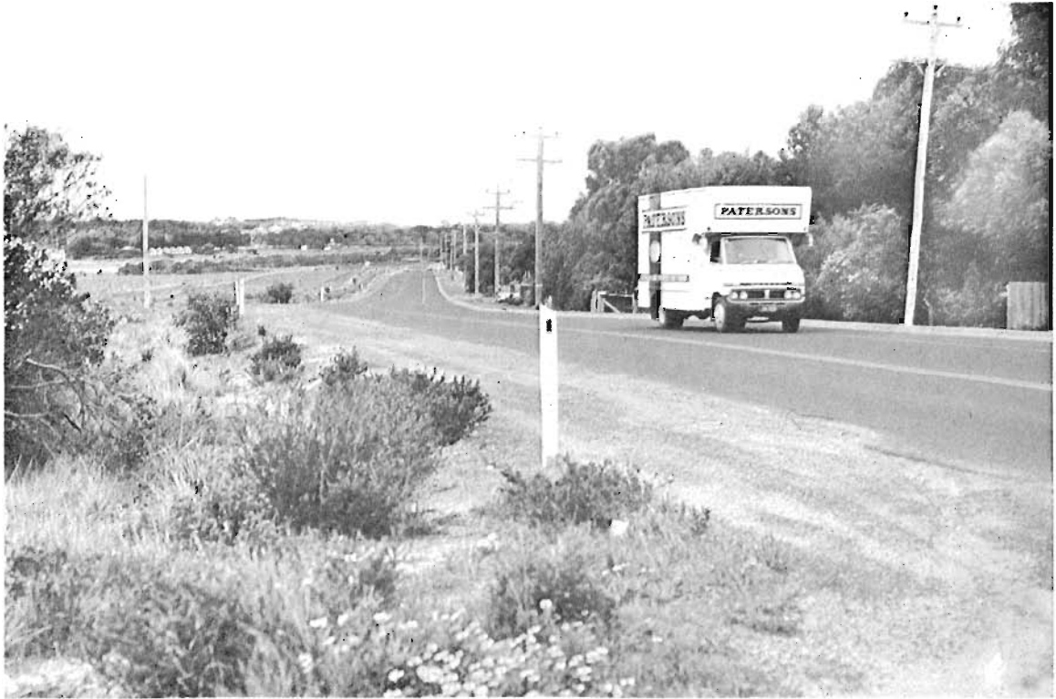
Reconstructed section of the Great Ocean Road west of Torquay.
