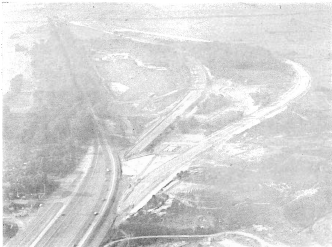
The Frankston Freeway under construction south of Eel Race Road, Seaford.
