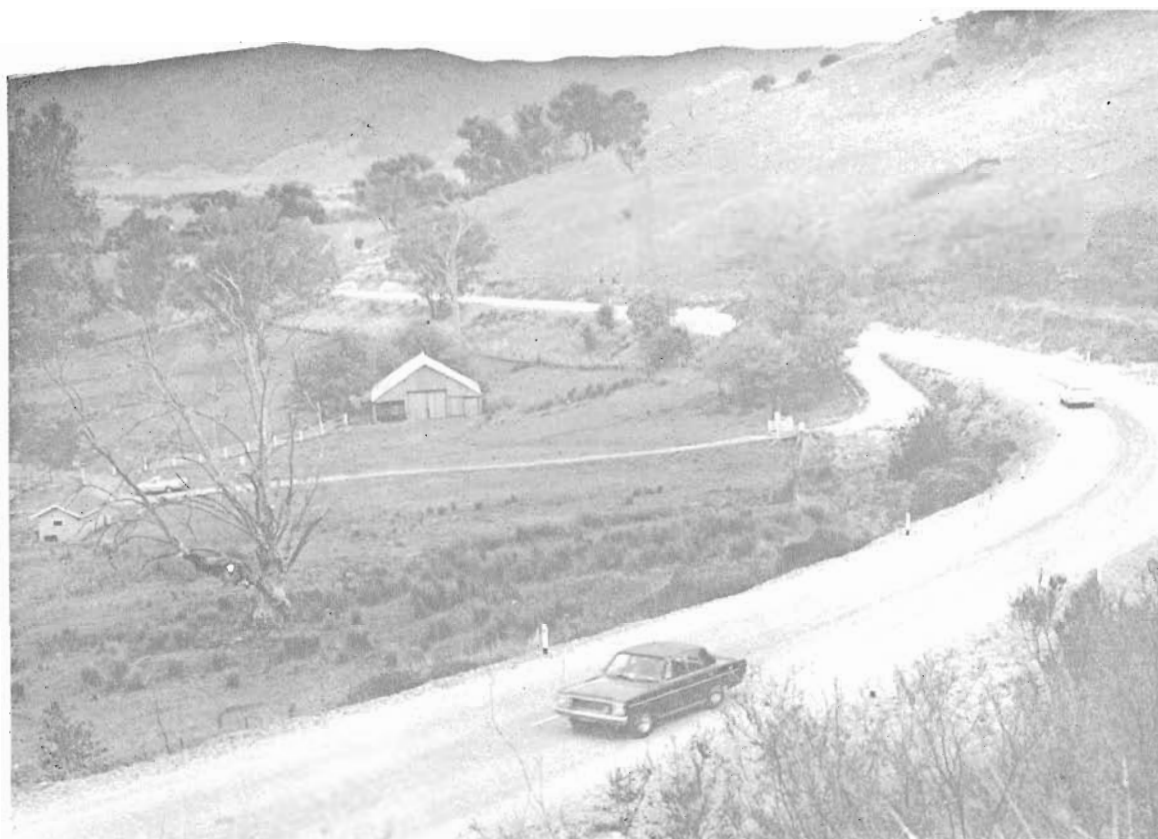
The Omeo Highway, reconstructed north of Noorongong.
