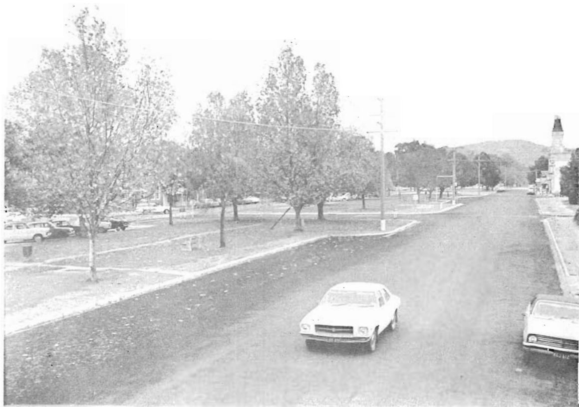
The Goulburn Valley Highway in Yea township—the west bound carriageway was reconstructed during the year.
