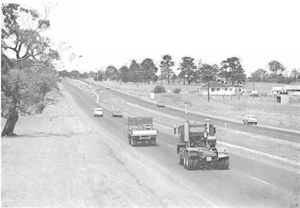
Dual carriageways constructed on the South Gippsland Highway.
