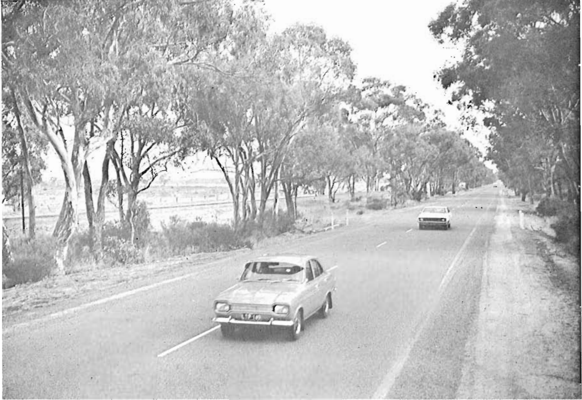
Section of the Calder Highway reconstructed near Kurting, between Bendigo and Charlton.
