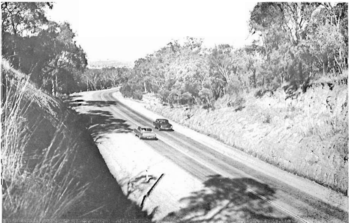
The Ballan-Daylestord Road, reconstructed in the Shire of Ballan.
