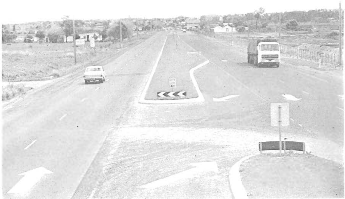
Dual carriageways constructed on the Geelong-Portarlington Road by the Bellarine Shire Council.
