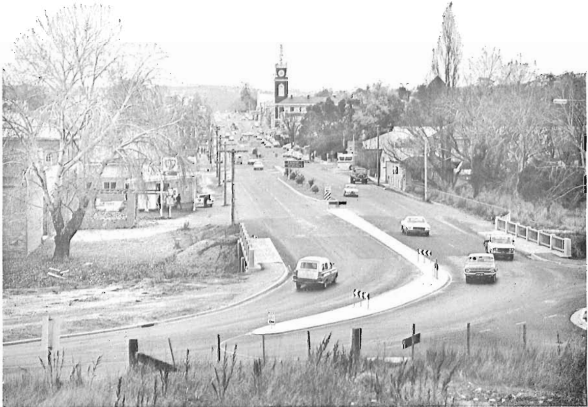
Midland Highway, Castlemaine City, reconstructed to provide dual carriageways.
