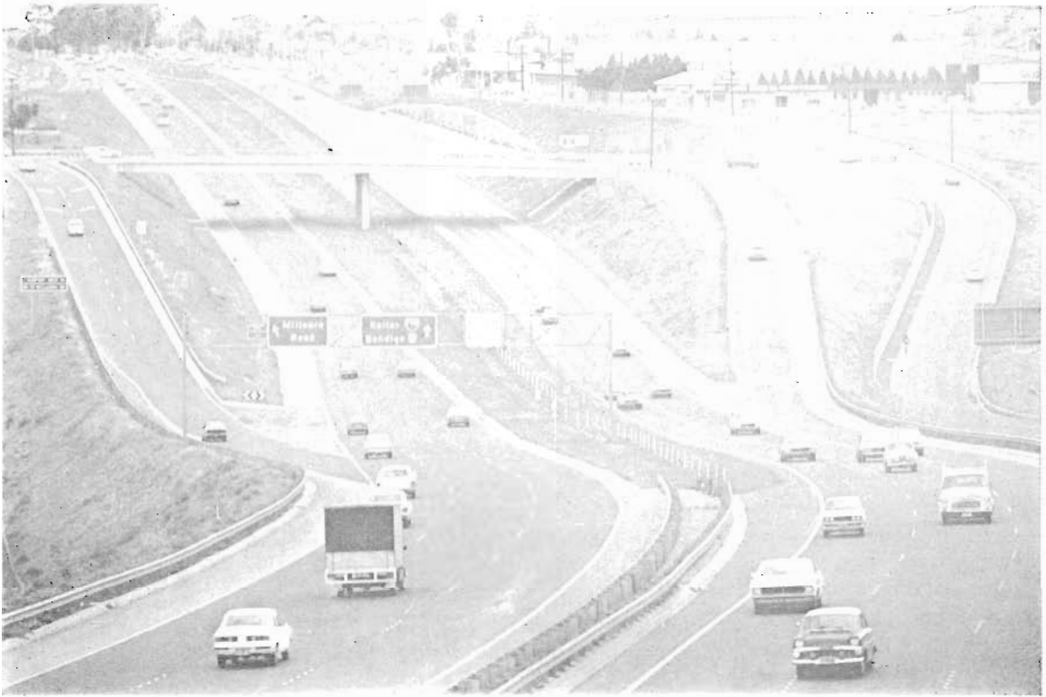
The Calder Freeway at Keilor East.
