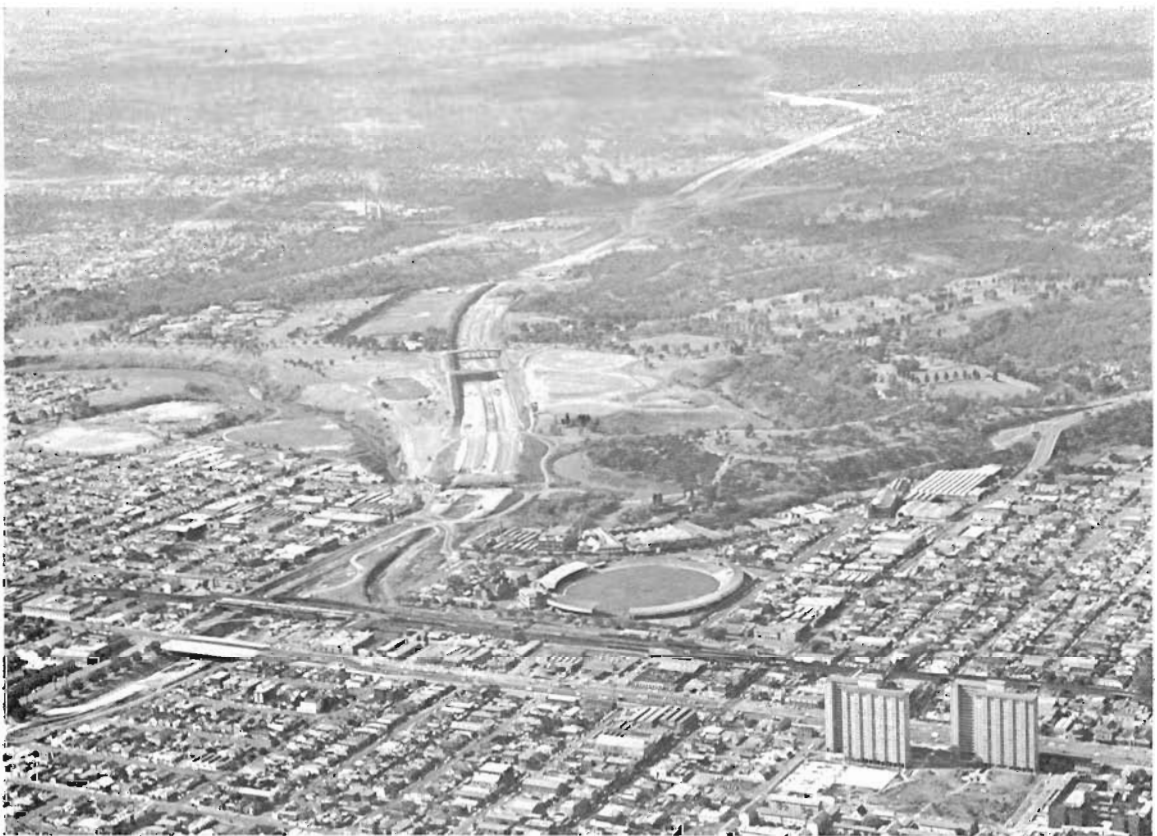
The Eastern Freeway under construction.
