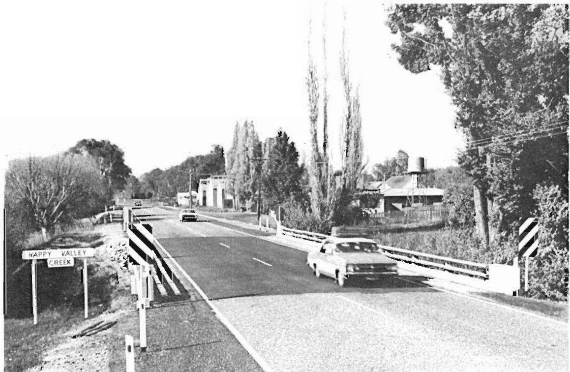
New reinforced concrete bridge on the Ovens Highway at Happy Valley Creek.
