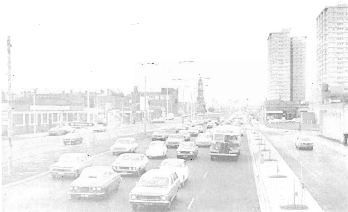
Dual carriageways provided on Hoddle Street, Collingwood.
