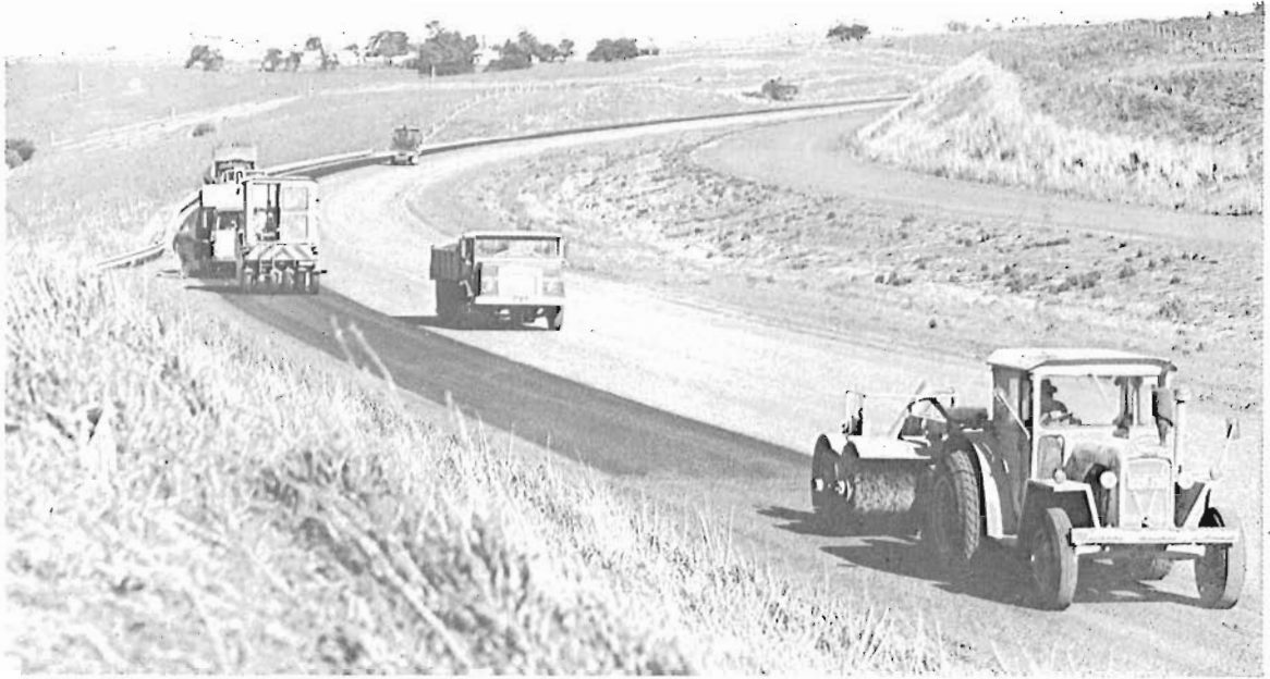
Work in progress on the Western Freeway (Myrning Section).
