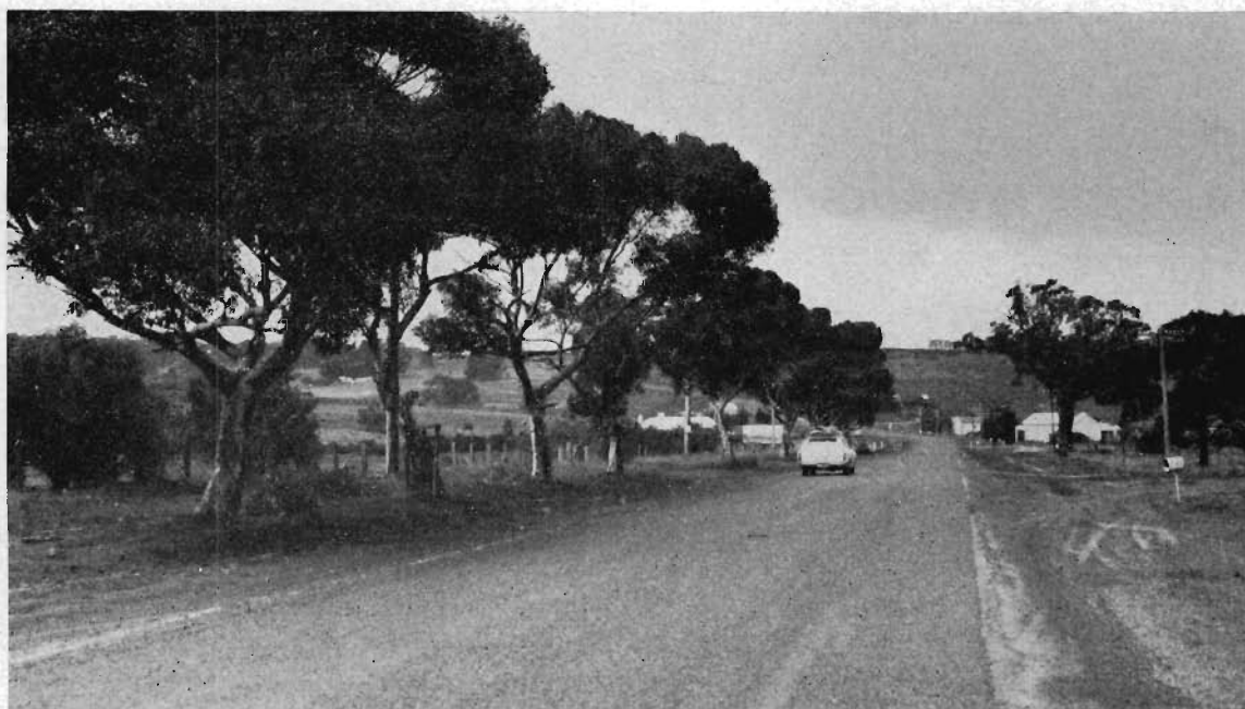
Reconstructed section of Cape Clear—Rokewood Road, Shire of Grenville.
