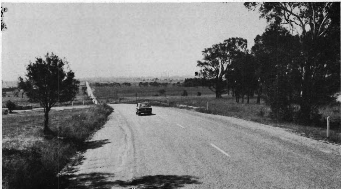
New construction on the Midland Highway deviation south of Morwell.
