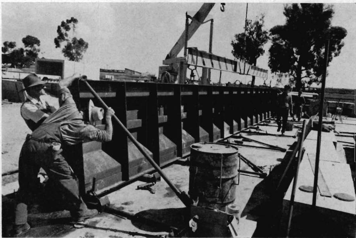
Plate 1—Setting up I-beam form.
