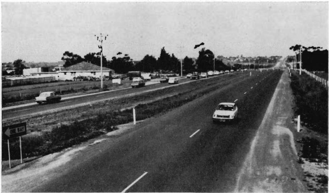
Dual carriageways on the Bellarine Highway between Moolap and Leopold.
