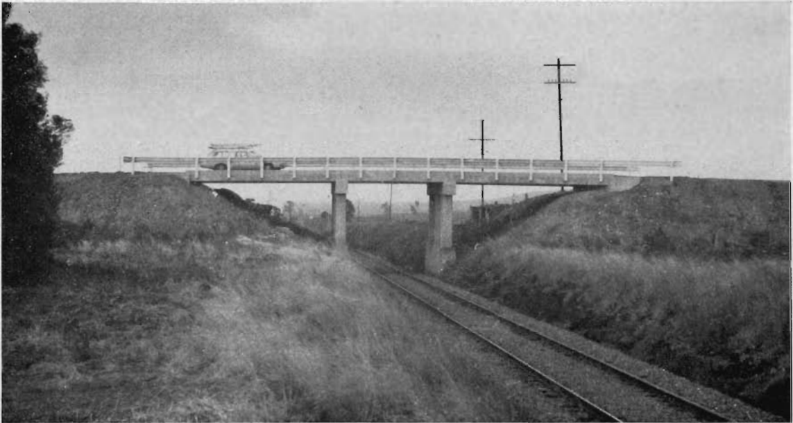
Moolort-Barringhup Road, Shire of Tullaroop. Bridge over railway at Moolort.
