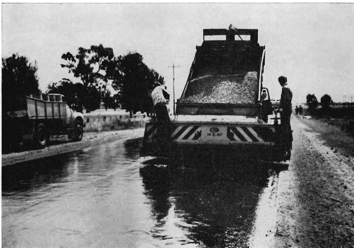
Spreading aggregate on a sprayed bitumen binder.
