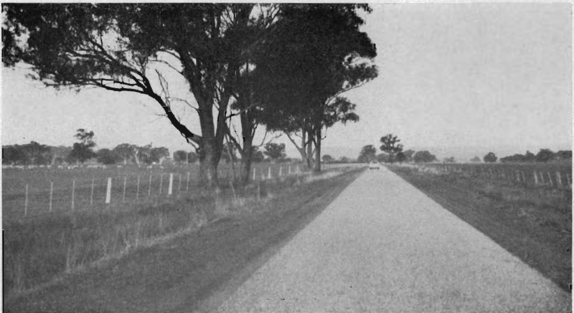
Reconstructed section of Devenish-Wangaratta Road north of Thoona, Shire of Benalla.
