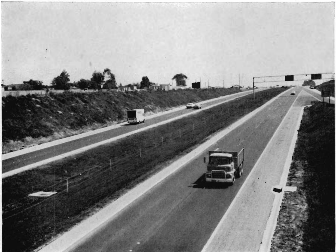
New section of the Calder Freeway at Keilor East.
