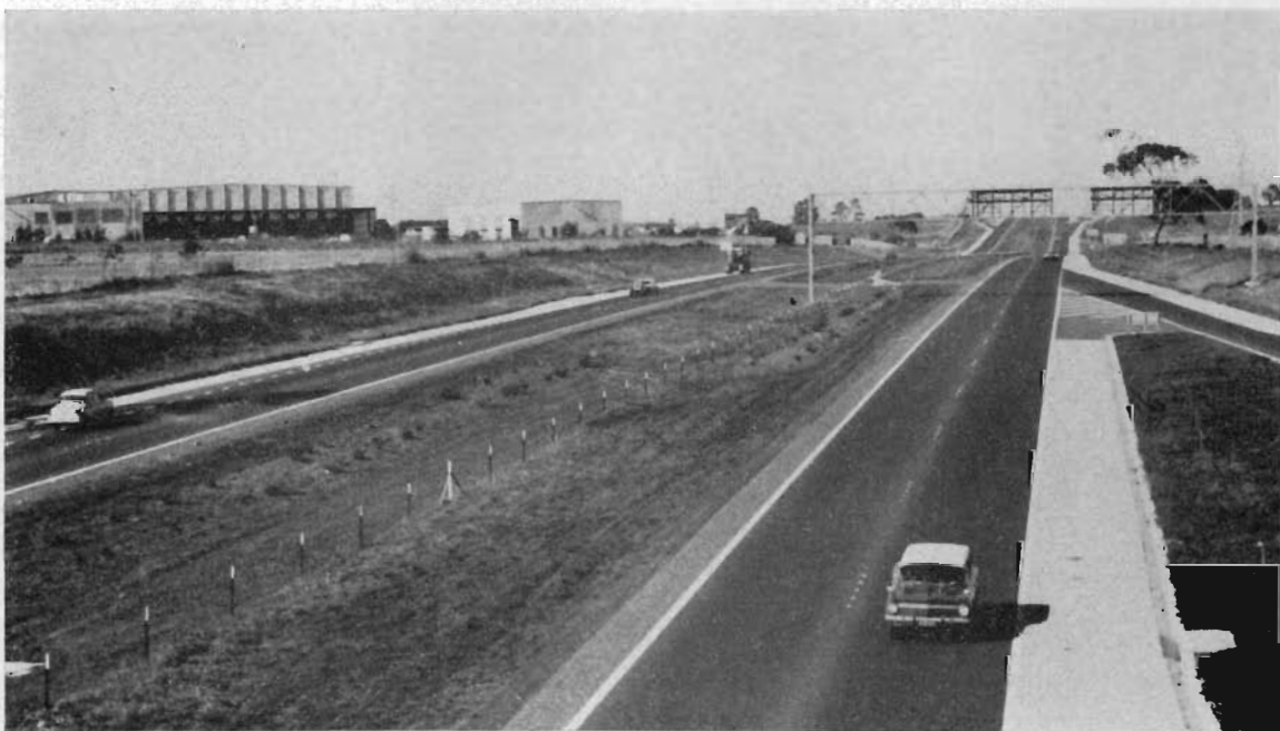
The Mulgrave Freeway south-east from Wellington Road.
