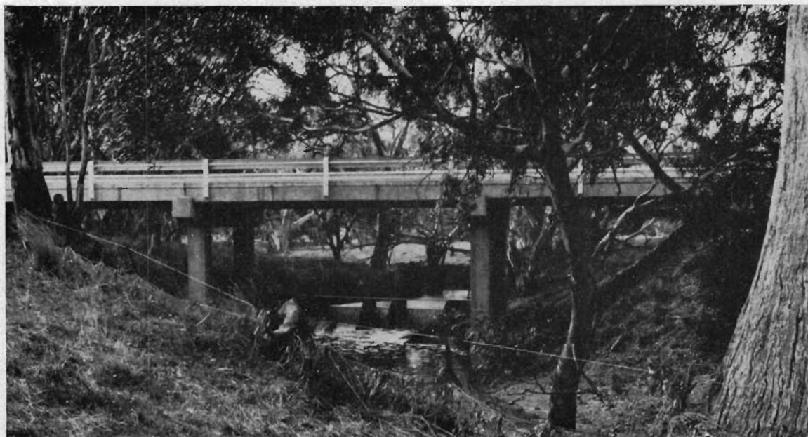
Bridge over Wattle Creek, Navarre-Wattle Creek Road, Shire of Avoca.
