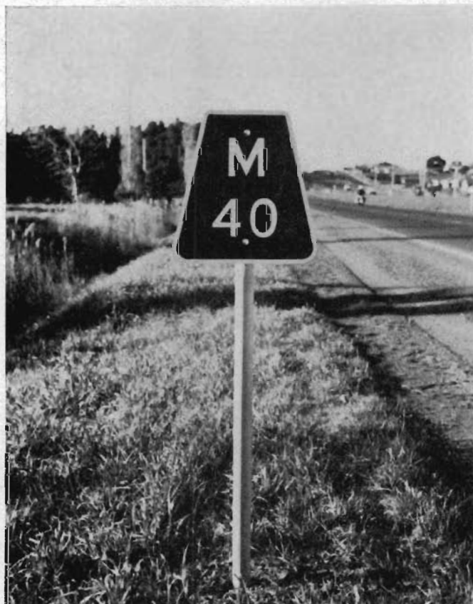
Distance markers to be erected at 5 km spacing.
