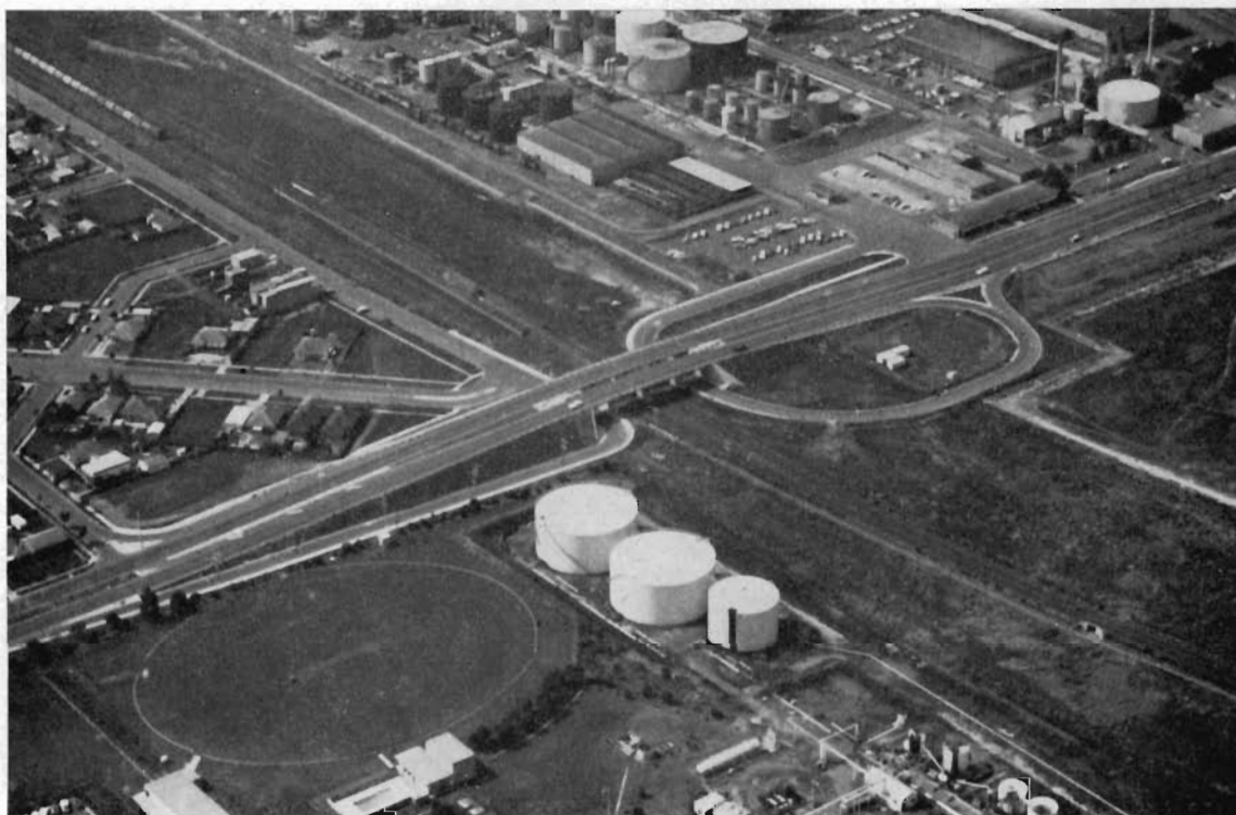
Road over rail overpass on Millers Road, Paisley.
