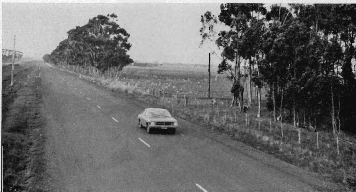
Hamilton Highway—reconstructed east of Lismore.
