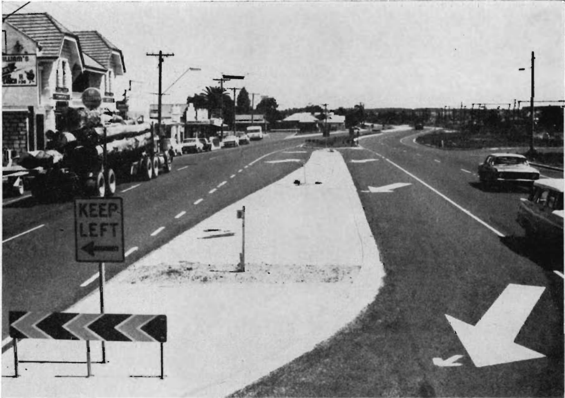
Dual carriageways on the Princes Highway East through Yarragon.
