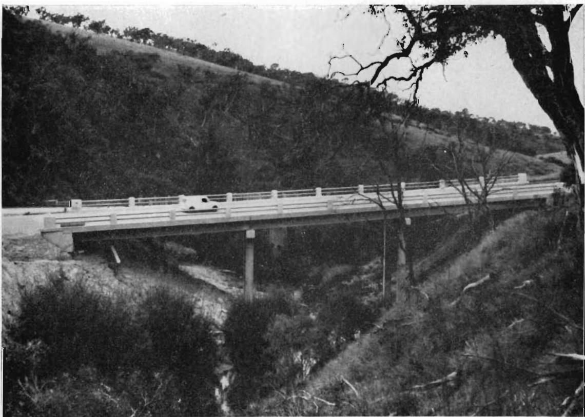
Bridge over Livingstone Creek, Day Avenue, Shire of Omeo.
