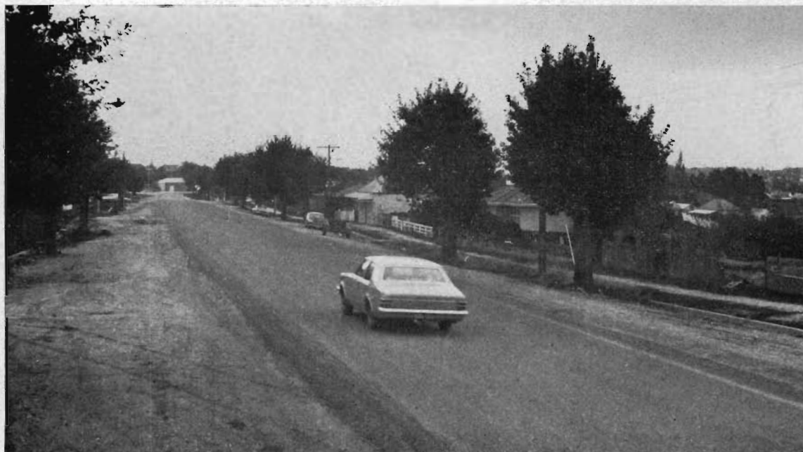
Reconstructed section of Creswick-Dean Road, Shire of Creswick.
