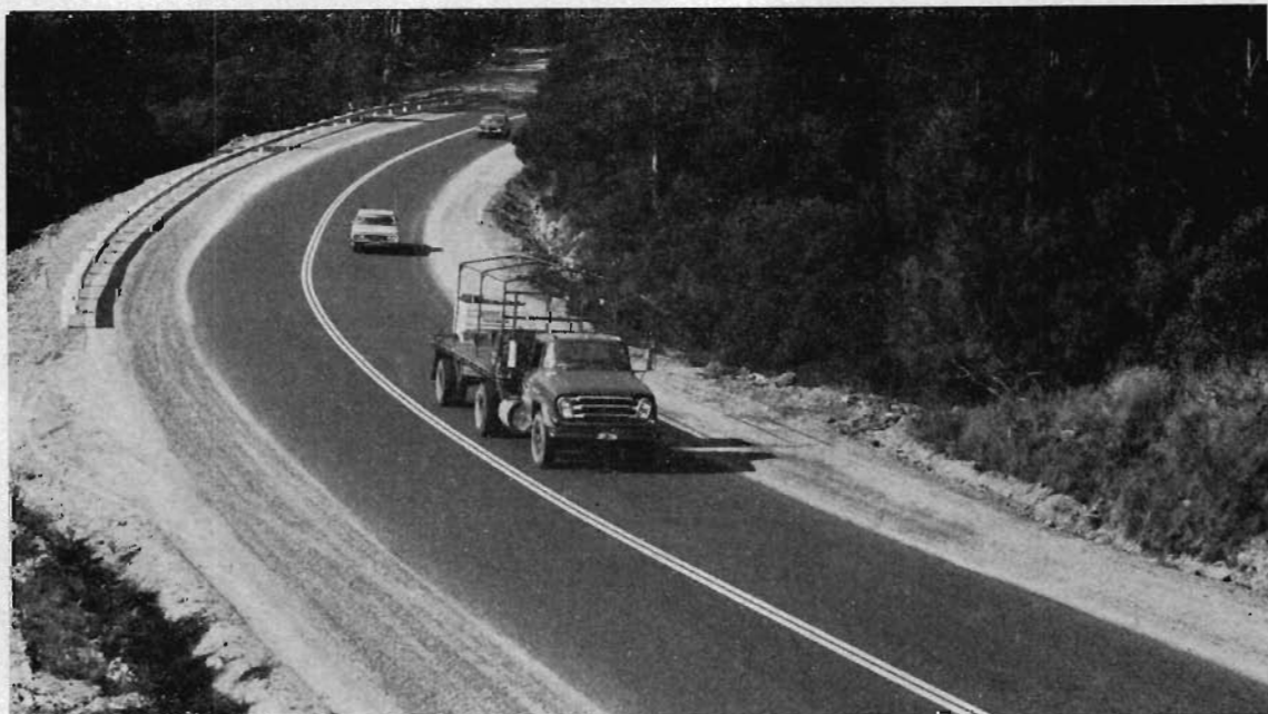
Reconstructed section of the South Gippsland Highway east of Korumburra.
