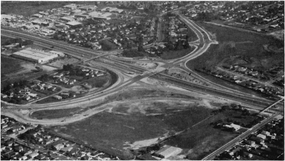
Seaford Road overpass of the Frankston Freeway during construction.
