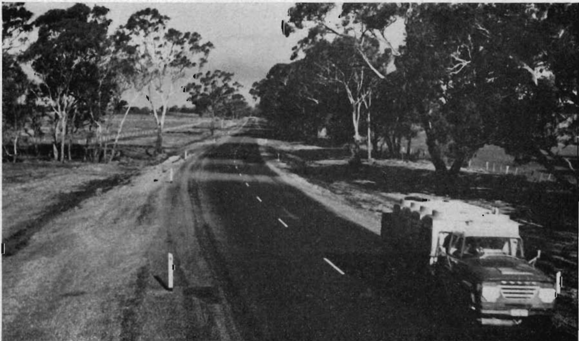
Reconstructed section of the Sunraysia Highway near Lamplough.
