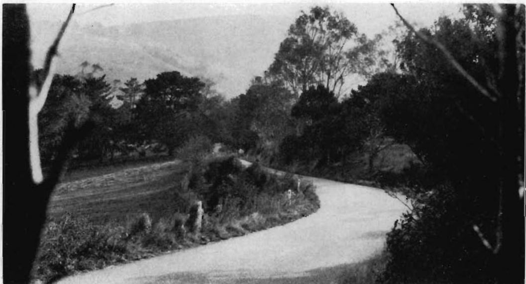
Reconstructed section of Kardella Road, Korumburra Shire.
