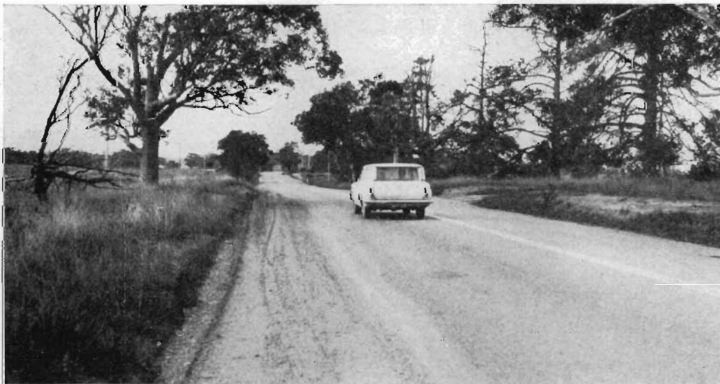
Reconstructed section of the Princes Highway east of Nicholson River.
