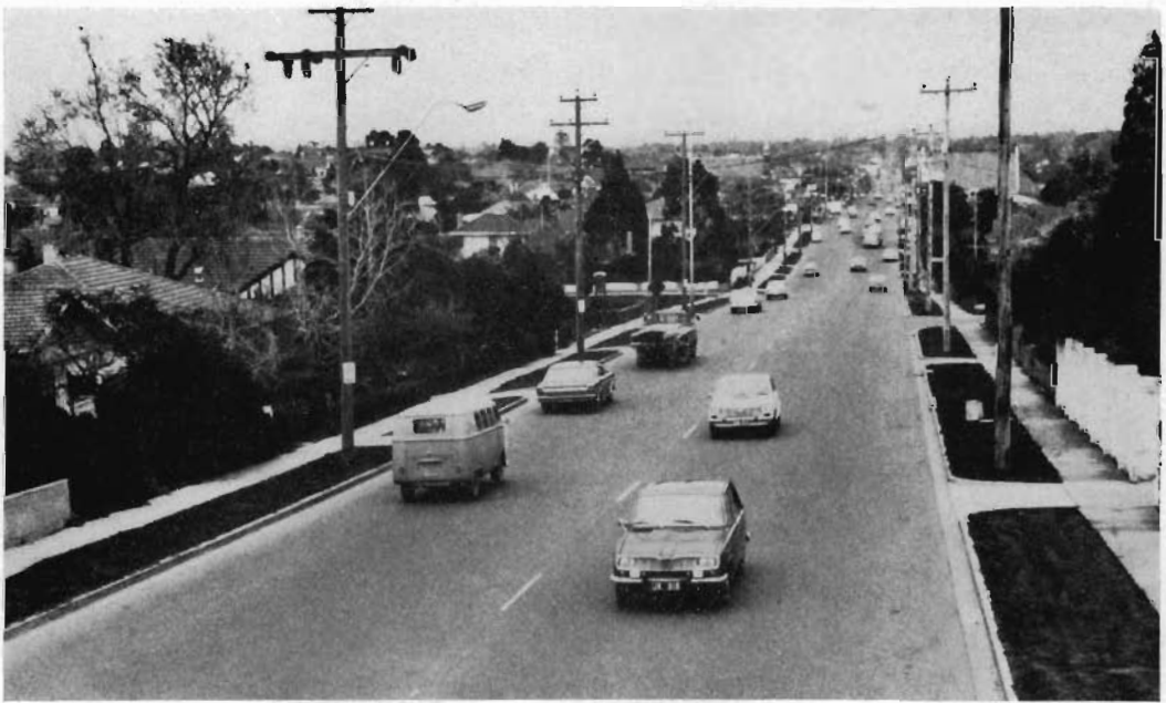
Reconstructed section of Canterbury Road east of Warrigal Road, Box Hill City.
