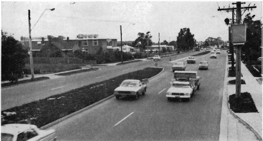
Dual carriageways constructed on Blackburn Road, Nunawading City.
