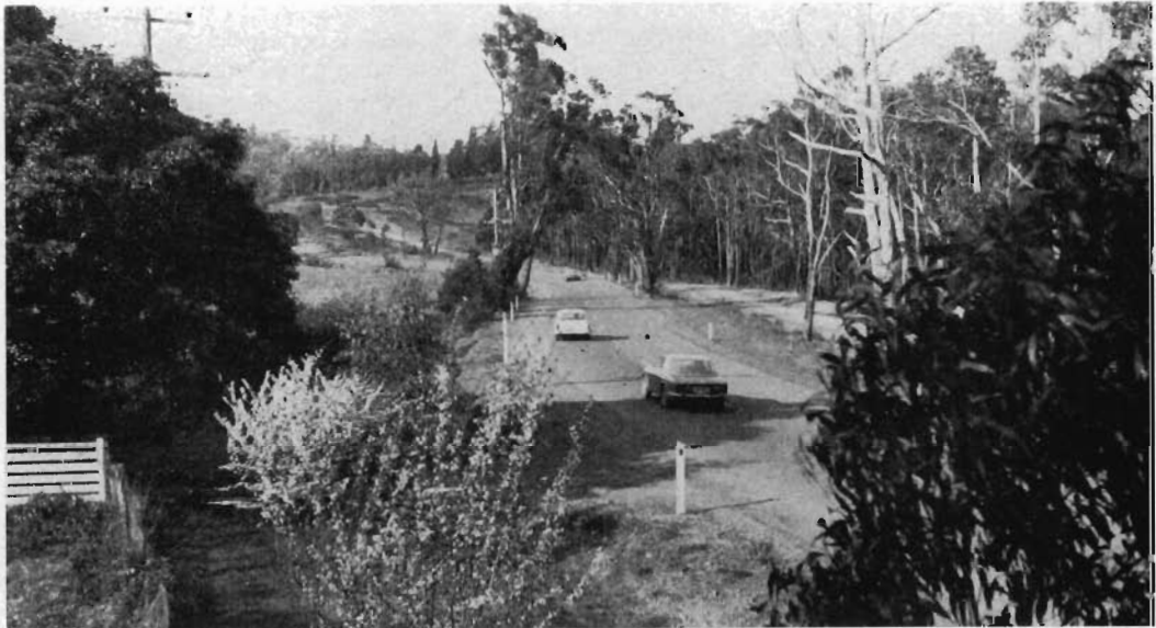
Beaconsfield-Emerald Road reconstructed north of Upper Beaconsfield, Berwick Shire.
