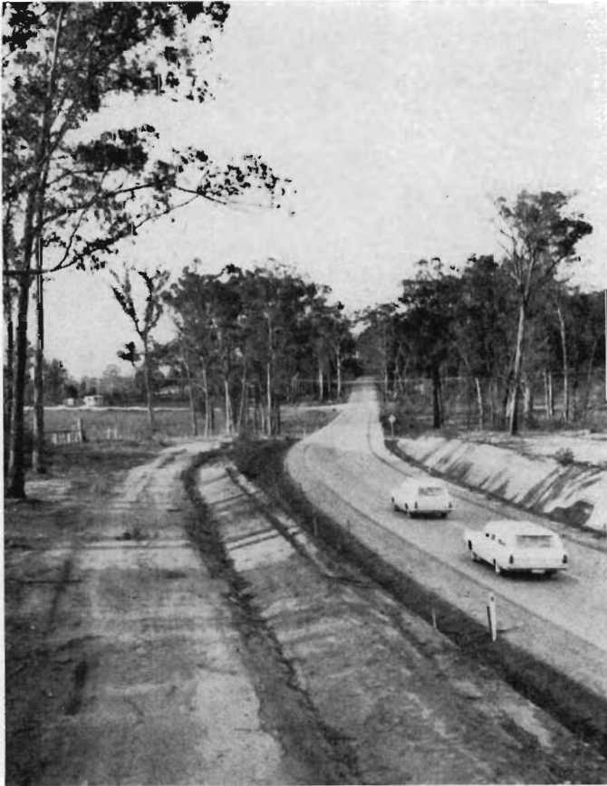
Reconstructed section of the Bruthen-Buchan Road, Tambo Shire.
