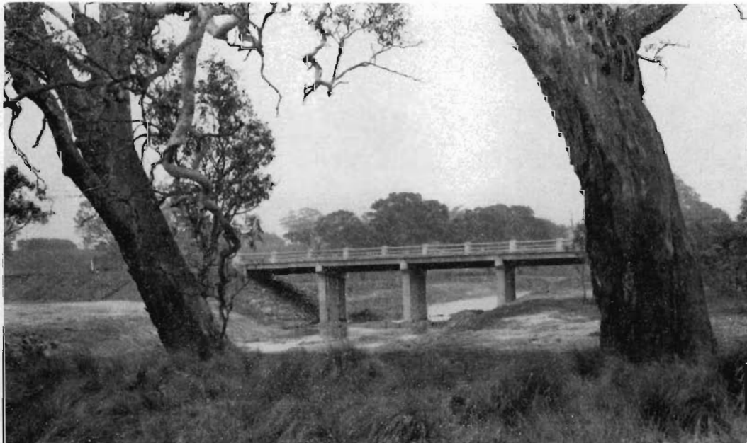
New bridge over the Dundas River — Cavendish-Coleraine Road, Dundas Shire.
