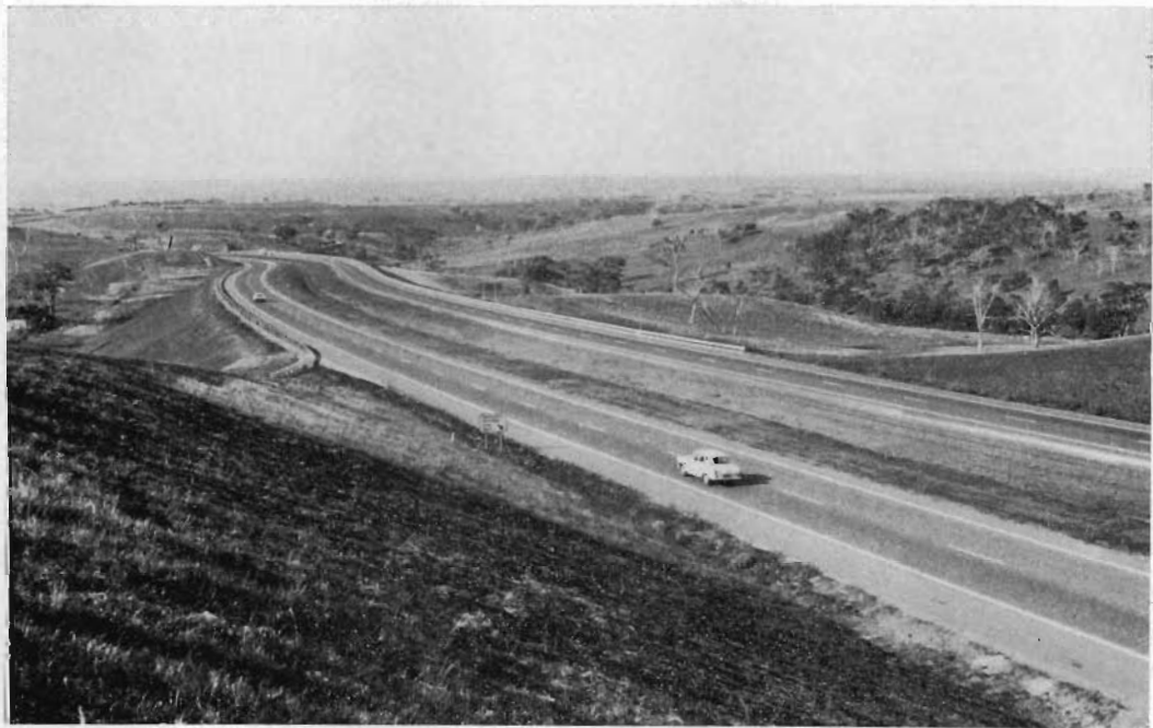
Newly completed section of the Western Freeway (Pentland Hills Section).
