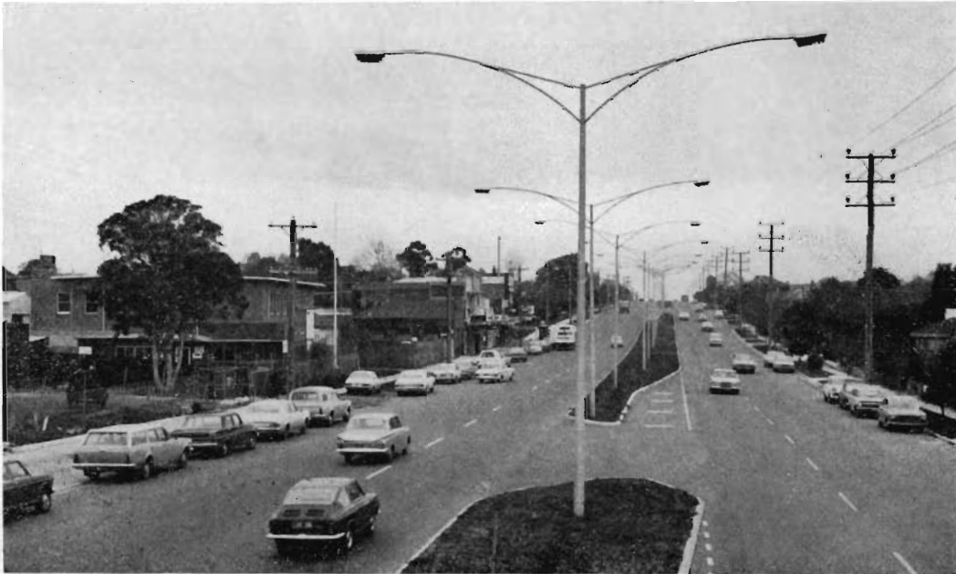
Dual carriageways on North Road between Bambra Road and Booran Road, Caulfield City.
