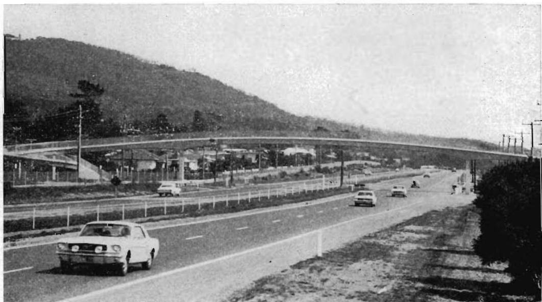
Mornington Peninsula Freeway — pedestrian overpass constructed at Pier Street, Dromana.
