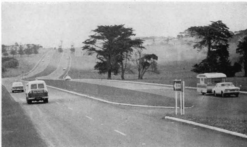
Dual carriageways constructed on the Princes Highway West near Warrnambool.
