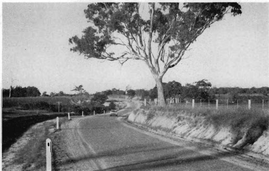
Reconstructed section of the Rosedale-Longford Road (unclassified), Rosedale Shire.
