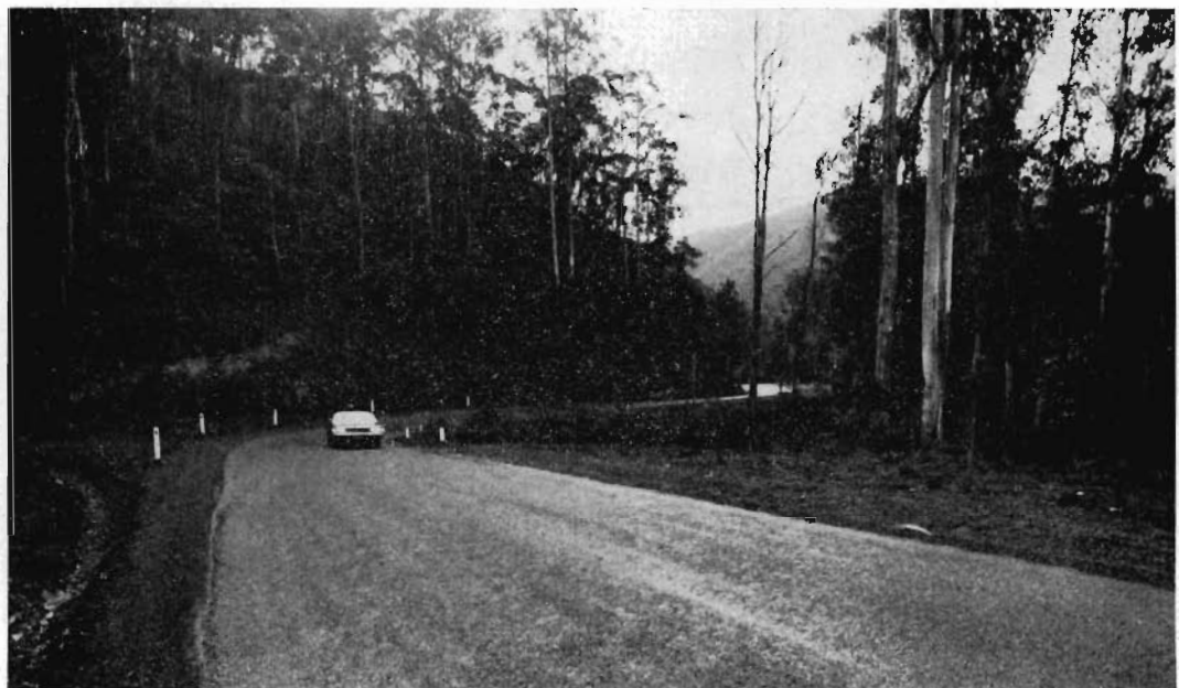
Walhalla Forest Road — reconstructed section north of Erica.
