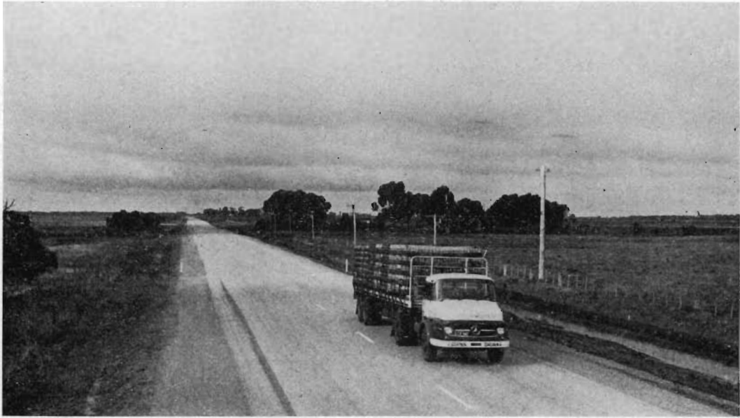
Reconstructed section of the Loddon Valley Highway at Durham Ox.
