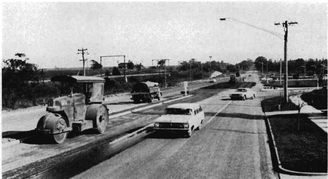
The Princes Highway East — dual carriageways under construction at Traralgon.
