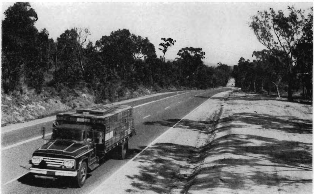
Climbing lane constructed on the Hume Highway at Teneriffe Hill.
