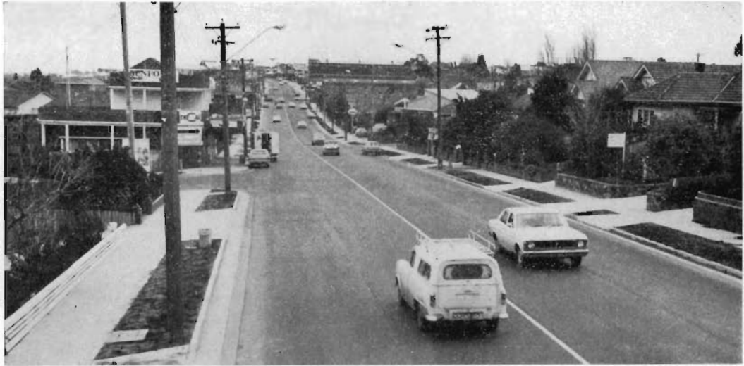
Whittlesea Road reconstructed between Tyler Street and Albert Street, Preston City.
