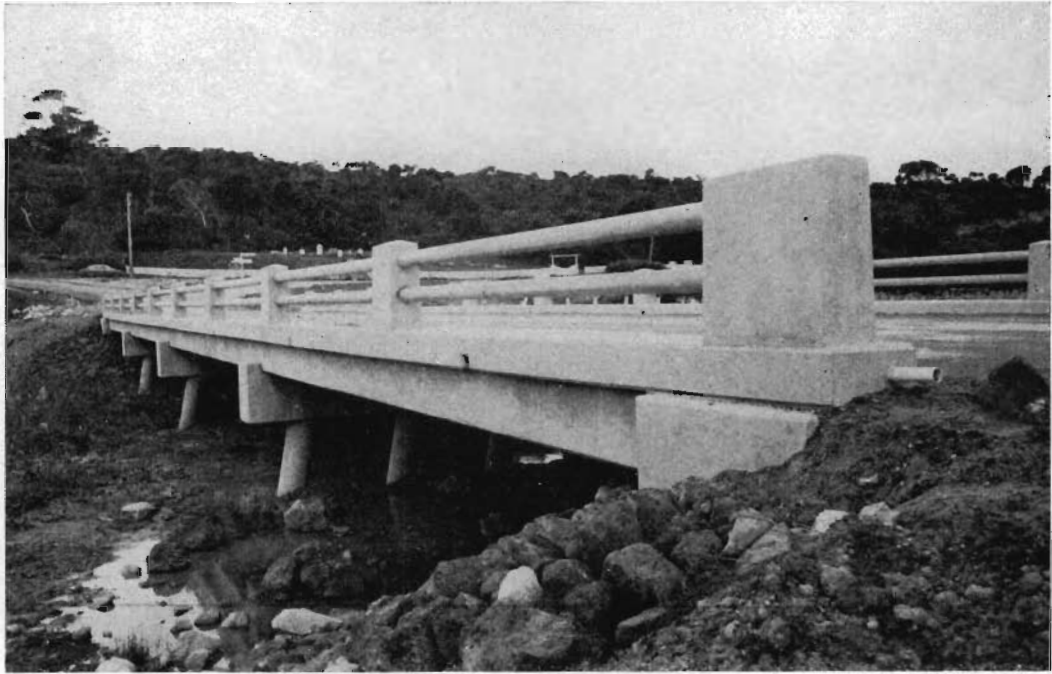
New bridge over Port Campbell Creek on the Great Ocean Road.
