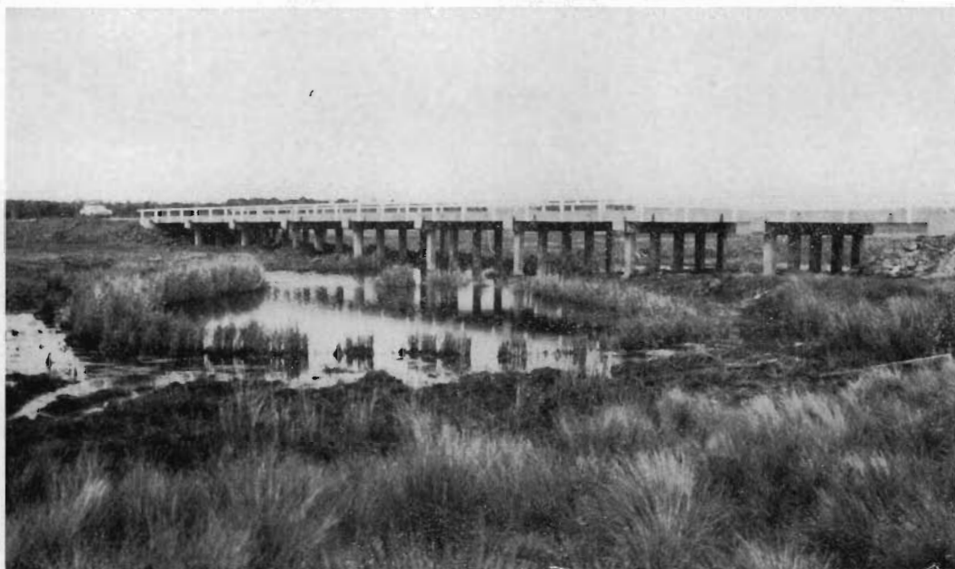
Delacombe Way, Shire of Ararat — new bridge over Hopkins River.
