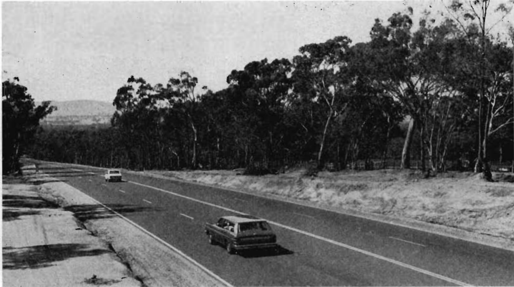
Additional lanes constructed on the Hume Highway at Tubbs Hill.
