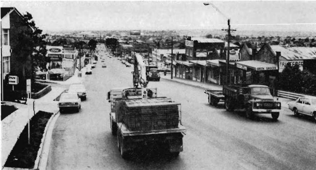
Reconstructed section of Bell Street between Waterdale Road and Upper Heidelberg Road, City of Heidelberg.
