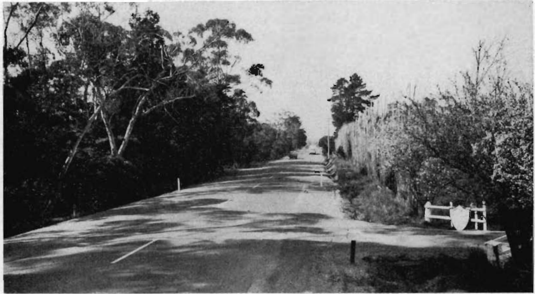
Tyabb-Mornington Road — reconstructed section in Hastings Shire.
