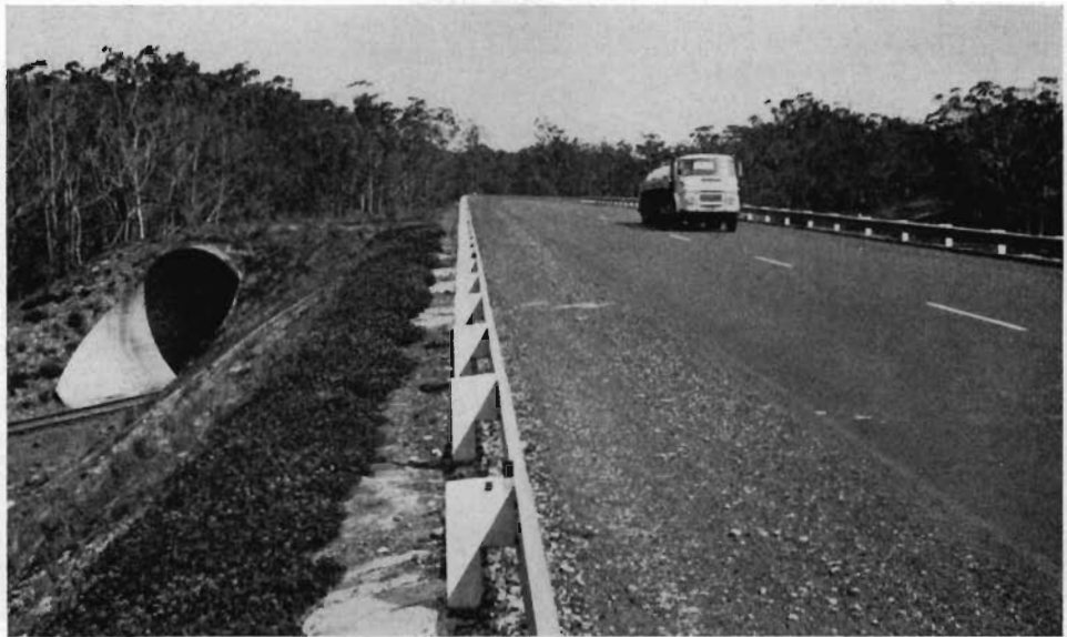
Princes Highway West—railway level crossing eliminated at Lyons.
