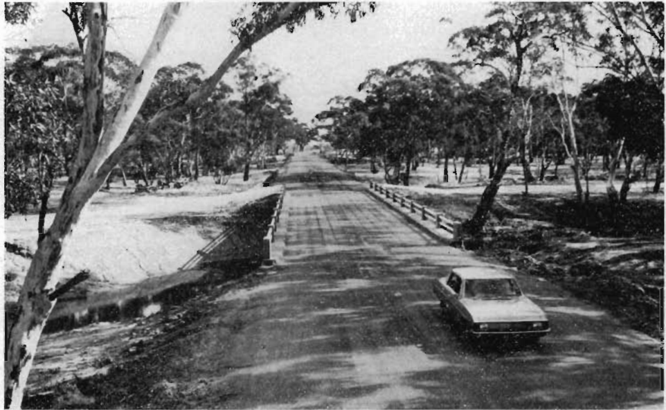
New bridges over the Wimmera River and Mount William Creek on Horsham-Lubeck Road, Shires of Dunmunkle and Wimmera.
