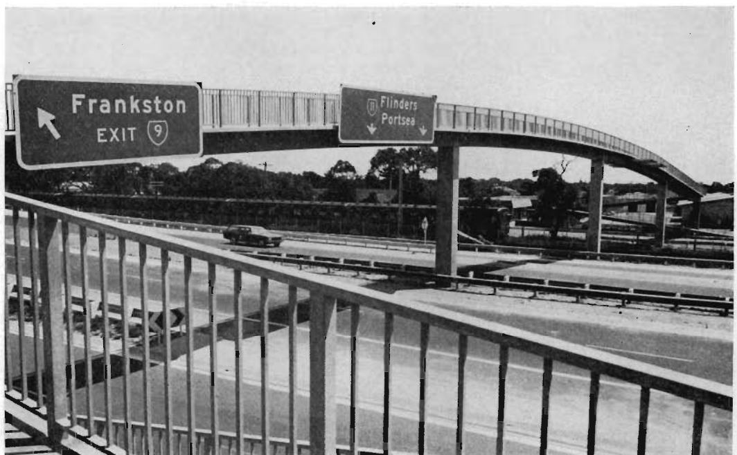
Pedestrian overpass of the Frankston Freeway serving Kananook Primary School.
