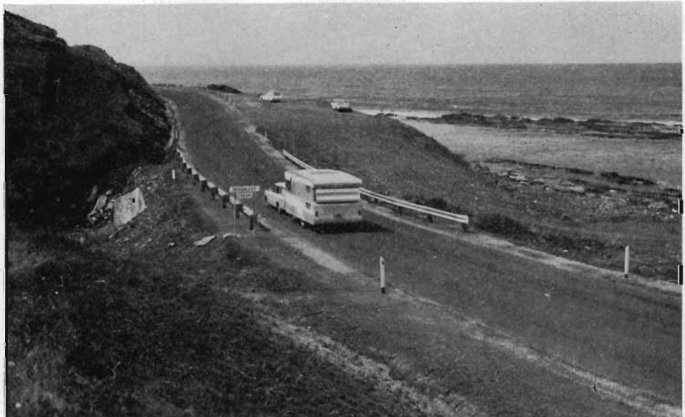
New bridge on the Great Ocean Road at Boggaley Creek.
