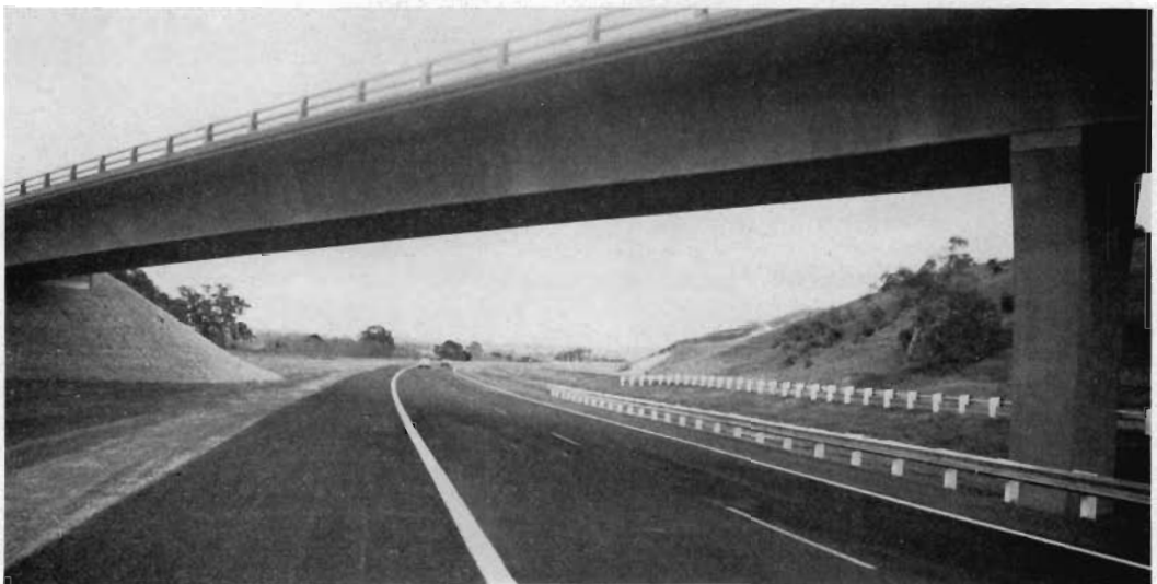
The Western Freeway (Bacchus Marsh Section) at the eastern interchange.
