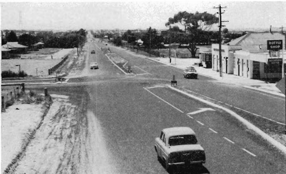
Dual carriageways constructed on the Torquay Road, Shire of South Barwon.
