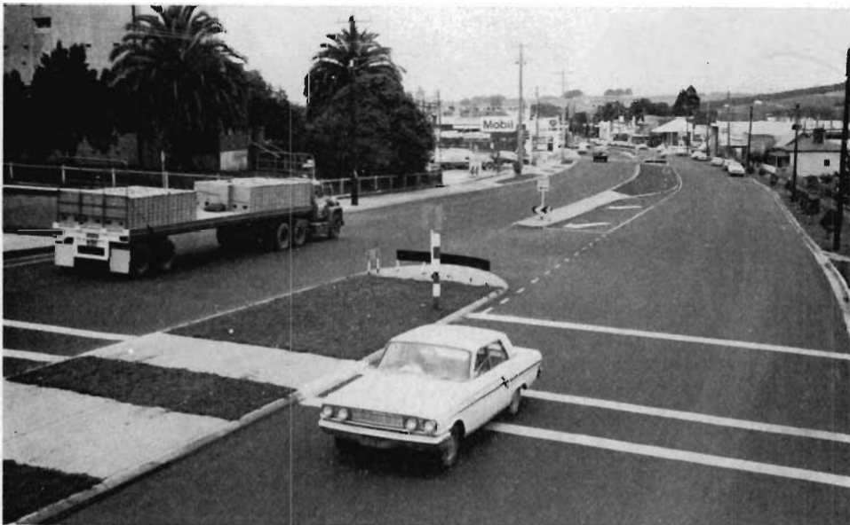
Dual carriageways constructed on the Princes Highway East in Warragul.
