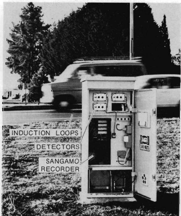
Plate 2—Typical urban counter installation.
