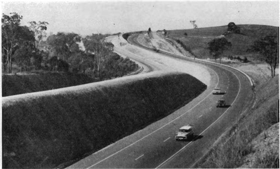
Dual carriageways constructed on the Princes Freeway between Gunns Gully and Hernes Oak.
