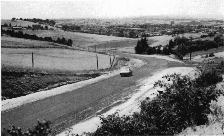
Reconstructed section of Barrabool Road, Shire of Barrabool.
