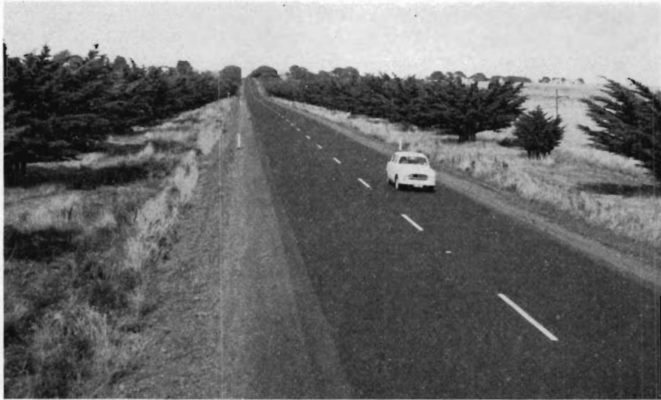
Hamilton Highway—reconstruction east of Mortlake.
