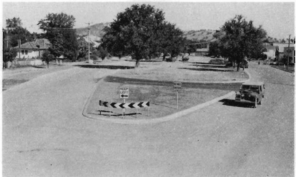
Dual carriageways constructed on the Midland Highway in Mansfield.
