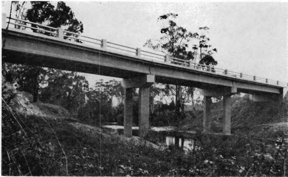
Omco Highway bridge over the Nicholson River.
