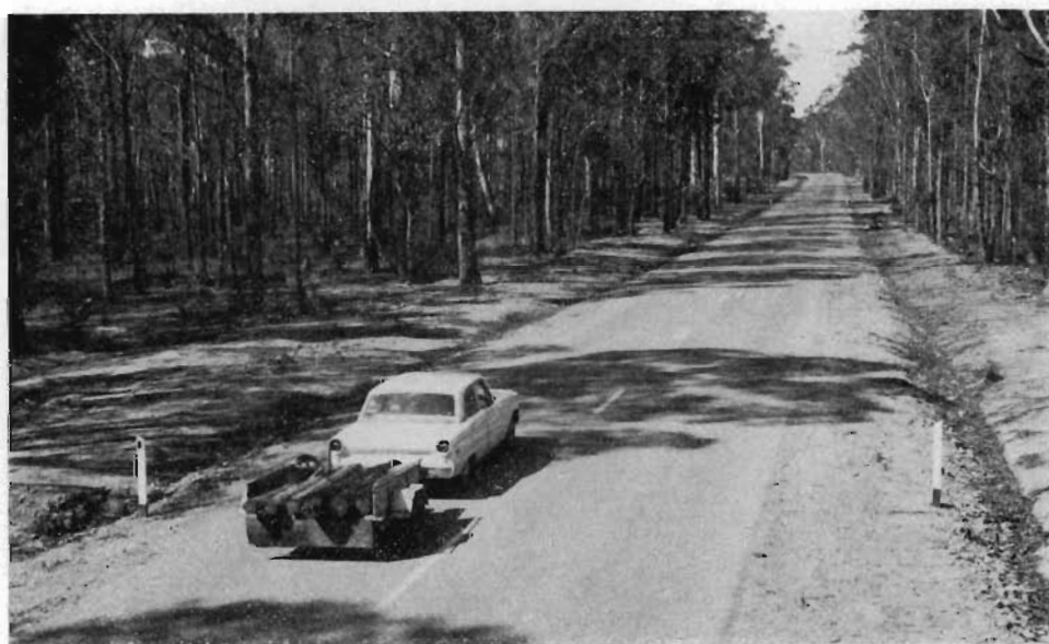
Reconstructed section of the Bonang Highway at Orbost.
