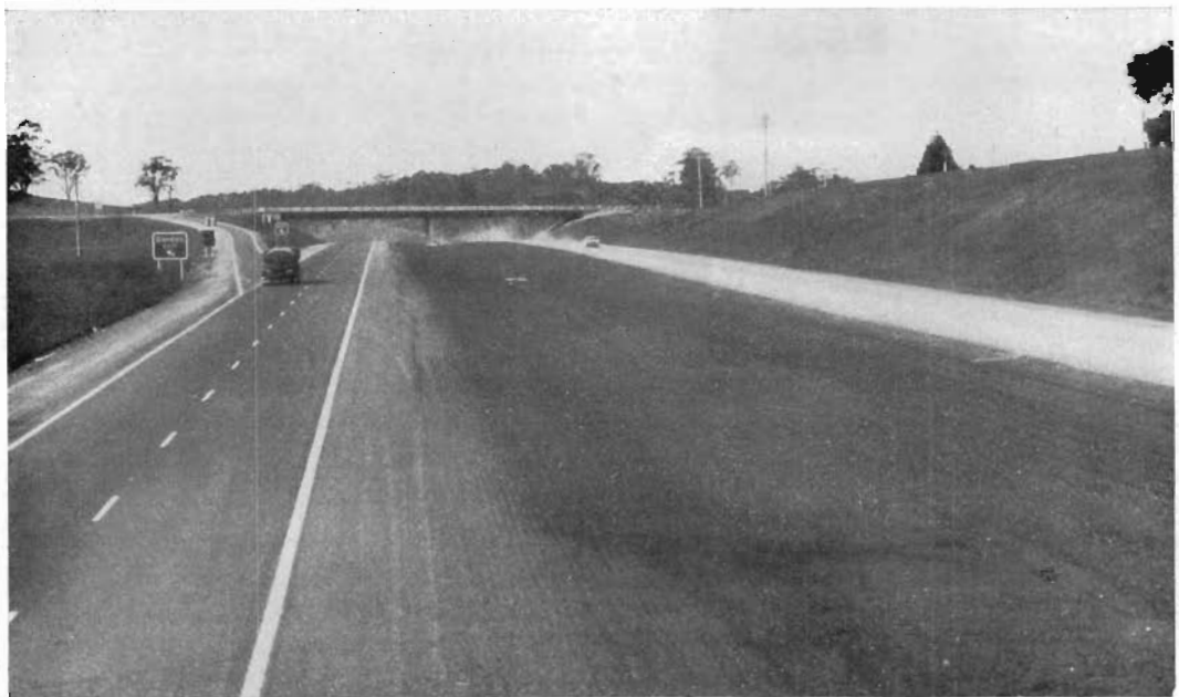
The Western Freeway (Gordon Section) in the vicinity of the Moorabool West Road interchange.
