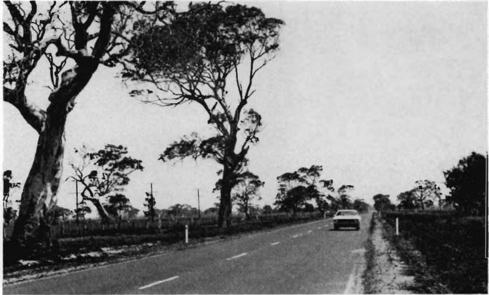
Reconstructed section of the Glenelg Highway west of Strathdownie.
