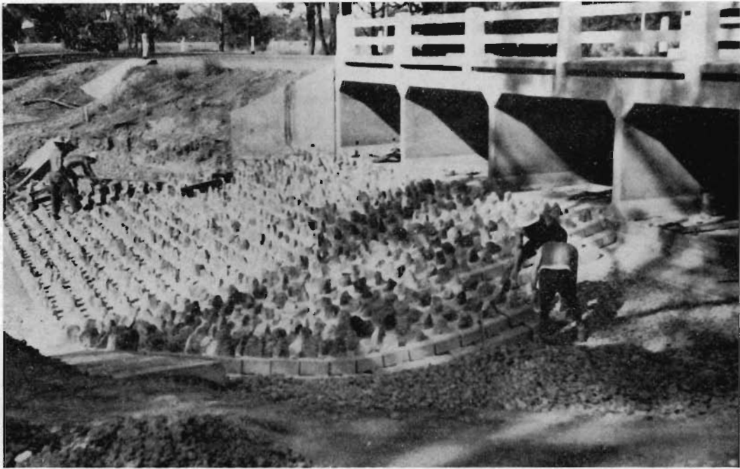
Plate 6—Placing the dissipator blocks.
