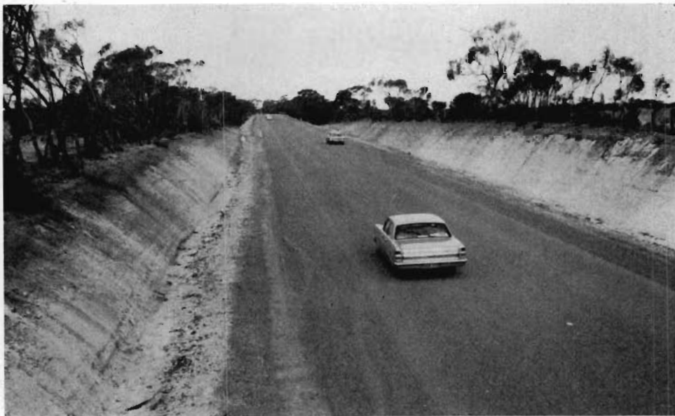
Reconstructed section of the Calder Highway north of Glenalbyn.
