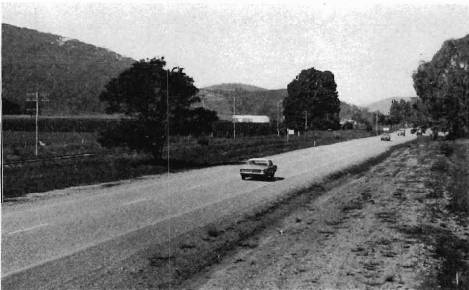
Reconstructed section of the Ovens Highway near Eurobin.
