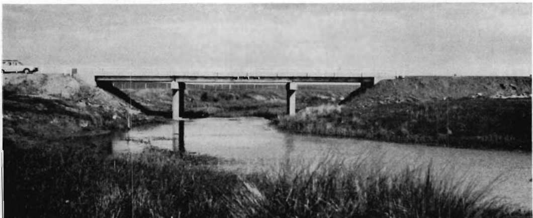
Bridge over the Hopkins River, Calvert Road, Shire of Ararat.
