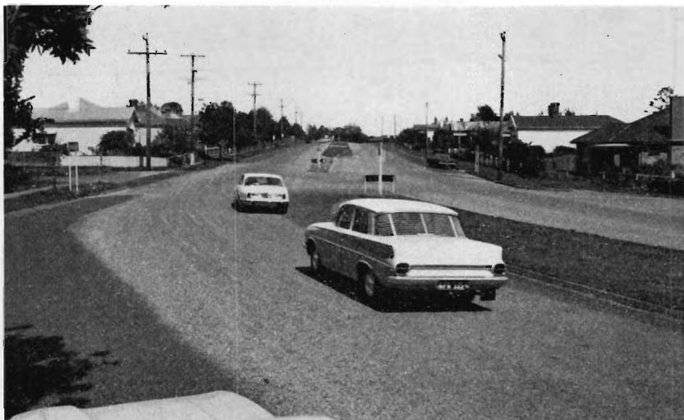
Dual carriageways constructed on the Henty Highway in the City of Hamilton.
