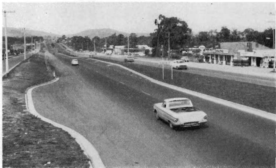
Dual carriageways constructed on the Burwood Highway, City of Knox.
