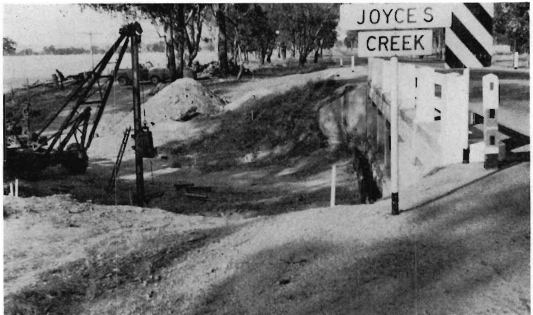
Plate 4—Hume Highway—Joyce's Creek. Driving steel sheet-piling for a cut-off wall.
