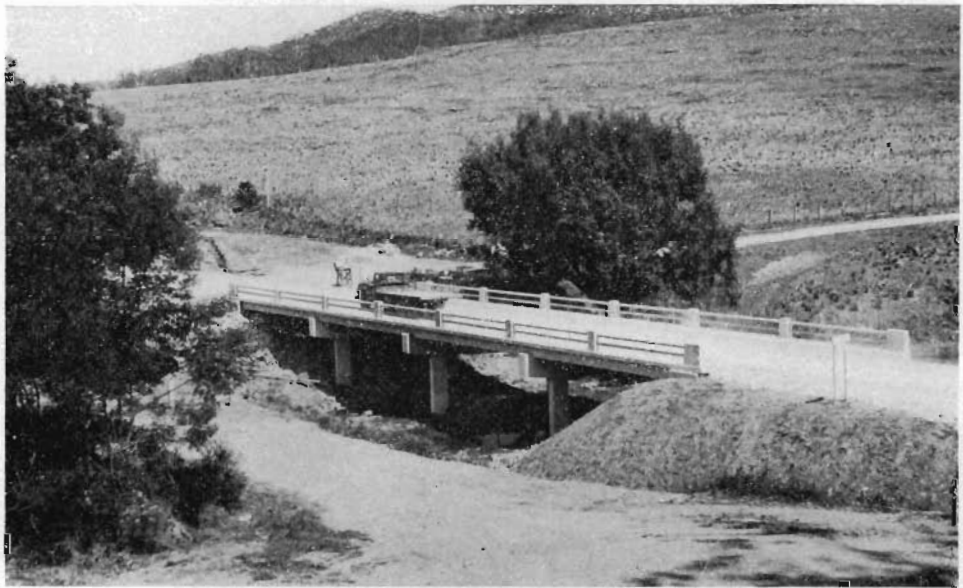
New bridge on Gelantipy Road at Murrindal River, Shire of Tambo.
