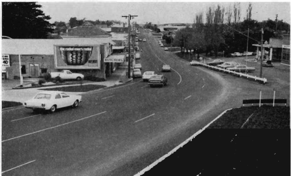
Reconstructed section of the Princes Highway East in Drouin.
