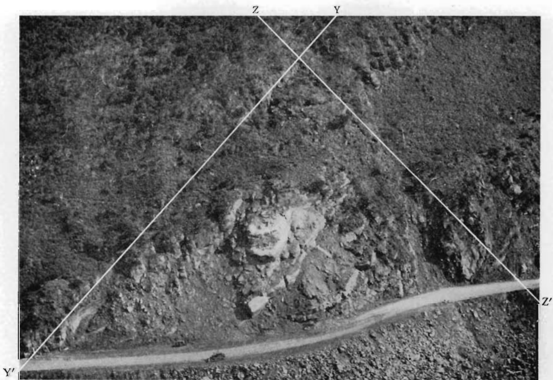
Plate 13—The Windy Point landslide. Y - Y' and Z - Z' indicate the major fissures which form the boundaries of the slide area.
