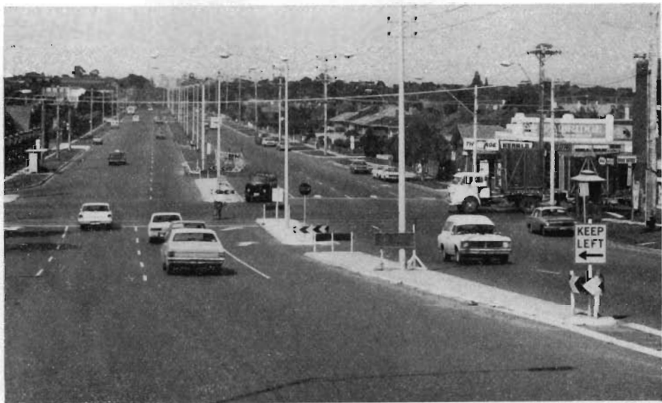
Dual carriageways constructed on North Road, east of Hawthorn Road, Cities of Brighton and Caulfield.
