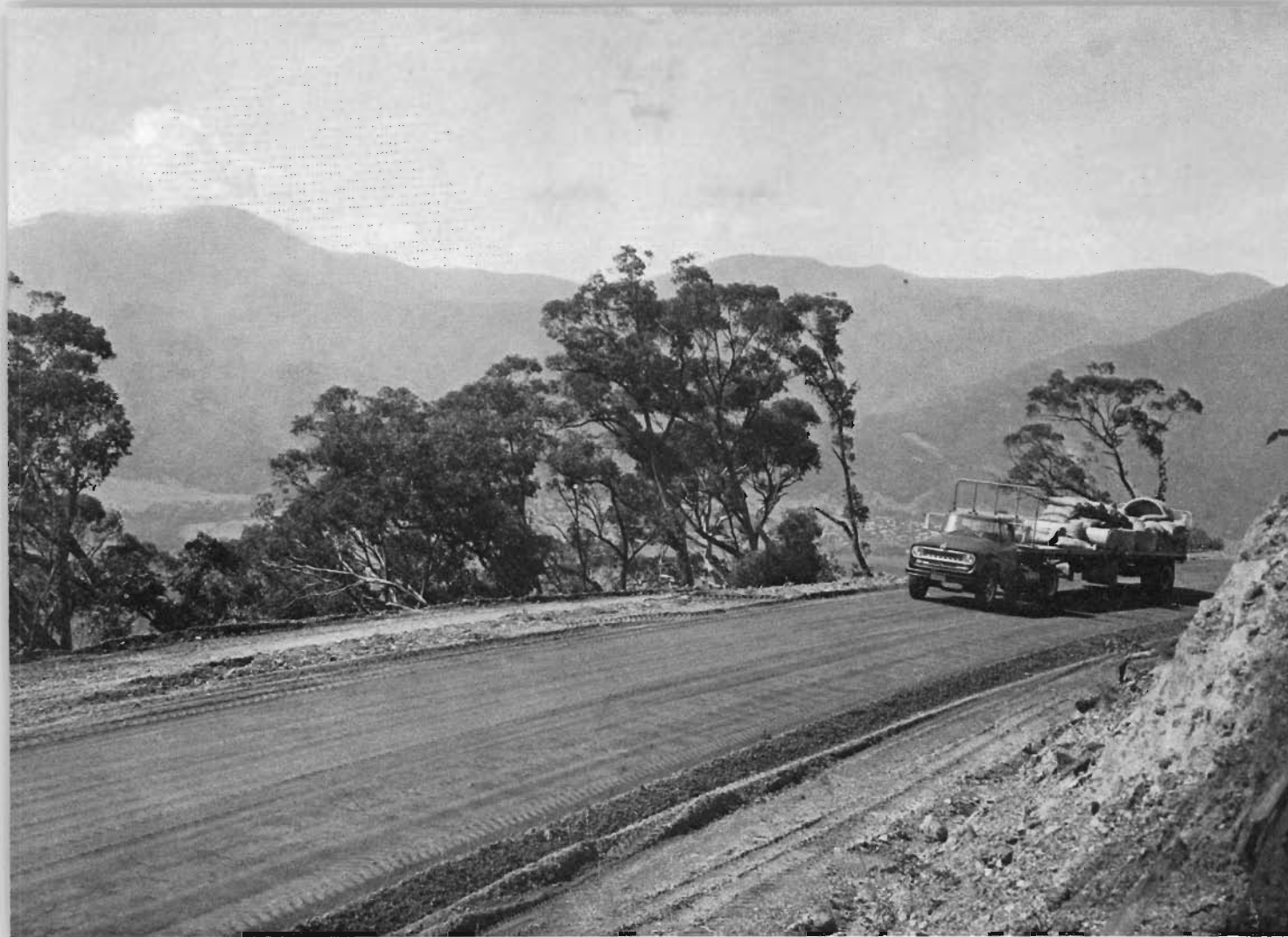
Widening in progress on the Bright - Tawonga Road, Shire of Bright
