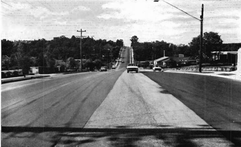
Widened section of Blackburn Road, Waverley City.
