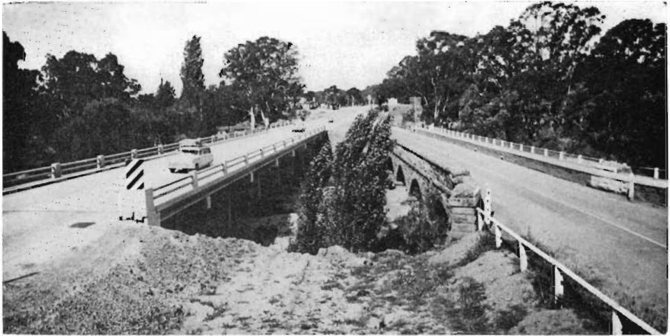
The new and old Hume Highway bridges over Hughes Creek at Avenel.
