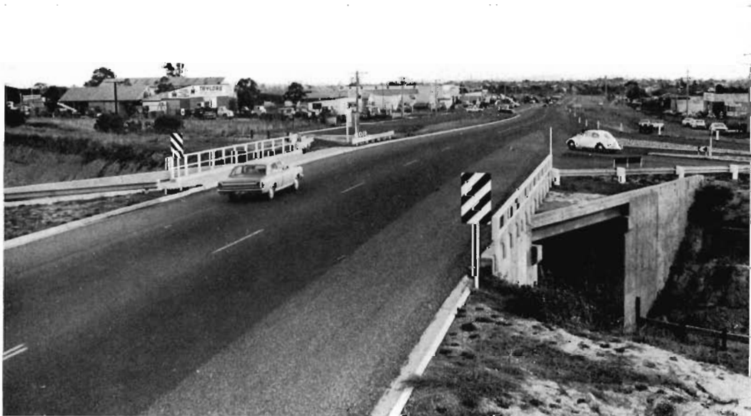
Road over rail bridge replacing the level crossing on the Princes Highway at Traralgon.
