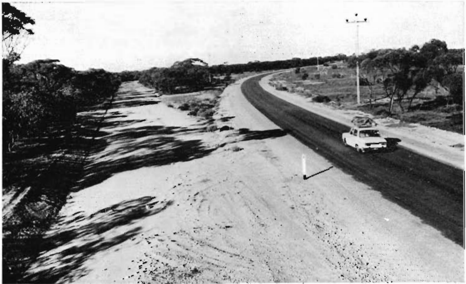
Reconstructed section of the Murray Valley Highway east of Hattah.
