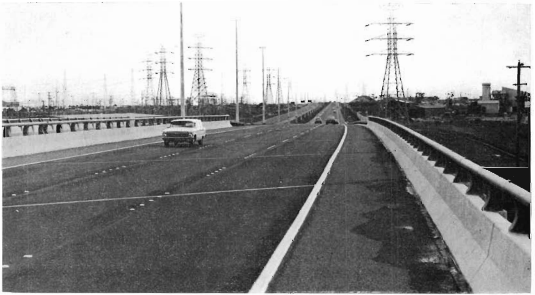
The Lower Yarra Freeway at the twin bridges over the Newport-Sunshine railway.
