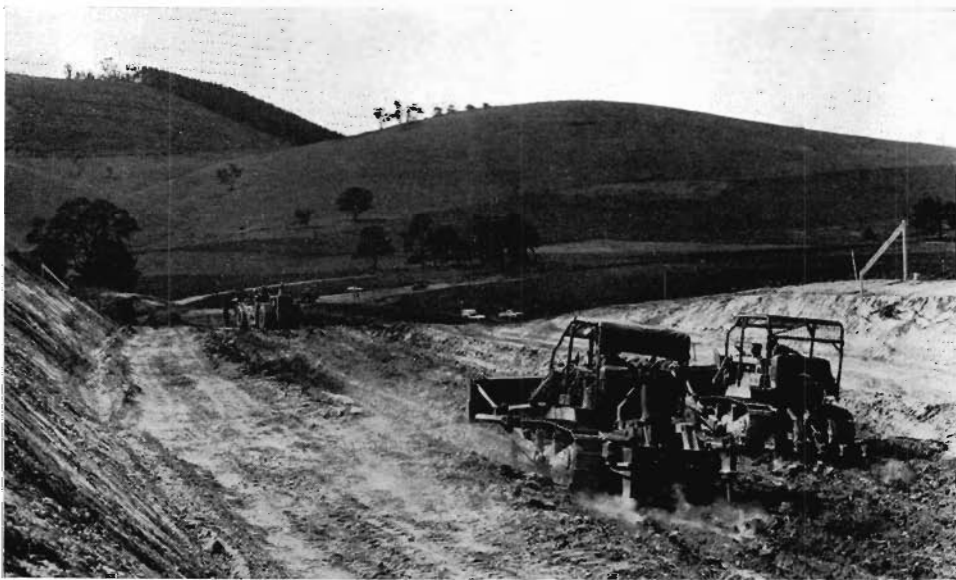
Reconstruction of the Midland Highway in progress at Mount Franklin.
