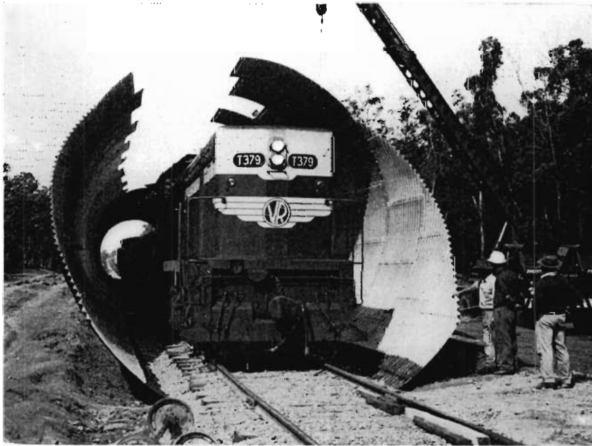
Plate 3—Lyons grade separation structure: multiplate ring partly completed.
