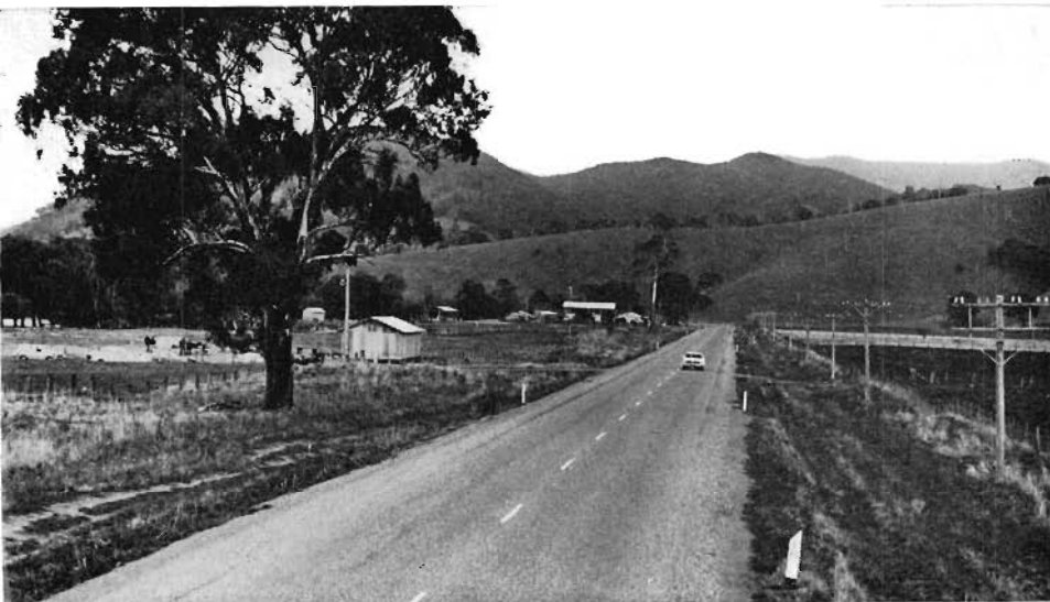
The Omeo Highway reconstructed north of Swifts Creek.
