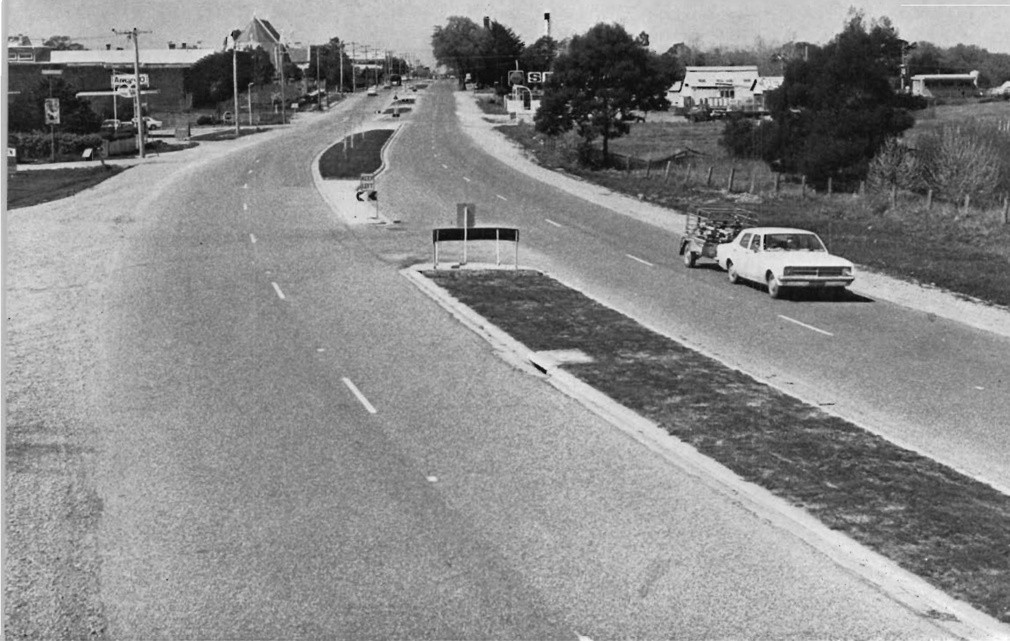
Dual carriageways constructed on the Princes Highway at Sale
