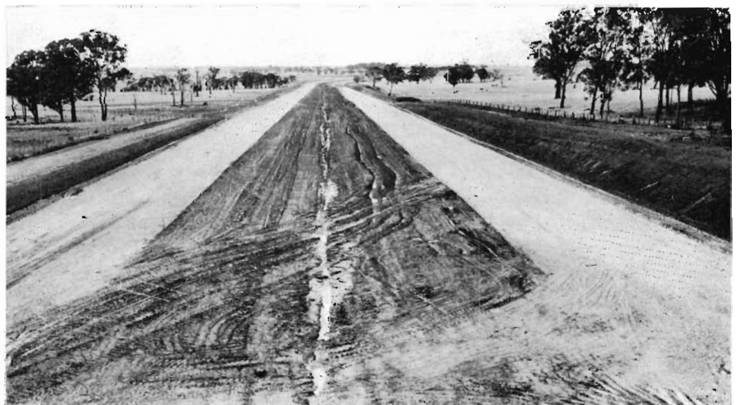
The Western Freeway (Gordon Section) under construction.
