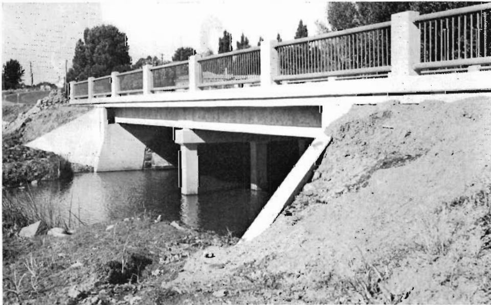
Henty Highway bridge over Grange Burn Creek showing widened section.
