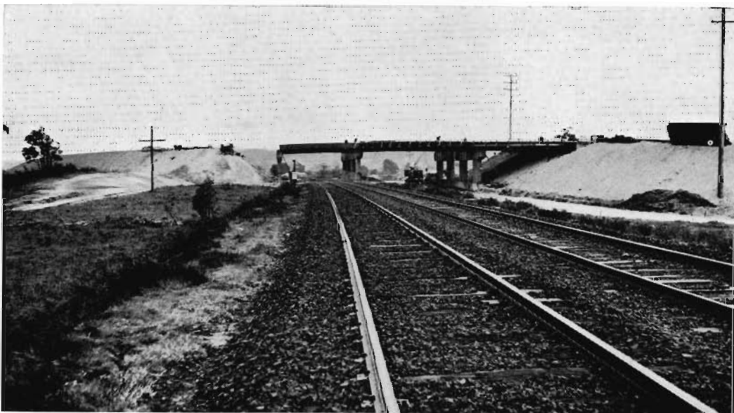
New Western Highway bridge under construction over the railway at Ballarat.
