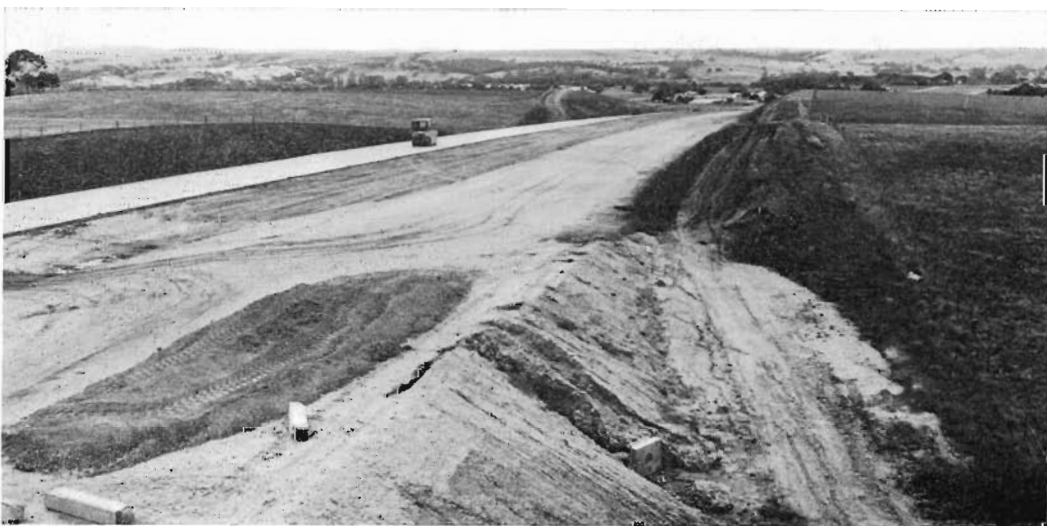
Construction of the Western Freeway (Bacchus Marsh section).
