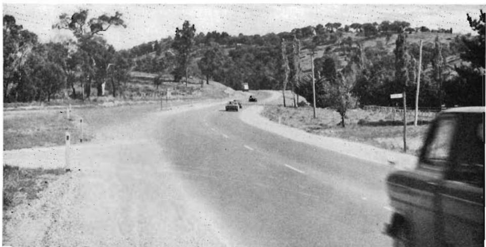
Reconstructed section of the Maroondah Highway east of the Warburton Highway.
