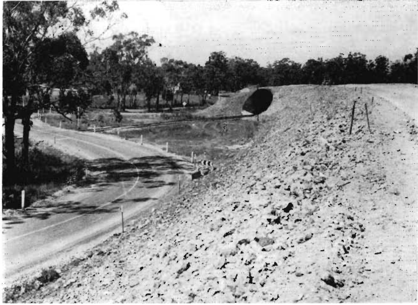
Plate 1—View of Lyons grade separation structure (before completion of the roadworks) showing the sharp approach curves to the rail level crossing.
