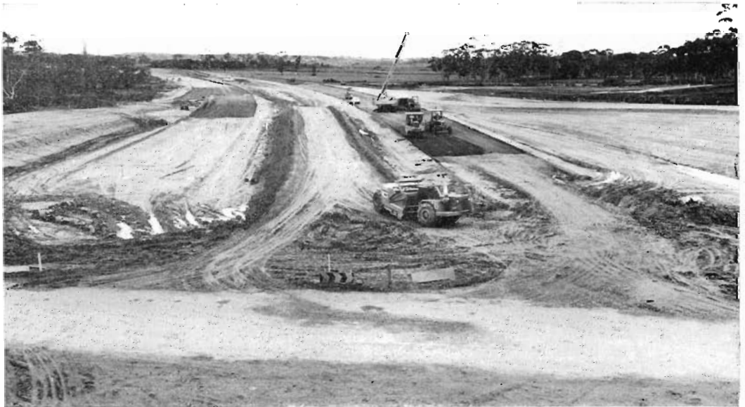
The Mulgrave Freeway under construction at Heather-ton Road.
