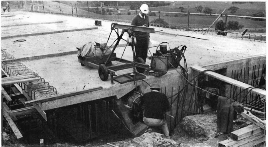
Construction of the western interchange bridge on the Western Freeway (Bacchus Marsh section).
