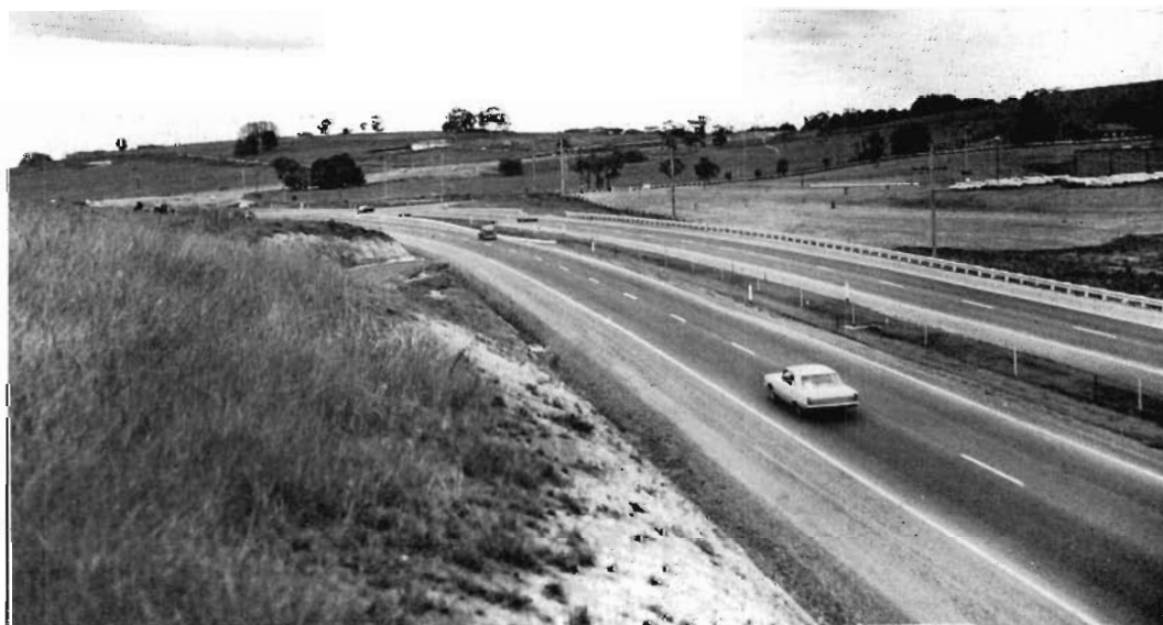
Dual carriageways constructed on the Maroondah Highway between Brushy Creek, North Croydon, and Hull Road, Lilydale.
