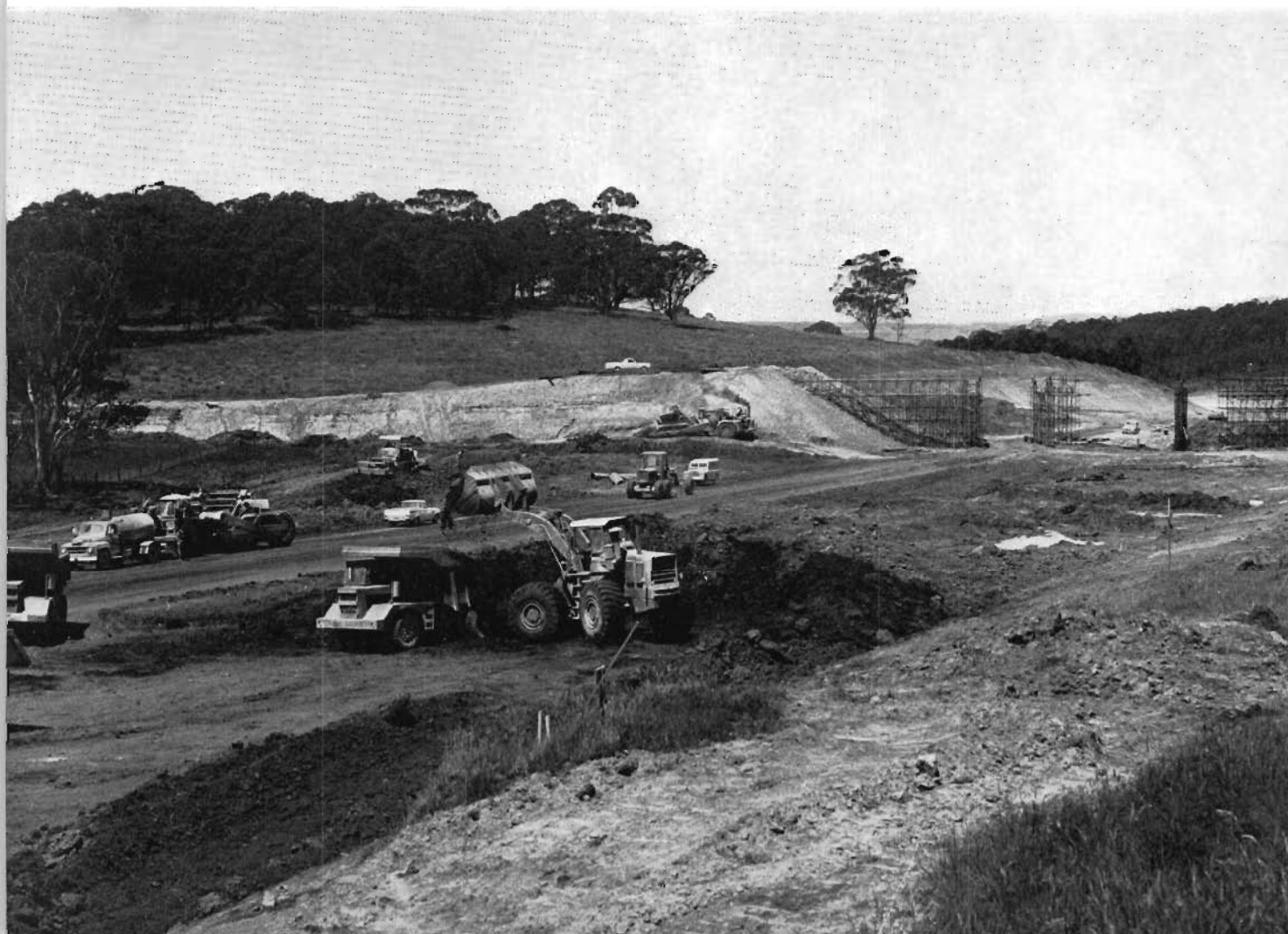
Work in progress on the Western Freeway (Gordon Section)
