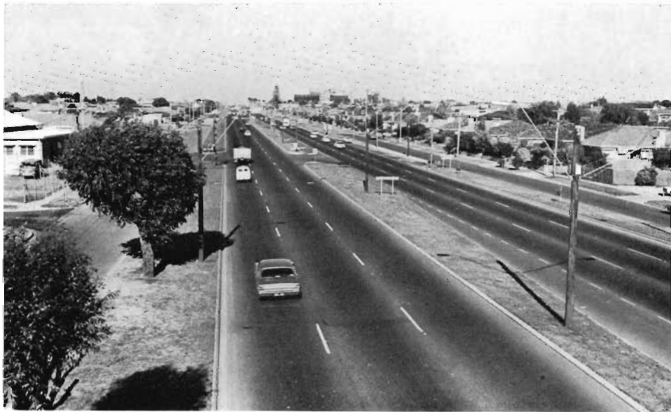
Dual carriageways constructed on the Nepean Highway at Moorabbin.
