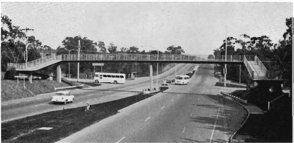
Nepean Highway, Shire of Mornington. Pedestrian overpass at Mount Eliza.
