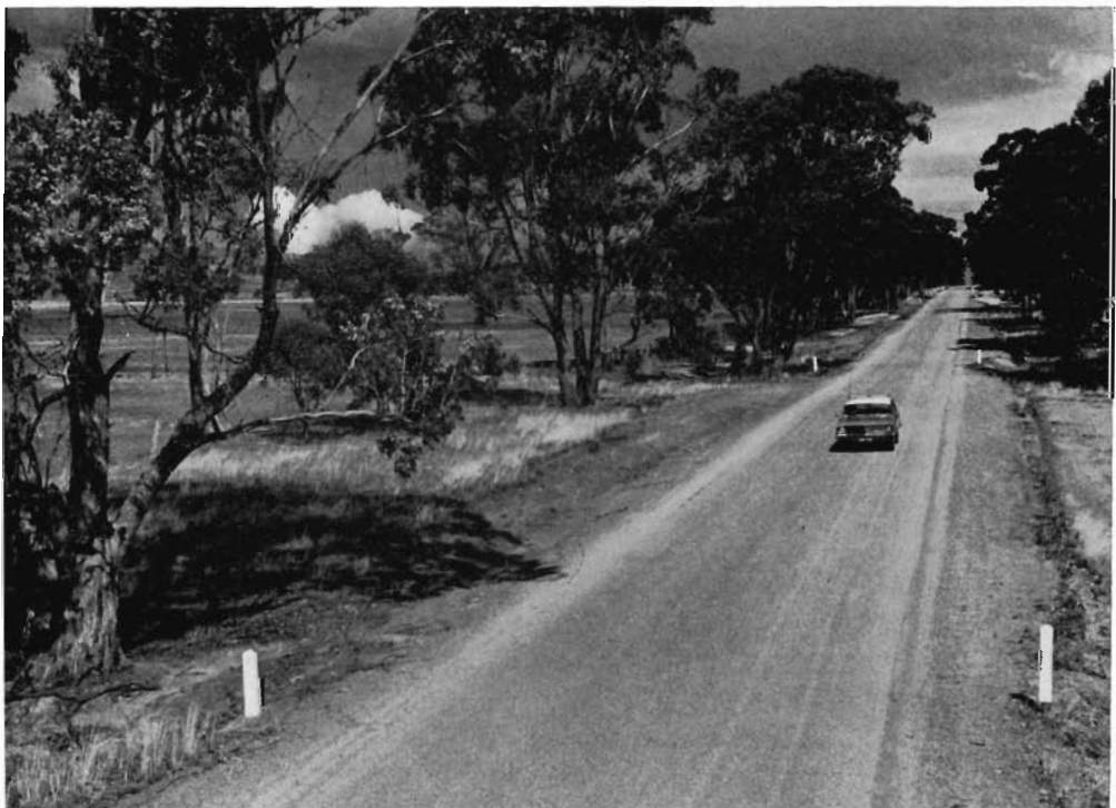
Benalla-Yarrawonga Road, Shire of Benalla. Widened section near Bungeet.
