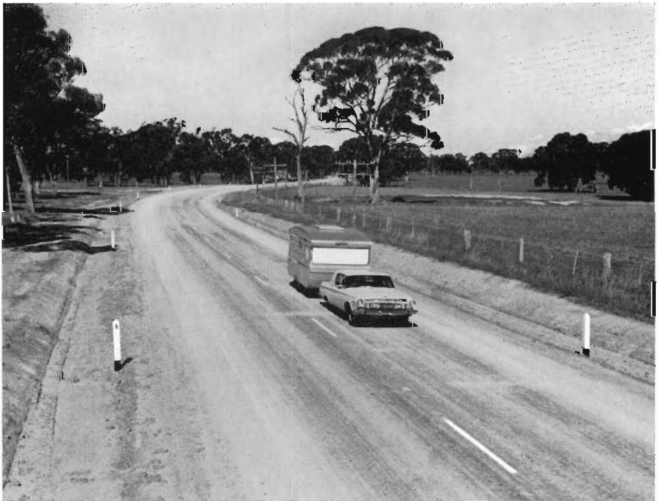
Henty Highway, Shire of Arapiles. Widened section between Mockinya and Wonwondah North.
