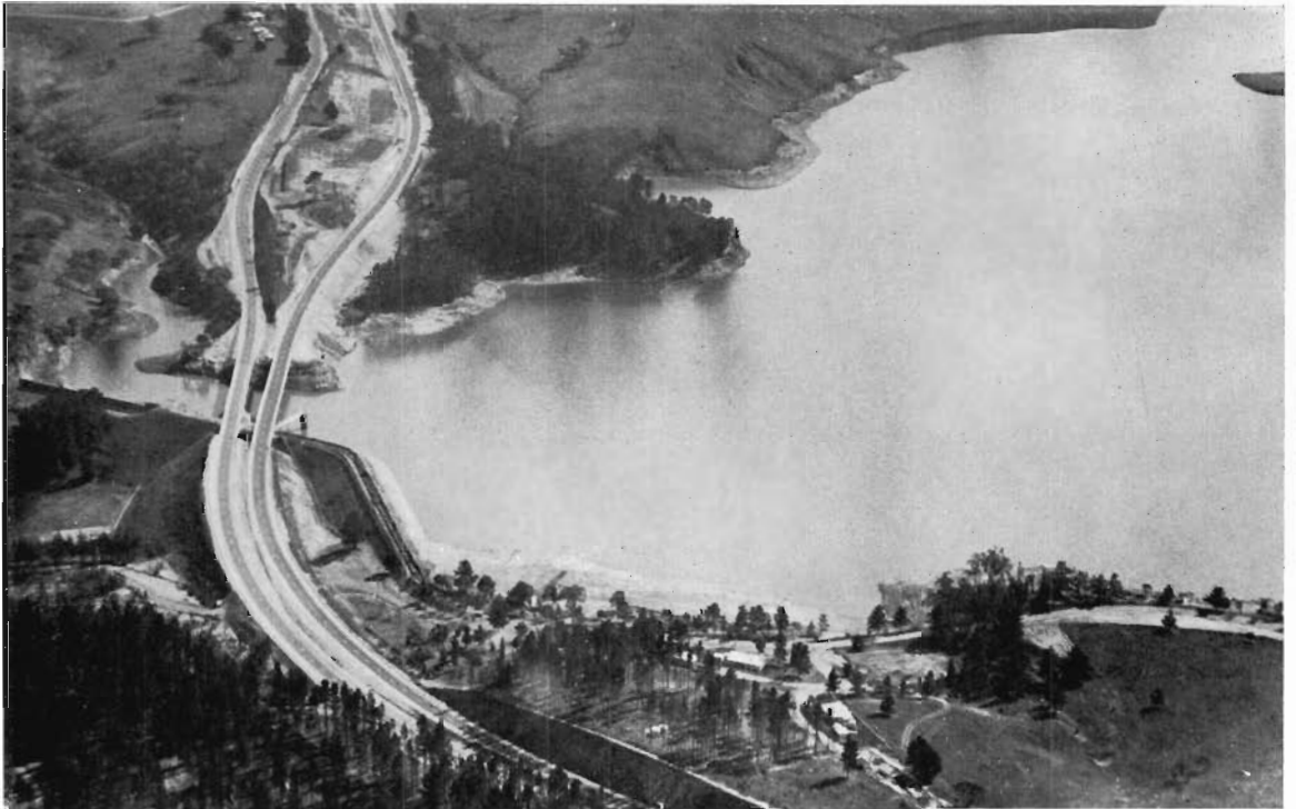
Western Highway, Shire of Ballan —Dual Carriageways and bridges at Pykes Creek Reservoir.
