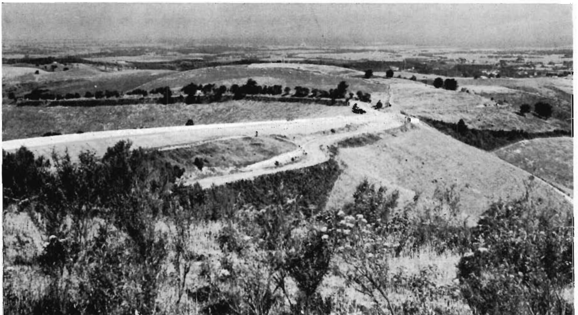
South Gippsland Highway, Shire of South Gippsland. Reconstruction on an improved alignment north of Foster.
