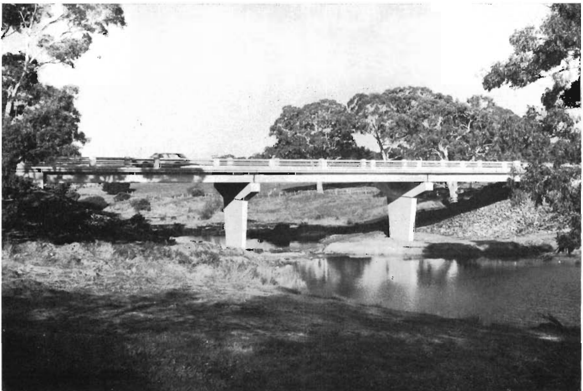
Glenelg Highway, Shire of Dundas. New Concrete Bridge over the Wannan River near Wannon.
