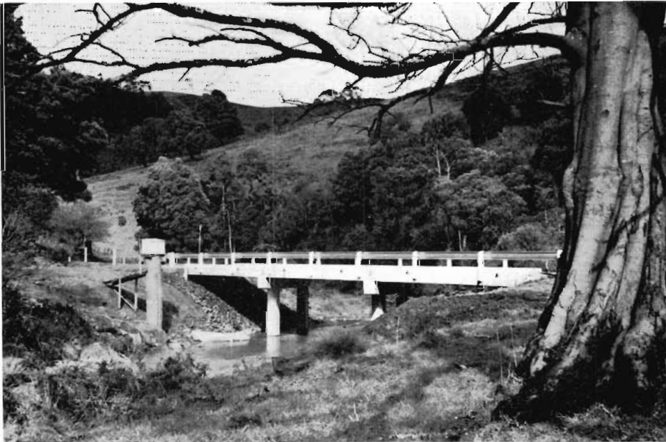
Albert River Road, Shire of Alberton. New reinforced concrete bridge at Hiawatha.
