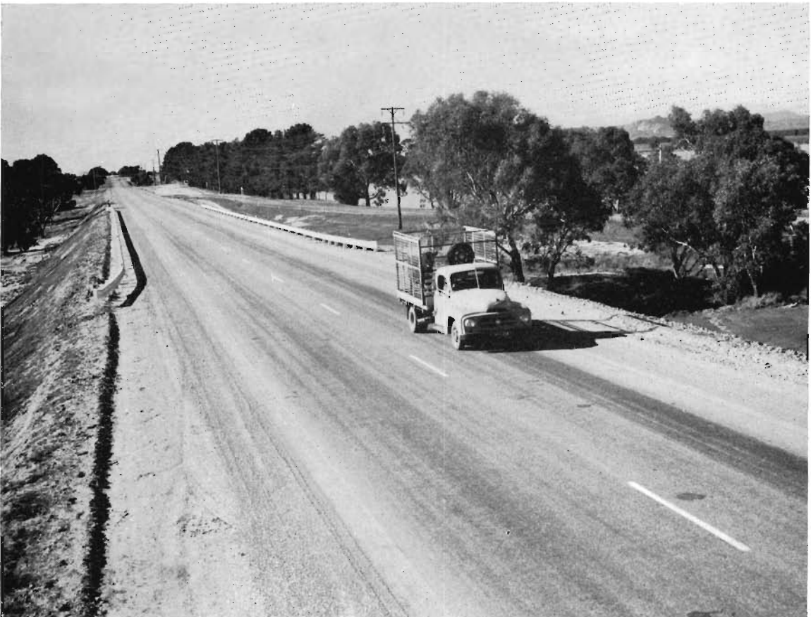
Western Highway, Shire of Wimmera. Reconstruction and realignment at Green Lakes.
