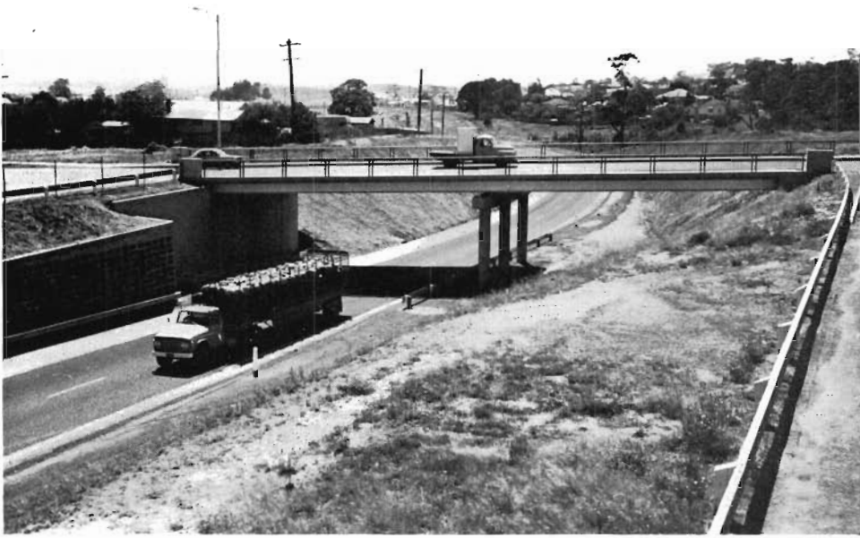
Princes Bypass Road (Moe Section) A reinforced concrete bridge providing grade separation.
