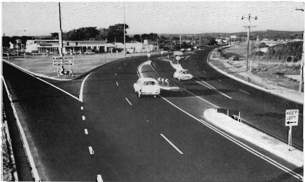
Nepean Highway, Shire of Flinders. Intersection treatment at Dromana.
