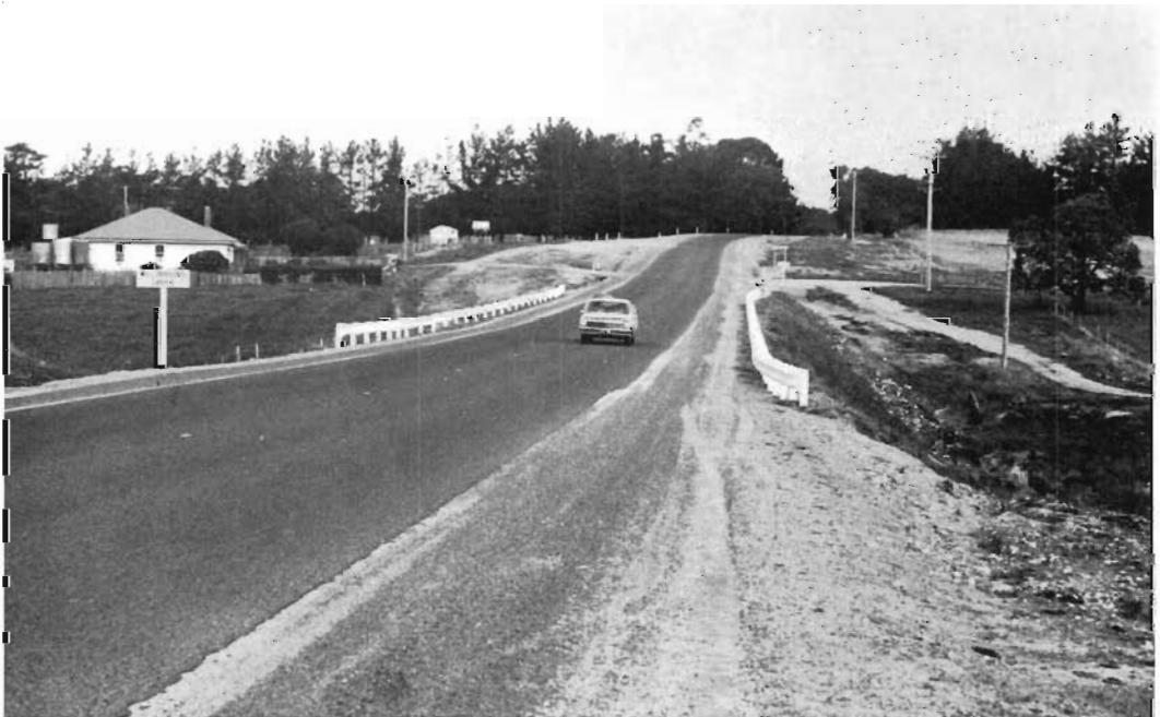
Midland Highway, Shire of Buninyong. Realignment and new culverts at Clarendon.
