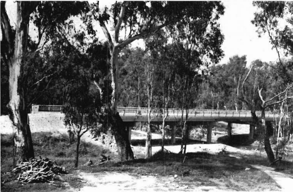
Bright Road, City of Wangaratta. New bridge over the King River.
