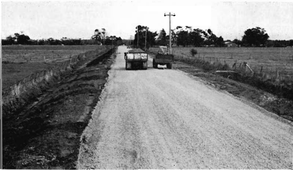
Billington Avenue, Shire of Cranbourne. Reconstructed section prior to sealing.
