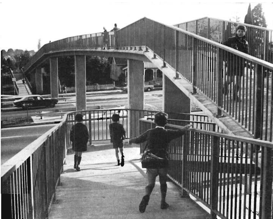
Pedestrian overpass at Mitcham, Maroondah Highway, City of Nunawading.
