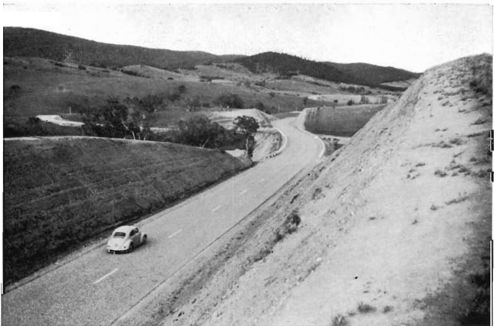
Omeo Highway, Shire of Omeo. Reconstructed section between Omeo and Black Camp Creek.
