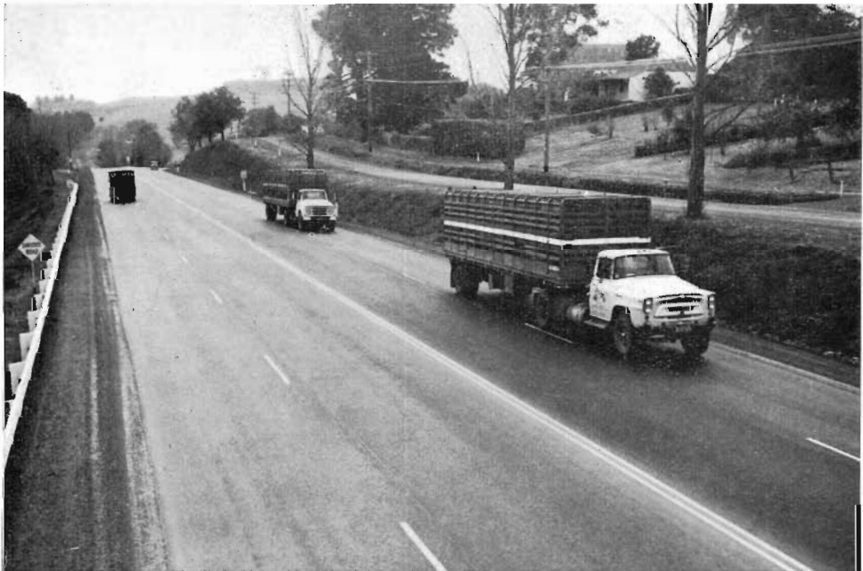
Princes Highway East, Shire of Berwick. Reconstruction to provide climbing lanes on Berwick Hill.
