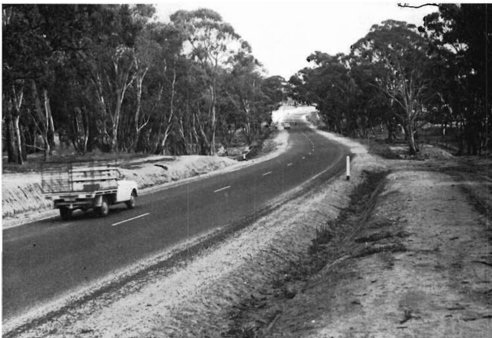
Pyrenees Highway, Shire of Ararat. Reconstructed section west of Elmhurst.
