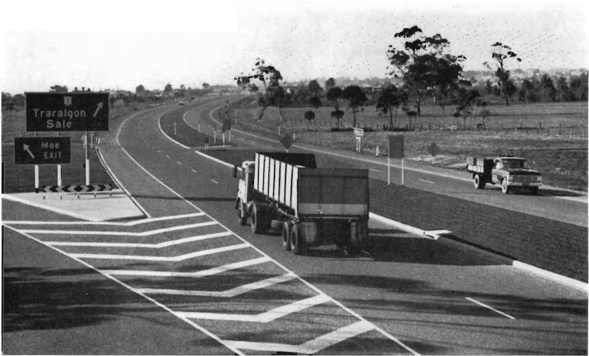
Special Project No. 9—The Princes By-pass Road (Moe Section) west of Moe.
