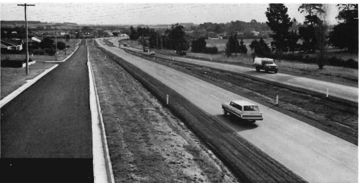
Princes Highway East, Shire of Berwick—Dual Carriageways east of Narre Warren.
