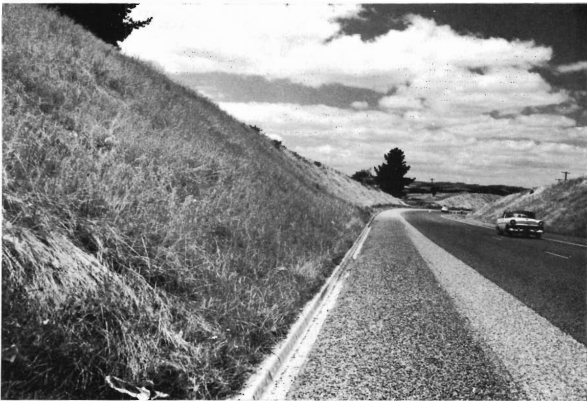
Plate 2 — Batter Stabilisation, Princes By-pass Road, Moe. Cover Growth for Stabilisation after Treatment.
