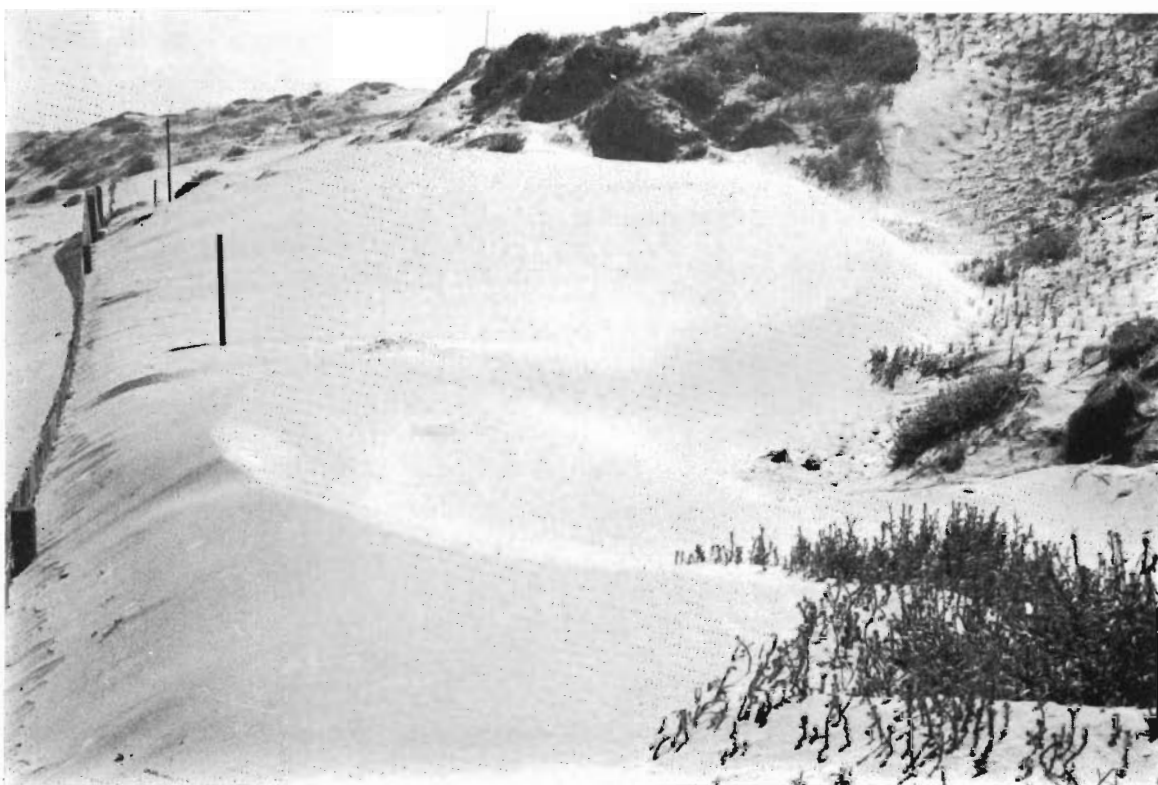
Plate 6 — Sand Drift Control. Closing Drift Built Up Behind Slat Fence.
