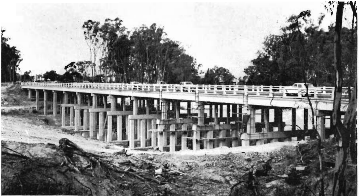
Midland Highway — Underpinning the bridge over the Goulburn River at Shepparton.
