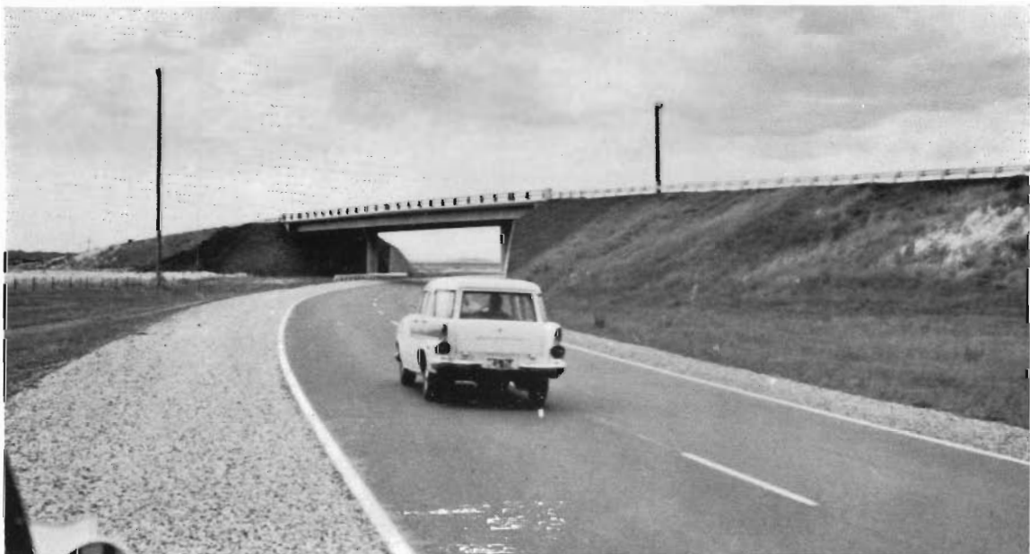
Tullamarine Freeway — Interchange bridge at Airport entrance.
