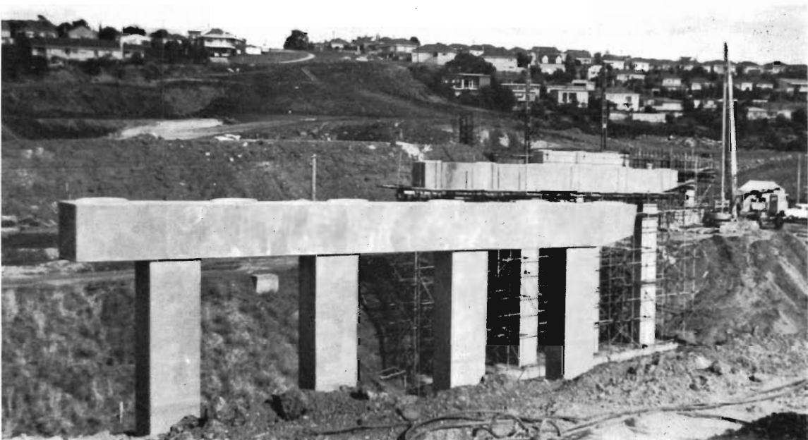
Strathmore By-pass Road — Work in progress — View from Bell Street end.
