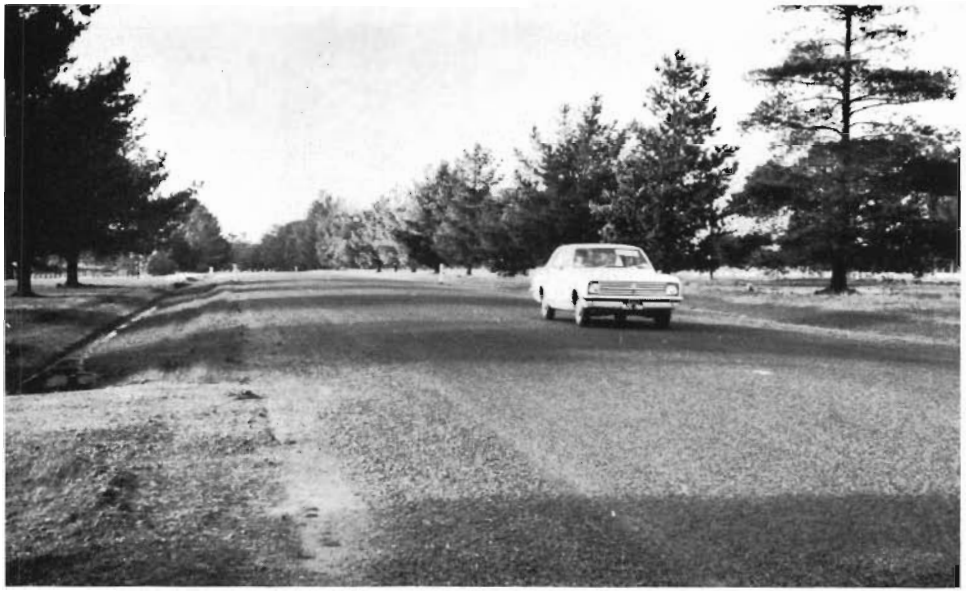
Glenelg Highway — Reconstructed section west of Hamilton.
