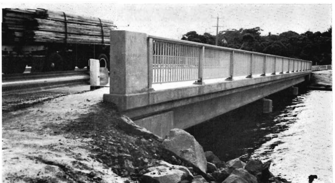
Anglesea River Bridge — Ocean Road, Barrabool.
