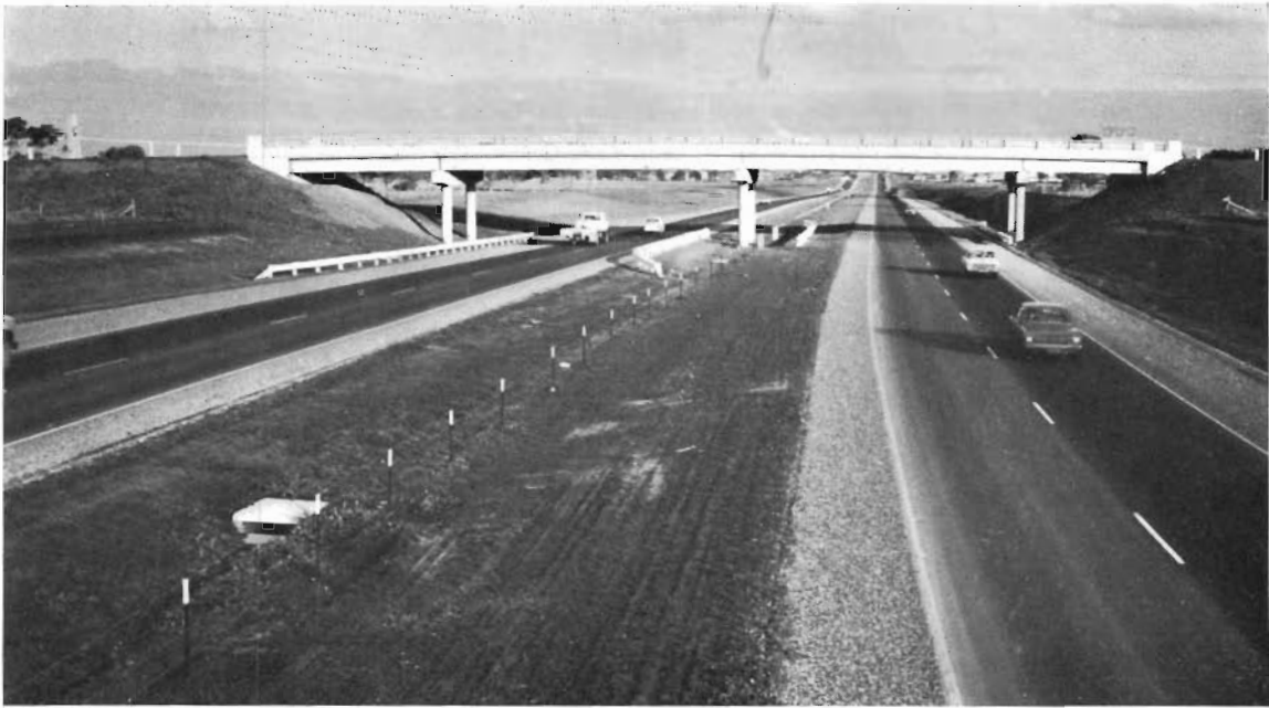
Tullamarine Freeway — View under Carrick Drive Overpass.
