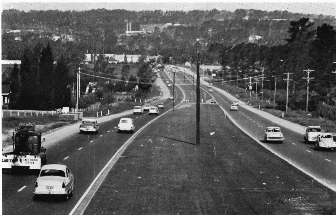
Burwood Highway — Dual carriageways between Springvale Road and Dandenong Creek.
