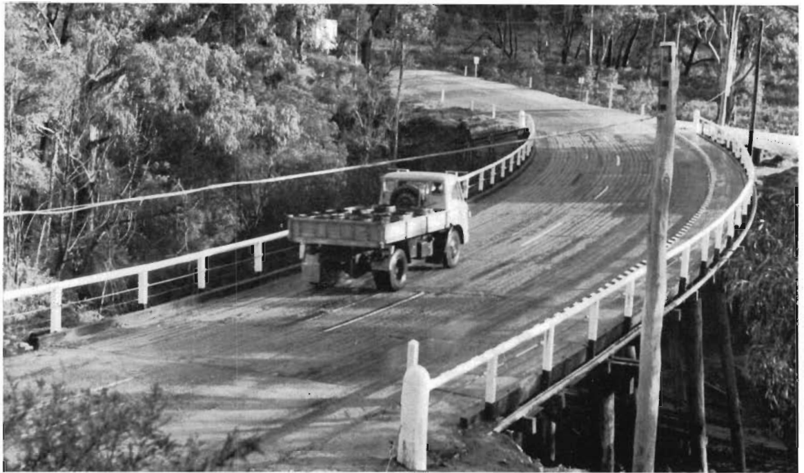
Grampians Tourists' Road — Widening of Delly's Bridge.
