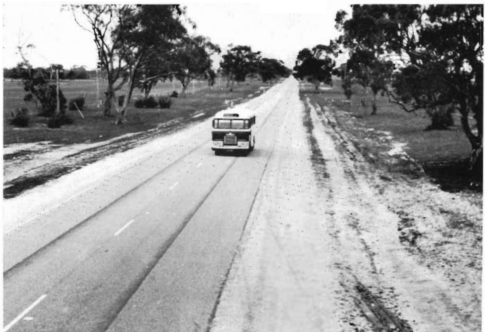
Henty Highway — Widened and resheeted section north of Kellalac.
