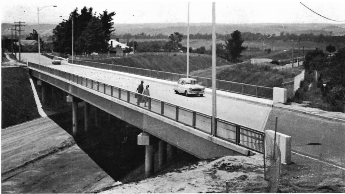
Princes By-pass Road (Moe Section) — Coalville Road Bridge.
