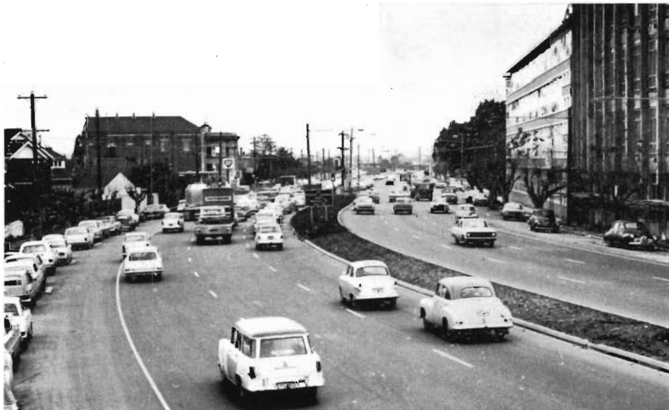
Princes Highway East — Waverley Road to Repton Road.
