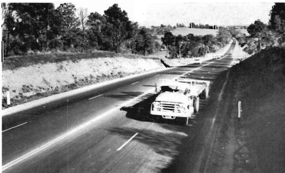
Princes Highway East — Widening East of Mt. Ararat.
