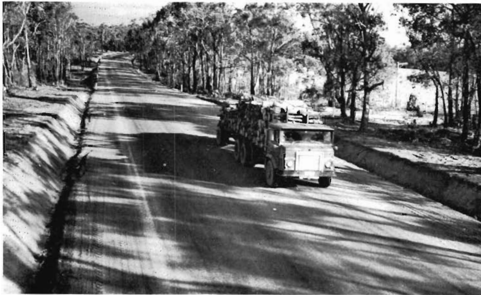
Midland Highway — Reconstructed section south of Yinnar.
