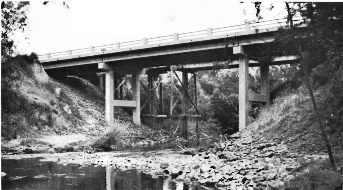
Heath Hill bridge over the Lang Lang River, Westernport Road, Cranbourne Shire.
