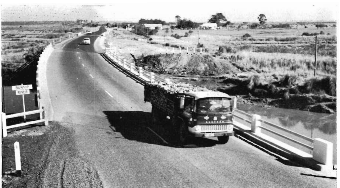
South Gippsland Highway — New bridge over the Bunyip River in Cranbourne Shire.
