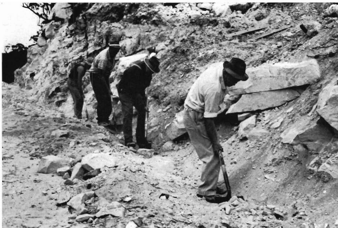
Drought Relief — Workers on Mt. Difficult Road, Wimmera Shire.
