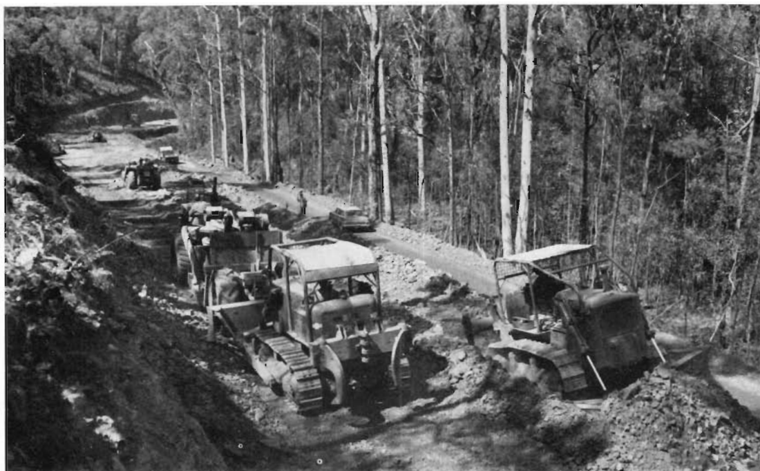
Yarra Glen-Glenburn Road—Board's plant at work—Shire of Healesville.
