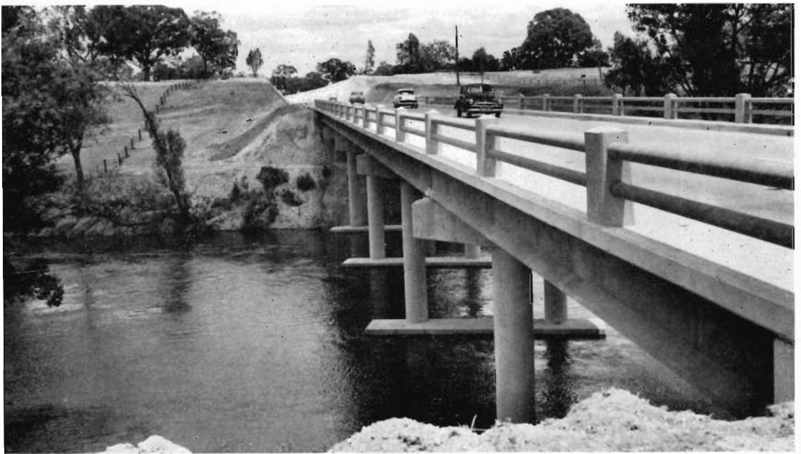
Hume Highway—New Bridge over the Goulburn River on the approach to Seymour.
