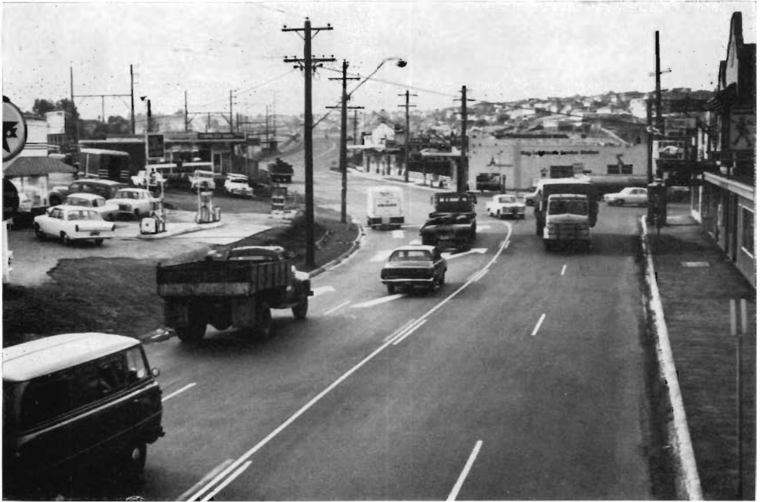
Pascoe Vale Road—Reconstructed section at Woodlands Street intersection.
