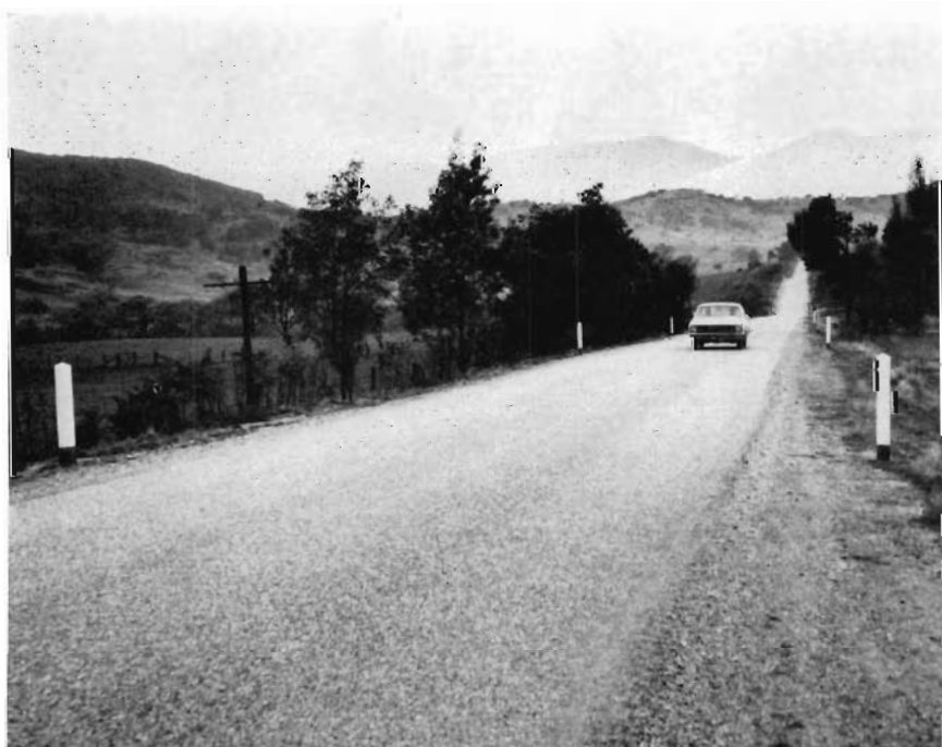
Dederang Road—Yackandandah Shire—Reconstructed section.
