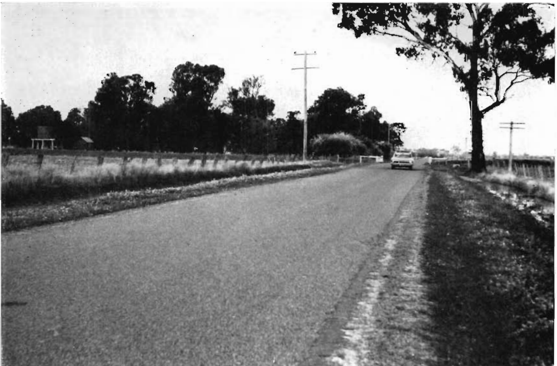
Baulkamaugh Hall Road—Strengthened and sealed to a width of 18 feet.
