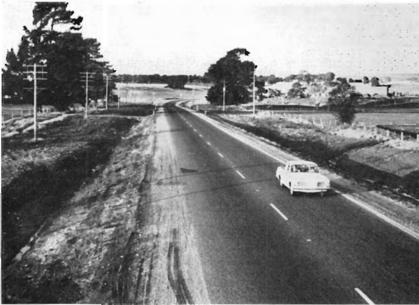
Glenelg Highway, Grenville Shire—Widening west of Ballarat.
