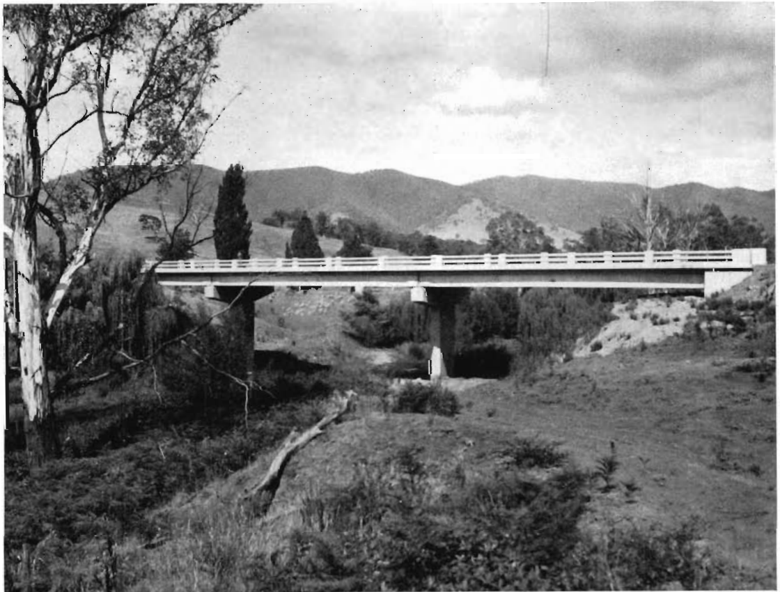
New bridge on Ramrod Flat Road over the Tambo River—Shire of Tambo.
