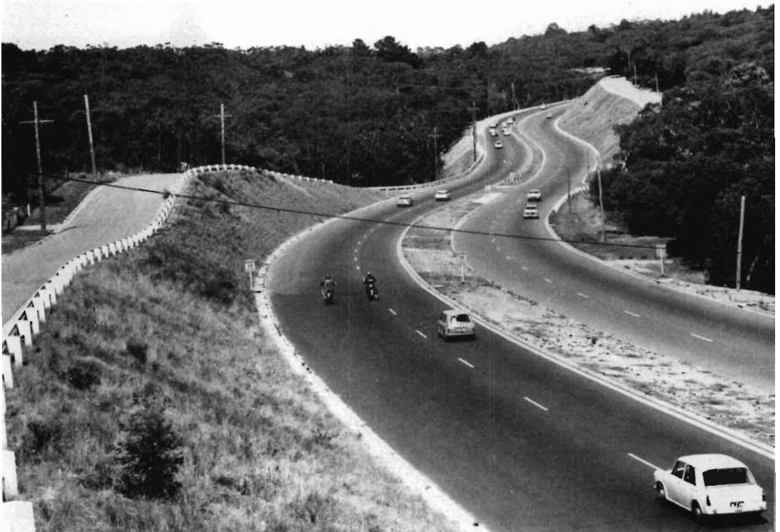
Special Road Fund Project No. 13—Dual carriageways on the Nepean Highway South of Frankston.
