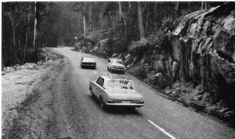
Mount Buffalo Road—A "freeze-thaw" resistant pavement at road level 4000 feet.
