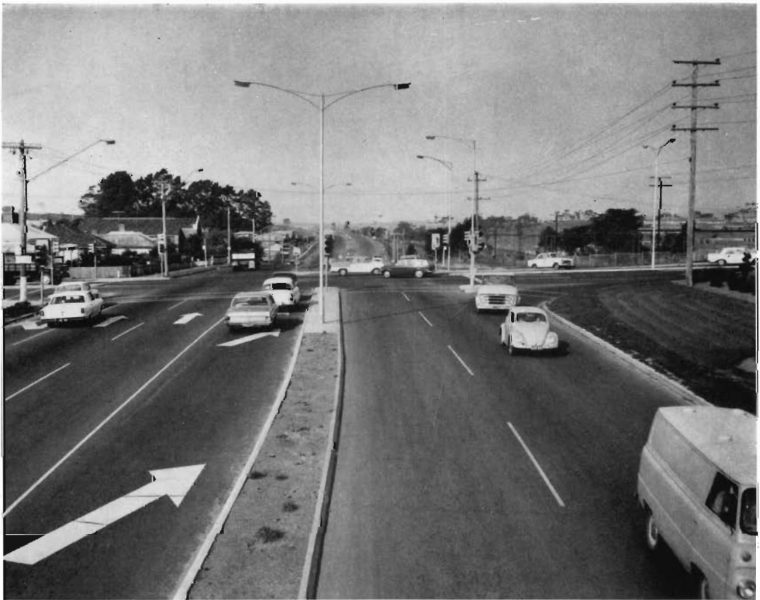
Princes Highway East—Dual carriageways at the McDonald Street intersection in Morwell.
