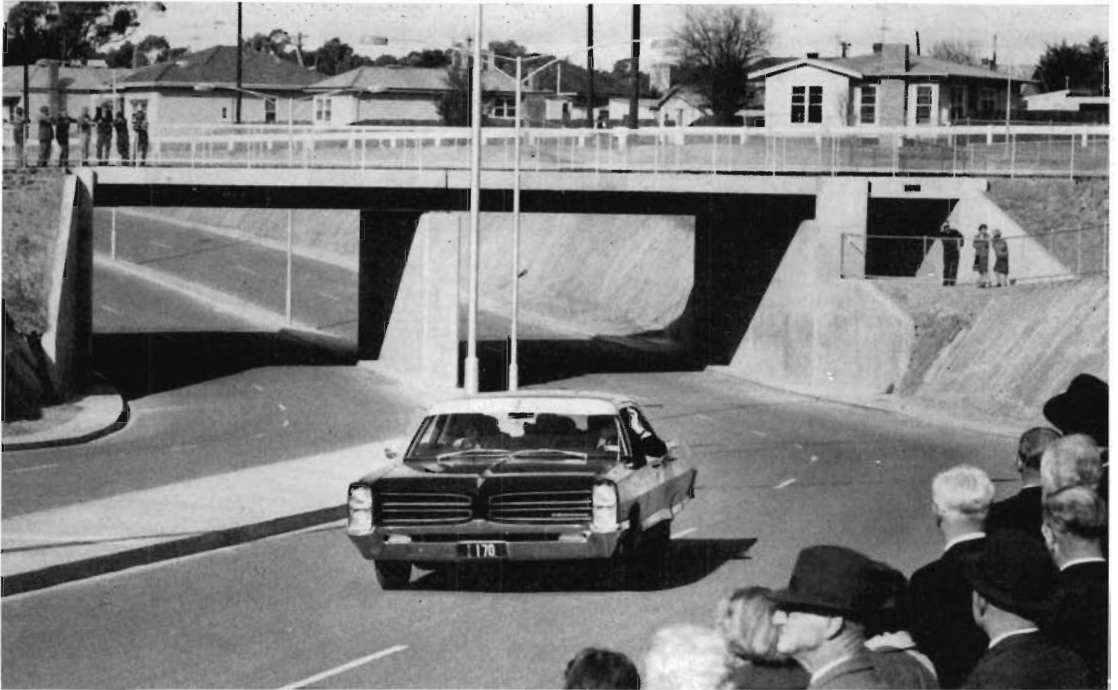
The Minister of Public Works, the Hon. M. V. Porter, M.L.A., becomes the first official traveller to use the Tuaggra Street underpass in Maryborough City. The opening ceremony was attended by the Chairman and Member of the Board, the Mayor of Maryborough and other invited guests.
