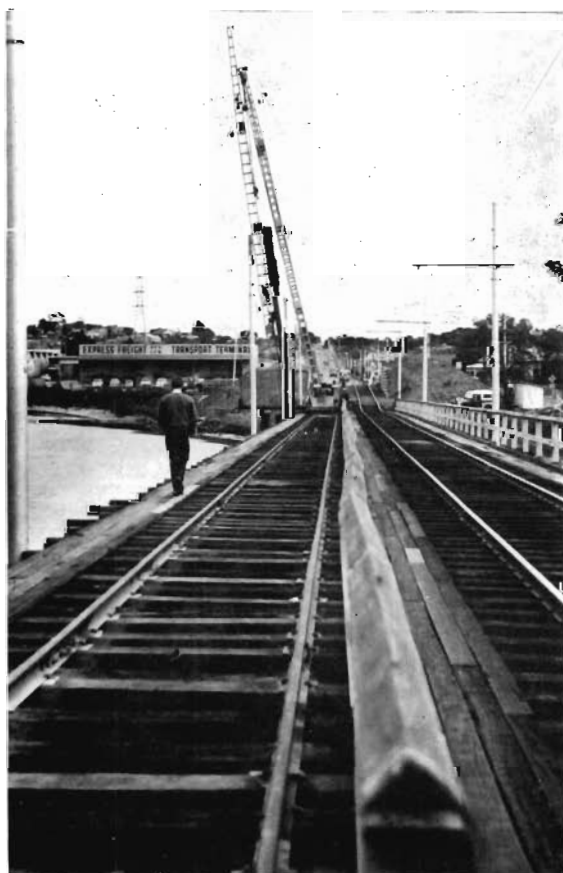
Plate 1—Maribyrnong River Bridge. Raleigh's Road. General view showing limited working space available for pile driving frame.
