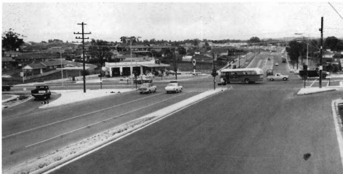
Dual carriageways and intersection treatment at the junction of Canterbury Road and Springvale Road —Nunawading City.
