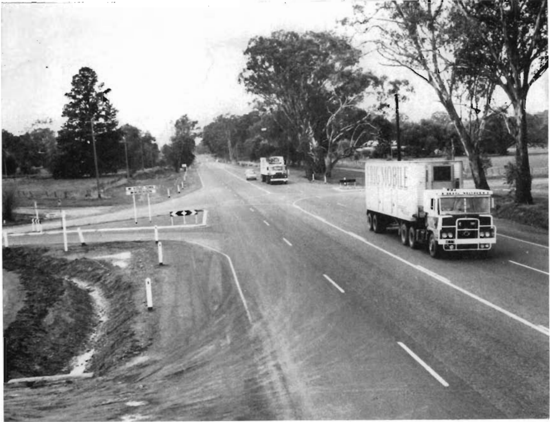
Hume Highway—Intersection treatment at the junction with the Murchison Violet Town Road—Violet Town Shire.
