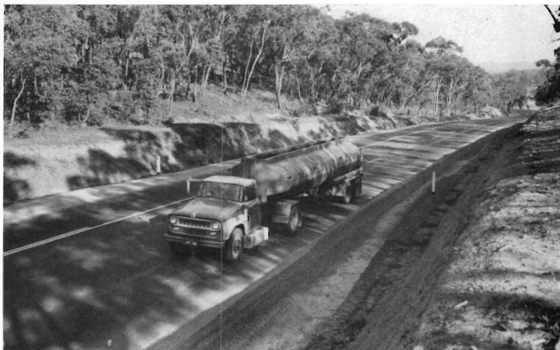
Calder Highway—Reconstruction with an additional climbing lane at Taradale.
