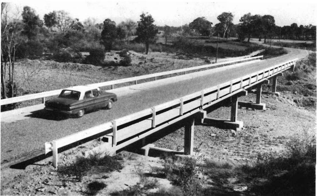
Delta Bridge over Valencia Creek, Briagolong Road—Shire of Maffra.
