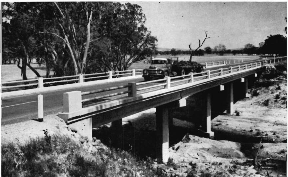
North Western Highway—New bridge over the Avoca River at Vale of Avoca—Avoca Shire.
