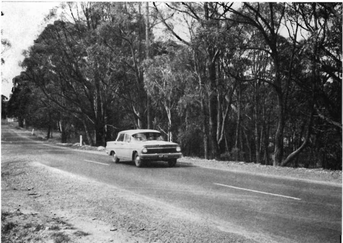
Ballan Road—Daylesford and Glenlyon Shire, reconstructed section.
