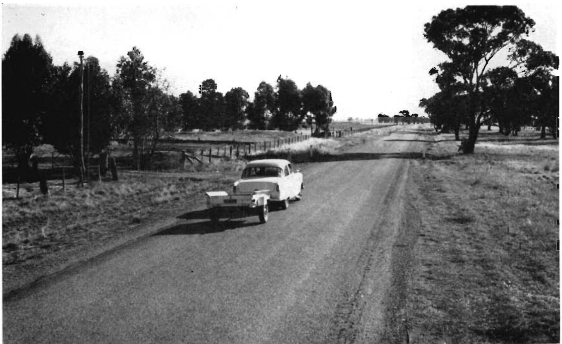
Charlton Road—Kara Kara Shire—Reconstructed section.
