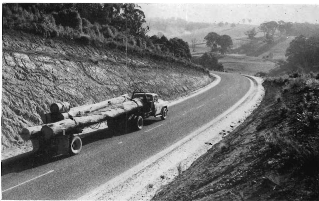
Yarram-Traralgon Road—Reconstructed section near Lays Road—Shire of Alberton.
