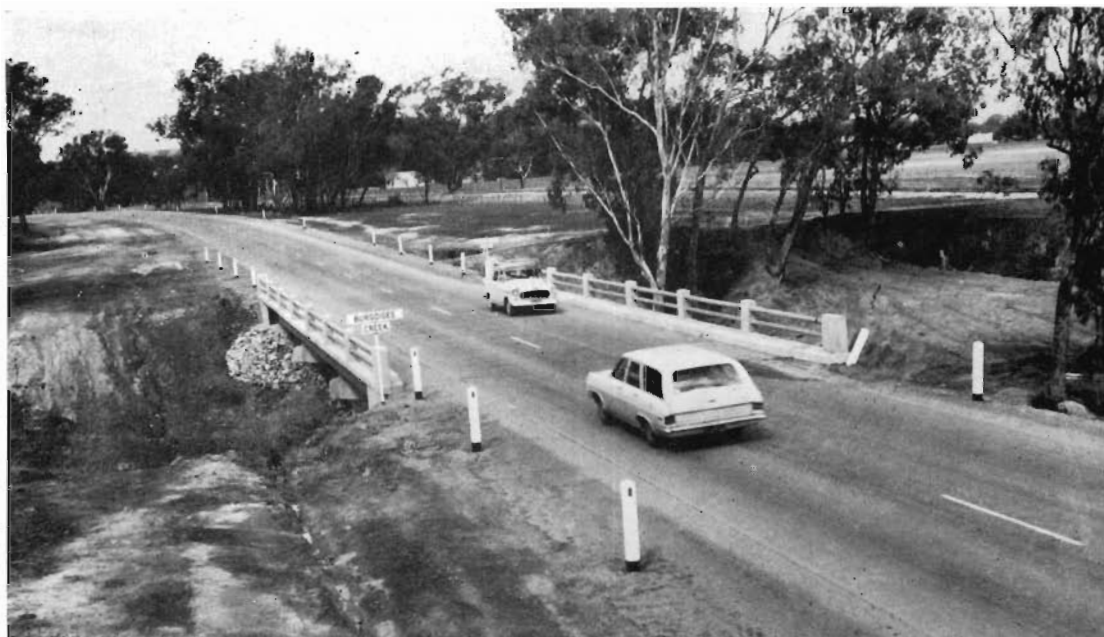
Ovens Highway—New bridge and approaches at Burgoigee Creek.
