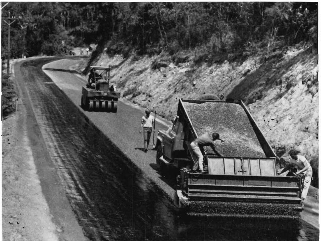
Completing the bituminous sealed pavement between Melbourne and Sydney on the Princes Highway East near Mount Drummer.
