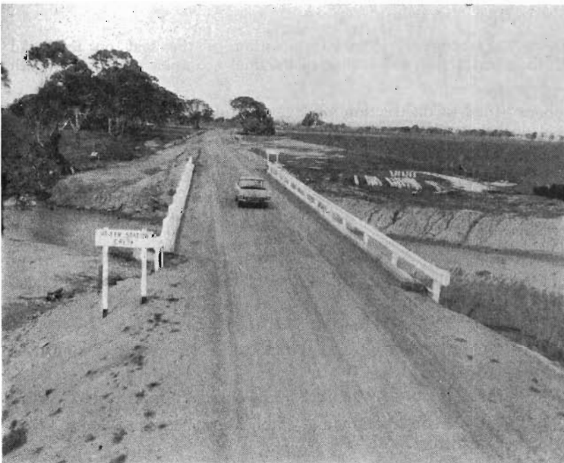
Plate 42.—Tyries Bridge over Heifer Station Creek on Campbells Bridge—Green Creek Road—Shire of Stawell.
