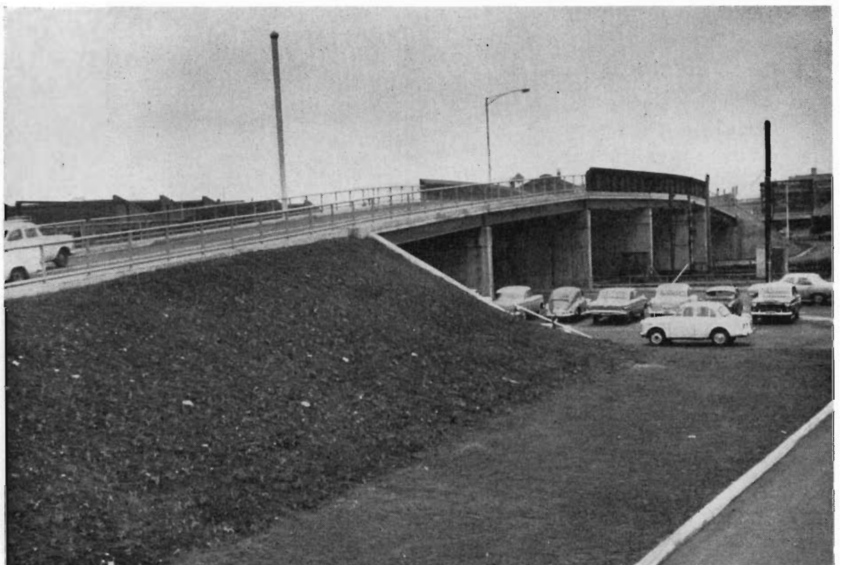
Plate 20.—Road over Rail Overpass at Burnley Street—City of Richmond.
