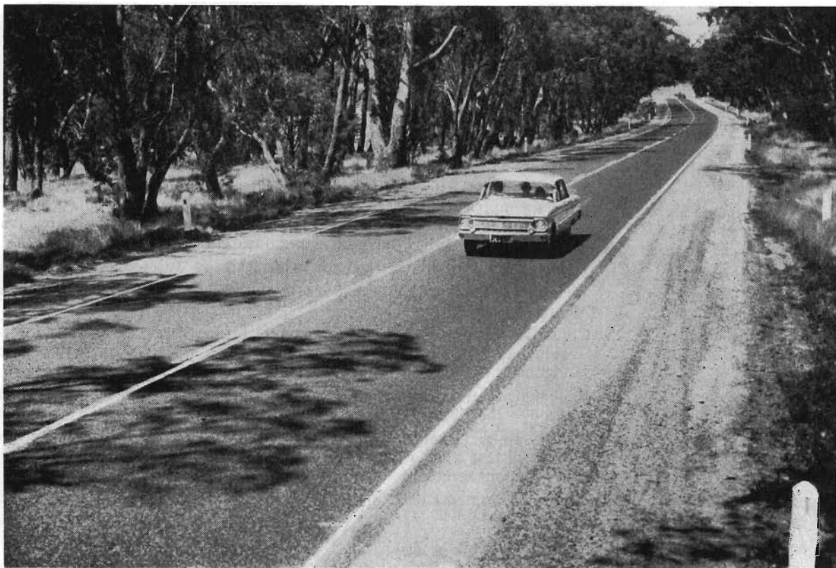
Plate 31.—Edge lining on the Calder Highway in the Black Forest area—Shire of Gisborne.
