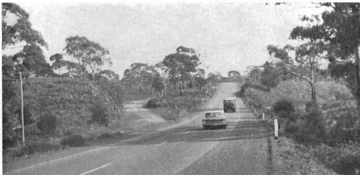
Plate 8.—Princes Highway West—New construction through the Stony Rises—Shire of Heytesbury.
