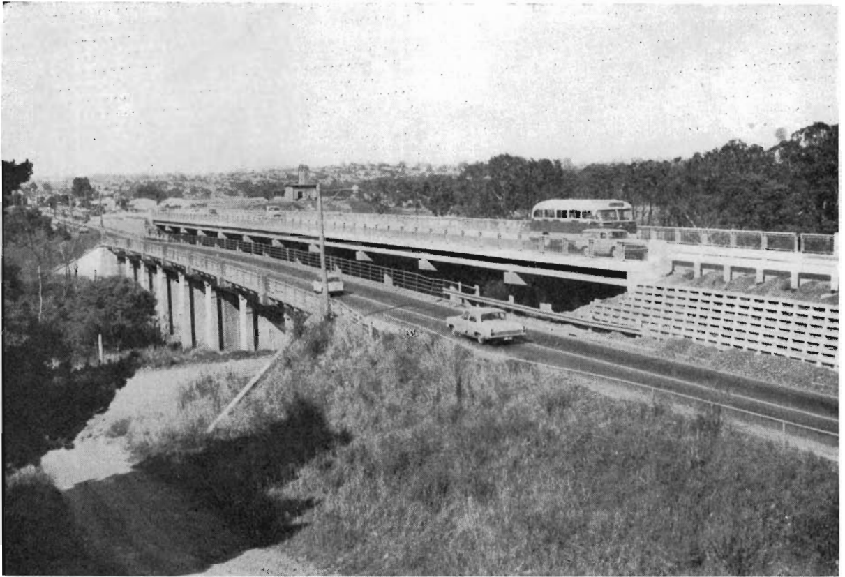
Plate 19.—New Duplicate Bridge over the Yarra River on Burke Road at the boundaries of the Cities of Camberwell, Kew and Heidelberg.
