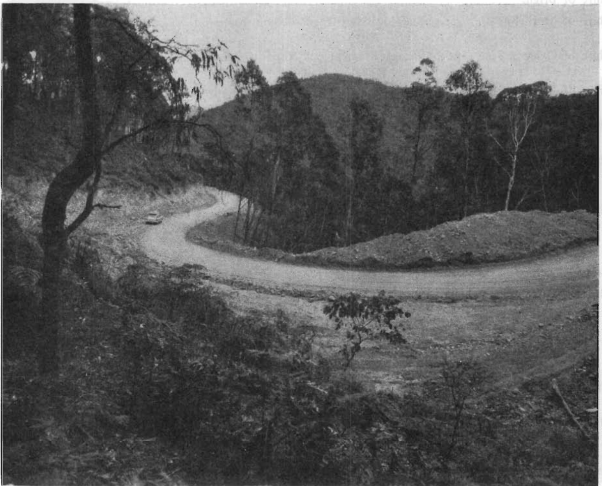
Plate 39.—Reconstructed section of the Bright-Tawonga Road—Shire of Bright.
