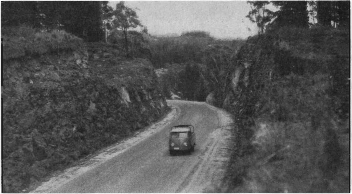
Plate 38.—Ballarat-Daylesford Road reconstructed and realigned near the "Gong" Reservoir—Shire of Bungaree.
