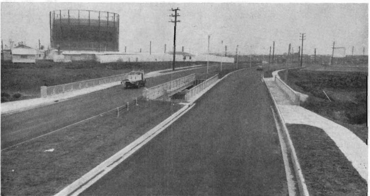
Plate 7.—New dual bridges over the Darebin Creek, Murray Road, City of Preston.
