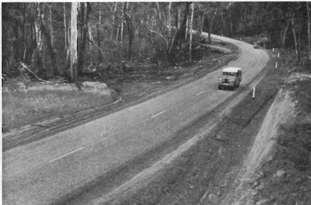
Plate 9.—Grampians Road—New deviation at Lake Bellfield—Shire of Stawell.
