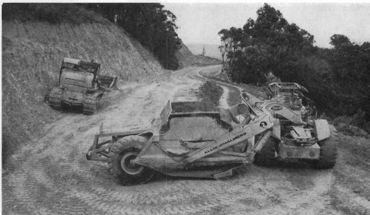
Plate 14.—Contractor's plant in operation on the Foster deviation—South Gippsland Highway—Shire of South Gippsland.
