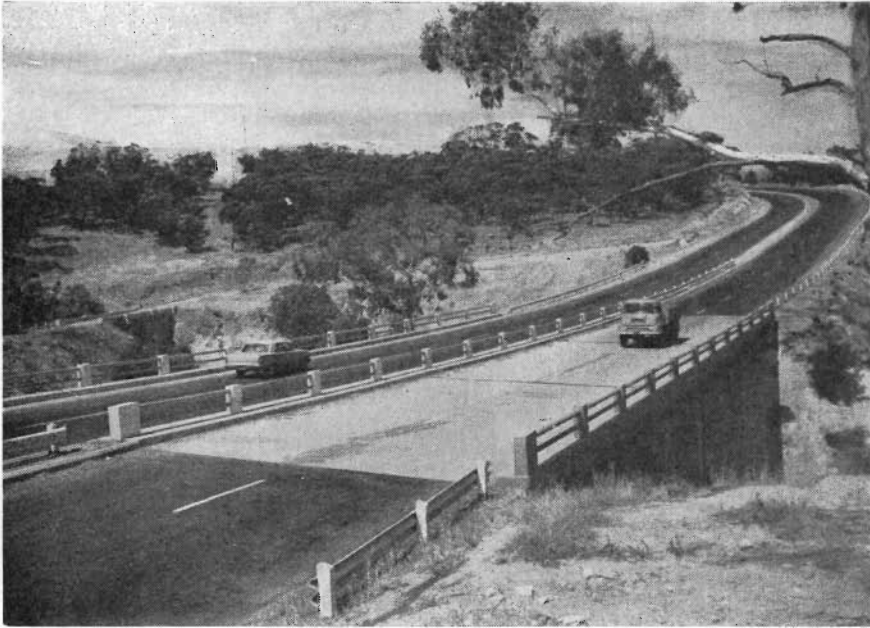
Plate 3.—Special Project No. 5.— New dual bridge and carriageway at Djerriwarrh Creek on the Western Highway.
