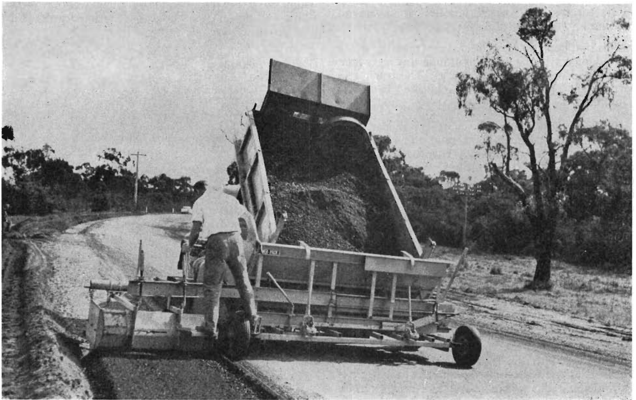
Plate 4.—Side casting trench spreader coupled to delivery truck.
