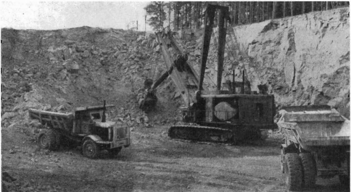
Plate 2.—Special Project No. 7. Heavy rock work in the cutting near Pykes Creek on the Western Highway.
