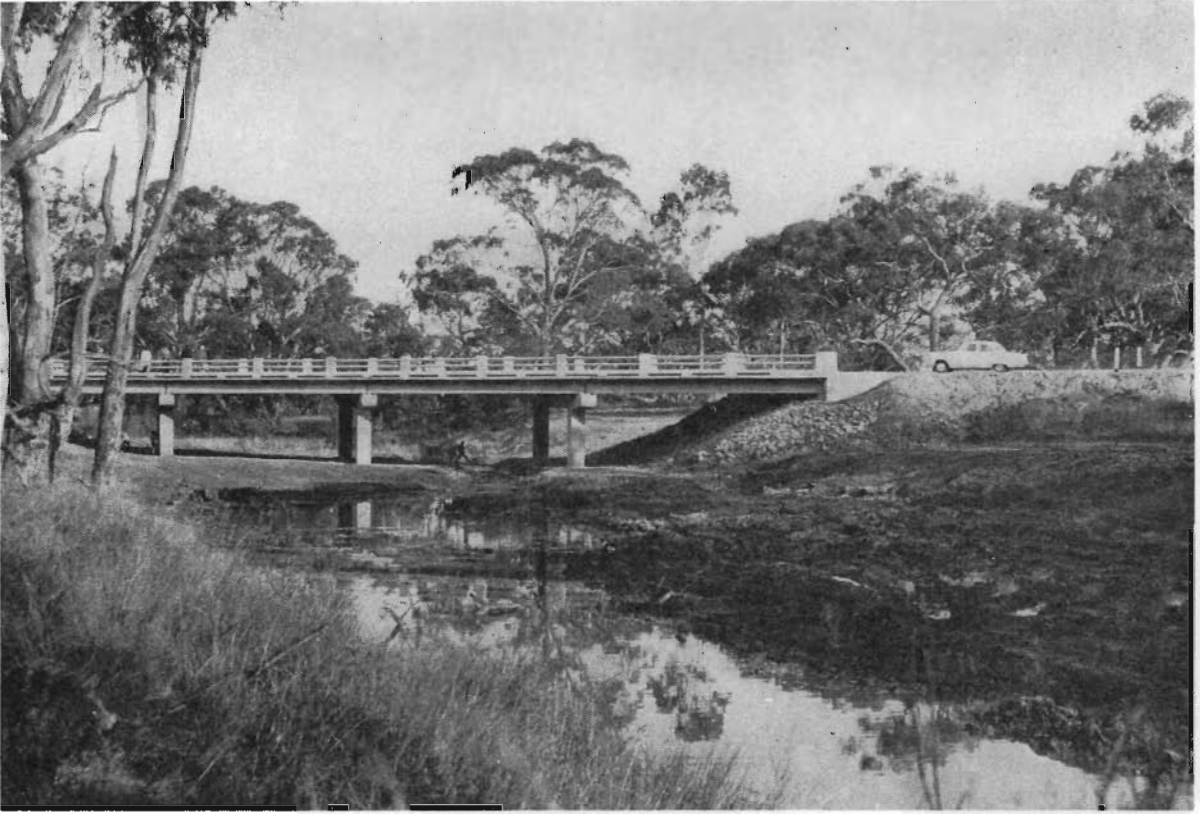
Plate 17.—The Lady Somers Bridge over Mount William Creek—The Halls Gap Road—Shire of Ararat.
