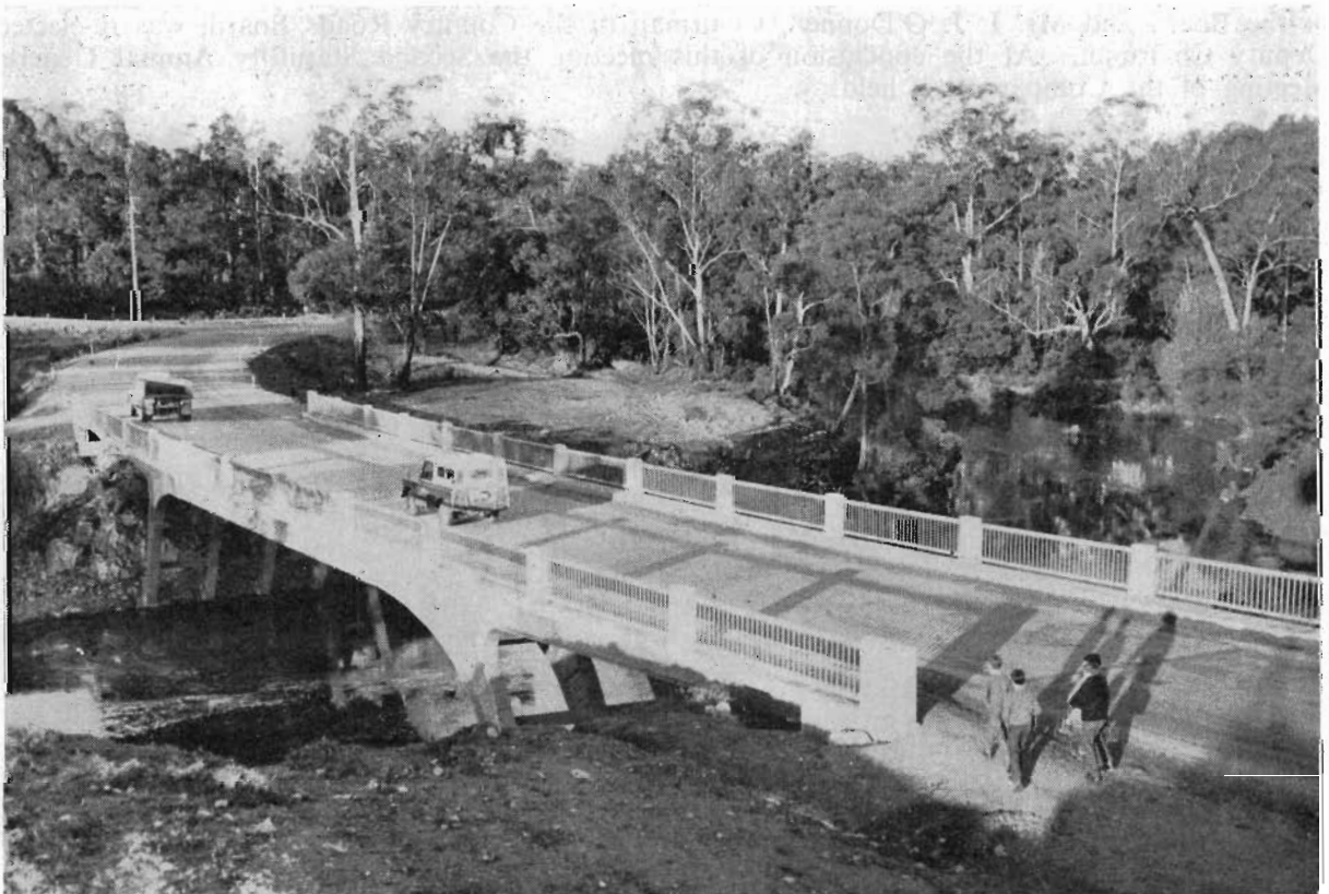
Plate 30.—New steel framed bridge with reinforced concrete deck over Boggy Creek at Nowa Nowa—Princes Highway East.
