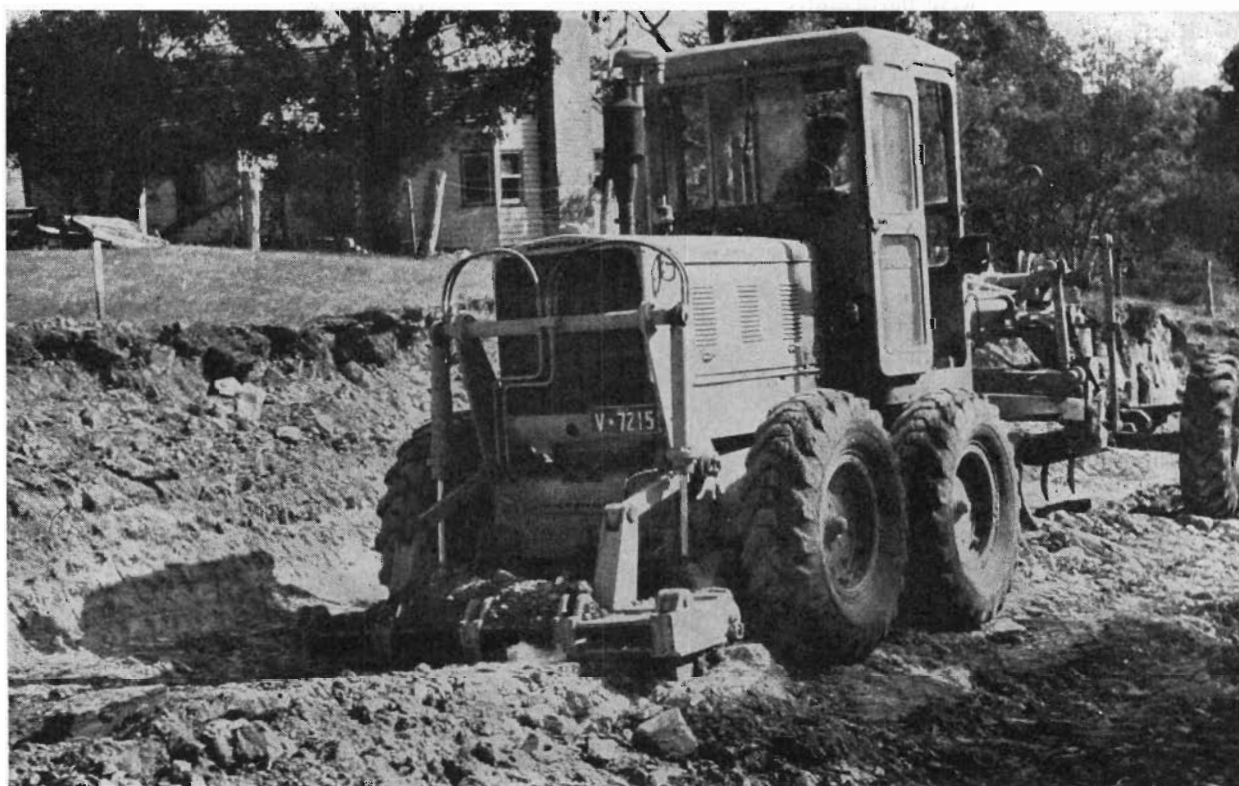
Plate 2.—Hydraulic ripper mounted on rear of power grader.
