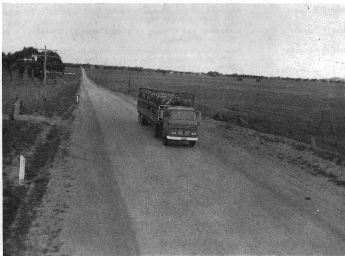
Plate 35.—Wimmera Highway—widened and resheeted section between Marnoo East and Boyles Bridge—Shire of Kara Kara.
