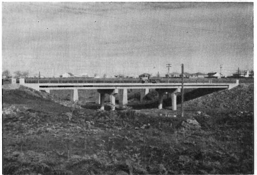
Plate 41.—City of Sunshine—new concrete bridge over Kororoit Creek on Forrest Street.
