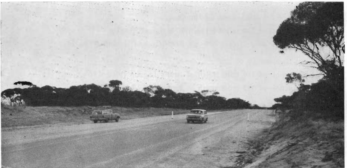
Plate 17.—Ouyen Highway—Reconstruction of 5.3 miles between Boinka and Tutye.
