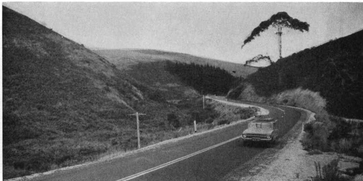
Plate 34.—South Gippsland Shire—Fish Creek—Yanakie Road—completion of final 2·3 miles.
