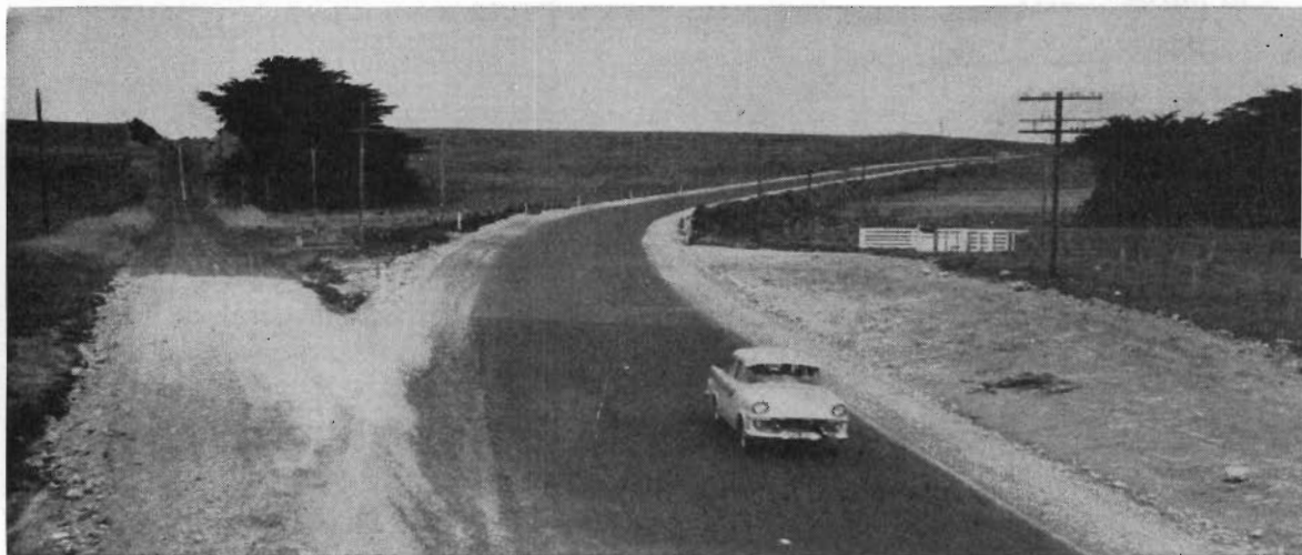
Plate 7.—Princes Highway West—Realignment at Livingston's Hill west of Tyrendarra.
