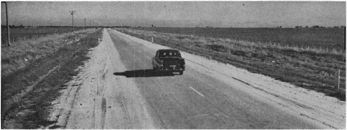
Plate 23.—Wimmera Highway—Widened section between Dooen and Murtoa.
