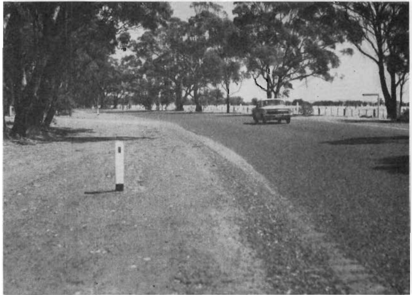
Plate 10.—Calder Highway—Reconstructed section between Marong and Leichardt.
