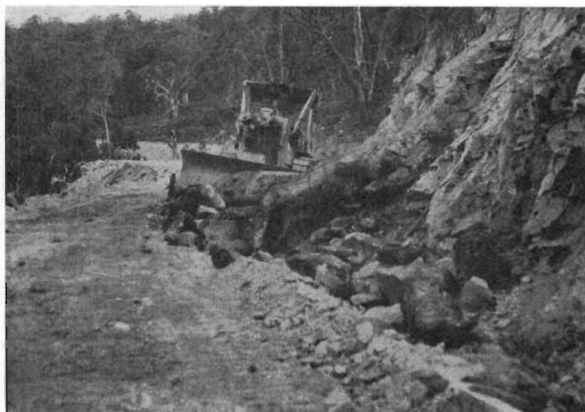
Plate 12.—Omeo Highway—Widening at Anglers Rest.
