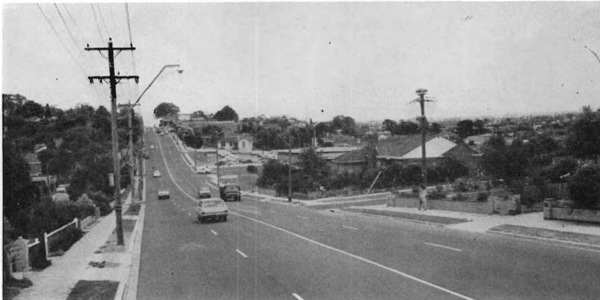
Plate 32.—Belmore Road between Wood Street and Greythorn Road, City of Camberwell.
