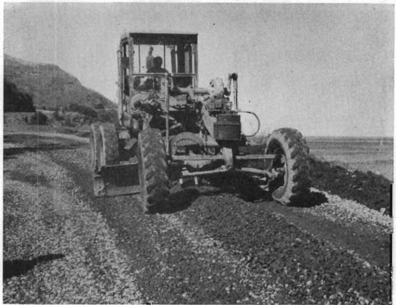
Plate 36.—Ocean Road—Construction of the approaches to the bridge at Carisbrook Creek.
