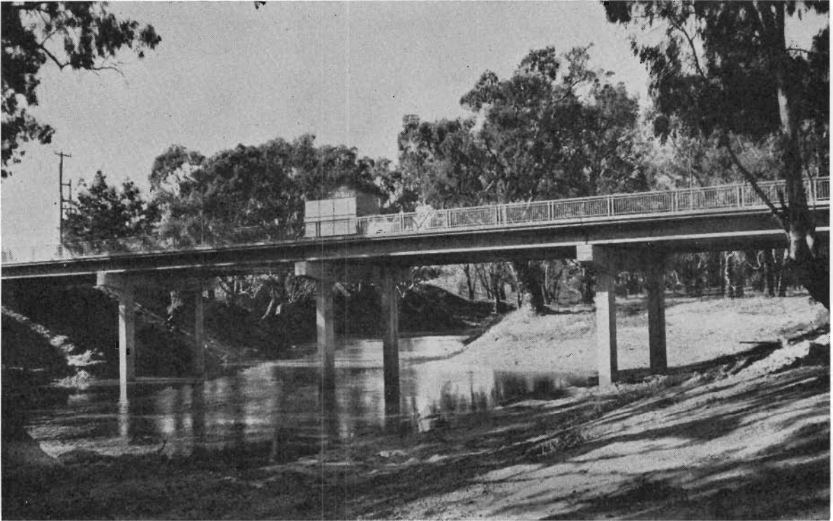
Plate 39.—New Bridge over the Campaspe River at Crossenvale, City of Echuca.
