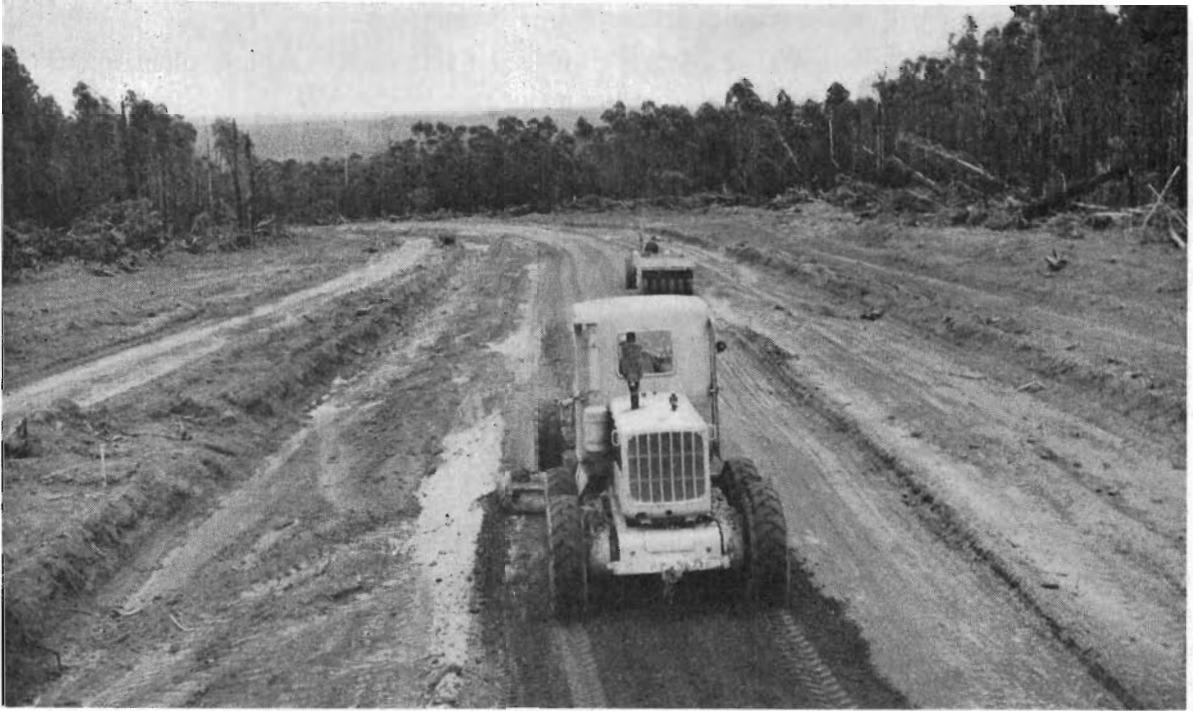
Plate 45.—Shire of Heytesbury—New road under construction near Kennedy's Creek.
