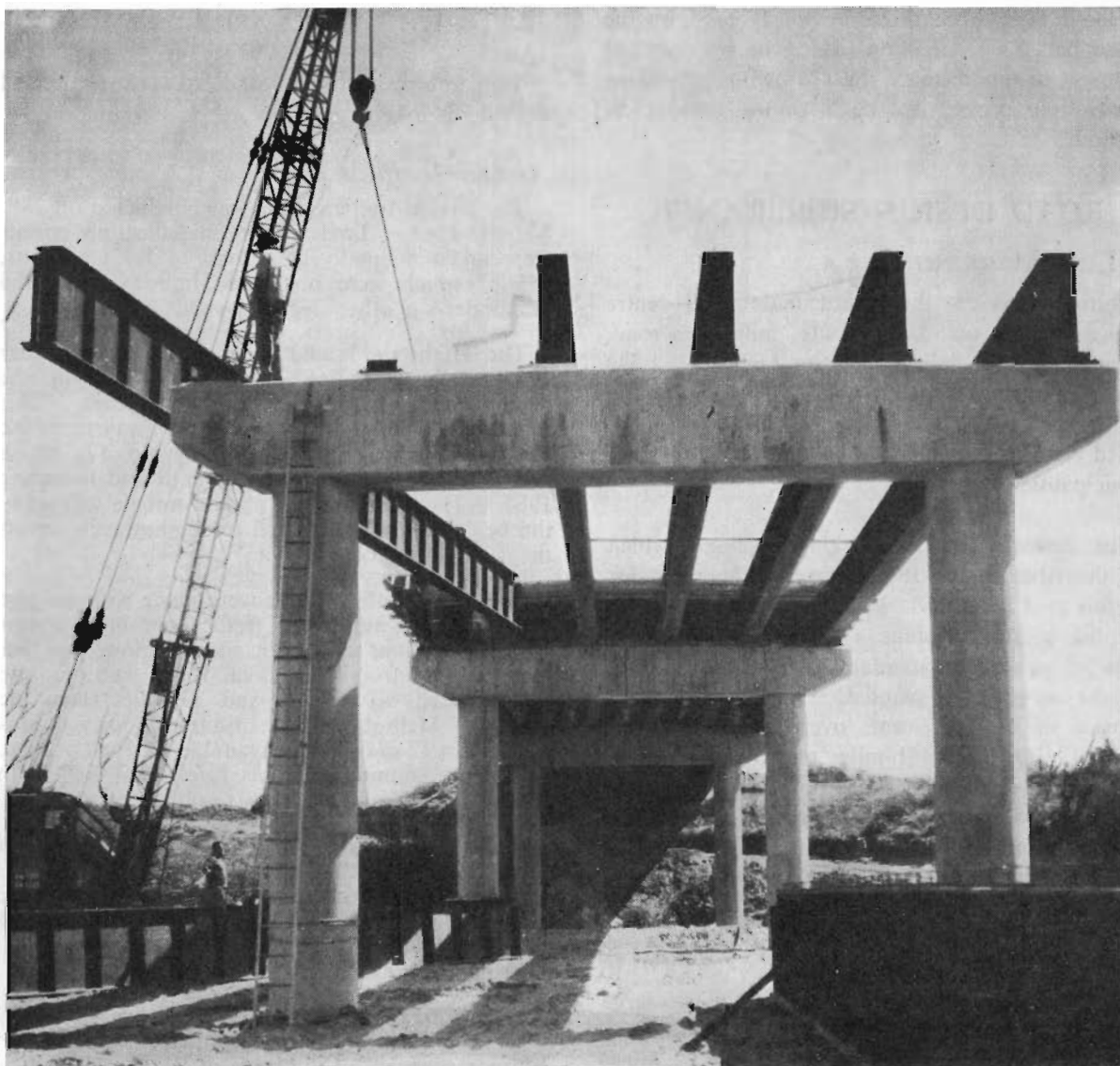
Plate 4.—Construction of Avon River Bridge at Stratford.
