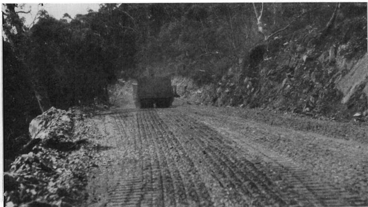
Plate 49.—Dargo High Plains Road—Work in Progress.
