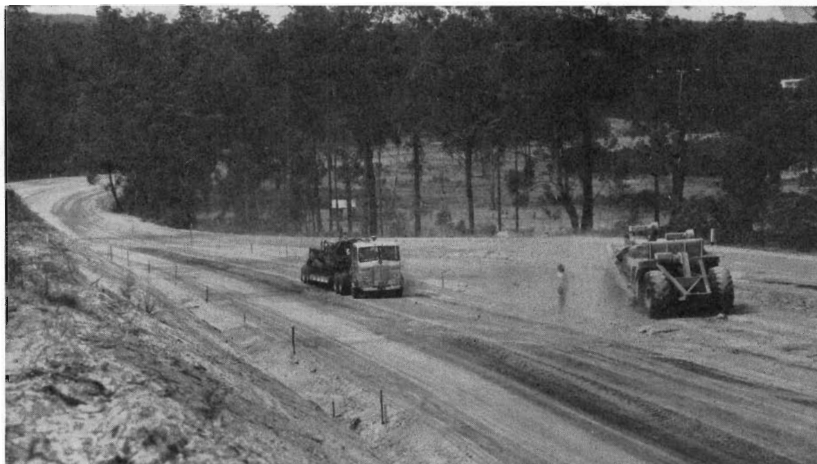
Plate 8.—Princes Highway East—Work in progress at Nowa Nowa.
