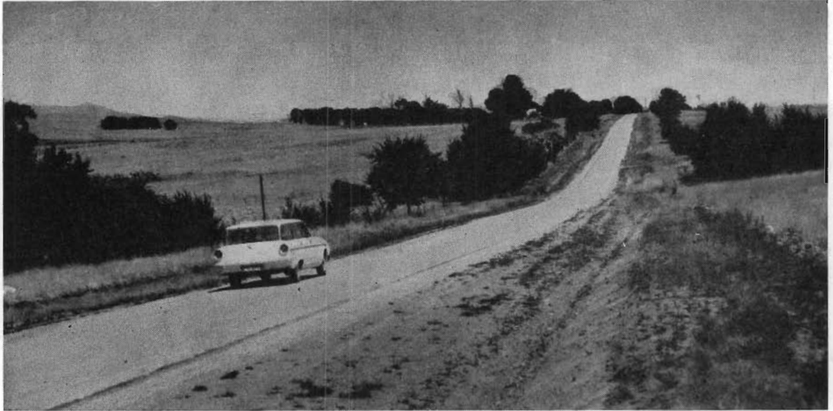
Plate 31.—Ripon Shire—Stockyard Hill Road—Reconstructed and realigned section.
