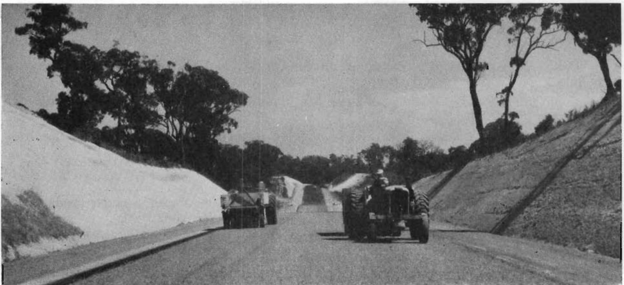
Plate 24.—Princes By-pass Road—Hernes Oak—Rolling aggregate on bitumen seal.
