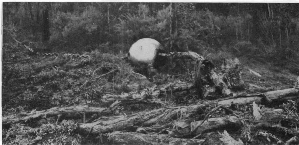
Plate 44.—Shire of Heytesbury—Clearing scrub near Coradgil with Ball and Chain.
