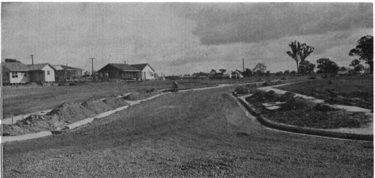
Plate 46.—Roadworks on the Seymour Housing Estate.
