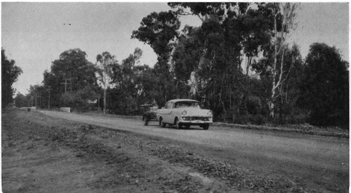
Plate 27.—Echuca City—Echuca Cohuna Road—Widened, resheeted and sealed.
