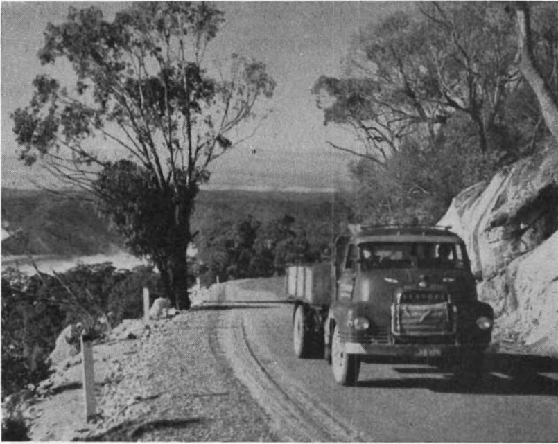
Plate 35.—Mt. Buffalo Road—Reconstructed section below Staker's Lookout.
