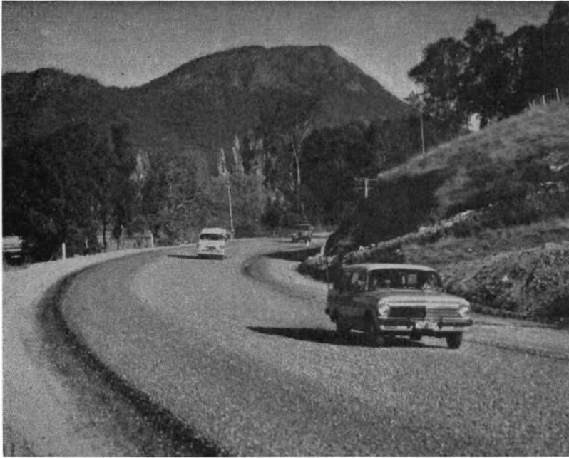
Plate 19.—Maroondah Highway— Reconstructed section near Taggerty.
