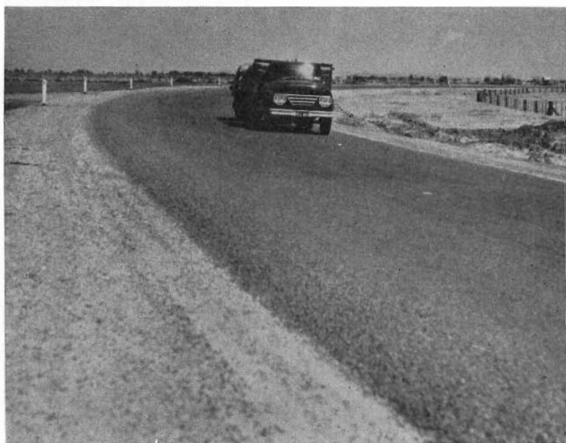
Plate 13.—Murray Valley Highway—Reconstructed section at Kerang East.
