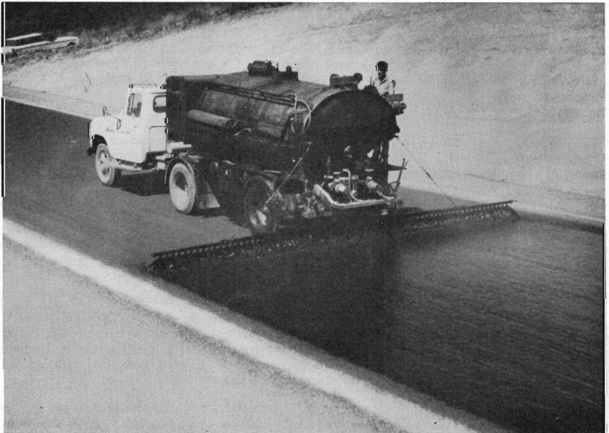
Plate 43.—Sprayer at work—Princes By-pass Road, Hernes Oak.
