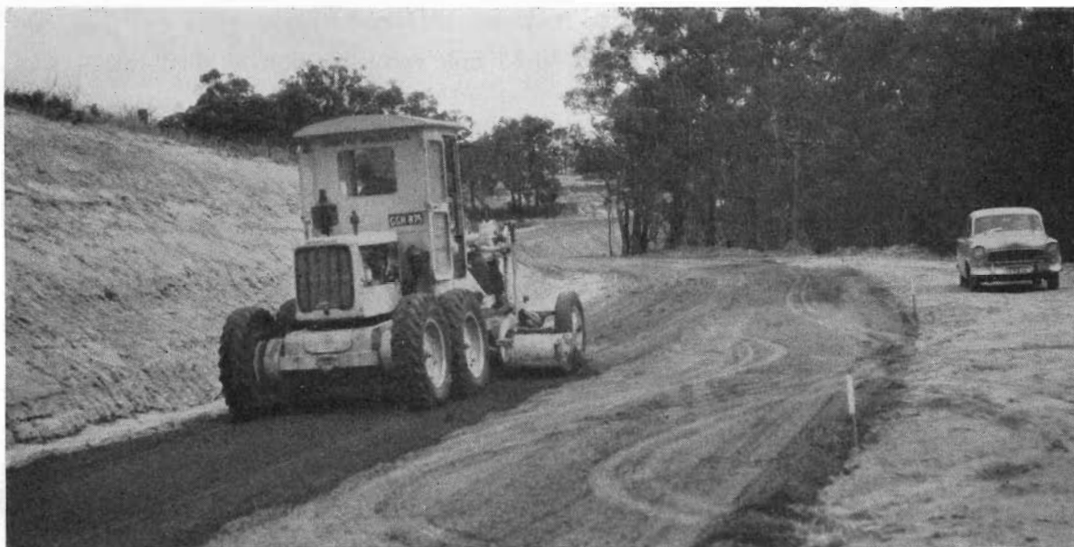
Plate 28.—Winchelsea Shire—Work in progress on the Winchelsea—Deans Marsh Road.
