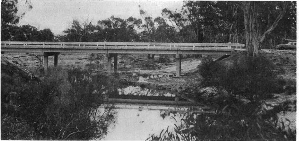
Plate 40.—Arapiles Shire—Five-span concrete bridge over the Wimmera River on Polkemet Road.
