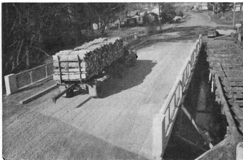
Plate 42.—Shire of Buln Buln—Four-span concrete bridge over the Latrobe River on the Loch Valley Road Noojee.
