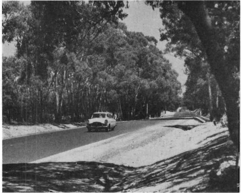
Plate 22.—Melvor Highway—Reconstructed section at Junorton.
