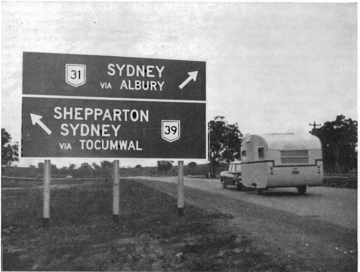
Plate 6.—Sign arrows of optimum size and proportions.
