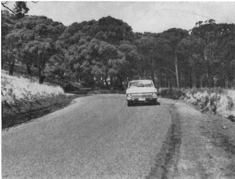
Plate 5.—Buninyong Shire—Mount Buninyong Lookout Road.—Re- constructed and sealed section of one and a half mile “up” road to Lookout.
