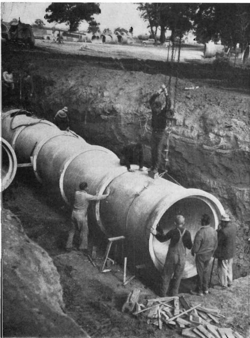
Installing twin 66-inch pipeline to carry the Campaspe No. 1 channel below the highway and railway 5 miles south of Rochester. Workmen had 37 hours between trains to complete the laying of the pipes.
