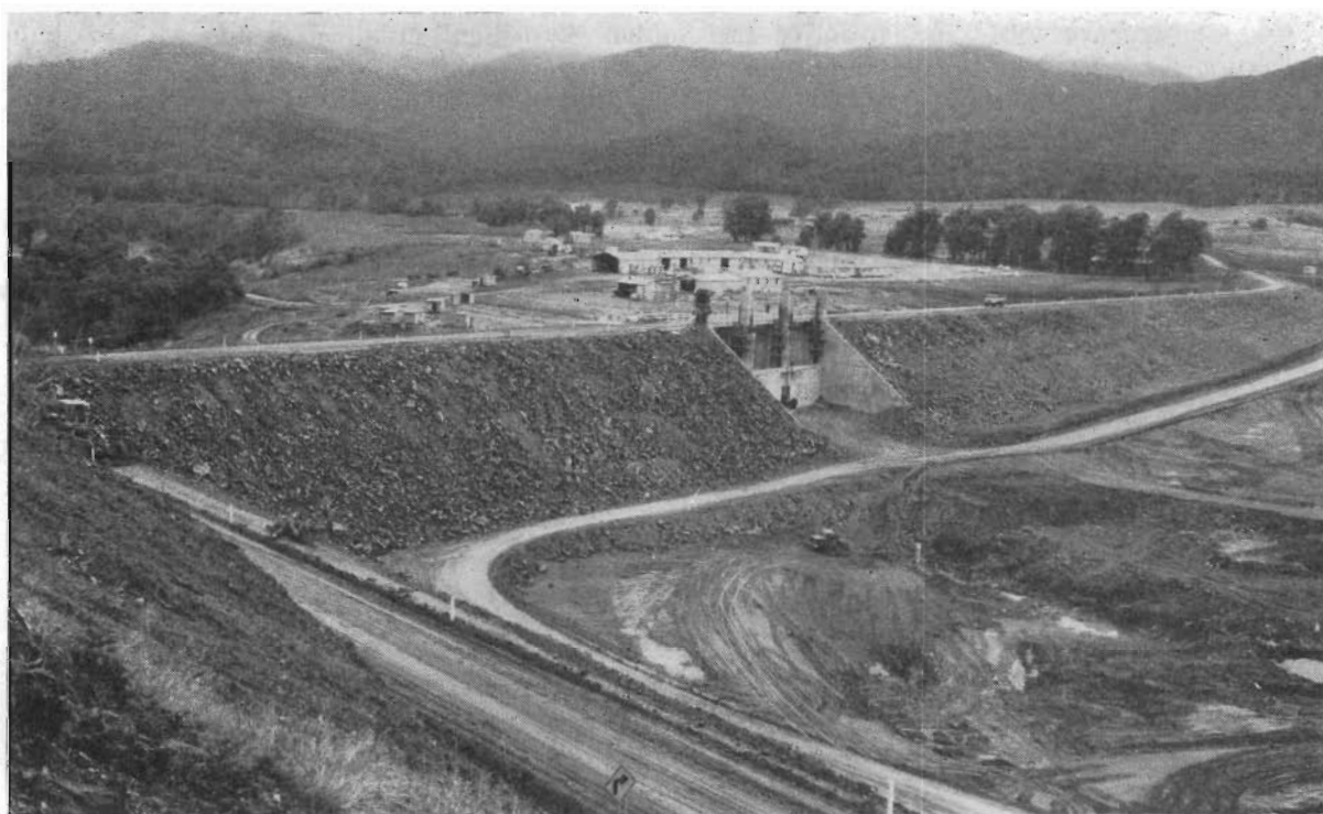
Lake Buffalo dam, first stage. This will act as the toe of the High Dam scheduled to start construction in 1968-69.
