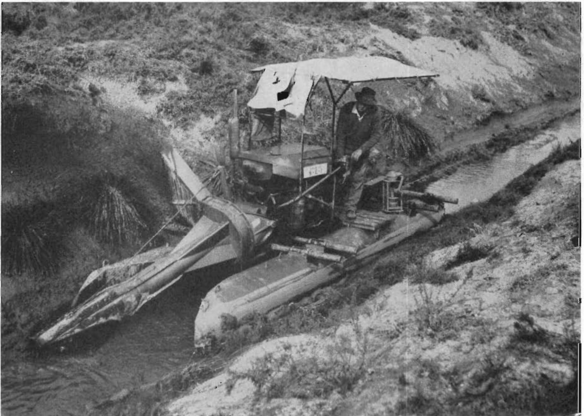
A York dredge, shown here removing silt and weed growth from a drain in northern Victoria. It was imported from Germany.
