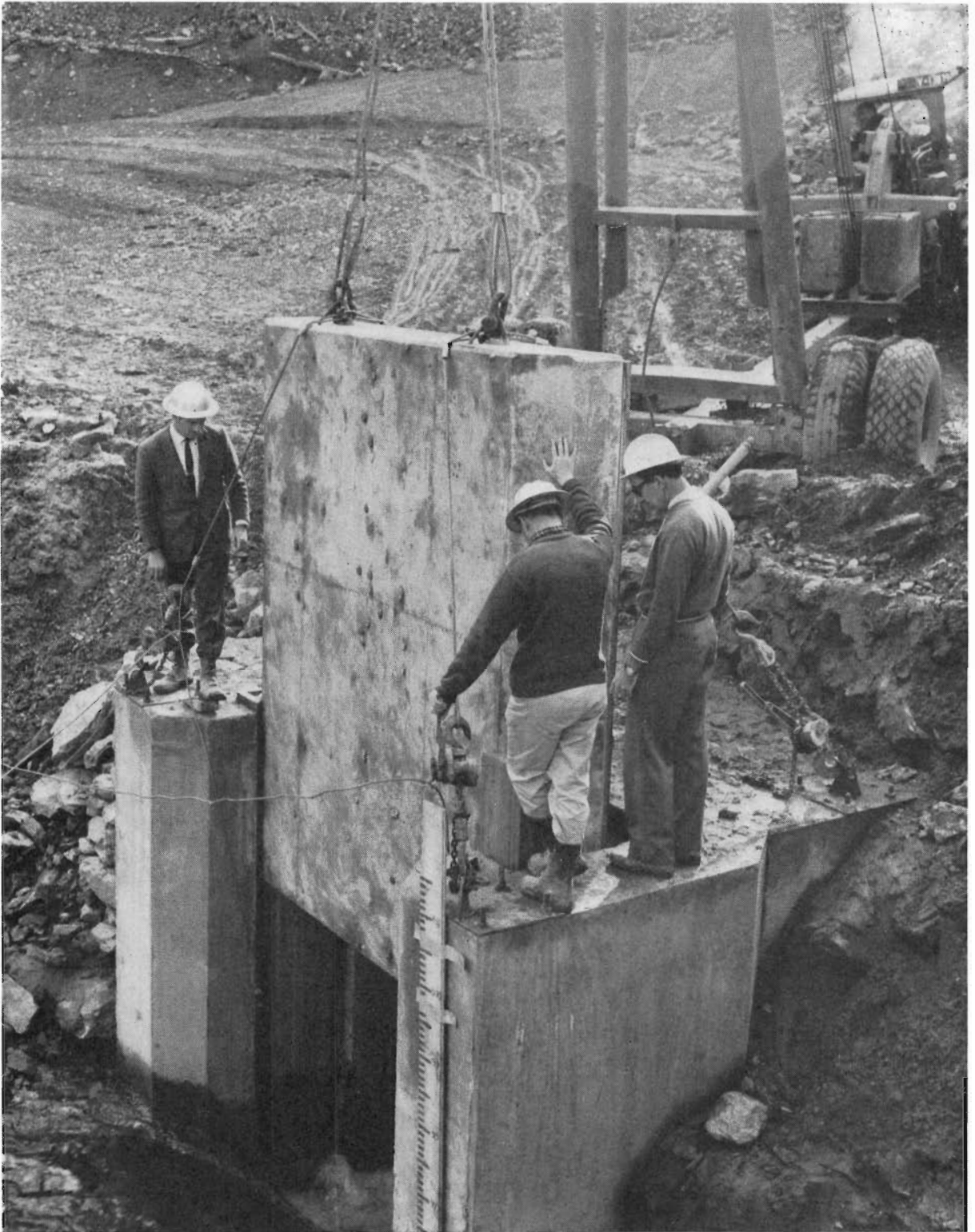
Sealing off the Lake Buffalo dam, first stage, with a 10-ton concrete plug.
