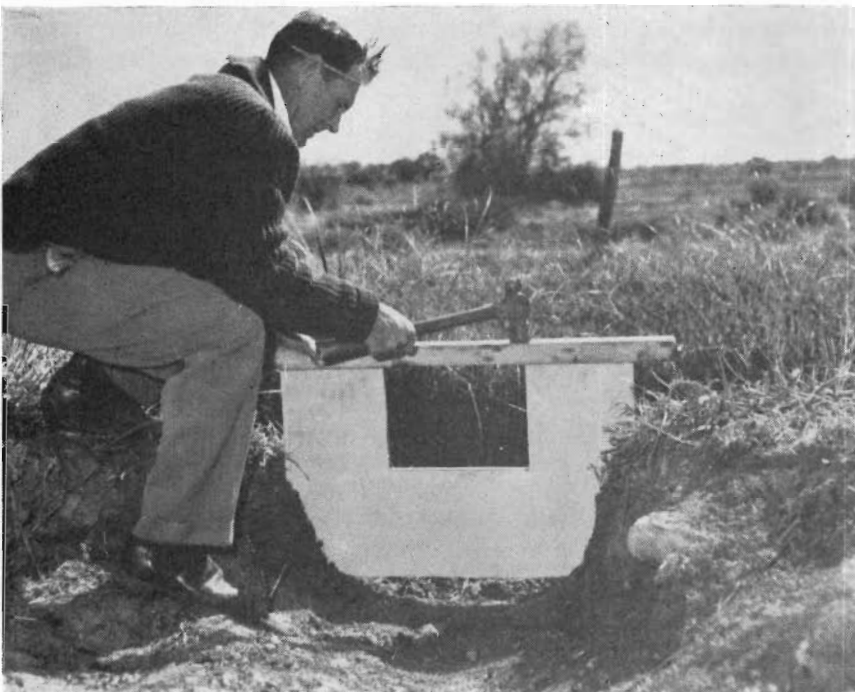
Fabricated from heavy gauge steel, this patented portable version of the original watertight seal for flow control structures developed by the Commission has been adapted for farm checks.
