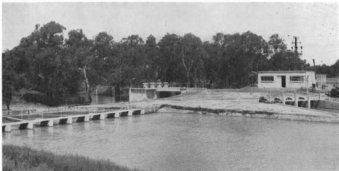
Campaspe Pumping Station which lifts water from river into Waranga Western Main Channel.
