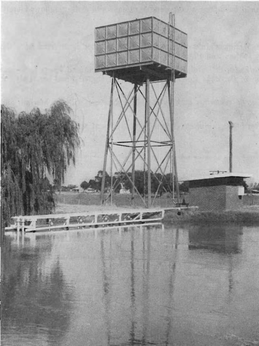
Gunbower township water tank. Capacity is 30,000 gallons and supply is from Taylor's Creek.
