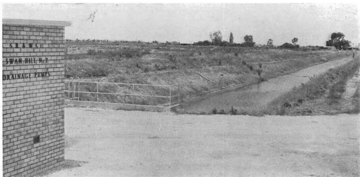
Swan Hill Flats drainage pumping station and No. 2 main drain at junction with Murray. Pumps lift water from drain into river when river level is above drain level.
