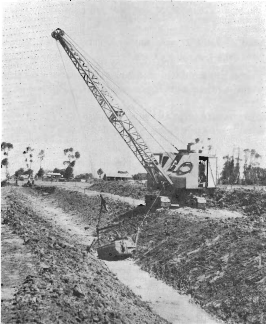
Excavating No. 2 main drain, Swan Hill Flats drainage scheme.
