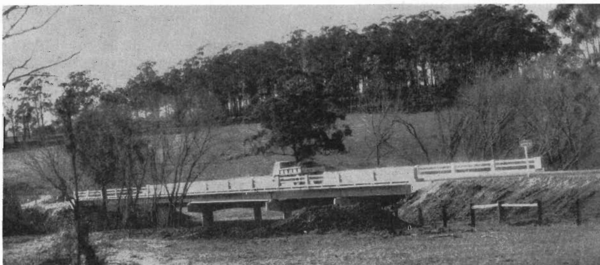
Plate 41.—Pre-stressed concrete beam and reinforced concrete bridge over the Latrobe River—Shire of Narracan.
