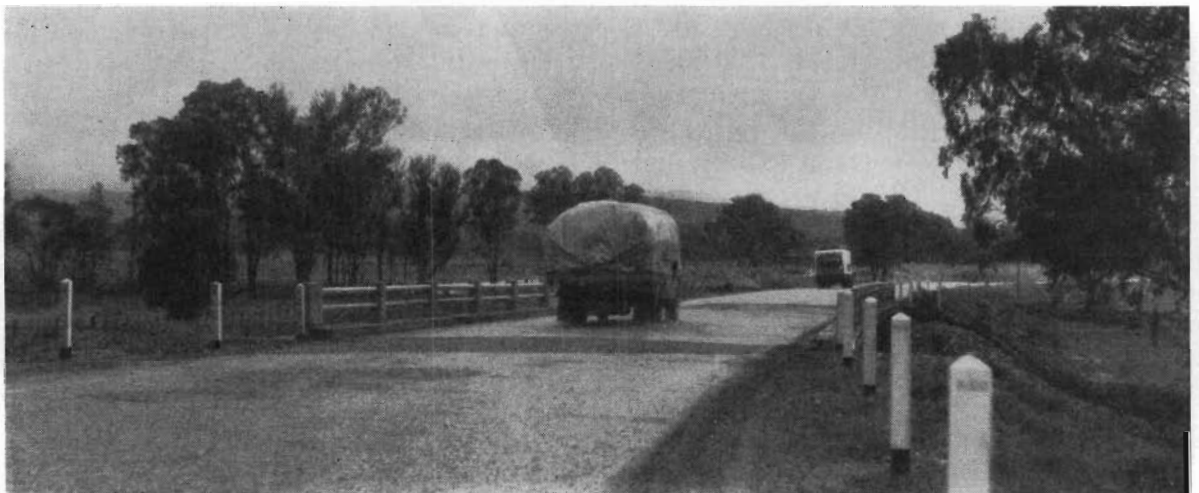
Plate 21.—Hume By-pass Road—New bridge over Black Dog Creek.
