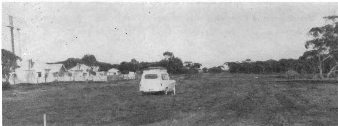
Plate 16.—Ouyen Highway—Tutye Deviation before construction.
