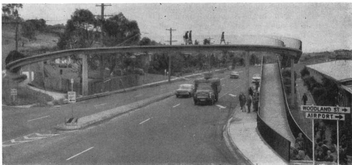
Plate 43.—Strathmore Pedestrian Over-pass—Pascoe Vale Road—City of Broadmeadows.
