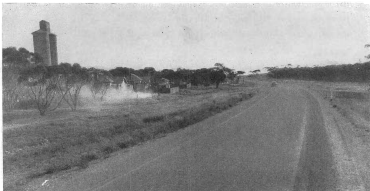
Plate 17.—Ouyen Highway—Realignment at Tutye completed.
