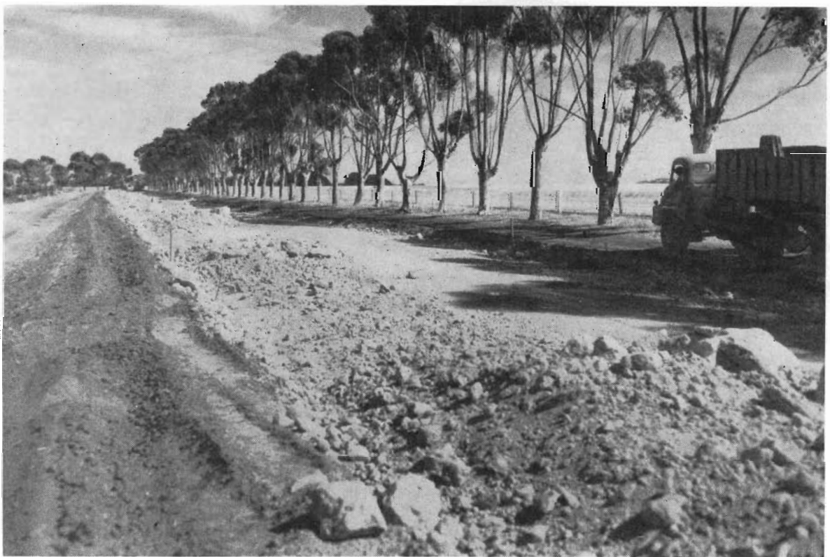
Plate 45.—Reconstruction and sealing of the road to Longerenong Agricultural College.
