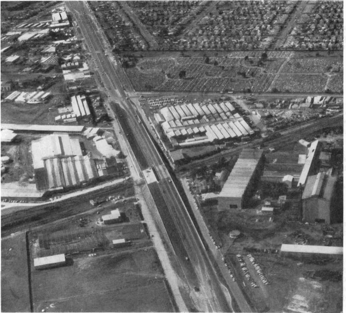
Plate 47.—Road over rail over-pass—Princes Highway West—Brooklyn.
