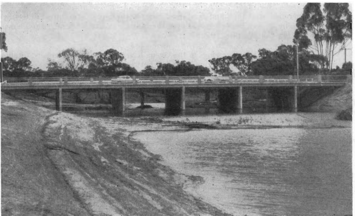
Plate 38.—North-Western Highway—Bridge over the Richardson River, Donald.
