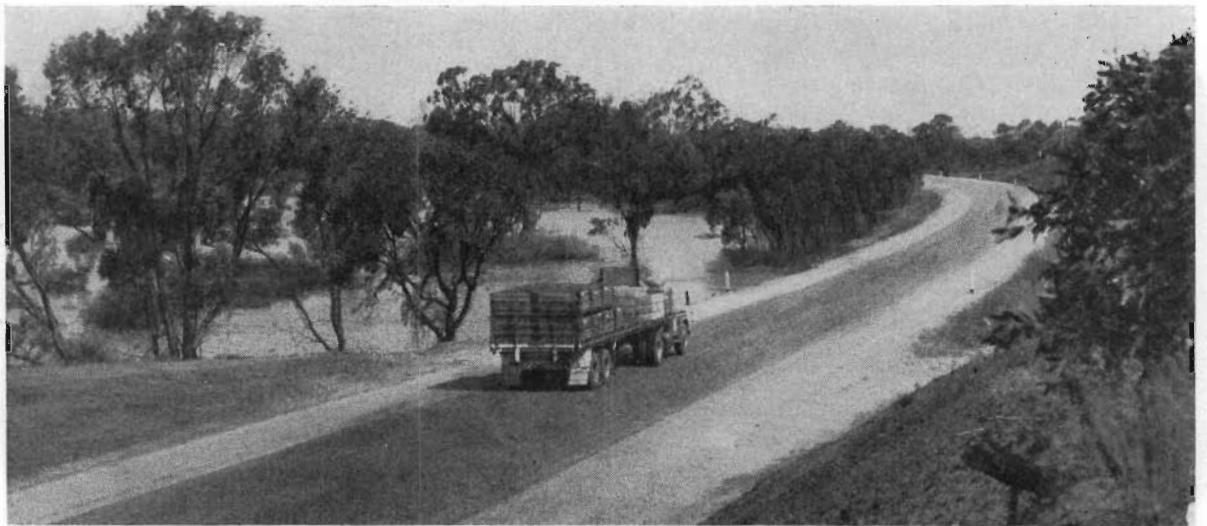
Plate 14. Murray Valley Highway—New construction between Piambie and Boundary Bend.
