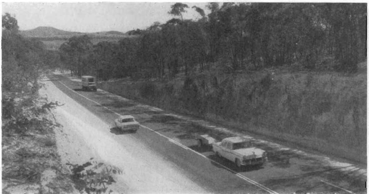
Plate 9.—Western Highway—Reconstruction at Box's Cutting near Beaufort.
