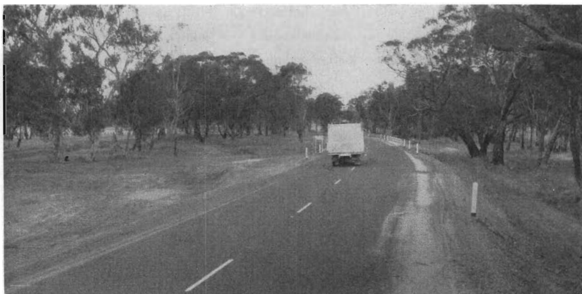
Plate 12.—Northern Highway—Realignment at Mt. Pleasant Creek.
