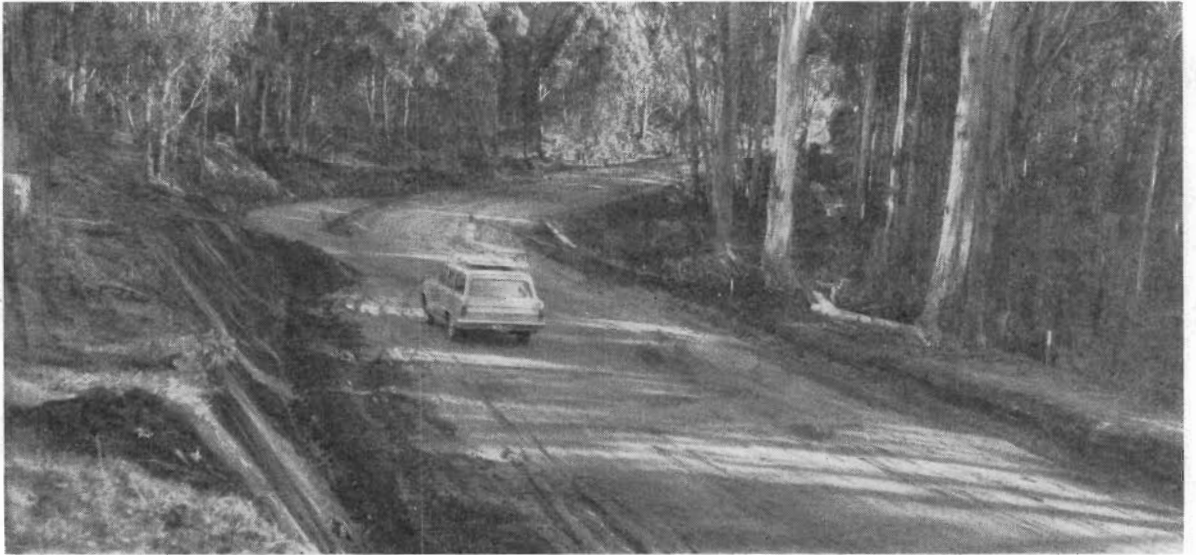
Plate 23.—Daylesford-Trentham Road—Reconstruction and realignment—Shire of Glenlyon.
