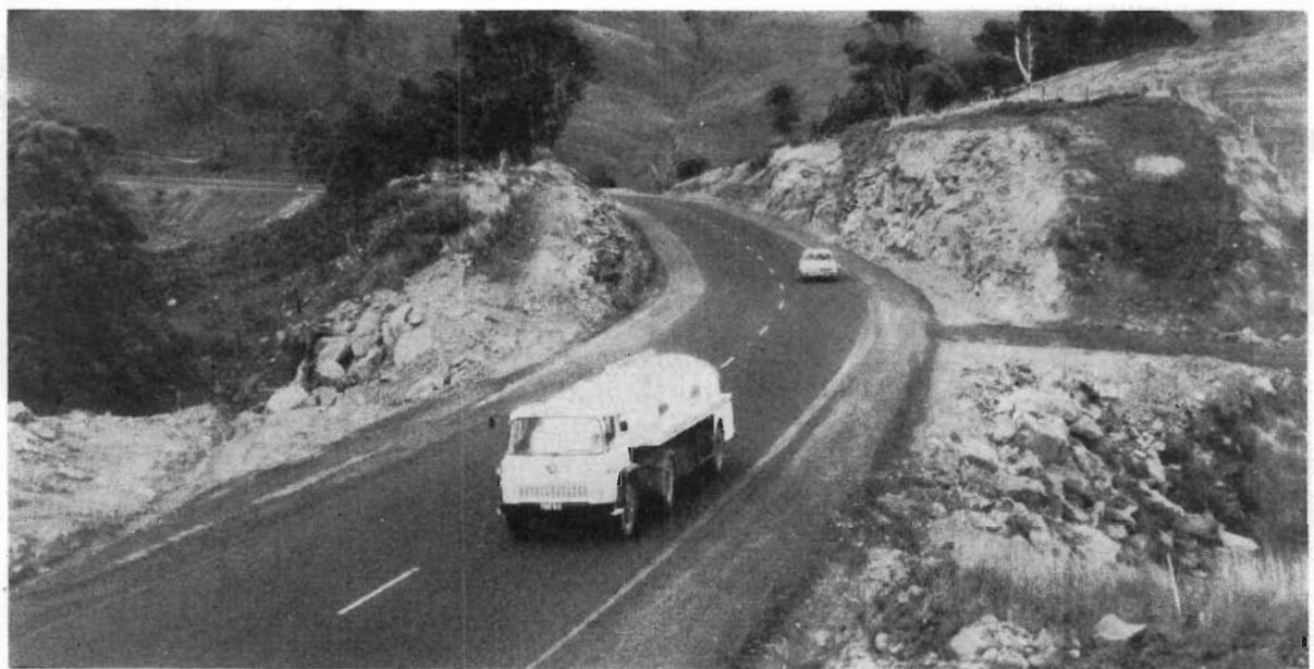
Plate 15.—South Gippsland Highway—Silkestone Hill, Korumburra.
