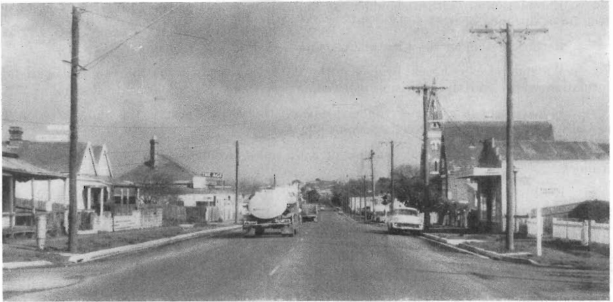
Plate 7.—Princes Highway West—Reconstruction in the City of Colac.
