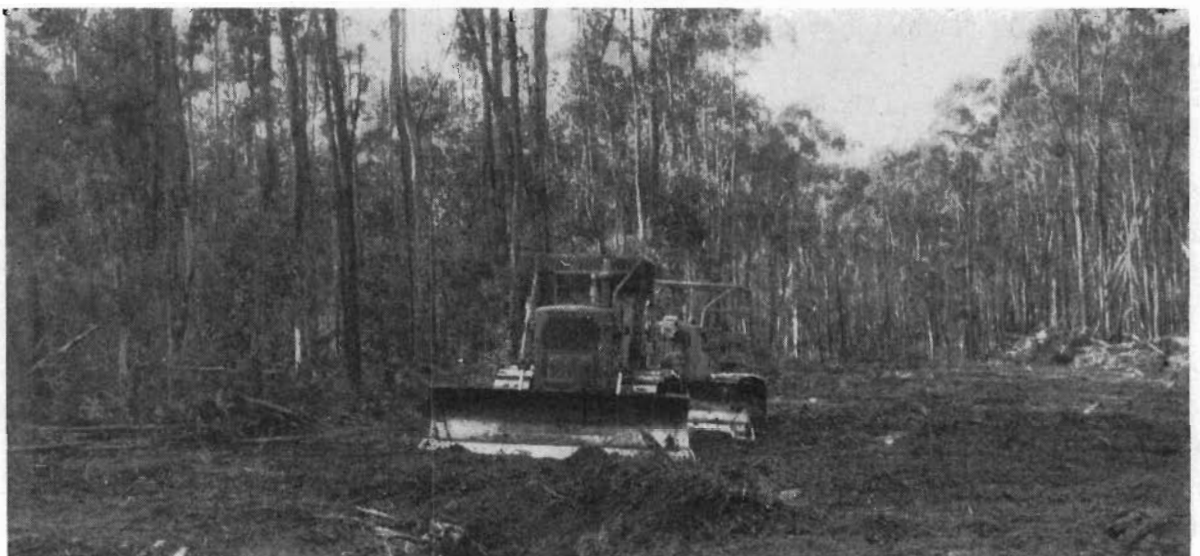
Plate 27.—Yarra Glen-Yea Road under construction—Healesville and Yea Shires.
