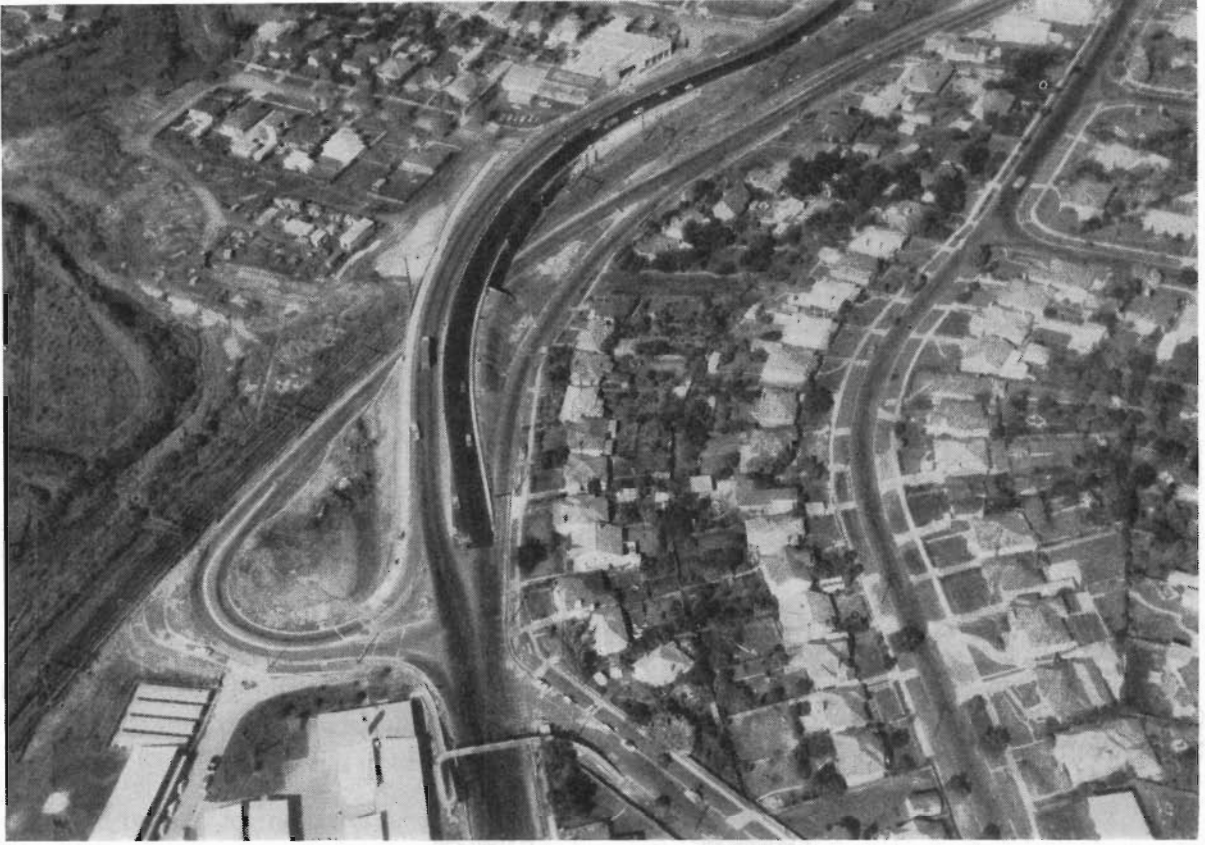
Plate 46.—Road over rail over-pass at Strathmore—City of Broadmeadows.
