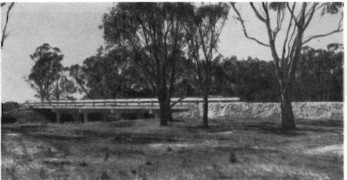
Plate 33.—Drung-Longerenong Road—Bridge over Wimmera River—Shire of Wimmera.
