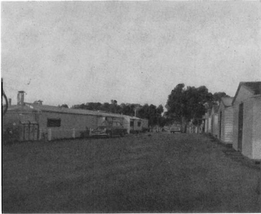
Plate 49.—Board's camp at Carrum Downs showing living huts.
