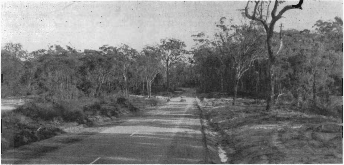
Plate 34.—Mallacoota Road—Resheeted and sealed section.
