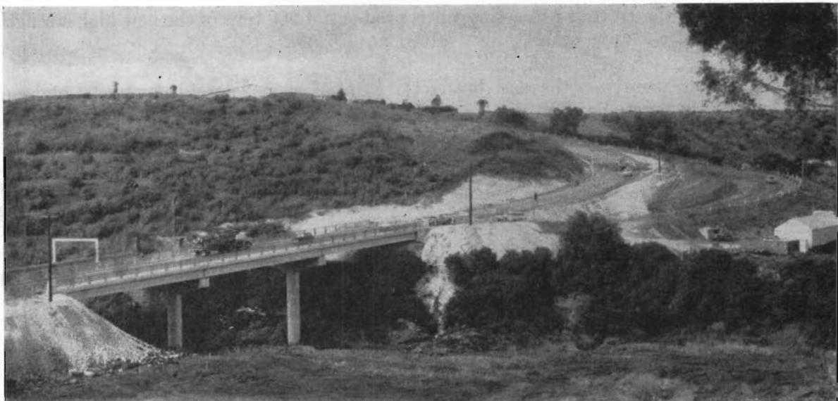
Plate 42.—Calder Highway—Bridge over the Maribyrnong River—City of Keilor.
