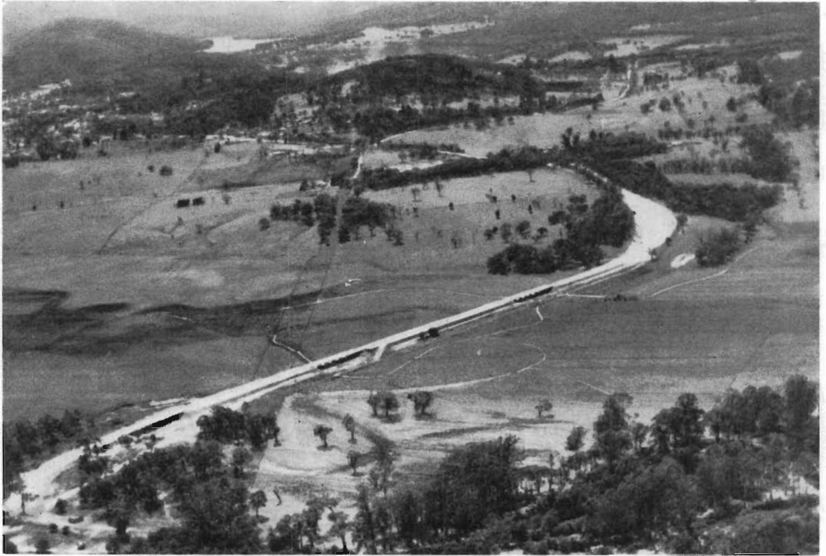
Plate 19.—Maroondah Highway—New construction at Yarra Flats.
