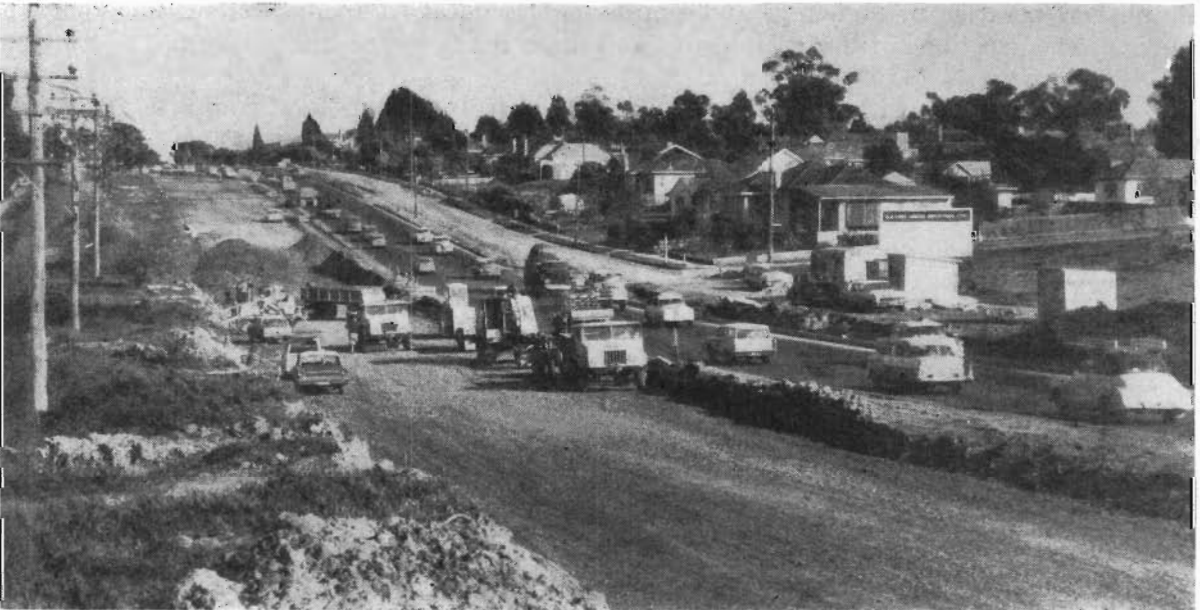
Plate 3.—Maroondah Highway—Duplication in progress between Mitcham and Ringwood.
