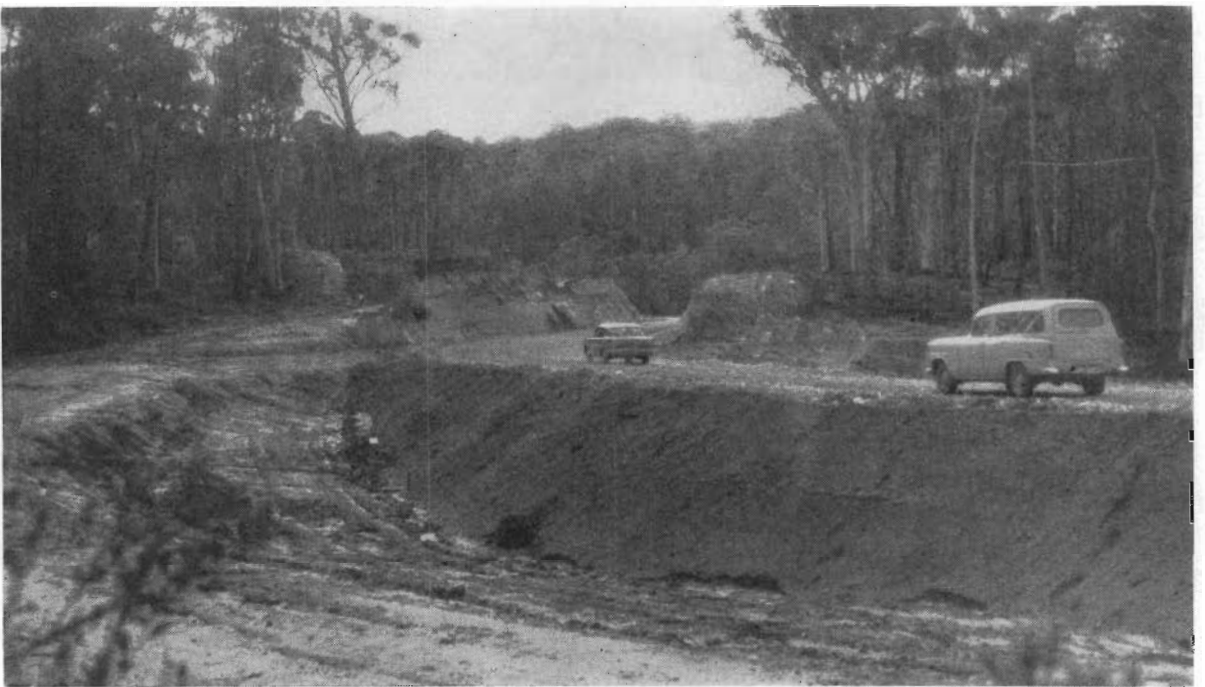
Plate 24.—Tallangatta-Corryong Road—Reconstruction—Shire of Towong.
