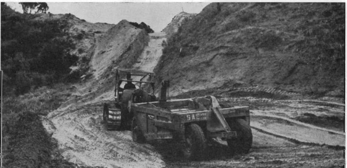
Plate 35.—South Gippsland Shire. Promontory Road—section through the sand hills under construction.
