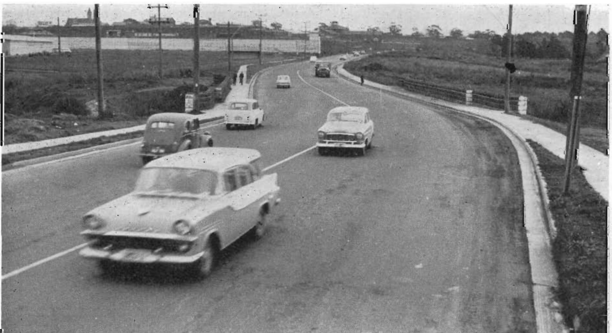
Plate 29.—Coburg City. Murray Road—Widened bridge over Merri Creek.
