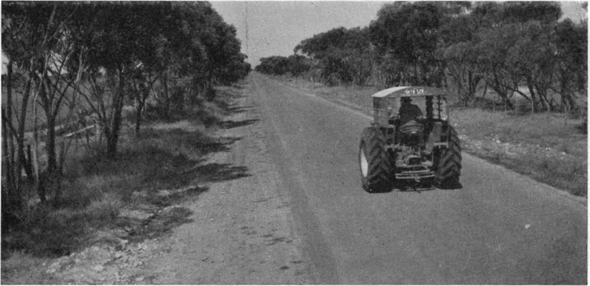
Plate 27. Birchip Shire. Berrwillock-Birchip Main Road. Reconstructed and sealed section.
