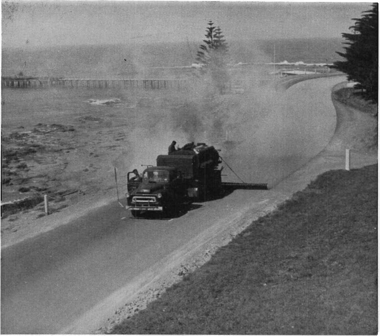
Plate 38.—Winchelsea Shire. Ocean Road—sealing in progress on widened section at Lorne.
