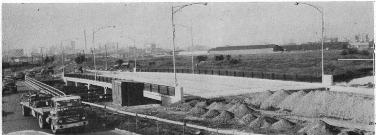
Plate 52.—Special Project—City of Melbourne—New Footscray Road—Coal Canal bridge during construction.
