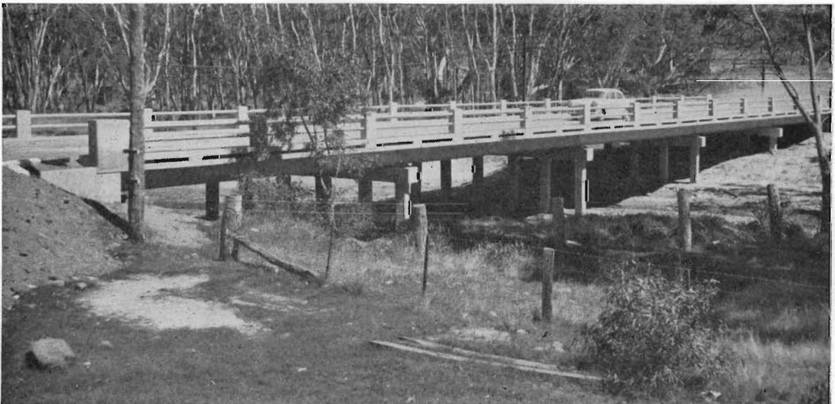
Plate 28.—Wannon Shire. Natimuk—Hamilton Main road—New bridge over Mathers Creek.
