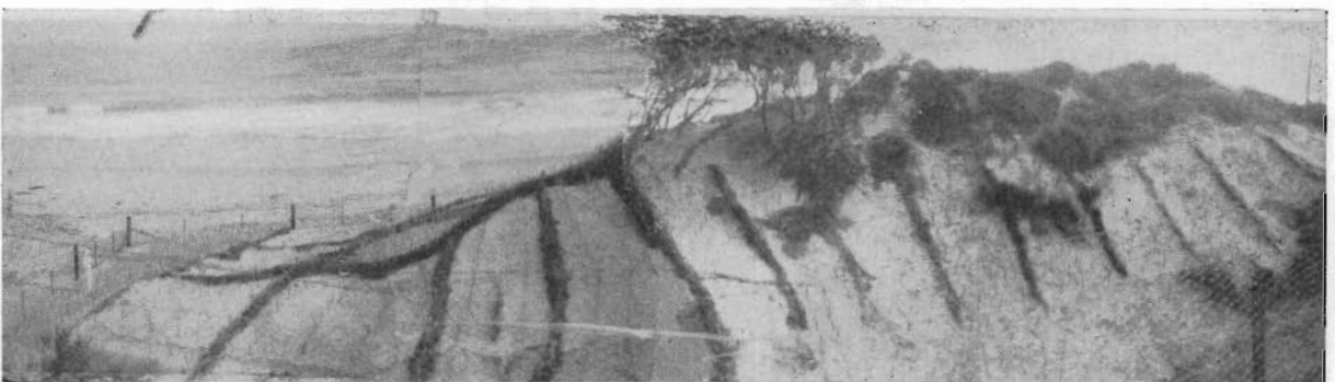
Plate 8.—The condition of the work on the 3rd June, 1963. Showing the reconditioned tea-tree fences, the vigorous growth of the native vegetation and the extensive replanting of marrum and spinifex grasses.
