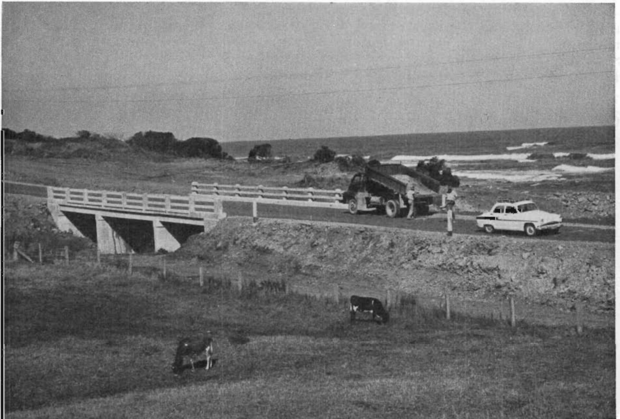
Plate 39.—Otway Shire. Ocean Road—new bridge over Sugarloaf Creek.
