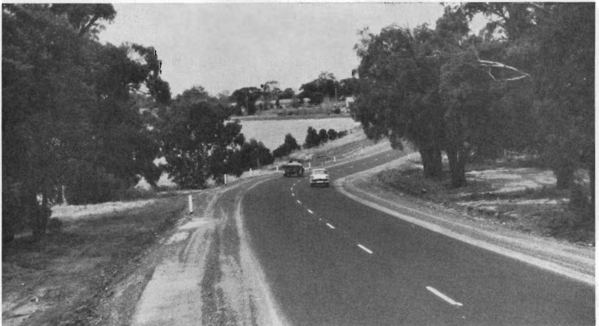
Plate 11.—Calder Highway—Reconstructed former corduroy section through the Black Forest, between Macedon and Woodend.
