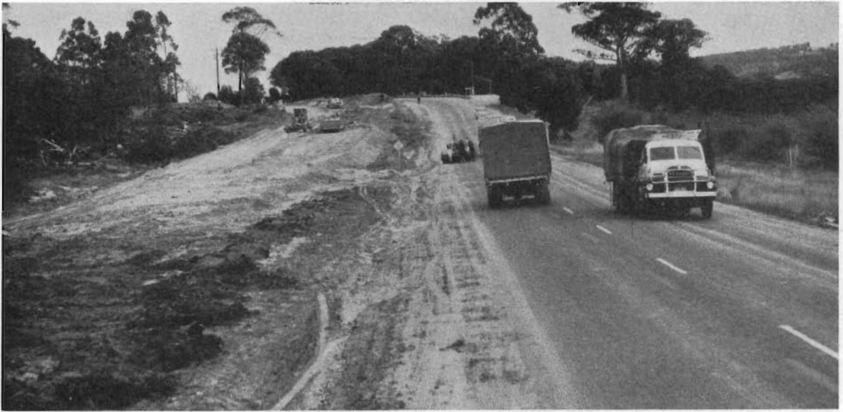
Plate 10.—Western Highway. Section being duplicated at Woodmans Hill. East of Ballarat.
