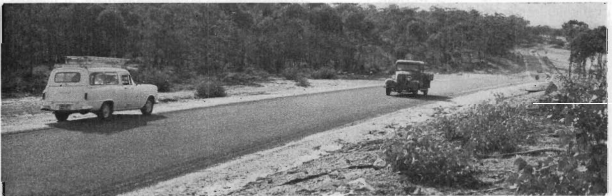
Plate 50.—State Rivers and Water Supply—Kimbolton Forest Road—Widened and sealed section on new alignment necessitated by construction of the Eppalock Weir.
