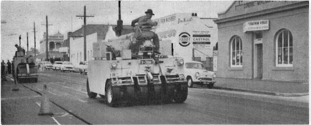
Plate 49.—Warrnambool City. Princes Highway West. Laying bituminous asphalt surface.
