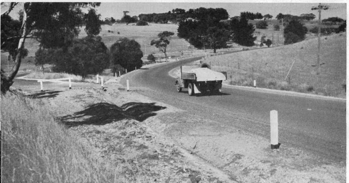
Plate 25 and 26.—Barrabool Shire. Anglesea Main Road. Realignment at Bellbrae. Above—before. Below—after.
