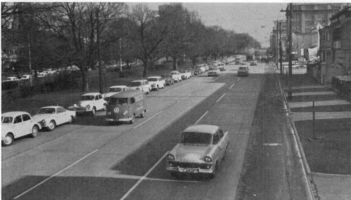
Plate 30 and 31.—Fitzroy City. Victoria Parade—Brunswick Street to Smith Street—before and after reconstruction.
