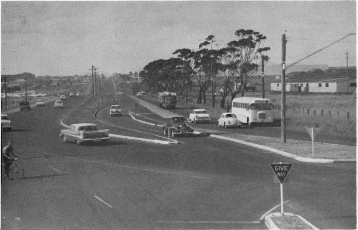
Plate 7.—Princes Highway West Section 1.—Divided Highway at Separation Street North Geelong looking north.
