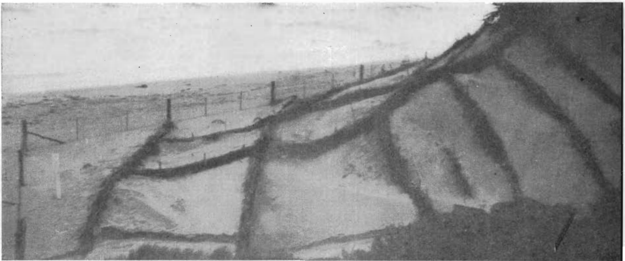
Plate 7.—The work at the Northern end of the dunes, 15 May, 1963. All tea-tree fences have been lifted and thickened with additional brush and three more fences have been laid at right angles to the original fences to prevent sand entering the gully.
