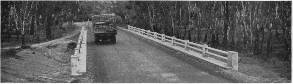
Plate 23.—Cobram Shire. Cobram—Yarrowonga Main Road. New six-span bridge over Murray River Flats at Cobram.
