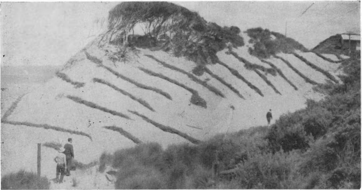
Plate 6.—Brush fences laid at 20-ft. intervals on the Northern end of the dunes. 30 October, 1962.
