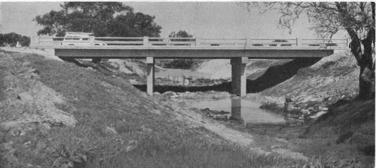
Plate 22.—Wimmera Highway Section 2. New bridge over Wallaloo Creek.
