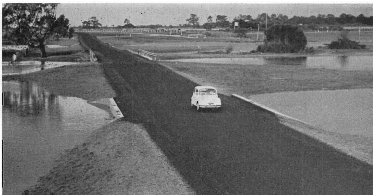
Plate 32.—Alberton Shire. Pound Road East—New culverts and bridge on new alignment over Tarra River, east of Yarram.
