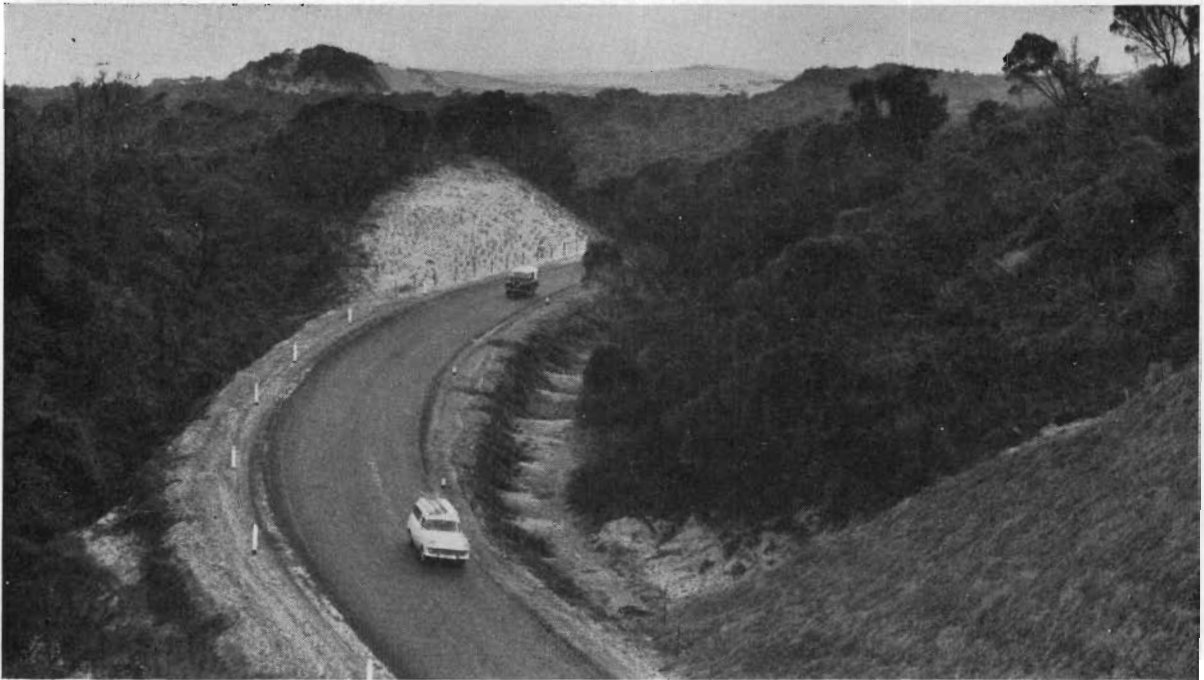
Plate 33 and 34.—South Gippsland Shire. Promontory Road—Section through the sand hills at "The Canyon" before and after reconstruction.
