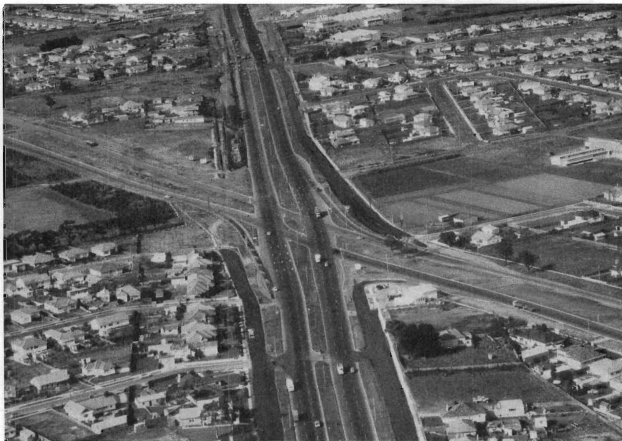
Plate 12.—Aerial view of Princes Highway East and North Road, Clayton, Intersection with adjacent service roads.
