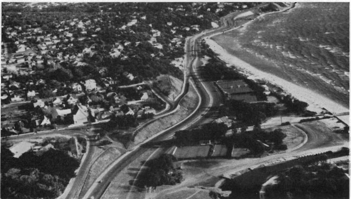
Plate 3.—Nepean Highway. Duplication approaching Olivers Hill. Shire of Frankston.
