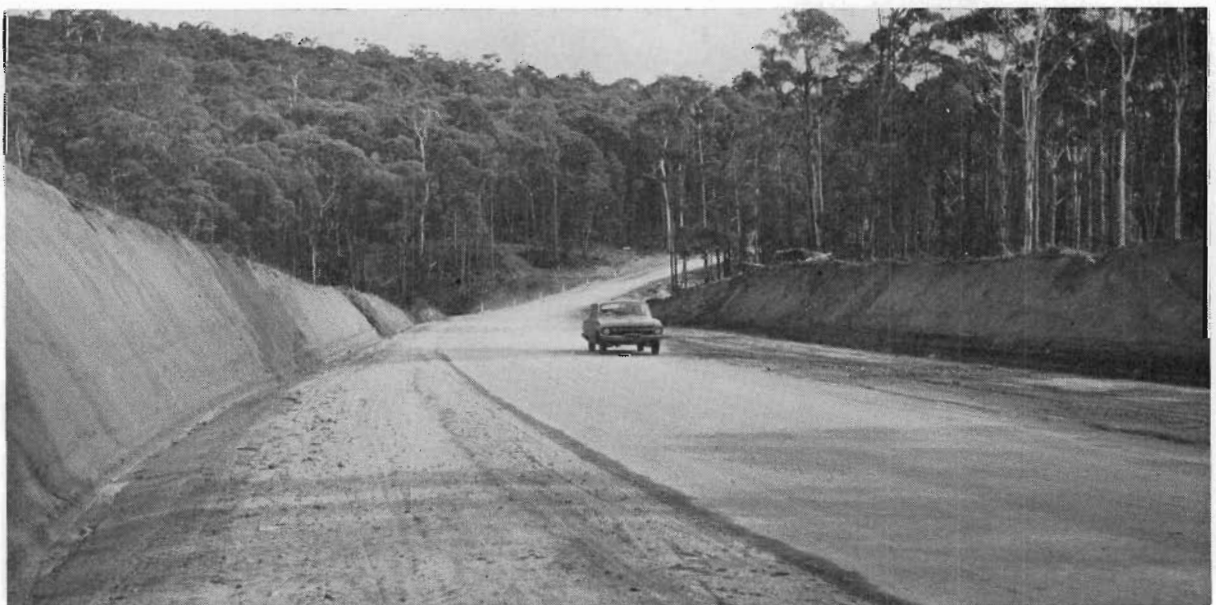
Plate 6.—Tallangatta—Corryong Road. Reconstructed section near Boggy Creek. Shire of Towong.
