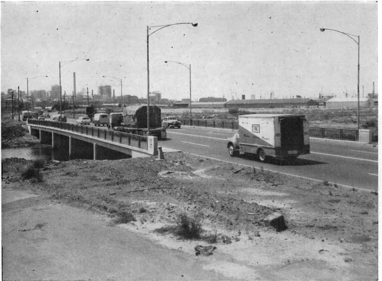
Plate 10.—Coal Canal Bridge—New Footscray Road.
