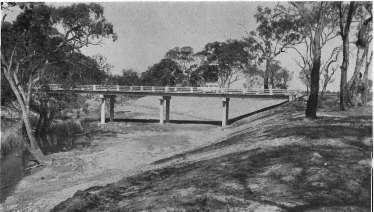
Plate 48.—Kara Kara Shire. Bendigo—St. Arnaud Road—Logan's bridge over Avoca River.
