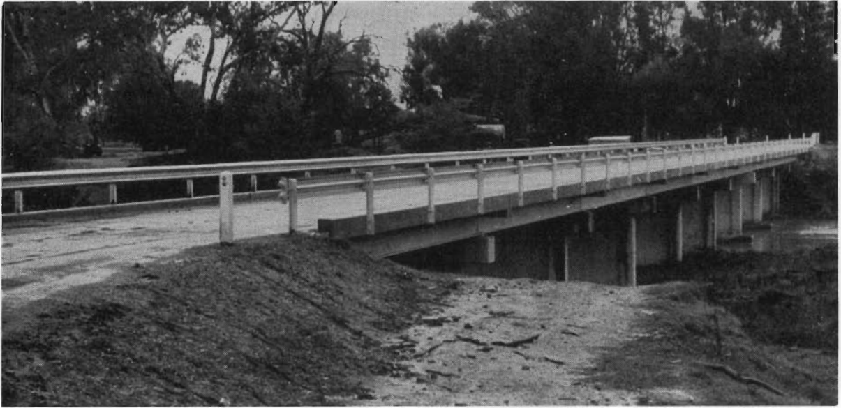
Plate 46.—Wangaratta and Oxley Shires. Tarrawingee—Milawa Road—new nine-span bridge over the Ovens River.
