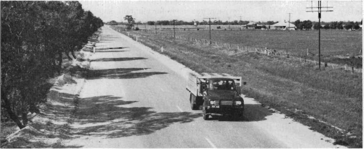
Plate 20.—North Western Highway—Widened section south of Kinnabulla.
