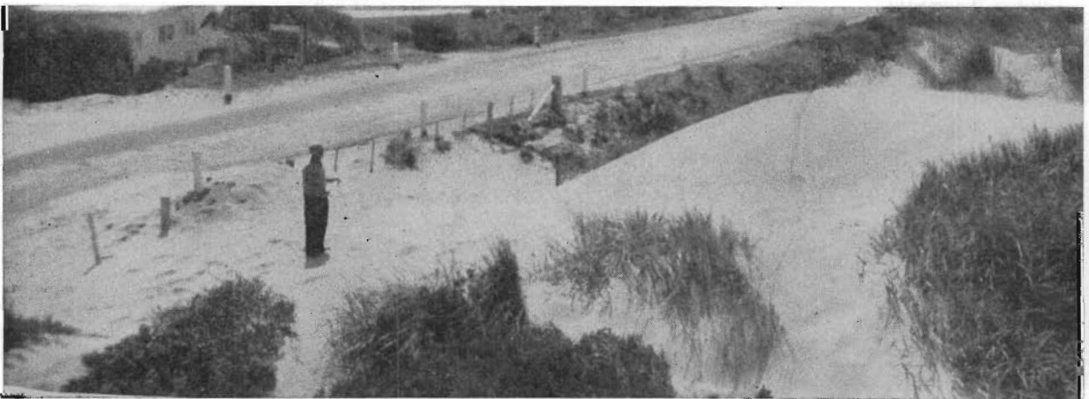
Plate 5.—Looking North at the leeward side of the dunes showing movement of sand over fence and onto the road pavement.
