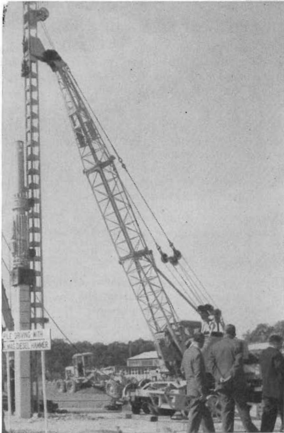
Plate 11 "Delmag" D 12 Diesel Pile Hammer
