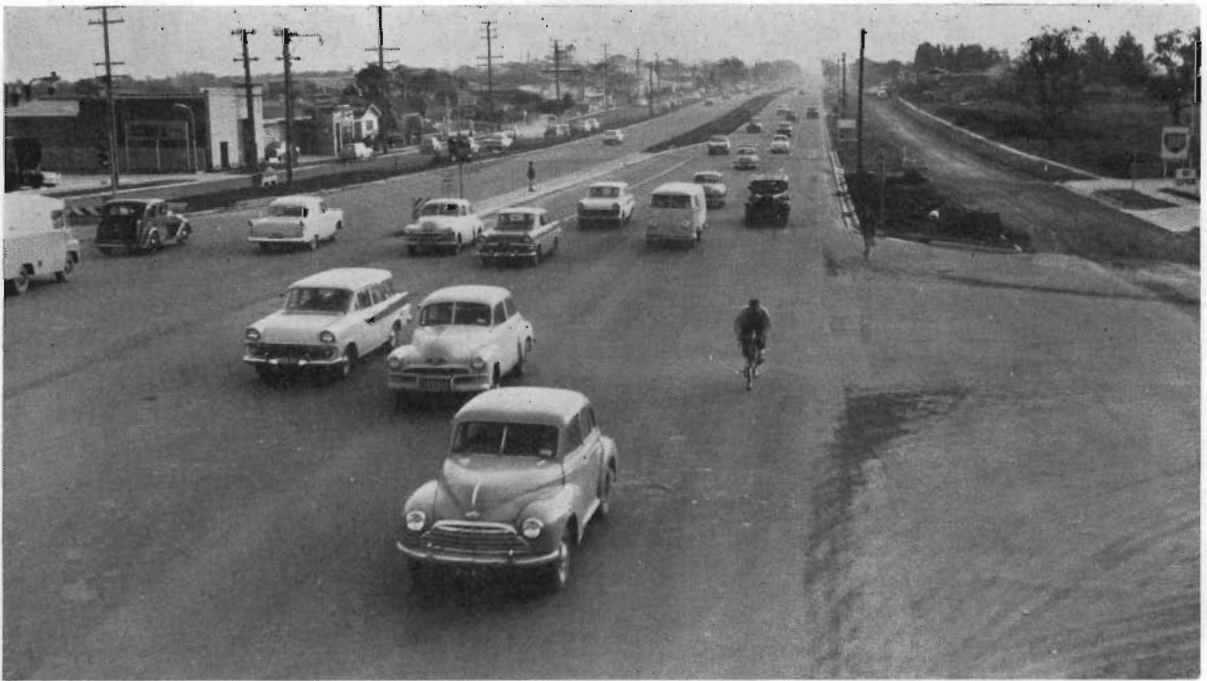
Plate 2.—Maroondah Highway—Duplication at Springvale Road intersection. City of Nunawading.
