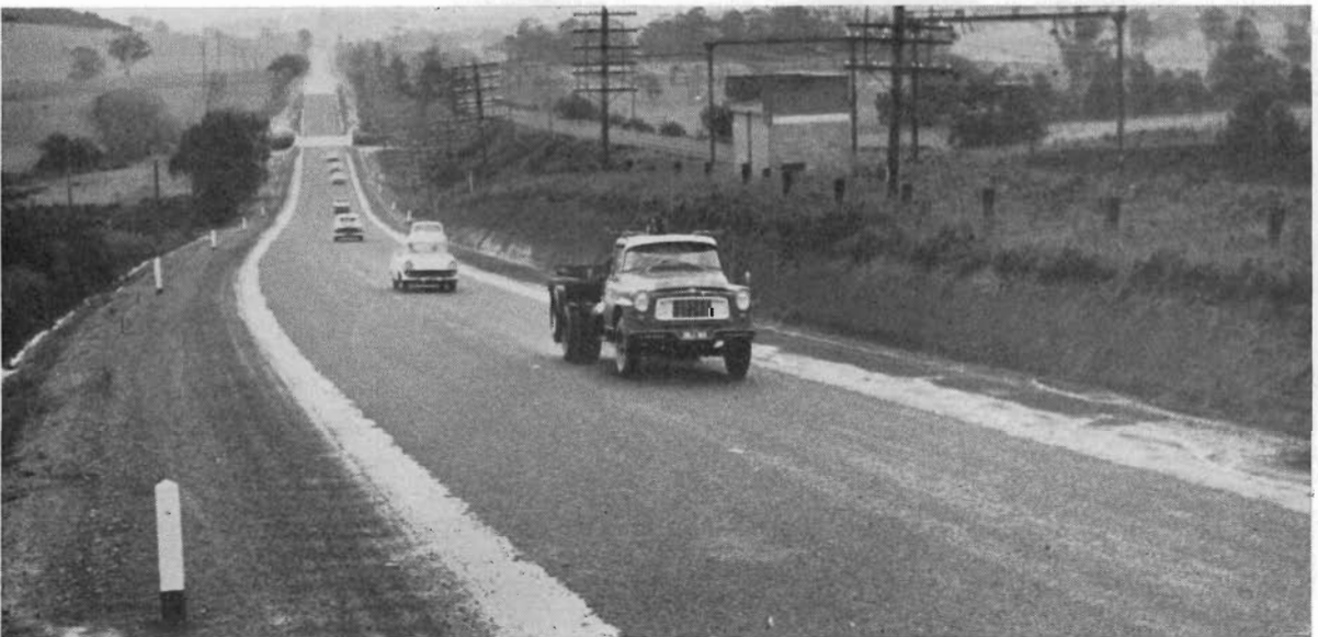
Plate 9.—Princes Highway East Section 2. Widened and reconstructed section near Darnum. Warragul Shire
