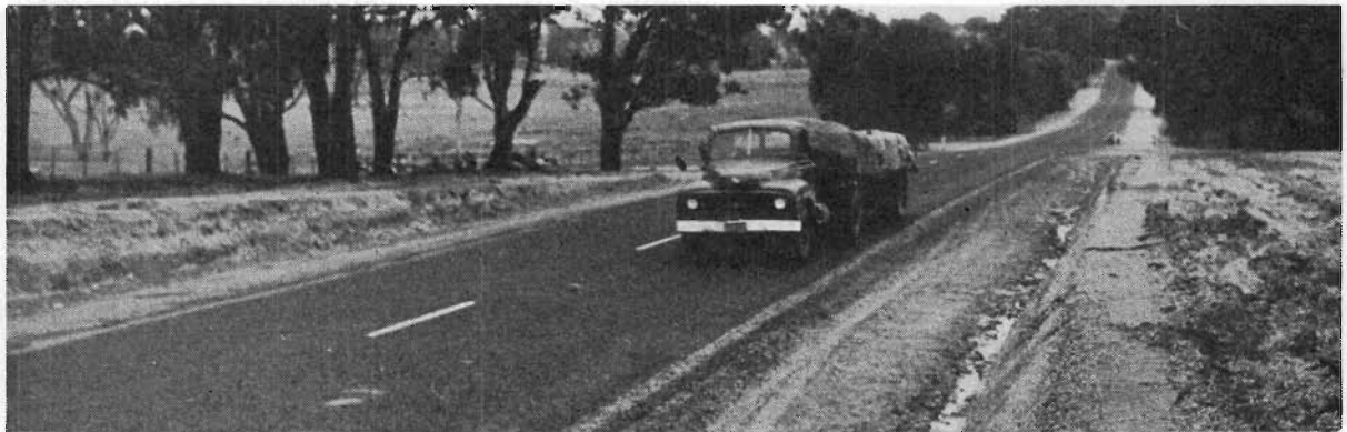
Plate 18.—Goulburn Valley Highway. Widened and reconstructed section at Mangalore West.
