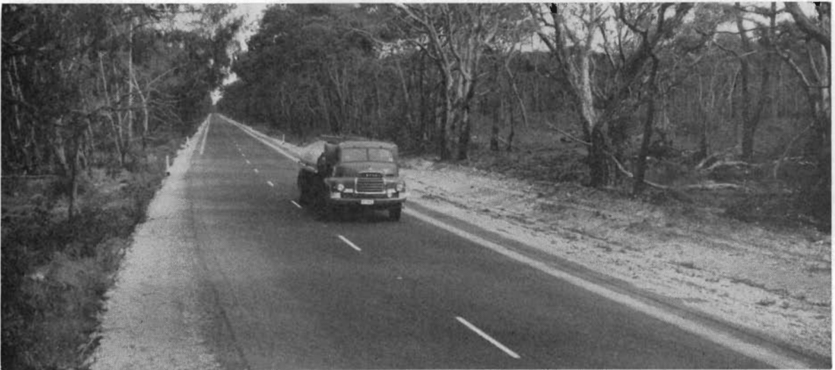
Plate 8.—Princes Highway West Section 5. Reconstructed and sealed section at 273 miles near Rennick. Portland Shire.
