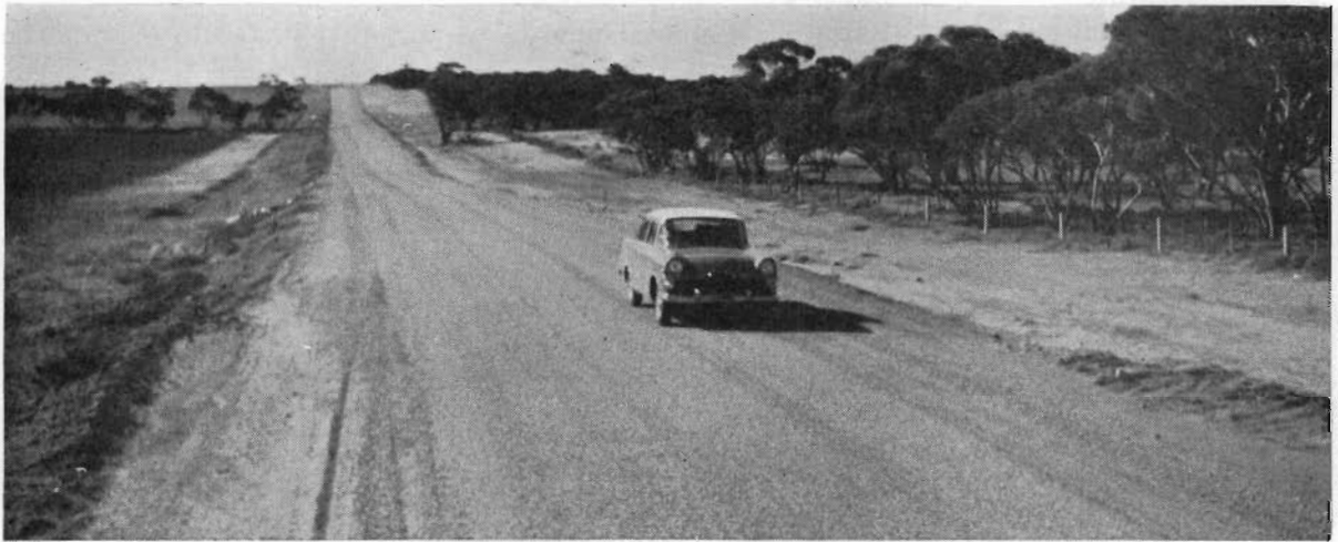
Plate 24.—Swan Hill Shire. Sea Lake—Robinvale Main Road Reconstructed and sealed section 5 miles north of Chinkapook.
