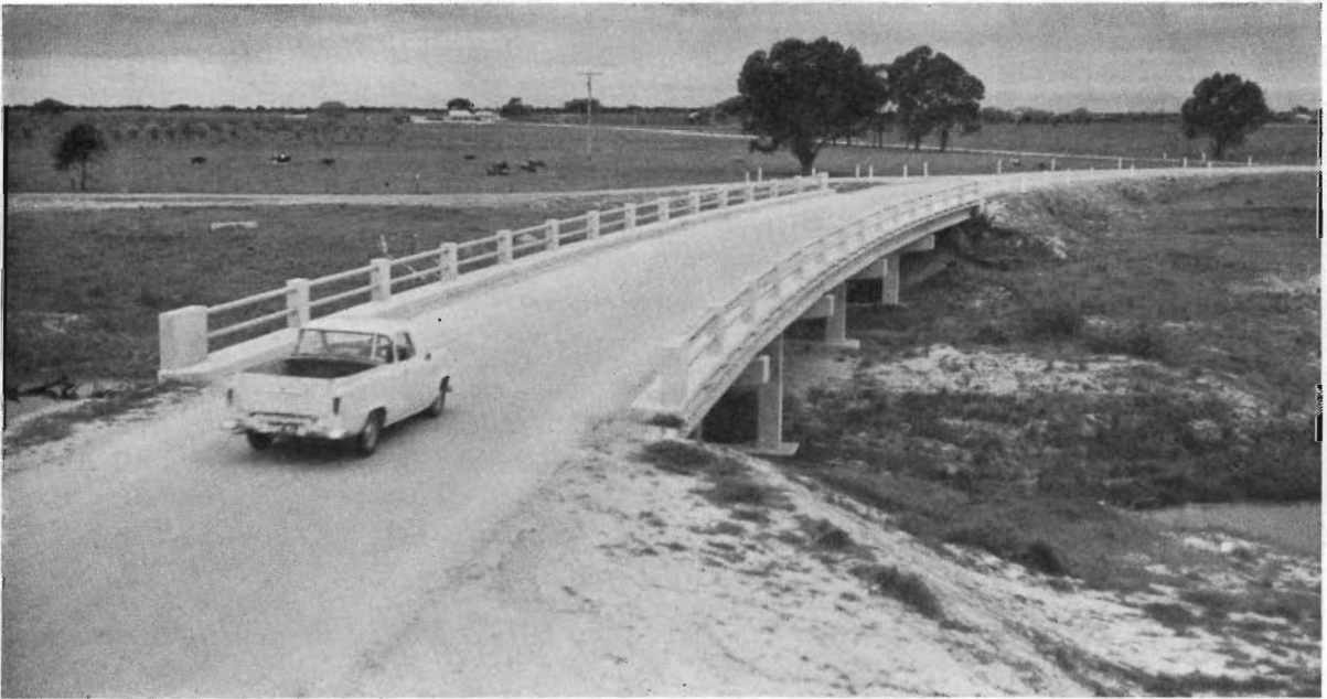
Plate 47.—Wimmera Shire. Riverside Road bridge over Wimmera River.
