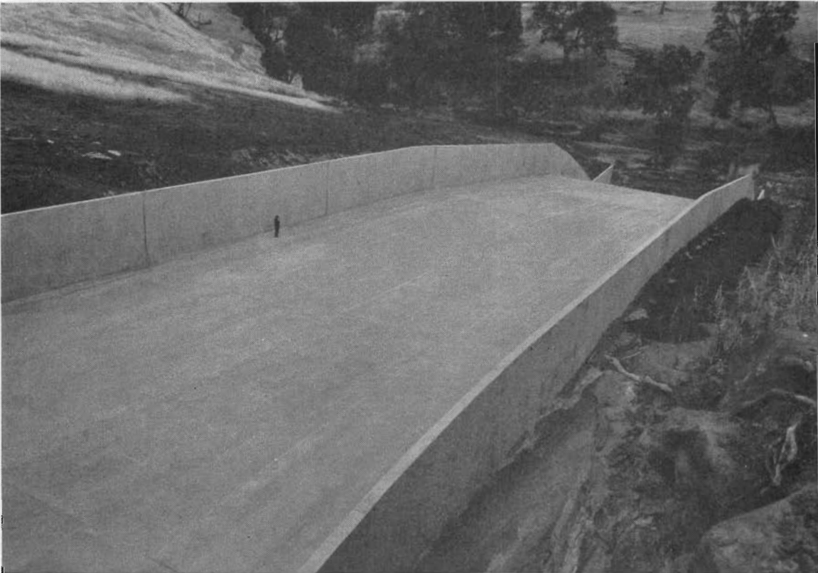
View down the concrete-lined main spillway at Lake Eppalock. Side wall is 16 ft. high. Full length of the concrete-lined section is 825 feet.
