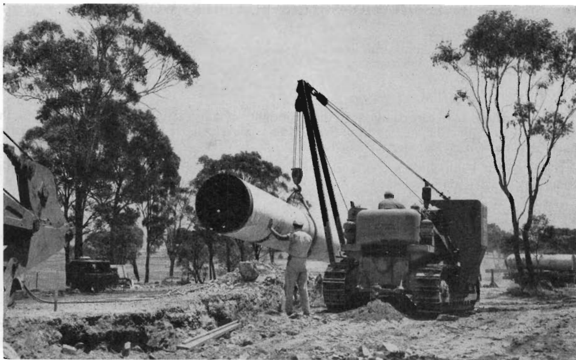
Laying a section of the pipeline between Lake Eppalock and Bendigo. The pipeline is of concrete lined mild steel, varying from 30 to 36 inches in diameter. It is nearly 18 miles long.
