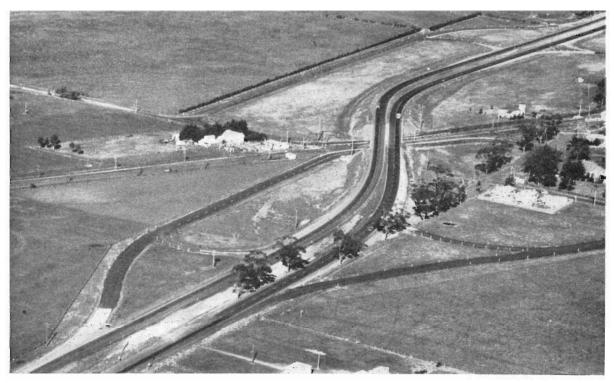
Plate 3.—Hume By-pass Road. Craigieburn Overpass. The completed Craigieburn section with dual pavements bridging the Sydney-Melbourne railway. Whittlesea and Bulla Shires.
