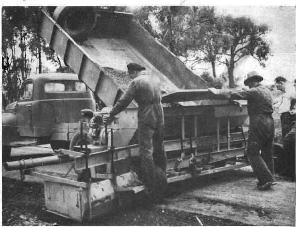
Plate 1.—Pavement widening of Hume Highway, Section 1, with a power pack hopper-conveyor. 10903/62.-5
