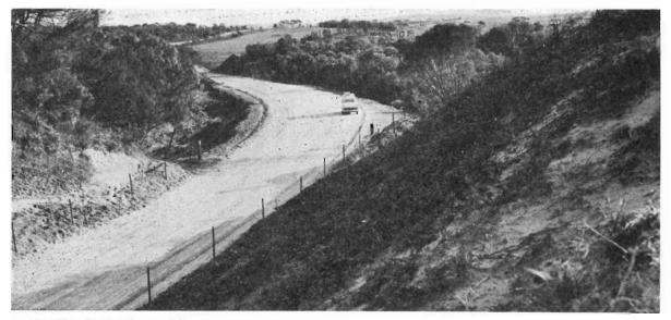
Plate 25.—South Gippsland Shire. Promontory Road. 1.1 miles of realignment through sand hills before sealing.
