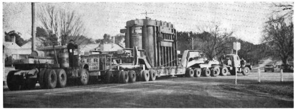
Plate 8.—71 ton State Electricity Commission transformer passing through Gisborne en route to Kerang.
