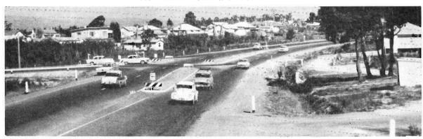
Plate 36.—Morwell Shire. Princes Highway East, Section 2. Channelization on deviation of highway at Hernes Oak constructed as result of operations of State Electricity Commission work in the area.
