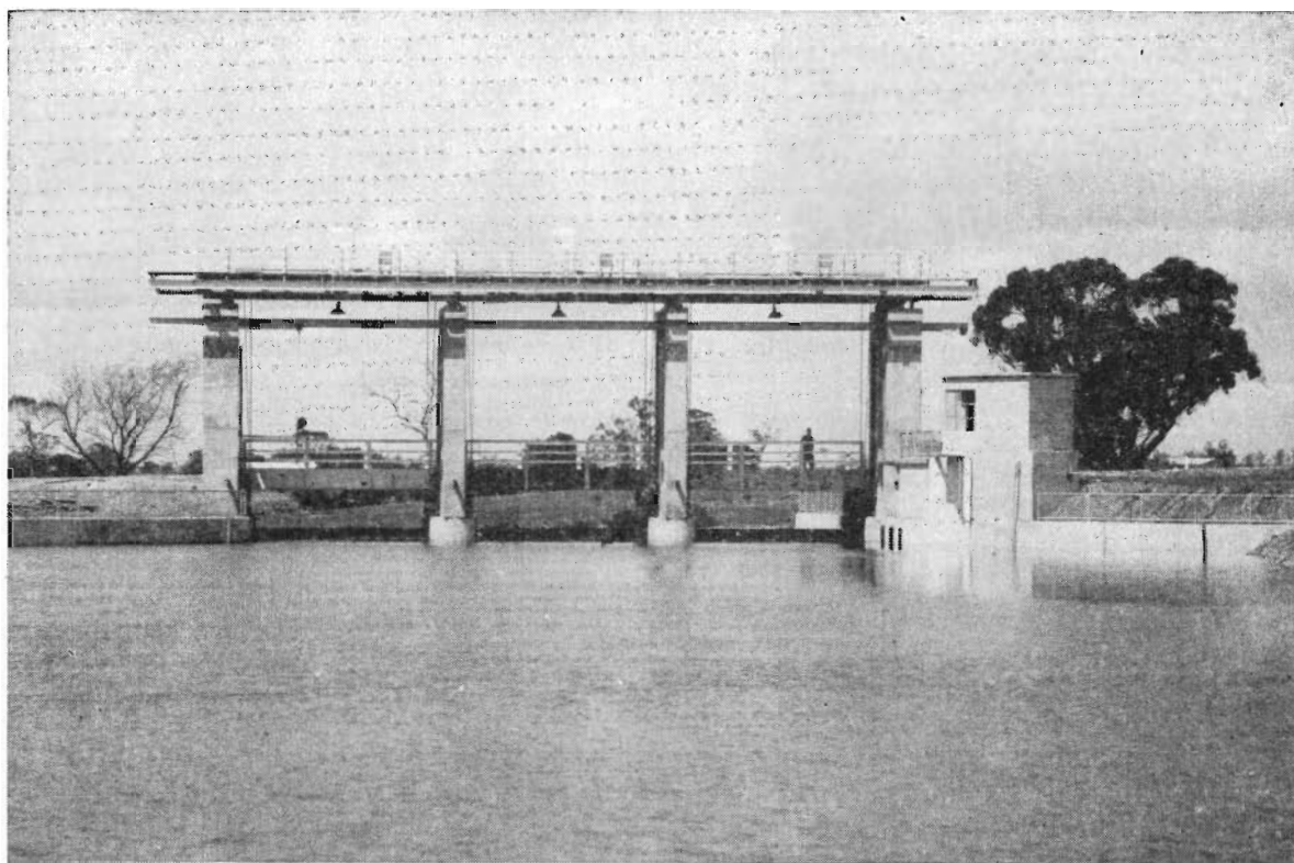
Cowwarr Weir, on the Thomson River, is used to divert water to the Central Gippsland Irrigation Area of the Macalister Irrigation District. It was first used for this purpose in 1960-61.
