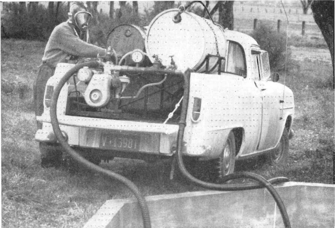
Injection of Aqualin, a new chemical for weed control, into a Commission channel. Use of this weedicide has greatly improved the capacity of main carriers such as the Yarrawonga Main Channel.
