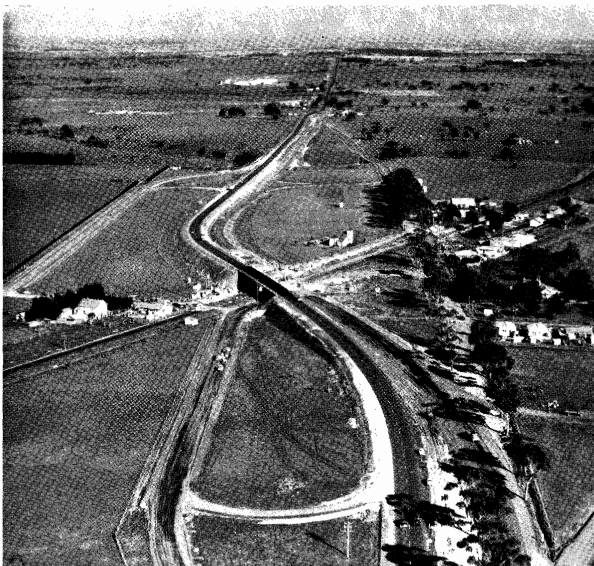
Plate 17.—Craigieburn Over-pass. Hume Highway. Aerial view of over-pass and road connections.
