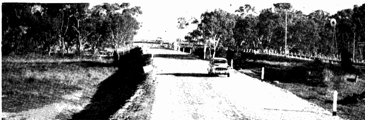
Plate 15.—Wimmera Highway. New concrete bridge over Wimmera River at Quantong.
