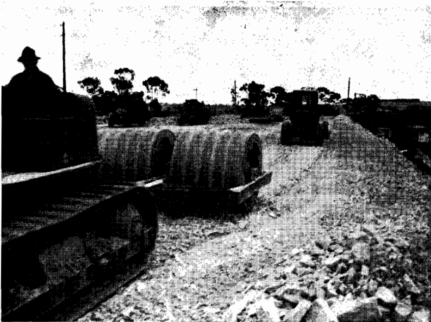
Plate 3.—Grooved roller working at Craigieburn.
