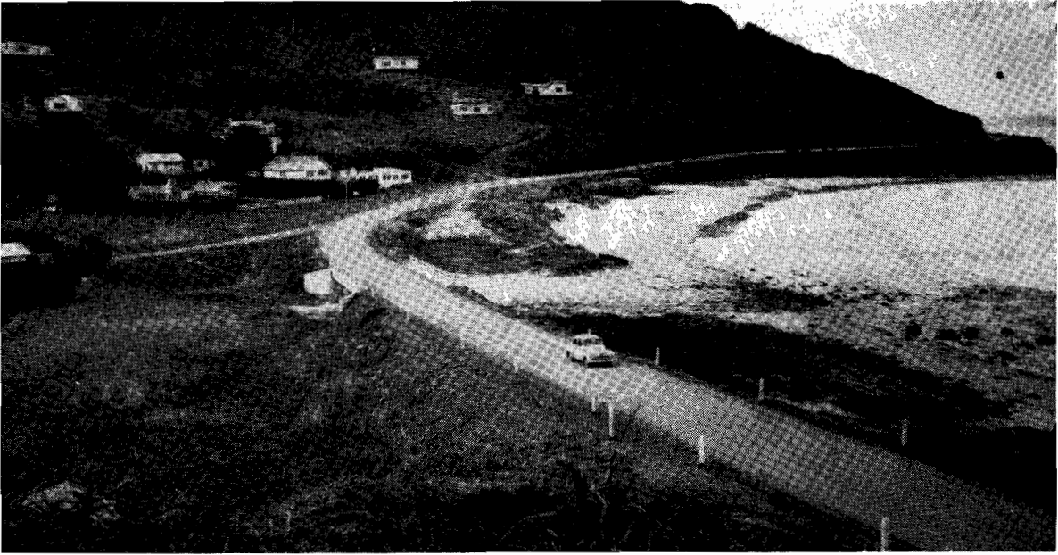
Plate 29.—Shire of Winchelsea. Ocean Road. Realignment including new bridge at Separation Creek.
