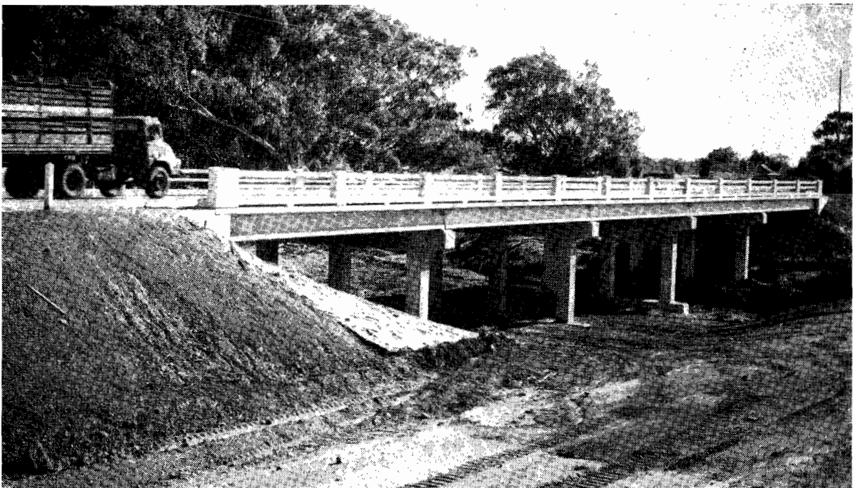
Plate 9.—Calder Highway. New bridge over Bullabul Creek.
