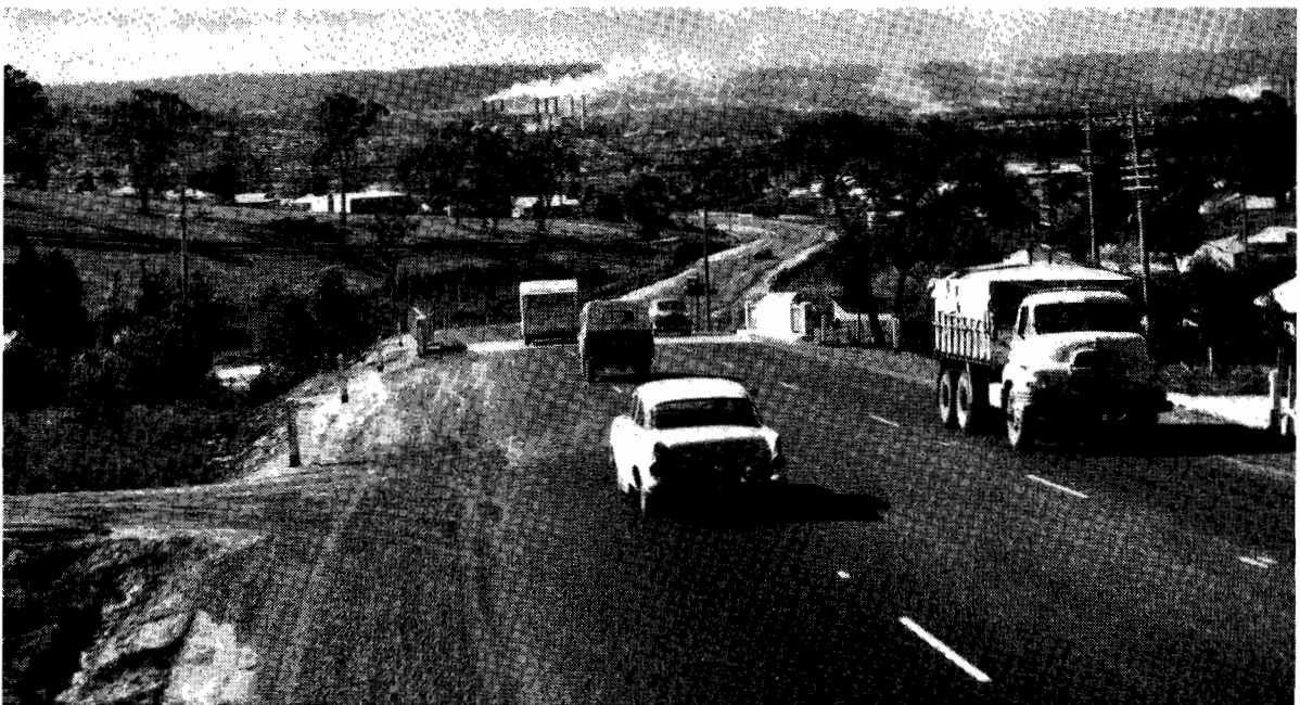
Plate 3.—Completed deviation and bridge at Hernes Oak at site depicted in Plate 2.
