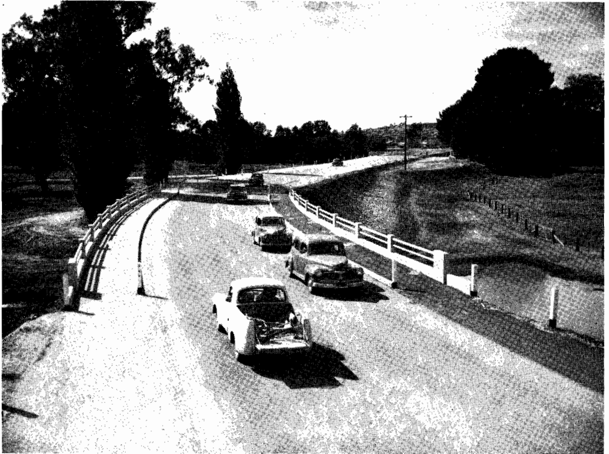
Plate 11.—Hume Highway. Widened bridge—Murray River flood plain between Wodonga and Albury.
