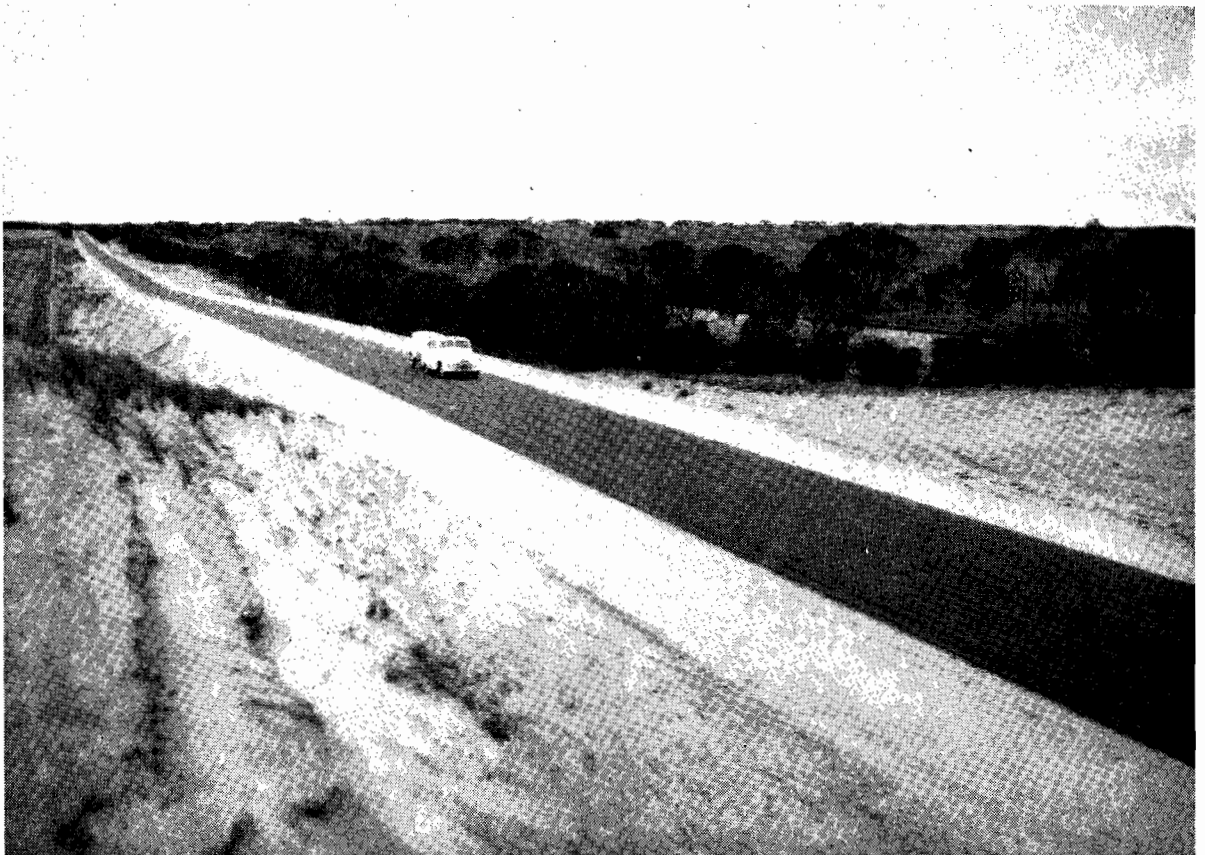
Plate 12.—Henty Highway—After reconstruction through sand hills south of Speed.
