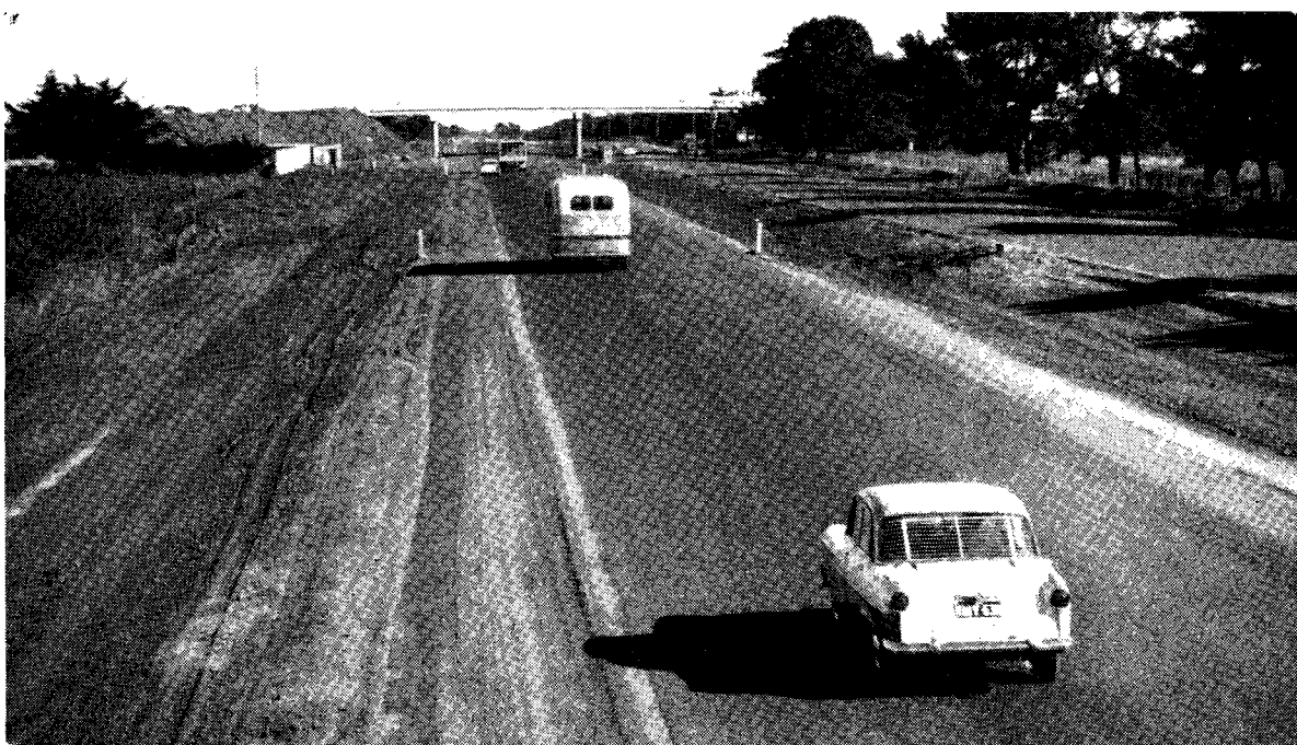
Plate 20.—Maltby By-pass. Duncan's Road Over-pass.
