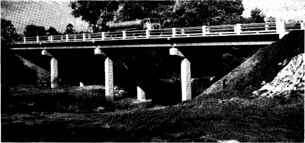
Plate 1.—Princes Highway East. New bridge over Bunyip River.
