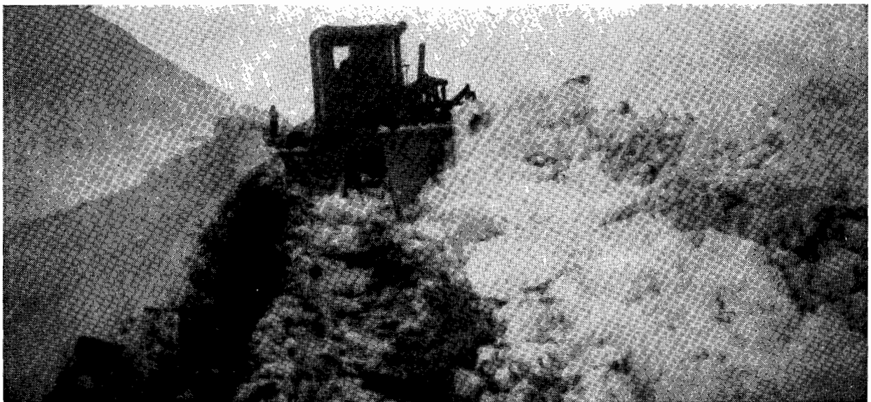
Plate 31.—Shire of Omeo. Alpine Road. Snow clearing.
