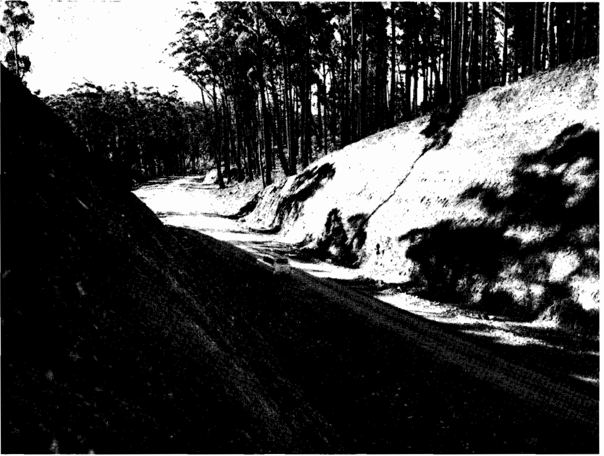
Plate 4.—Cutting—Depth 58 ft. at Donalds Knob—Club Terrace Deviation.
