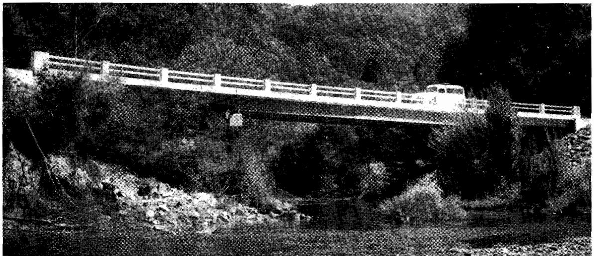
Plate 36.—Shire of Mansfield. Burns Bridge over Goulburn River on Mansfield-Woods Point Road.
