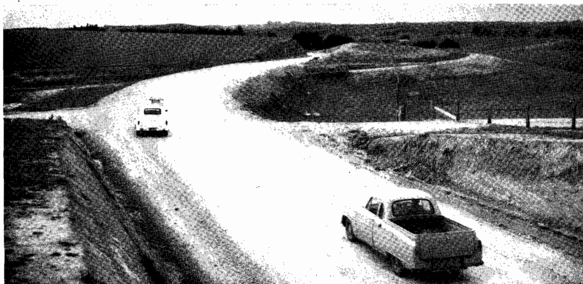
Plate 28.—South Gippsland Shire. Fish Creek—Yanakie Road. Reconstruction eliminating sharp bends south of Fish Creek.
