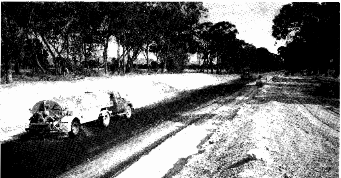
Plate 10.—Hume Highway. Reconstruction in progress south of Baddaginnie.
