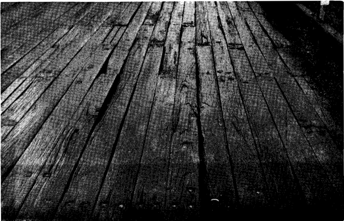
Plate 12.—Timber deck before treatment.
