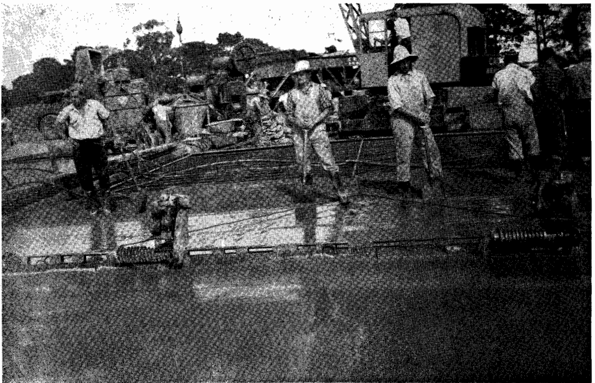
Plate 10.—Using vibrating screed moved longitudinally.
