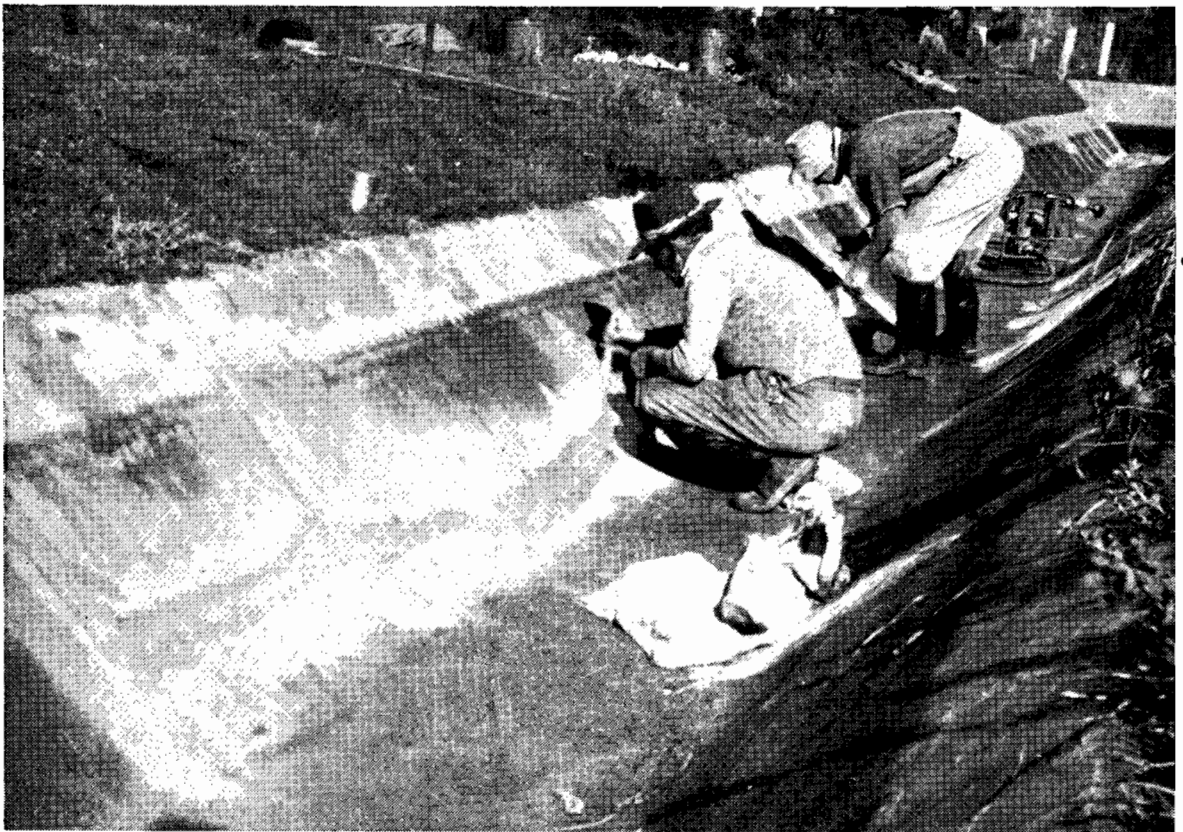
Workmen applying a plasticised material to a concrete-lined channel at Merbein. This is one of several methods of repairing cracks and joints in channels which the Commission's research engineers are investigating.
