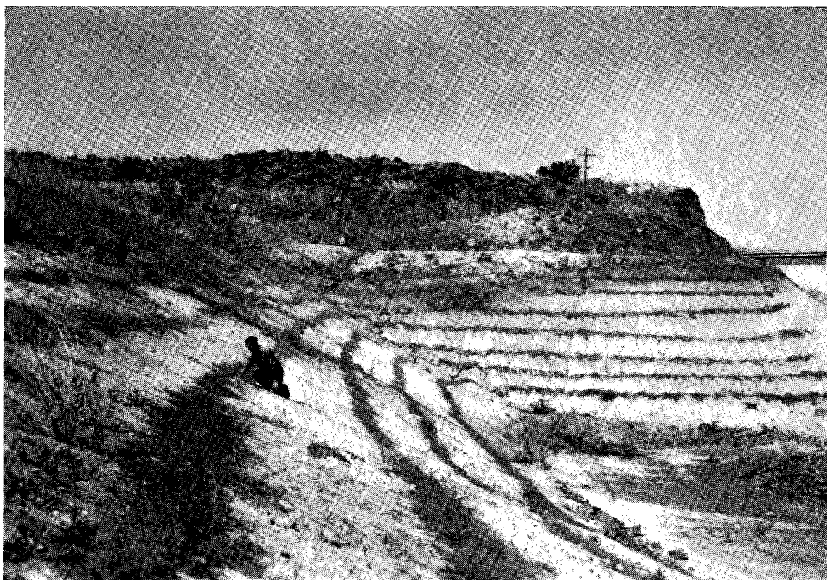
Face of the excavation for Tullaroop Reservoir spillway, seven months after treatment with the straw-strip method for establishing creeping saltbush.
