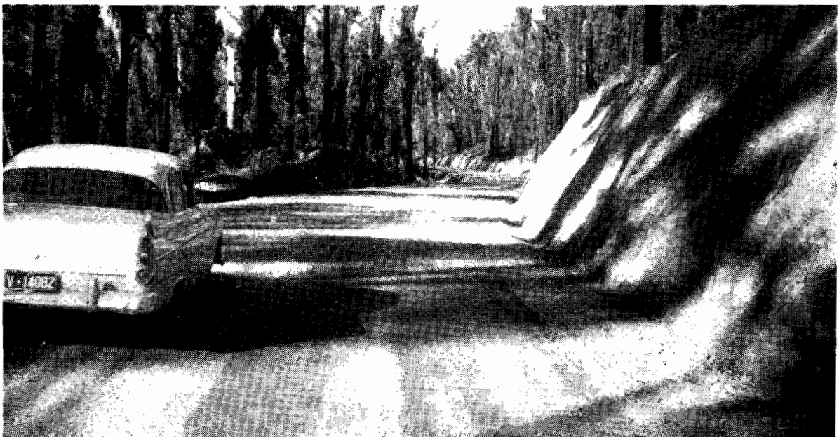
Plate 21.—Shire of Orbost. Club Terrace Loop. Section constructed by contractor on new alignment near Bemm River, Princes Highway East.
