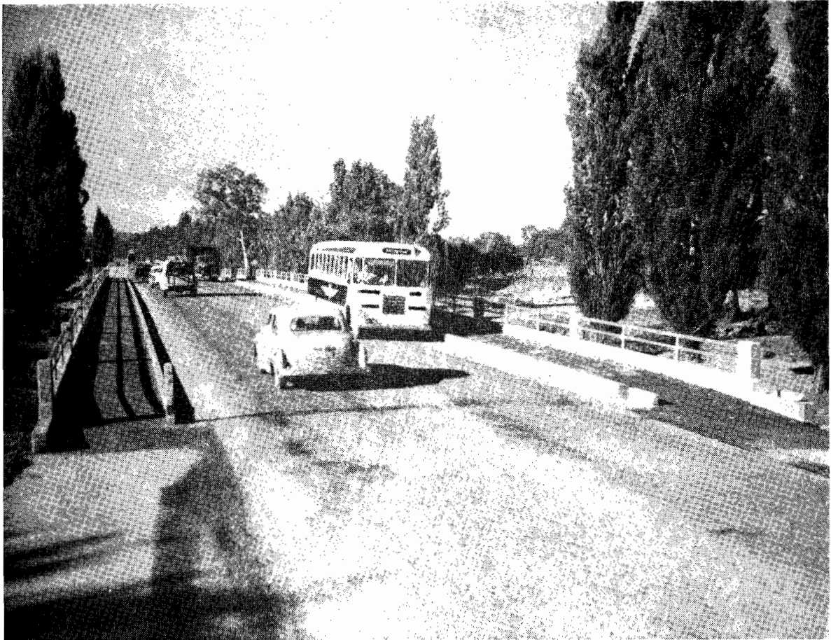
Plate 25.—Hume Highway, Section 3. No. 4 bridge over River Murray flats showing widening from 22 to 28 feet between kerbs, and the provision of two cycle tracks 6 feet wide.
