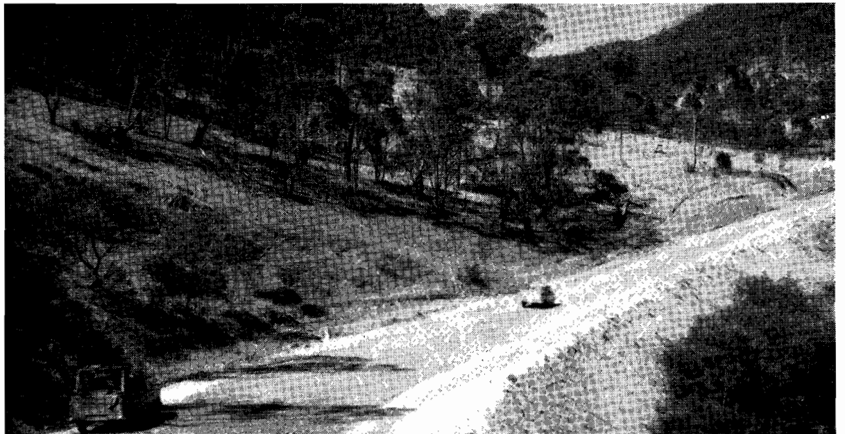
Plate 2.—Shire of Upper Murray. Tallangatta–Corryong Road, reconstructed and sealed section approximately 7 miles west of Cudgewa.
