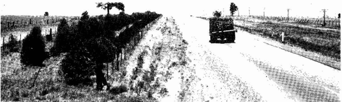
Plate 23.—Shire of Lowan. Western Highway, Section 5. Plantation of trees west of Nhill.
