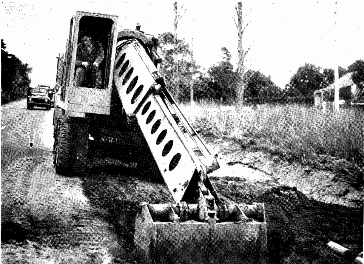
Plate 1.—“Gradall” combined excavator back-actor ripper, and grader.
