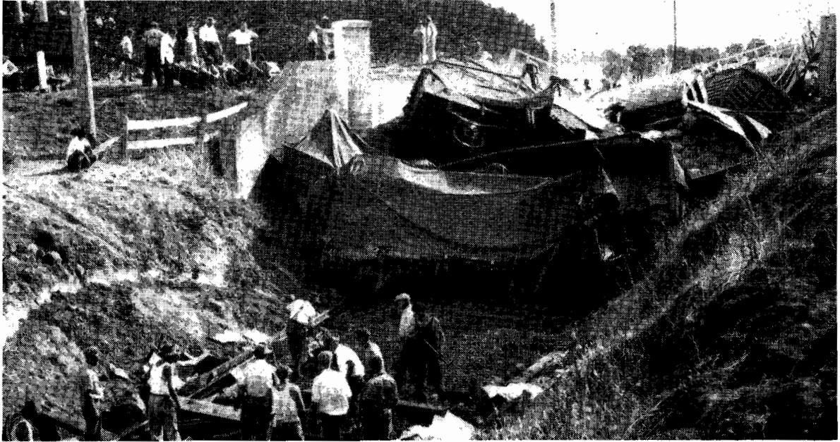
Plate 19.—Shire of Winchelsea. Princes Highway West, Section 2. Bridge demolished by train at Armytage.
