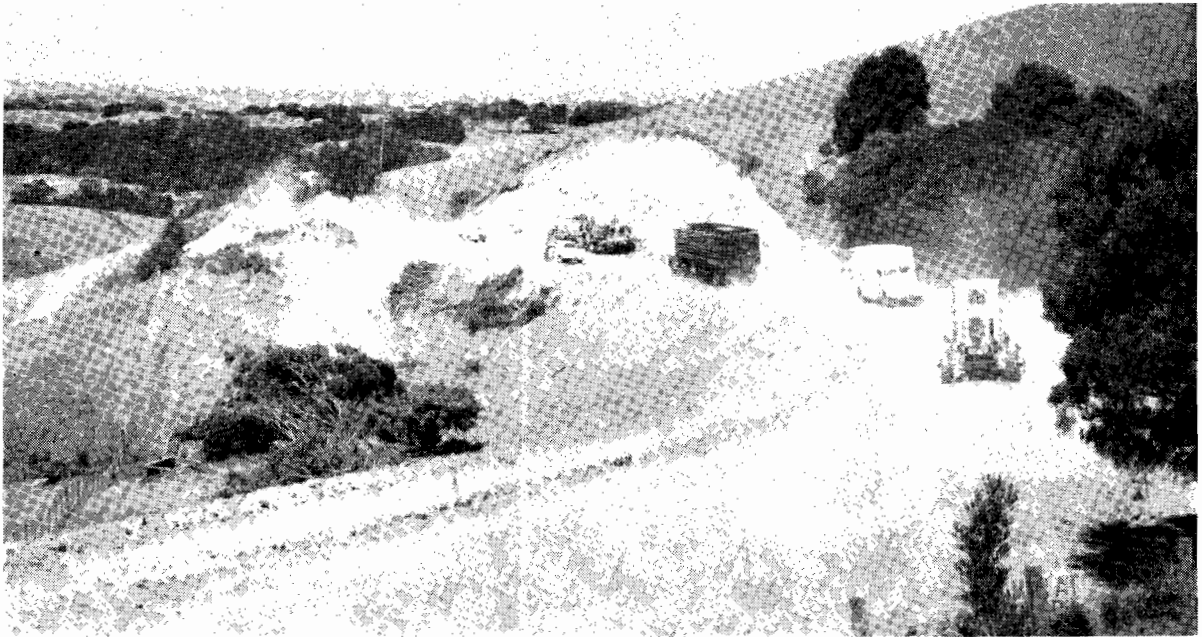
Plate 4.—Shire of Korumburra. Section of Korumburra-Warragul Road during reconstruction.
