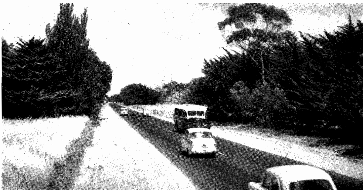
Plate 16.—Princes Highway West, 24 miles, before duplication of pavement (see below).
