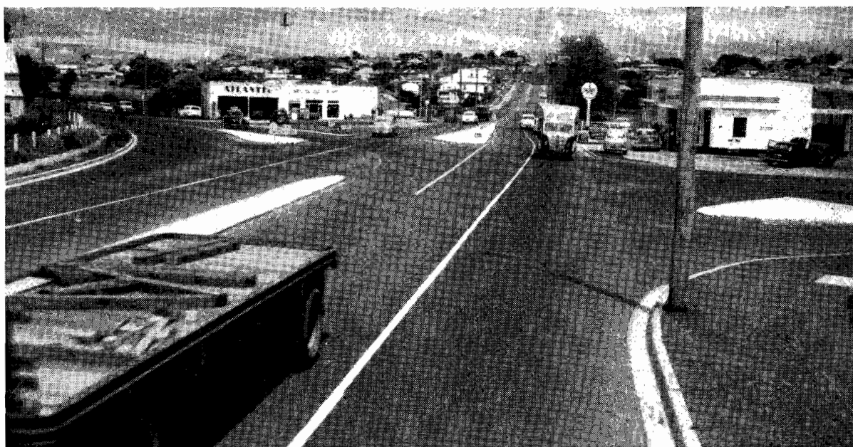
Plate 18.—Shire of South Barwon. Princes Highway West, Section I. Channelization at junction with Barwon Heads Road.
