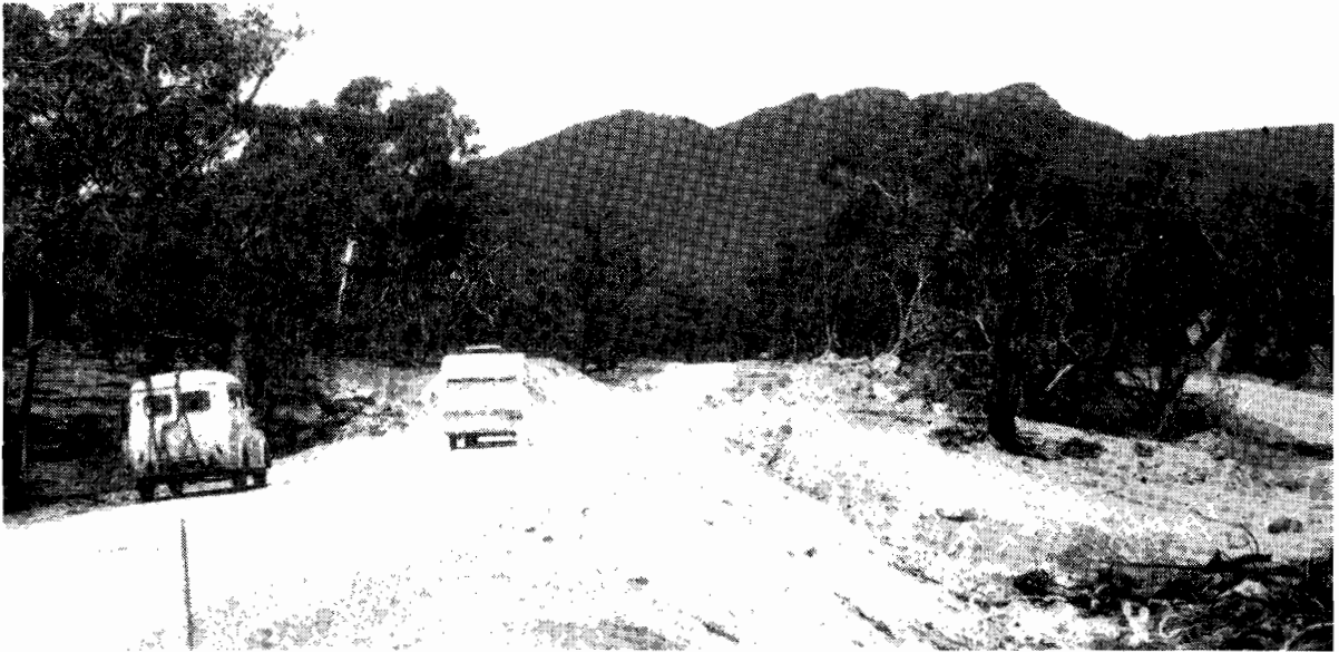
Plate 5.—Shire of Wimmera. Grampians Road, realigned section between Lah-Arum and Rosebrook; old alignment can be seen on right.
