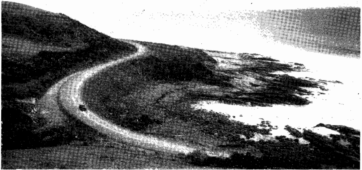
Plate 10.—Shire of Otway. Ocean Road. Realignment and reconstruction at Whalebone Creek, 108.3 miles.
