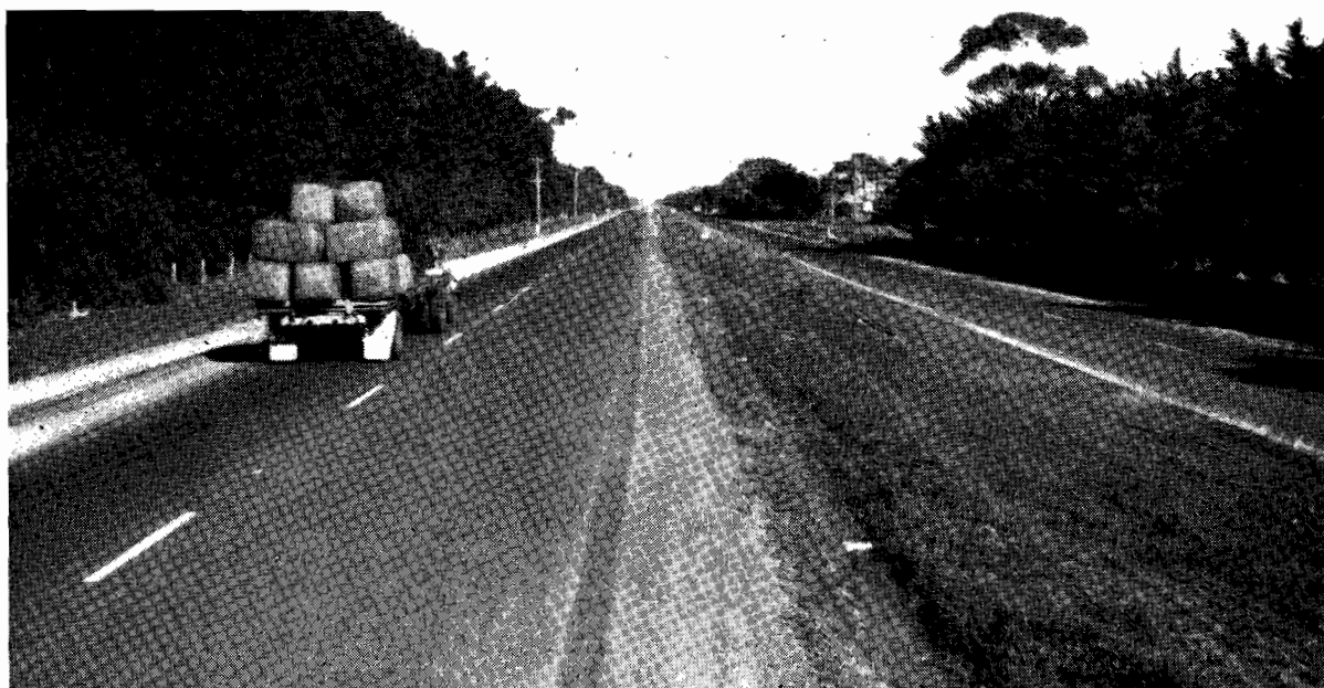
Plate 17.—Princes Highway West, 24 miles, after completion of the dual highway.
