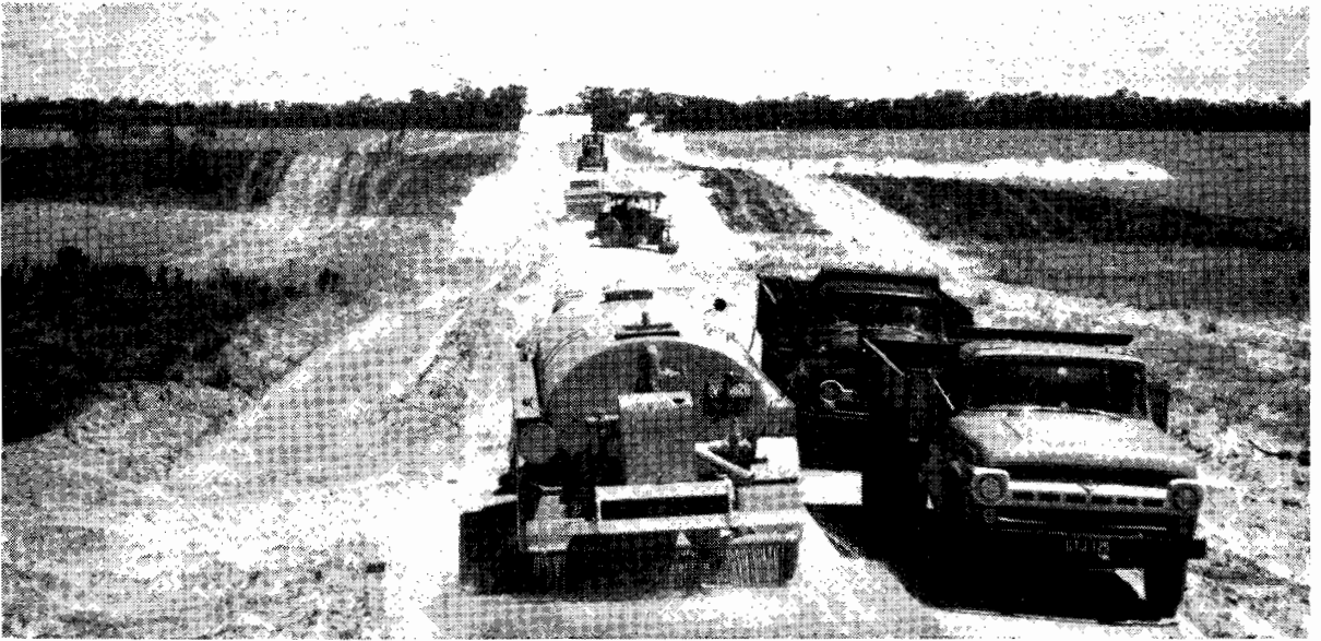
Plate 43.—Shire of Kaniva. Serviceton North Road. Big Desert Area. Spreading and consolidating sandstone pavement.
