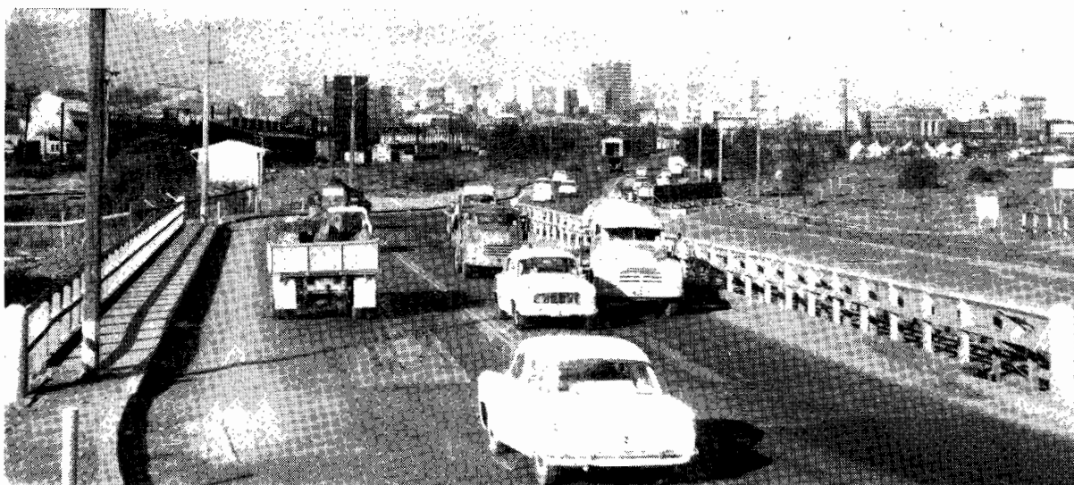
Plate 40.—City of Melbourne. New temporary bridge over Coal Canal on New Footscray Road.
