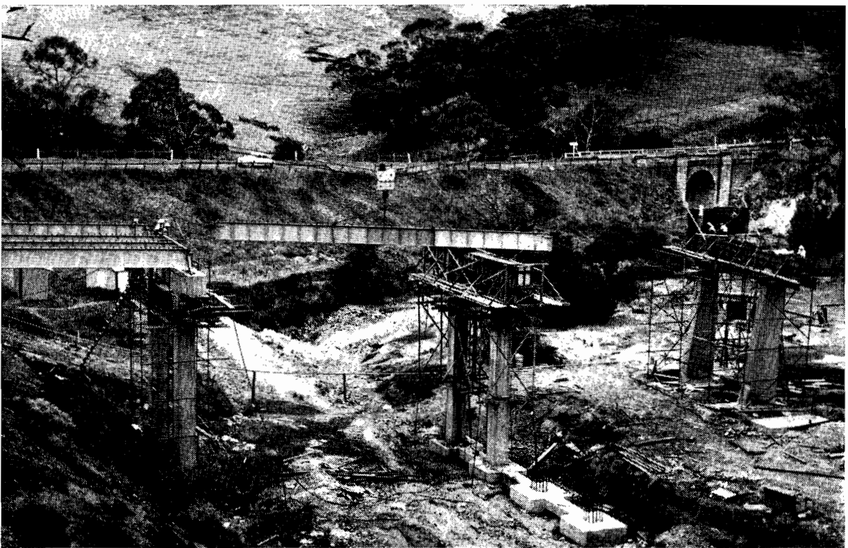
Plate 7.—4-ton capacity cable way used for placing 3.4-ton, 60-ft. plate girders.
