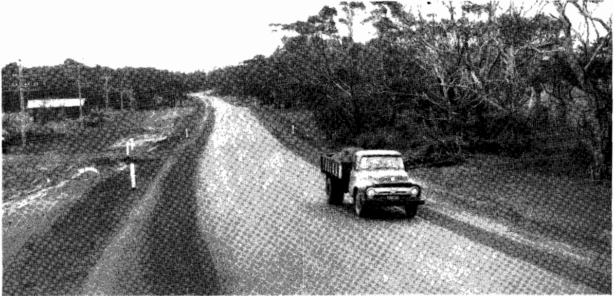
Plate 30.—Henty Highway, Section I. Reconstruction, widening and sealing completed on a section north of Portland.
