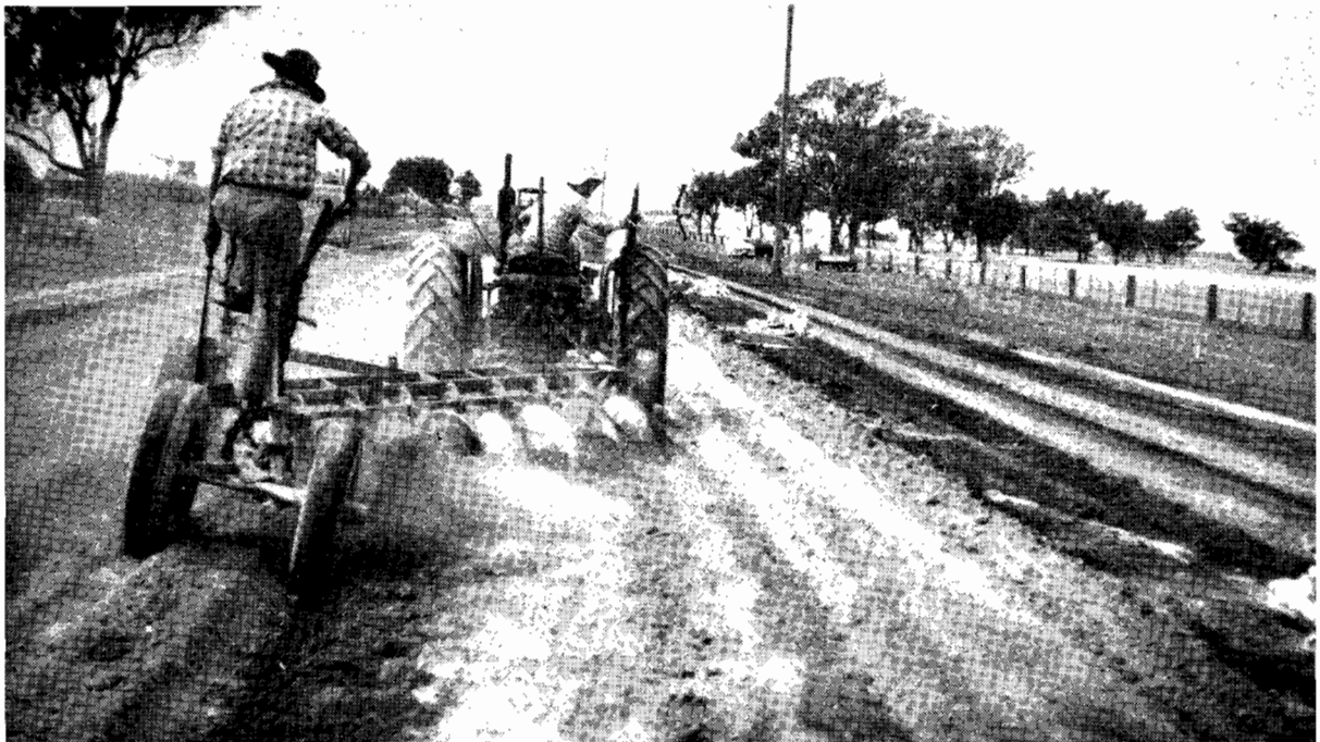
Plate 28.—Mixing "Limil" and soil by disc harrow.
