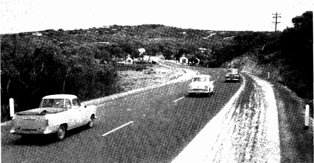
Plate 9.—Ocean Road, Shire of Barrabool. Realignment east of bridge over Anglesea River at 68.3 miles.
