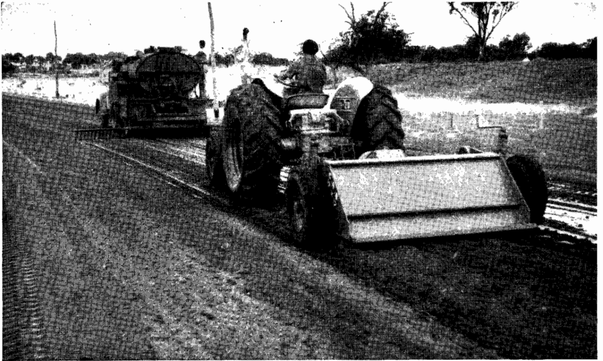
Plate 45.—Borong Highway, mileage 24. At Donald. Bituminous emulsion stabilizing, showing sprayer and tractor with attached rotary hoe.
