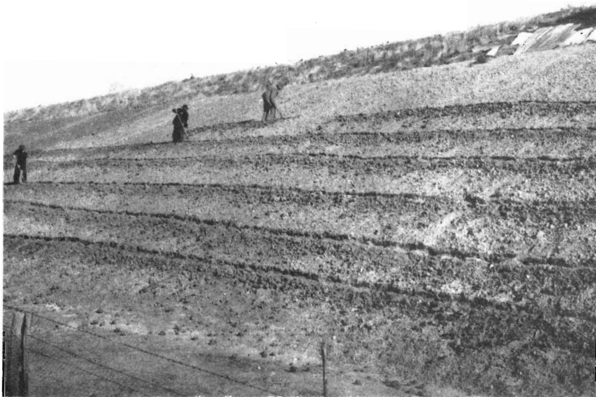
A major maintenance job extending over many years has been the stabilization of the 4½-miles embankment of the Waranga Reservoir. This photograph shows the trimming of earthworks completed and trenching in progress for planting out Kikuyu grass.
