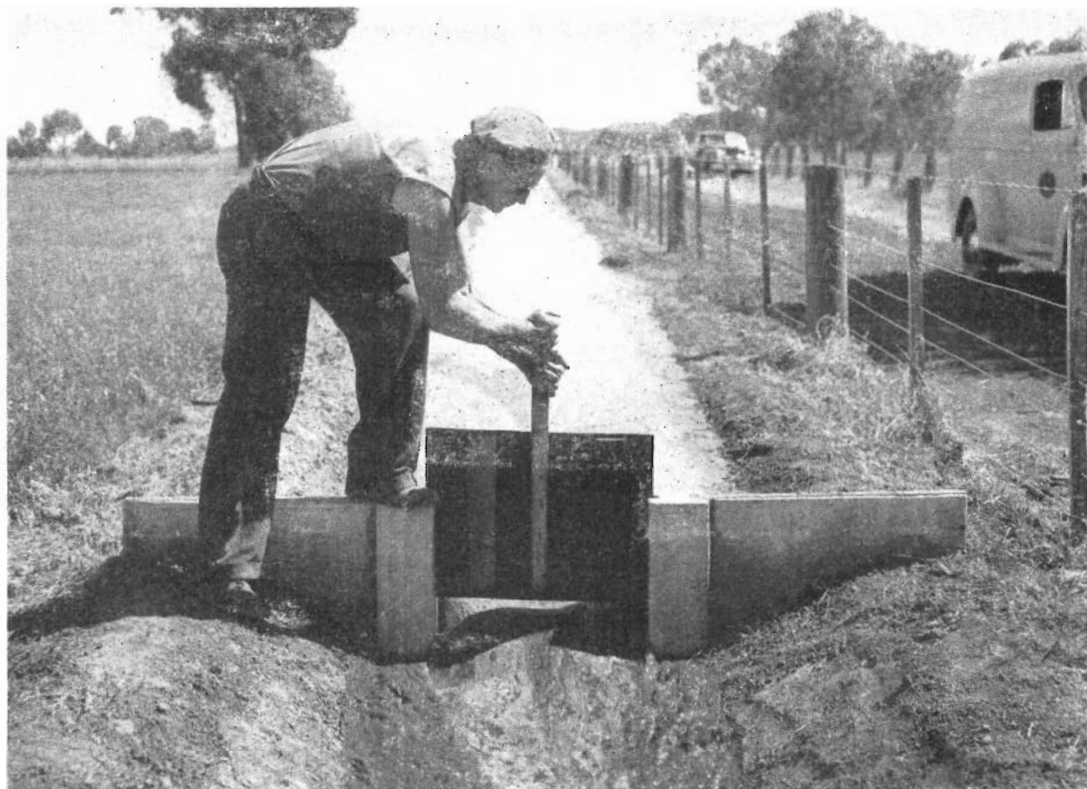
The improvement of small irrigation structures is one of many aspects of efficient water use being studied by the Commission's research officers. The use of concrete stops of this and similar types available commercially has increased efficiency on many irrigation farms.
