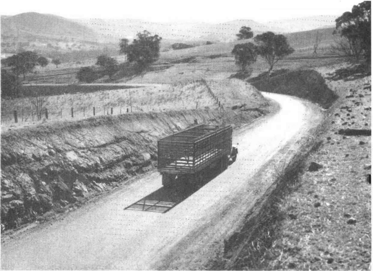
Plate 11.—Omeo Shire.—Ramrod Flat Road. Recently sealed section. Connor's Hill deviation.
