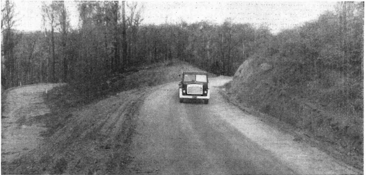
Plate 20.—Princes Highway East. Realignment and reconstruction. West of Club Terrace.
