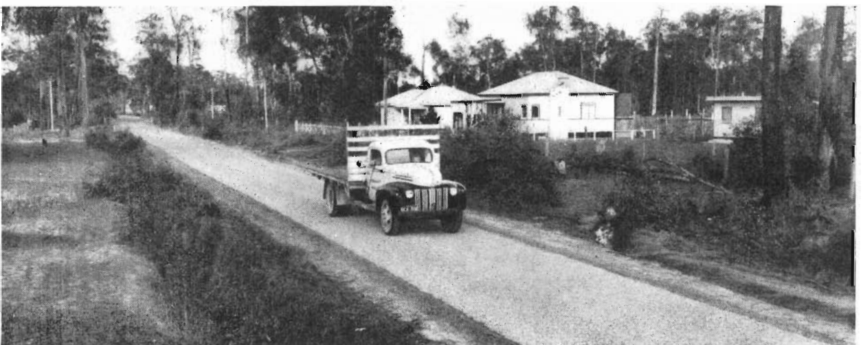
Plate 19.—Orbost Shire. Tamboon Road. Reconstruction and seal near Cann River Township.
