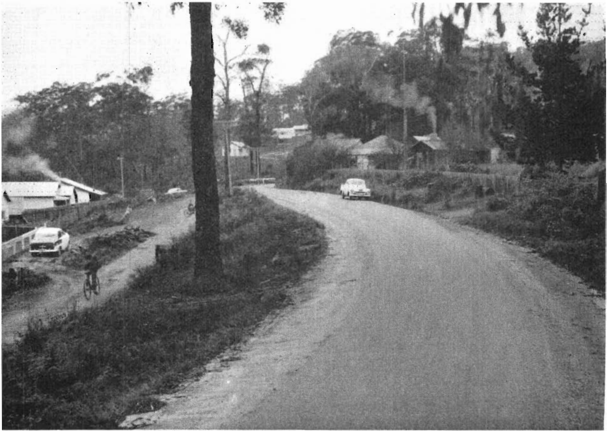
Plate 13.—Orbst Shire.—Combienbar Road. Bituminous sealed section in Club Terrace Township.
