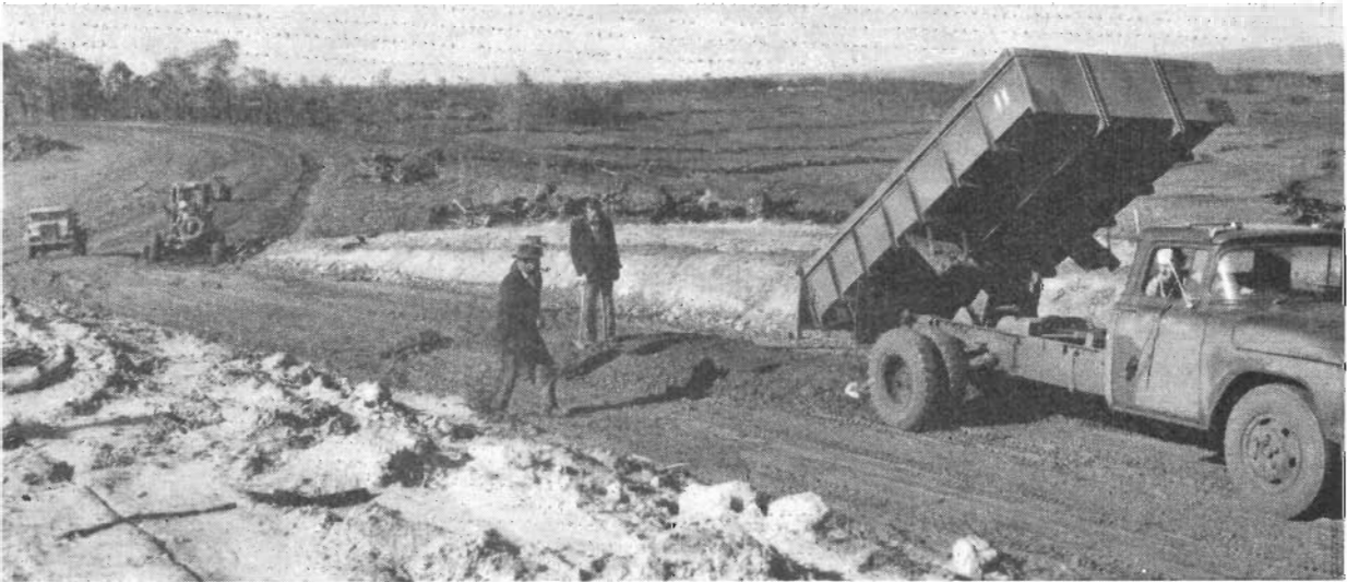
Plate 32.—Otway Shire. Heytesbury Settlement Area. New road under construction.
