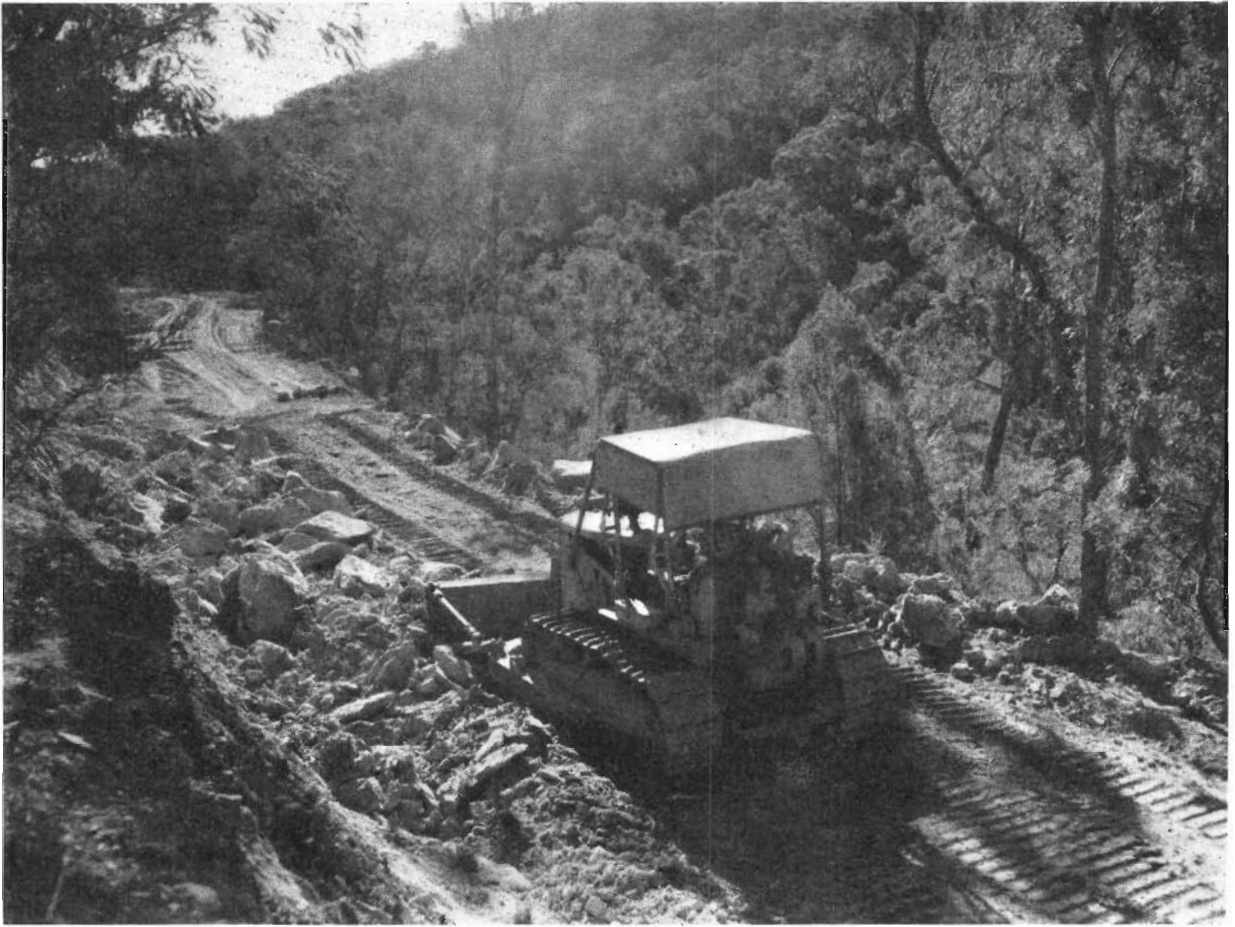
Plate 15.—Mt. Victory Road. Reconstruction in progress west of Wartook Road.
