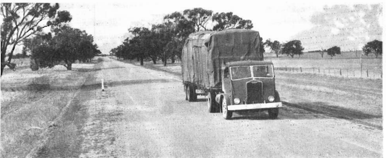
Plate 25.—Borong Highway. Cement stabilized section with Bitumen seal. West of Donald.
