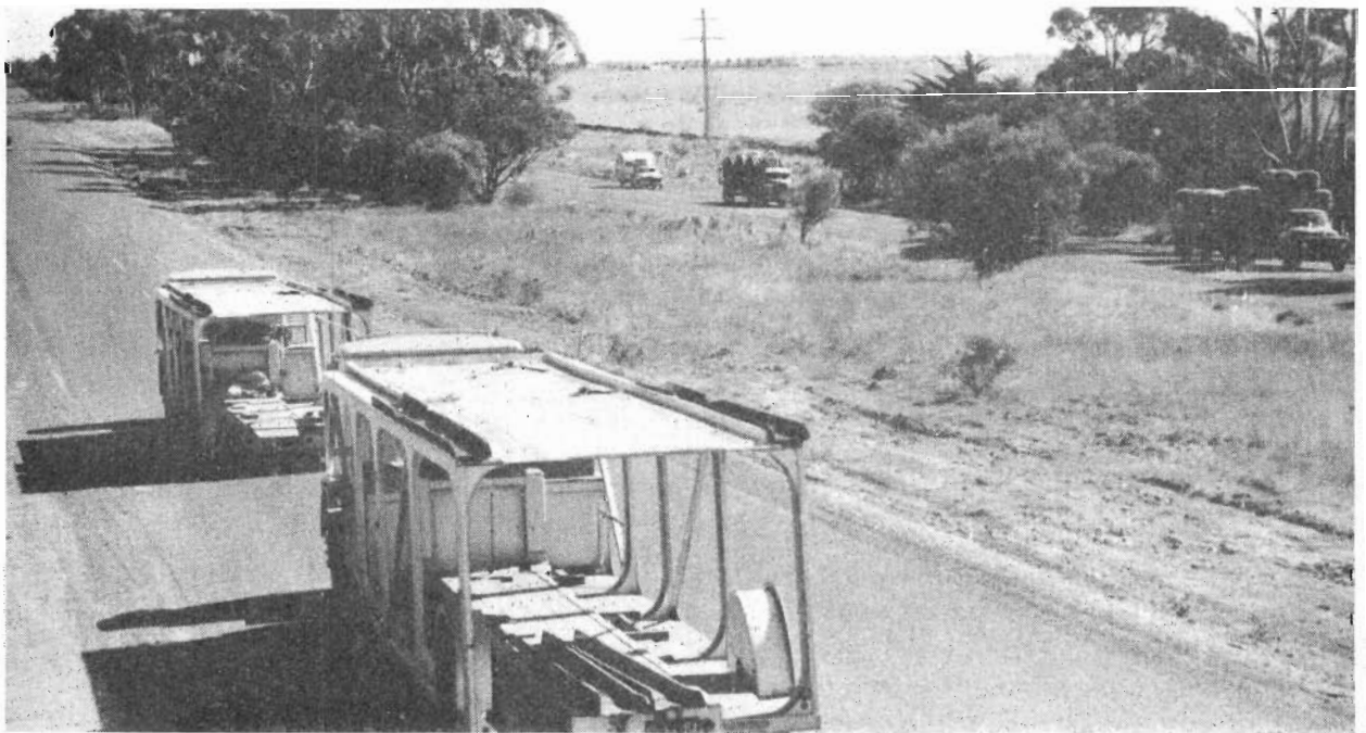
Plate 4.—Princes Highway West. Duplication south of Kororoit Creek.
