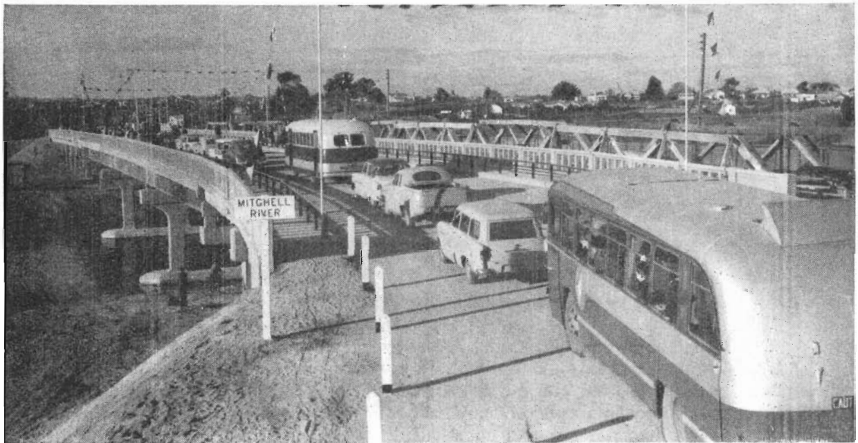
Plate 27.—Princes Highway East. Bridge over Mitchell River at Bairnsdale. Available to general traffic after official opening on 13th August, 1958.
