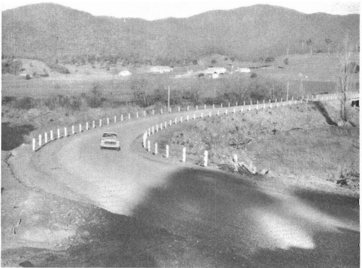
Plate 12.—Mansfield Shire.—Mansfield-Wood's Point Road. Reconstructed section at Howqua River.
