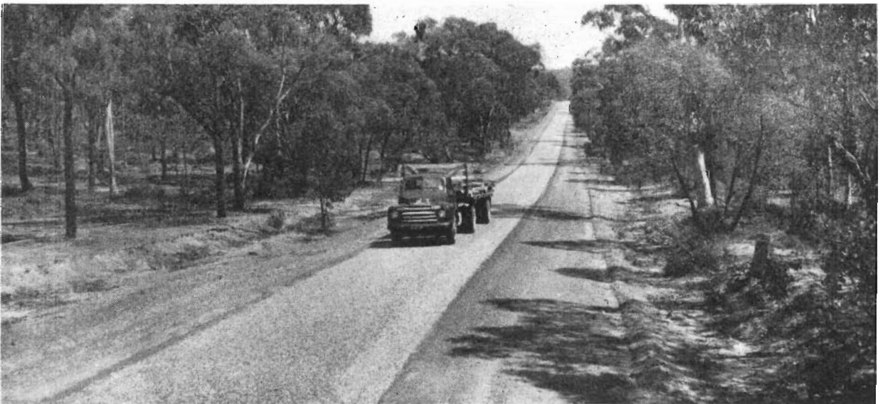
Plate 18.—Korong Shire.—Inglewood—Rheola Road. Reconstruction and sealing.
