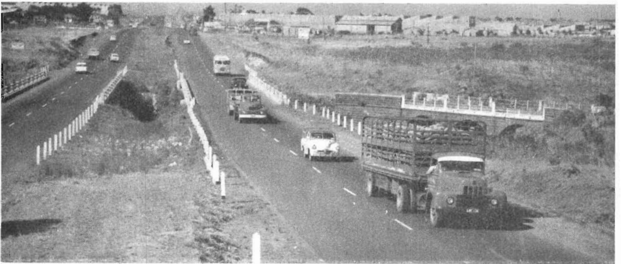
Plate 3.—Princes Highway West. Dual Bridges over Kororoit Creek. (Old Bridge at right).
