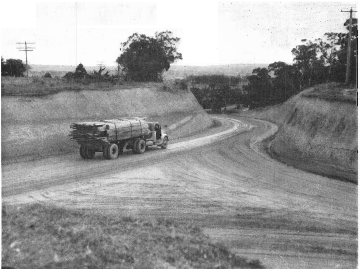
Plate 14.—Narracan Shire.—Walhalla Road. Deviation showing deep cutting 2 miles north of Moe.
