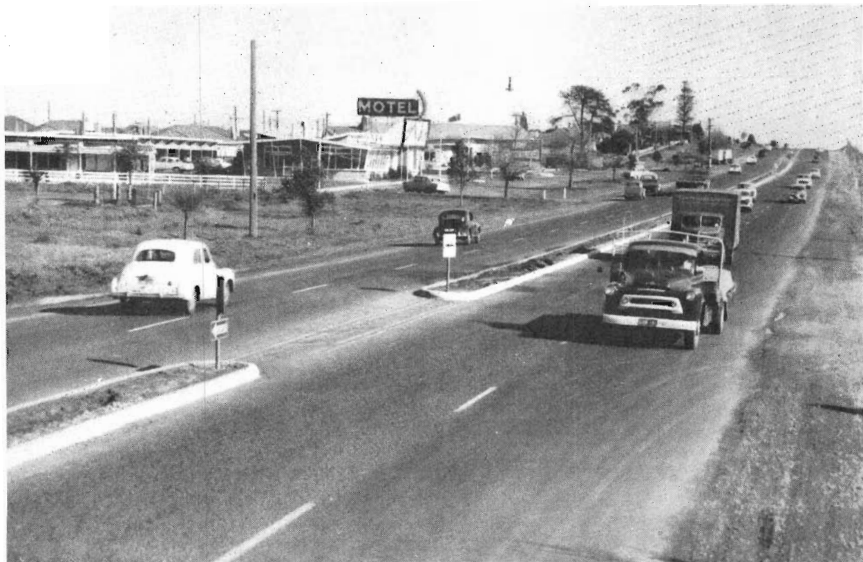
Plate 1.—Princes Highway East at Oakleigh. Duplicated Pavement with Median.
