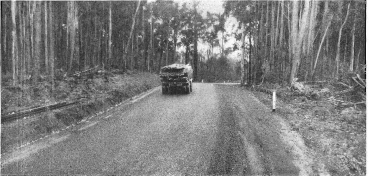
Plate 17.—Walhalla Road. Reconstructed, realigned and sealed section near Watson.
