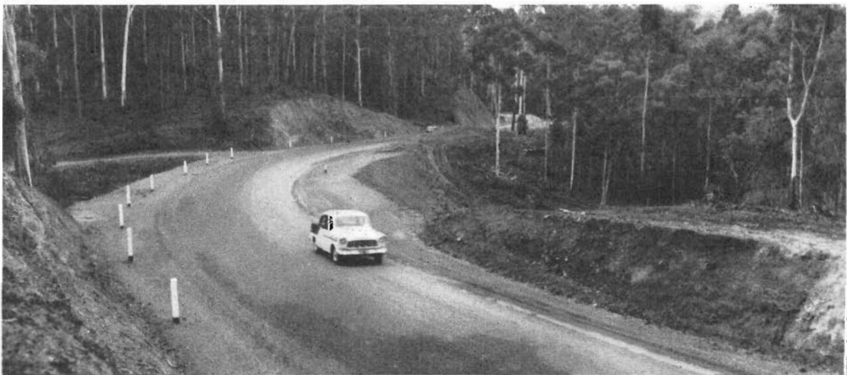
Plate 10.—Glenlyon Shire—Ballarat Road. Realigned and reconstructed section west of Daylesford.
