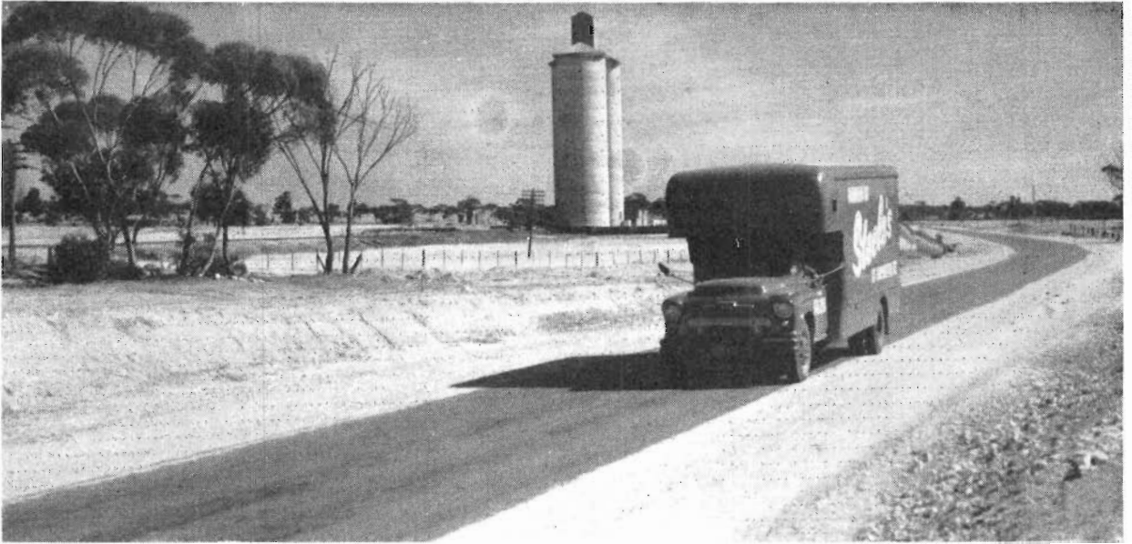
Plate 23.—Henty Highway. Reconstructed and sealed section near Gama.
