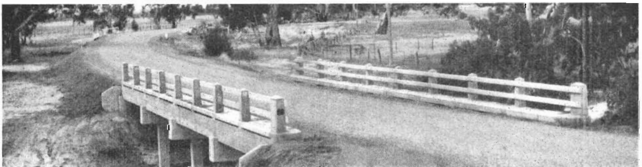
Plate 28.—Shire of Stawell.—Navarre Road. New bridge at Vinelea over Seven Mile Creek.
