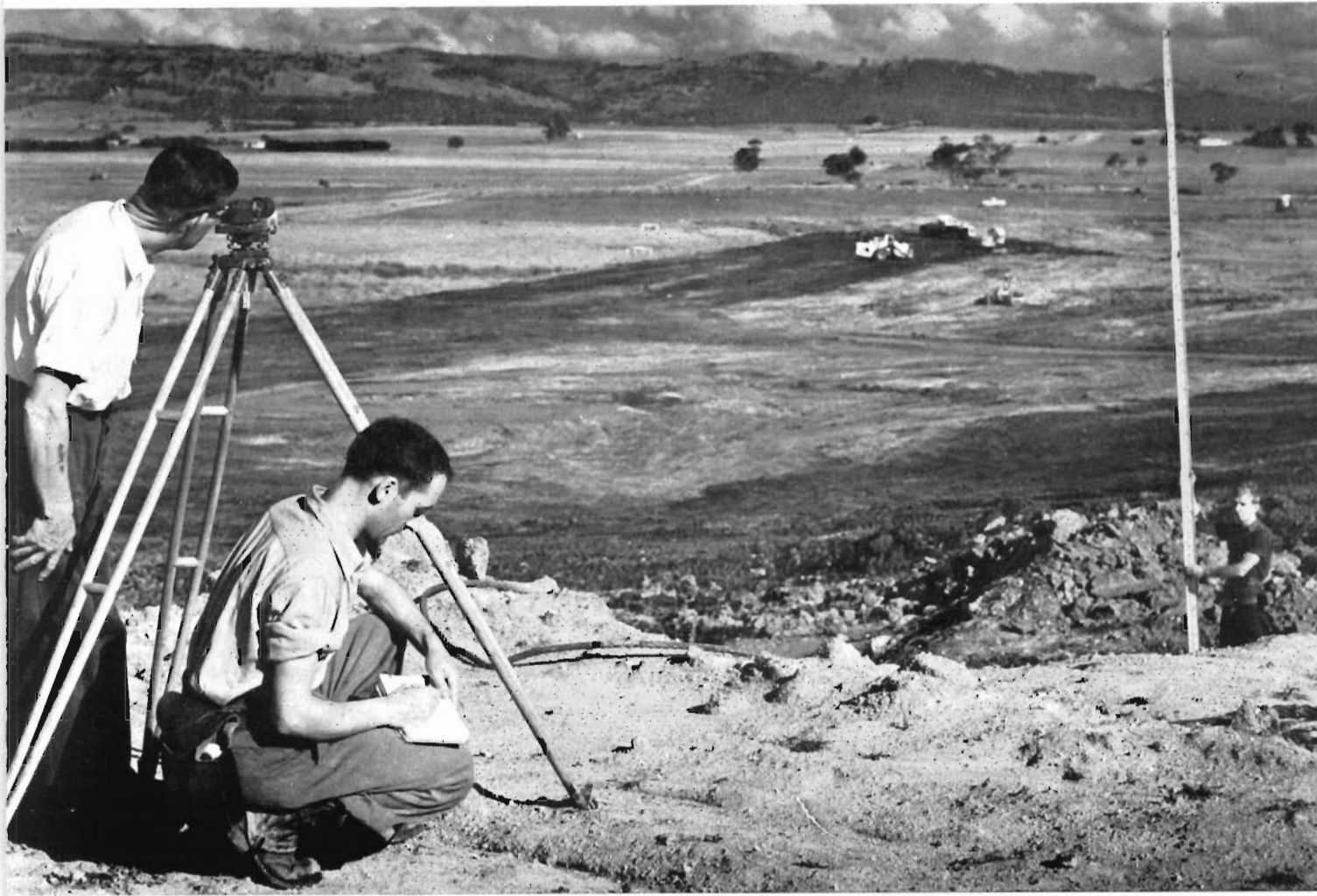
Site for new Hazelwood Power Station (1,200,000 kW capacity). Preliminary earthworks in progress.
