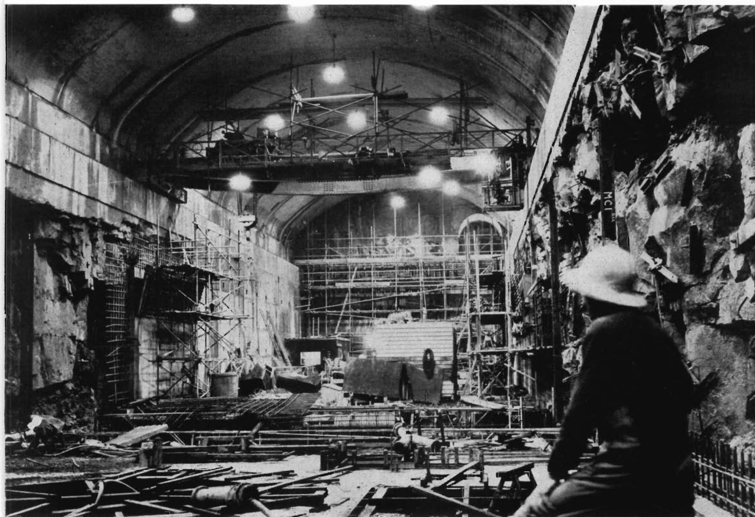
McKAY CREEK POWER STATION (KIEWA)—Planned capacity 96,000 kW. Excavation of underground chamber complete and placing of concrete lining and turbo-generators proceeding.
