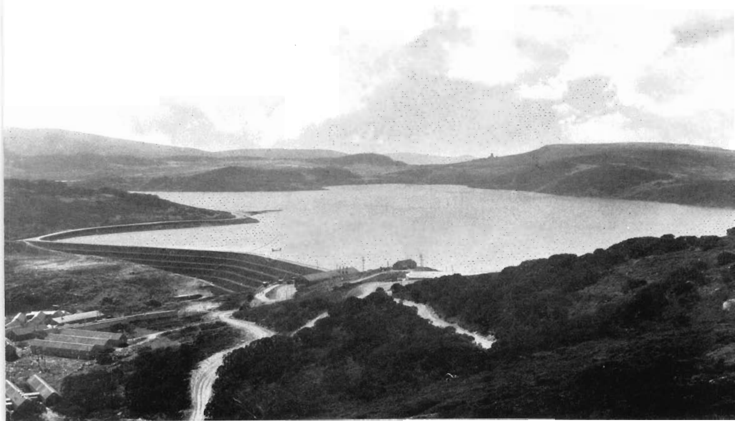
ROCKY VALLEY DAM (capacity 23,600 acre ft). This dam on the Bogong High Plains 5,338 ft above sea level is the highest altitude dam in Australia. It is the main storage for the Kiewa Scheme.
