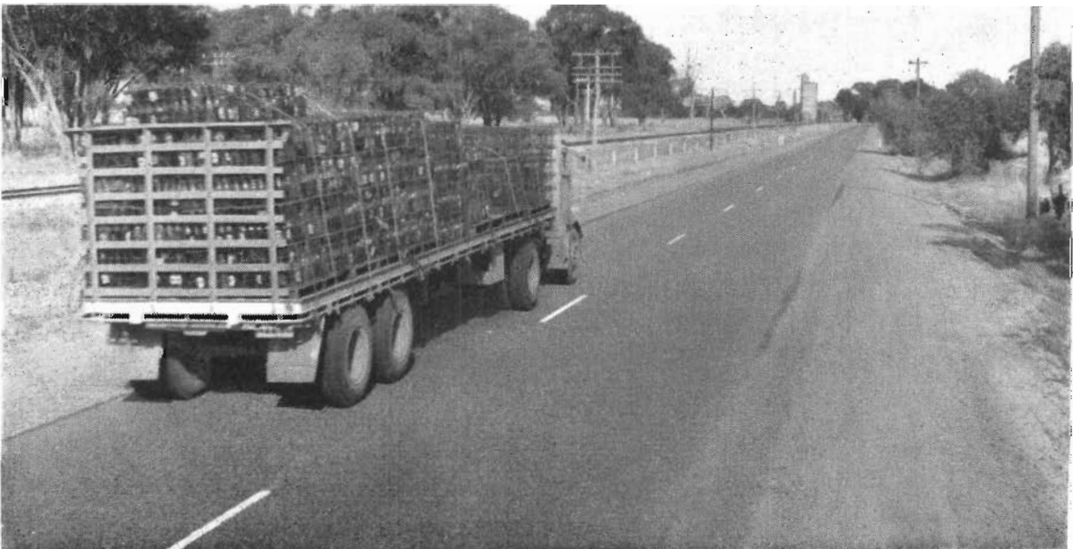
Plate No. 5 :—Goulburn Valley Highway—Reconstructed section north of Tallygaroopna.
