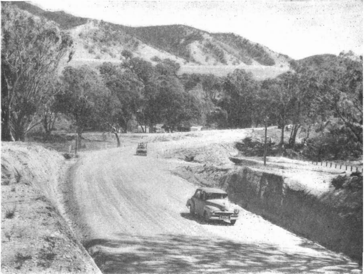
Plate No. 1 :—Omeo Shire—Ramrod Flat Main Road realignment and reconstruction near Doctor's Flat.
