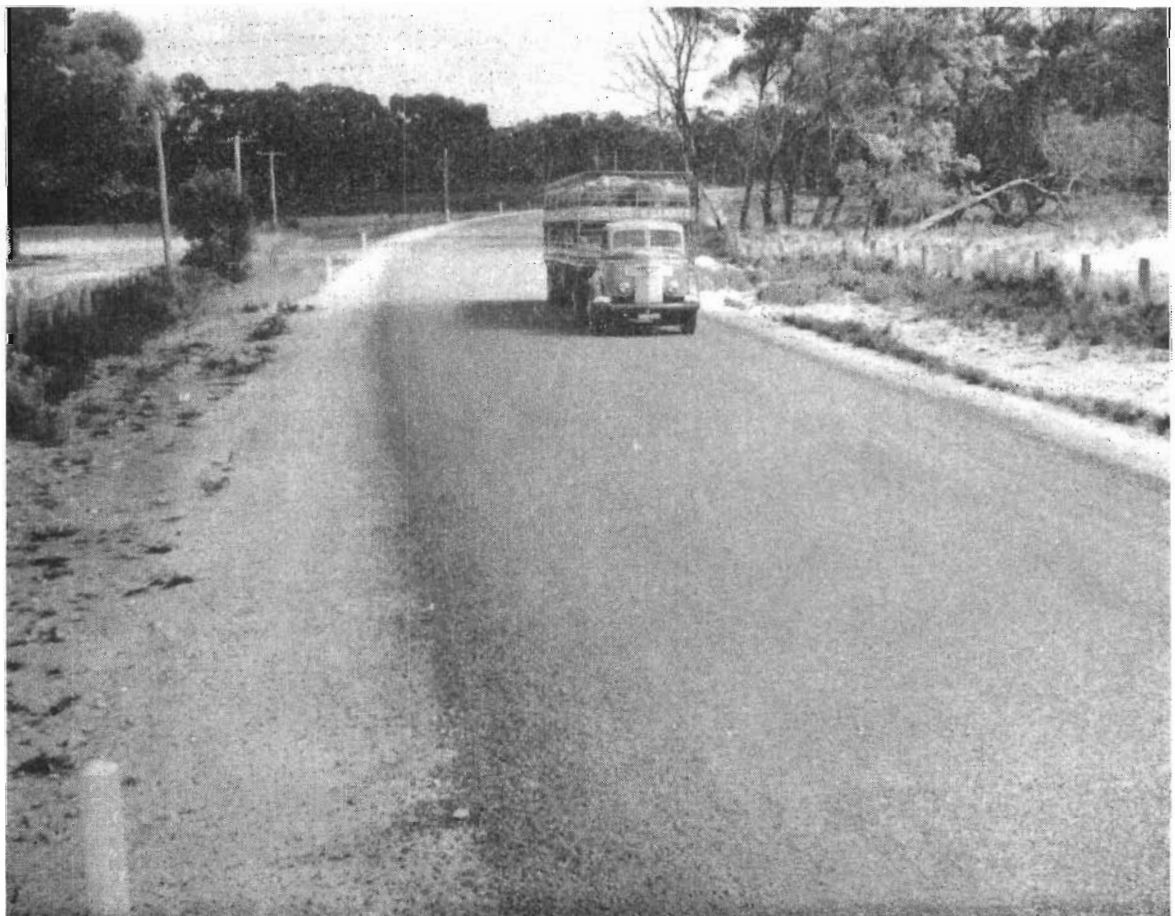
Plate No. 7 :—Princes Highway West showing reconstructed and sealed section west of Dartmoor.
