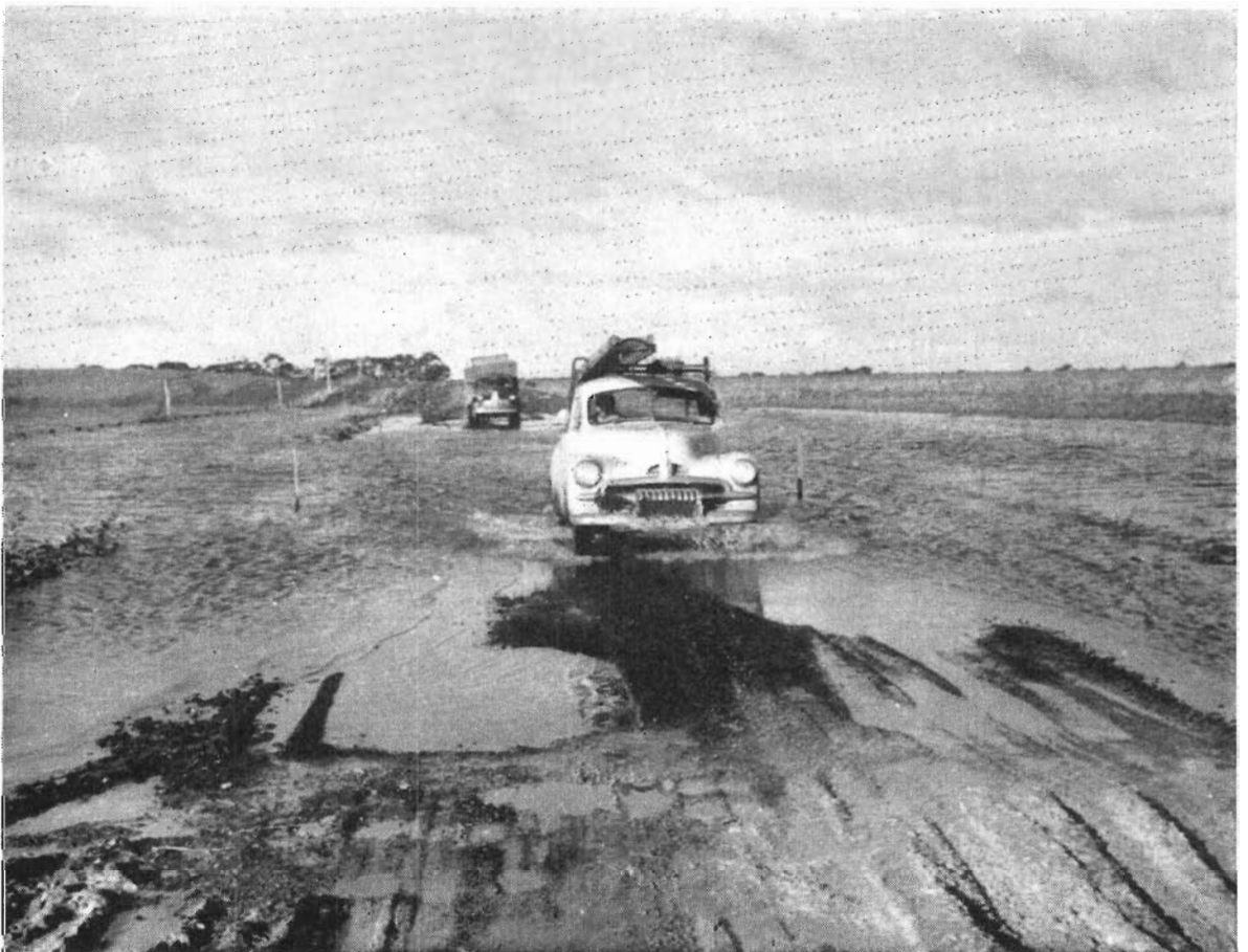
Plate No. 9 :—Midland Highway—Flood conditions—Near Corp.
