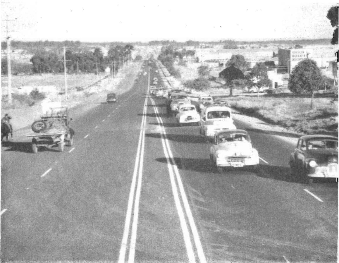
Plate No. 2 :—Princes Highway East, duplicated pavement approximately 1 mile west of Springvale.
