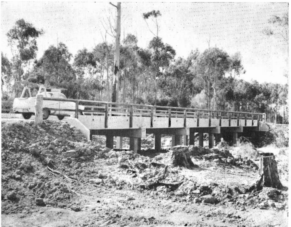
Plate No. 22 :—Heytesbury Soldier Settlement—Scott's Creek area new bridge over Coorimungle Creek, western section.
