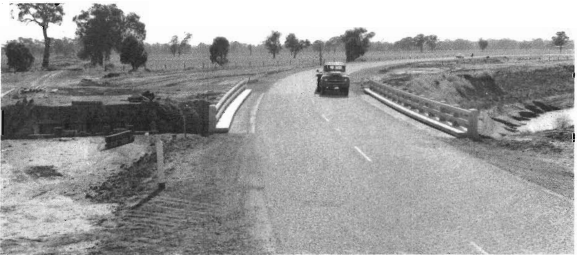
Plate No. 4 :—Goulburn Valley Highway—New bridge over irrigation channel at Wahring.
