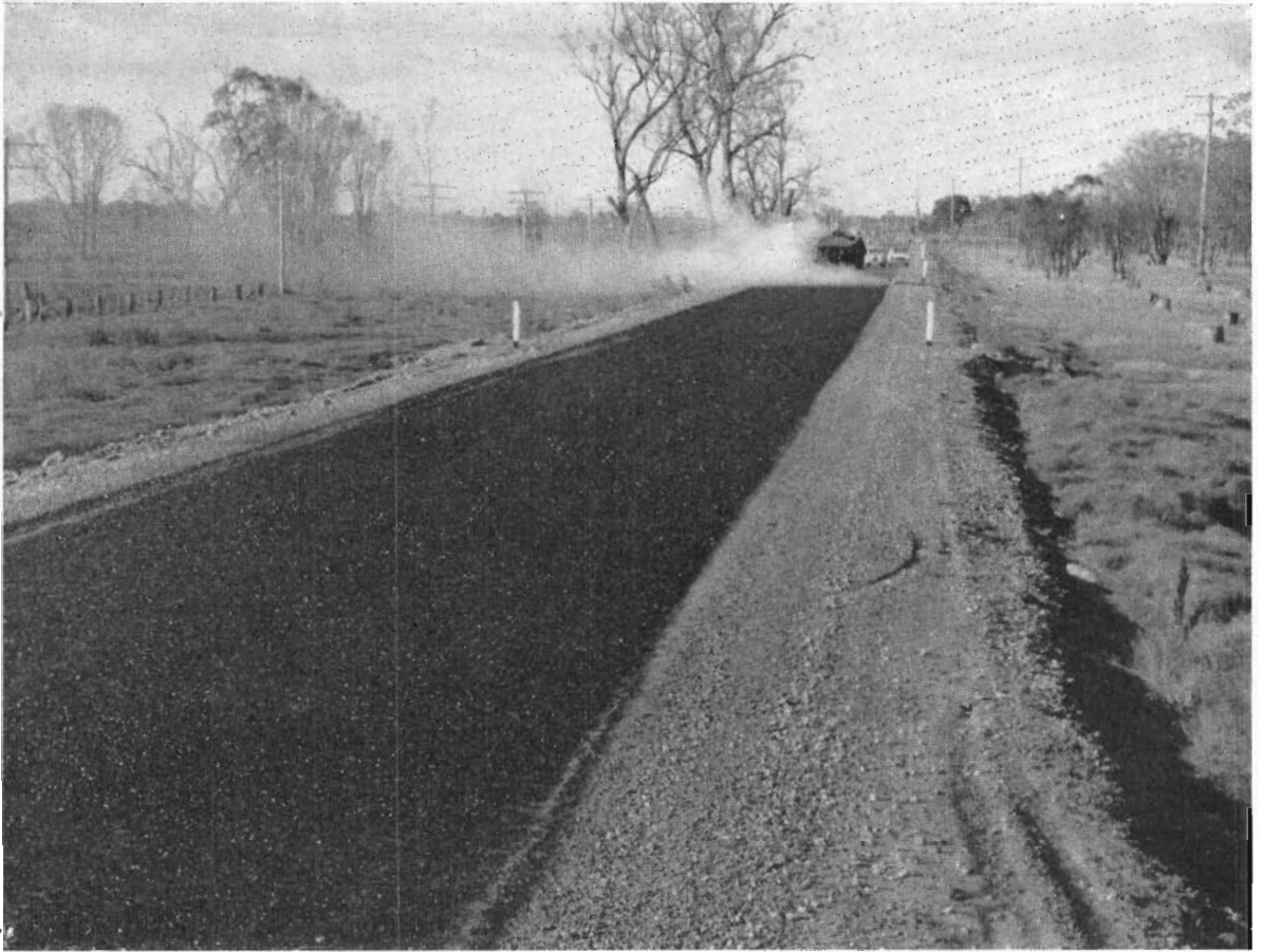
Plate No. 10 :—Midland Highway section 3—Sealing near Mooroopna township.
