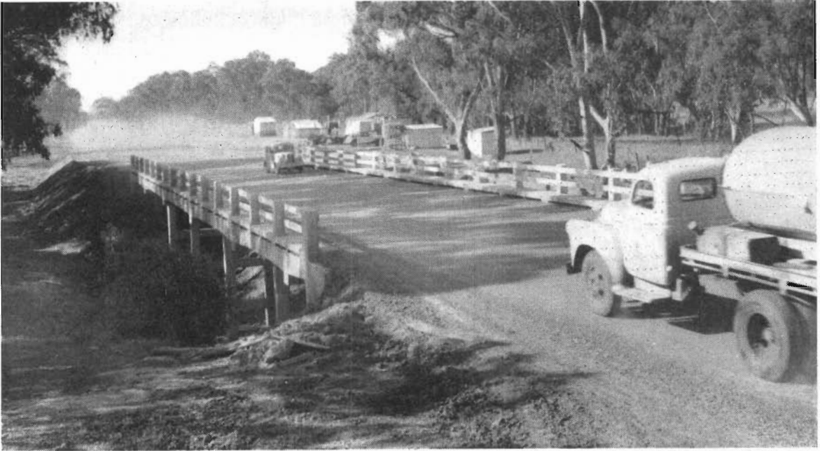
Plate No. 3 :—Goulburn Valley Highway—New bridge over Muddy Creek—between Wahring and Arcadia.
