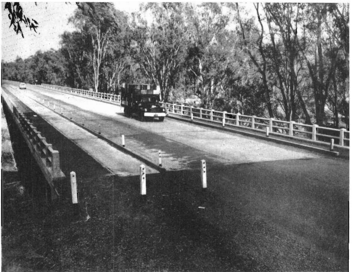
Plate No. 11 :—Midland Highway—Completed No. 2 bridge west of Shepparton.
