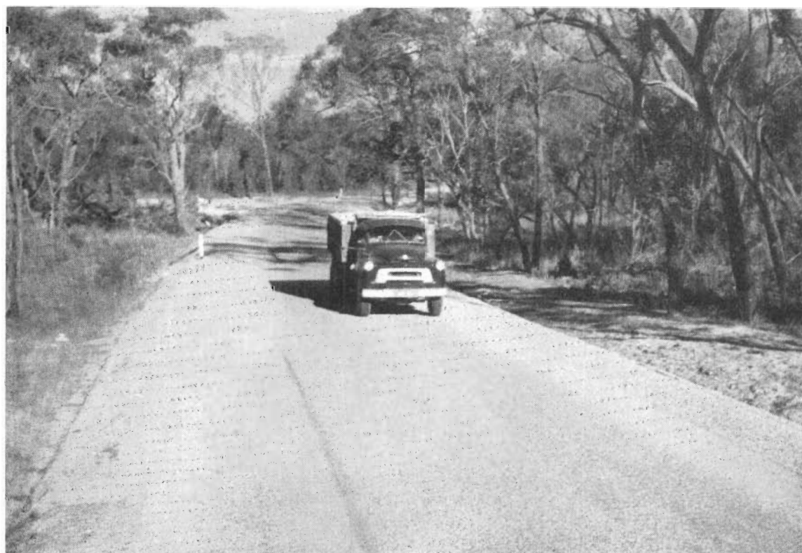
Plate No. 20 :—Rosedale–Stradbroke Road, which was constructed and sealed for the cartage of limestone.
