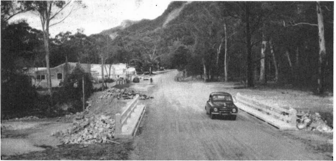
Plate No. 12 :—New bridge over Stony Creek and realignment and reconstruction of Grampians Road at Hall's Gap.
