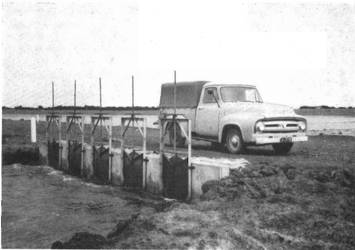
Lake Corangamite Project—Oftake regulator of the Woody Yaloak Diversion Channel. The Cundare Pool is in the background.
