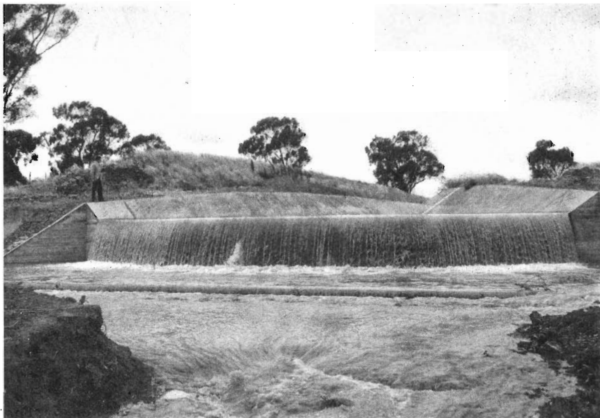
Murray Valley District—No. 1. Outfall from Yarrawonga Main Channel, remodelled during the year to increase its capacity from 300 cusecs to 900 cusecs.
