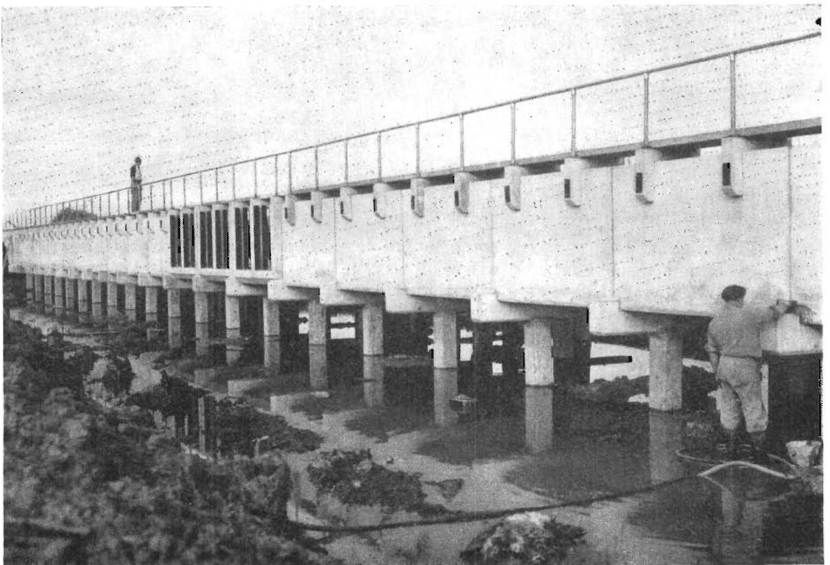
Kerang Centre—Flume on the Macorna Channel in the Torrumbarry Irrigation System constructed from pre-cast elements.
