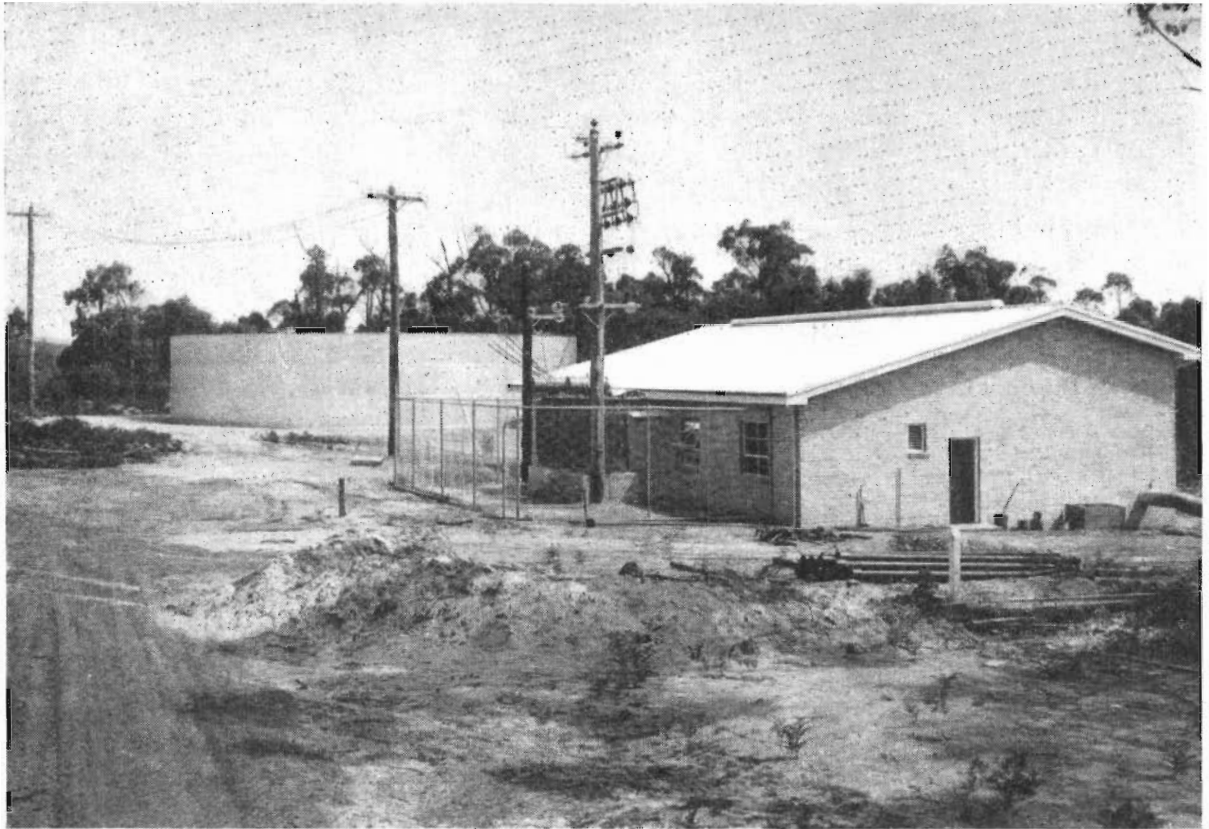
Otway System—The Gellibrand Main Station and 300,000 gallon steel tank from which water is injected into the Otway pipeline system to supplement supplies to Western District towns.
