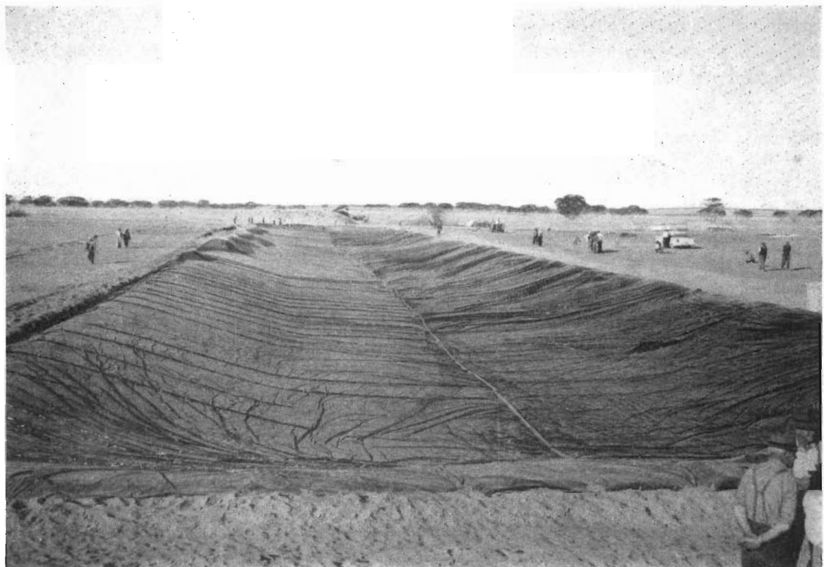
Ouyen storage with lining completed. Lining of the reservoir is designed to prevent seepage and permit accurate measurement of evaporation losses during experiments now being carried out by the C.S.I.R.O.
