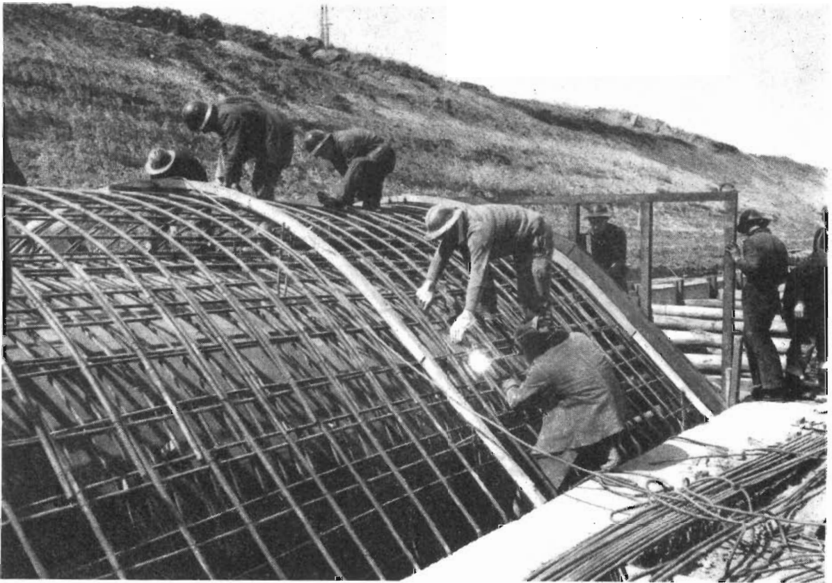
Construction of the 10 ft. 6 in. diameter reinforced concrete diversion culvert in progress. The culvert will carry the flow of the Tullaroop Creek under the embankment of the dam during construction and will later house the permanent outlet works.
