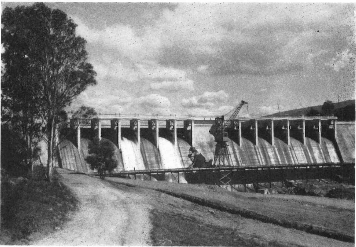
Glenmaggie Dam, on the Macalister River in Central Gippsland. The installation of spillway gates has increased the capacity of the storage from 104,500 to 154,300 acre feet.
