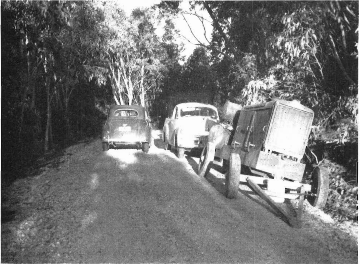
Plate 17.—Mount Buffalo Road. Narrow section leading to "The Horn" before widening.
