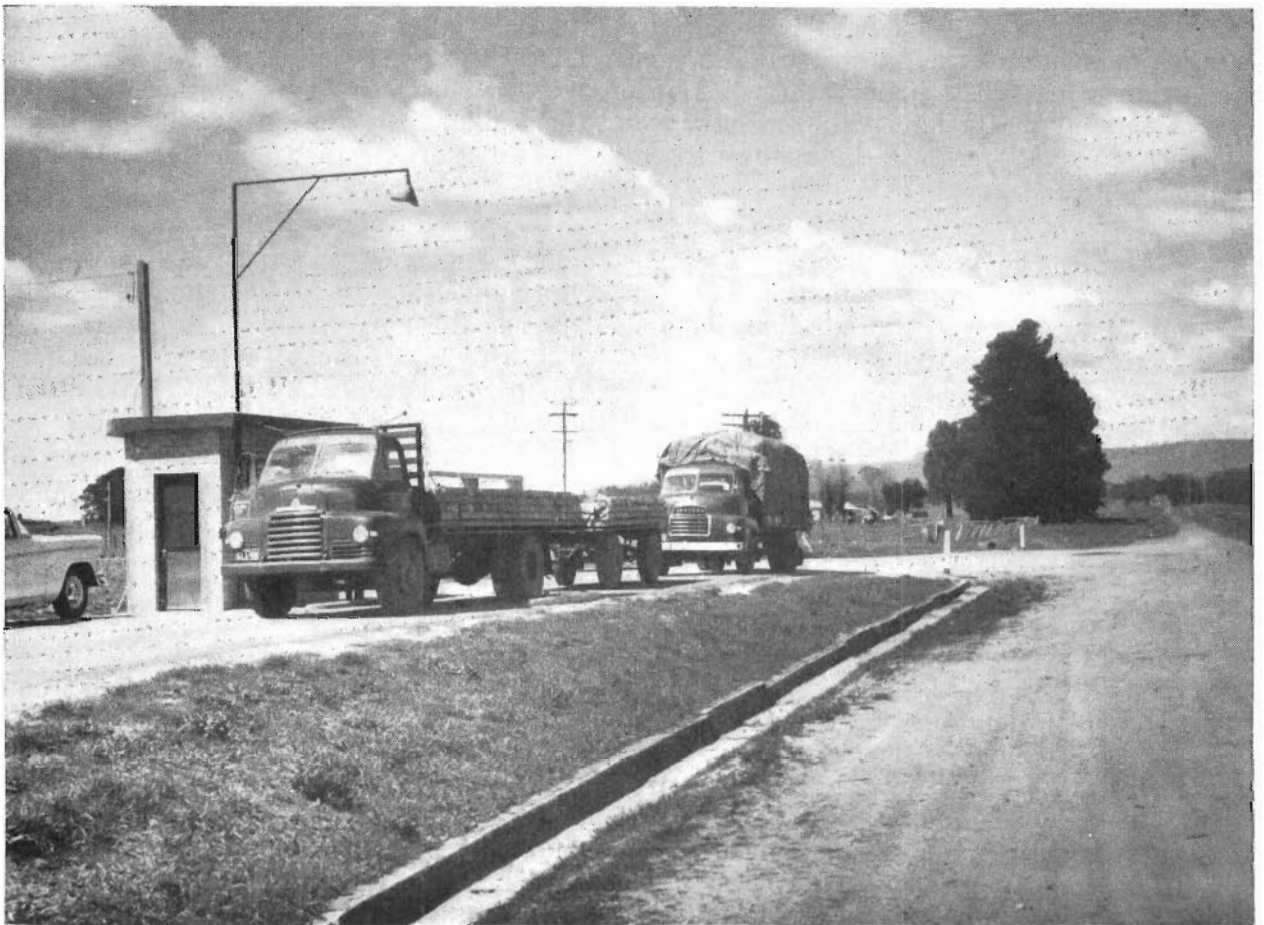
Plate 31.—Heavily loaded trucks being checked at Carlruhe Weighbridge, Calder Highway.
