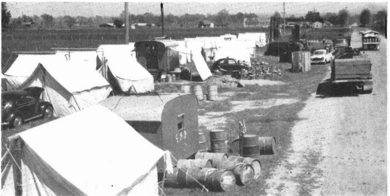
Plate 37.—Bitumen Spraying Camp alongside Traralgon—Maffra Road near Tinamba. Shire of Maffra.
