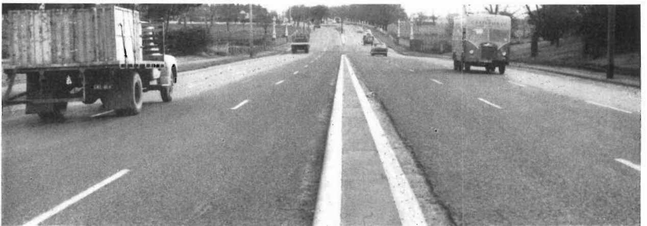
Plate 33.—Heidelberg City. Heidelberg-Eltham Road. Narrow median strip separating dual carriageways.
