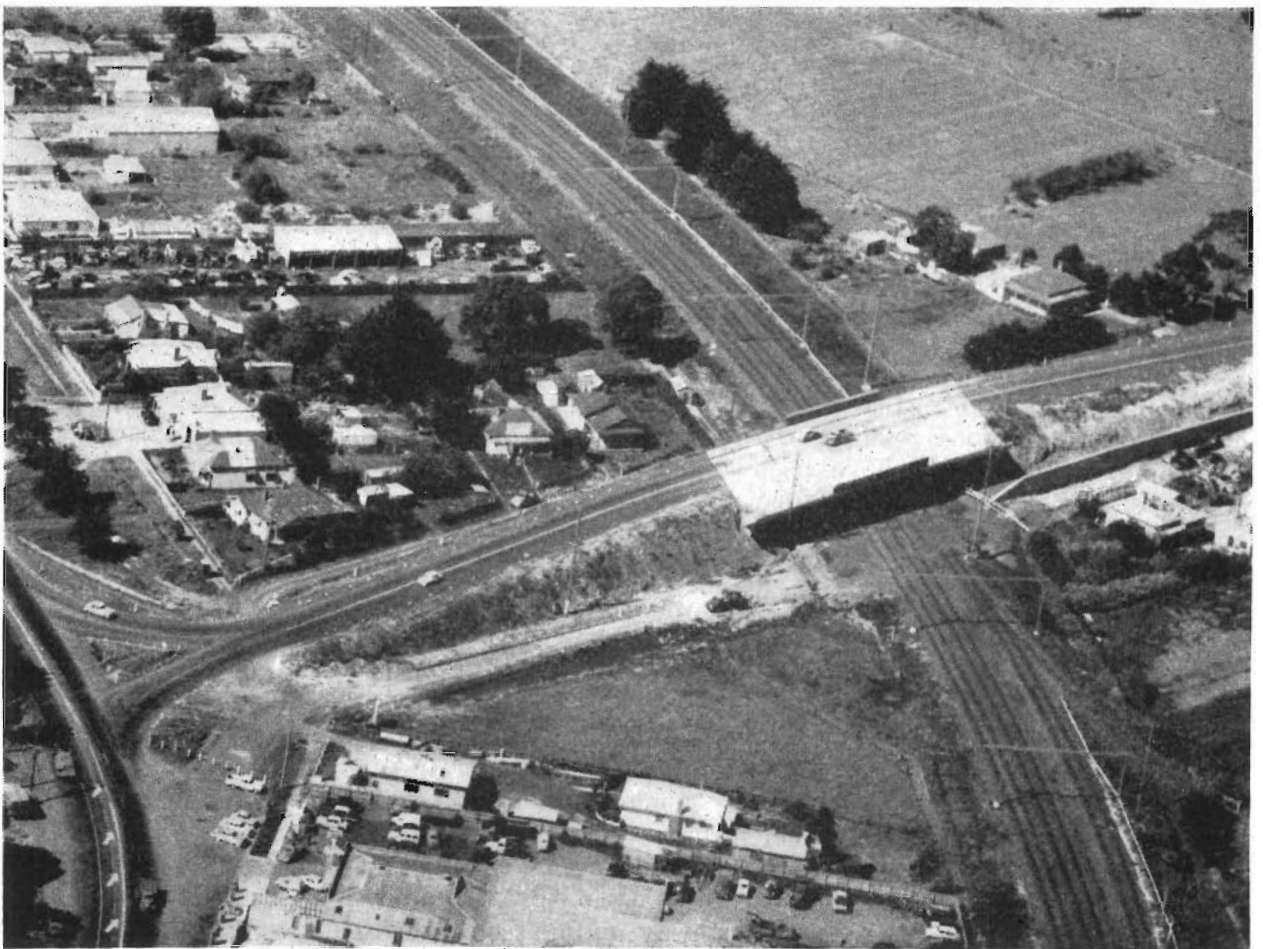
Plate 26.—Dandenong Shire. Dandenong—Frankston main road—Railway overpass at Dandenong.
