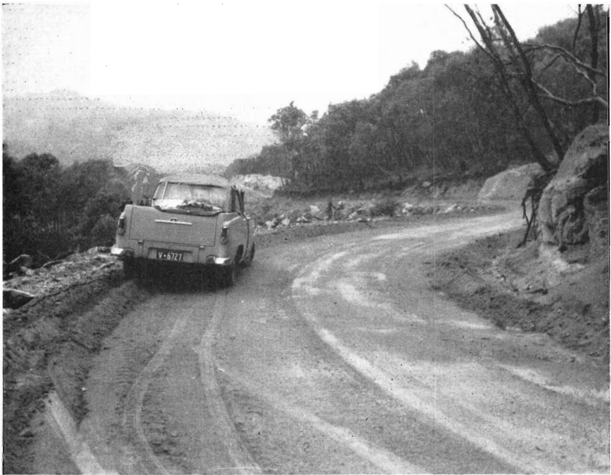
Plate 18.—Mount Buffalo Road. Widened section leading to "The Horn".
