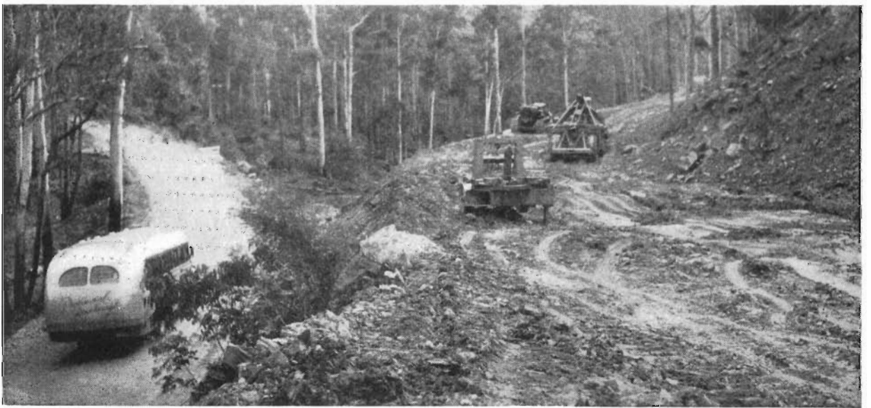
Plate 9.—Realignment and reconstruction of Pesca's Hill, Ballarat-Daylesford Road—Glenlyon Shire.
