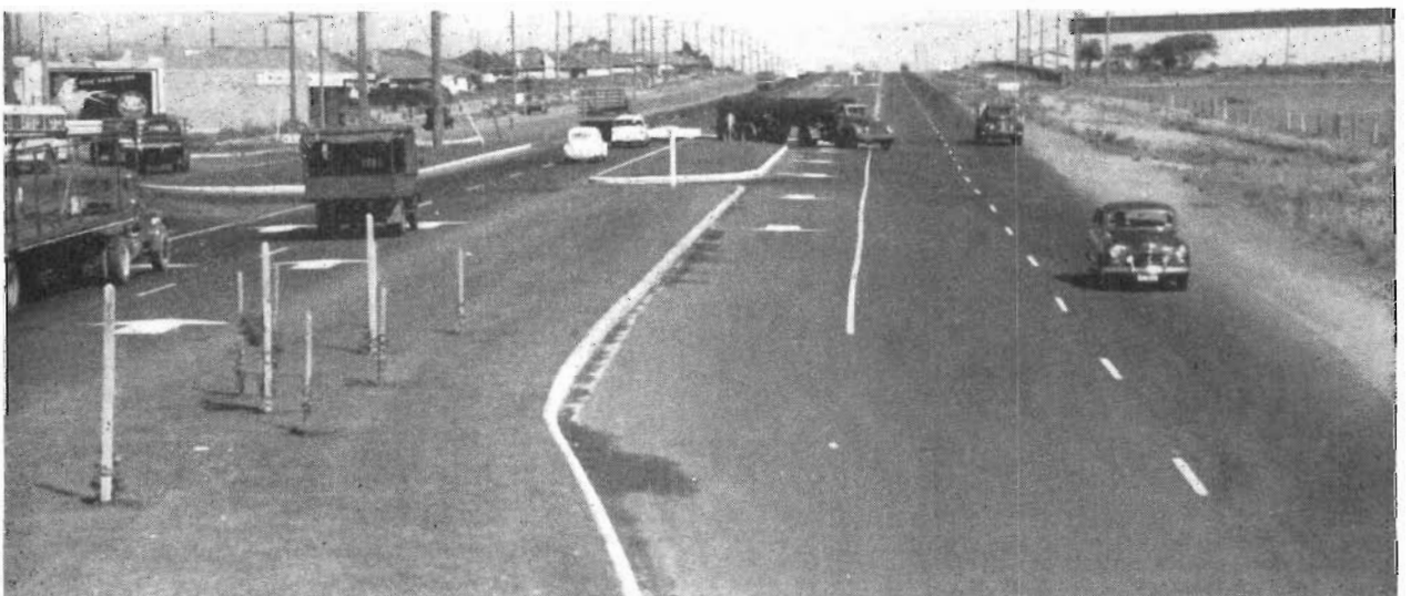
Plate 35.—Footscray City. Junction of Millers Road and Princes Highway West, showing shrub plantation in median strip with indentation of median for turning lane. Service road at left.
