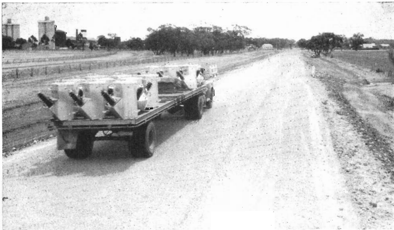
Plate 15.—Borong Highway. Reconstruction of failed section east of Warracknabeal.
