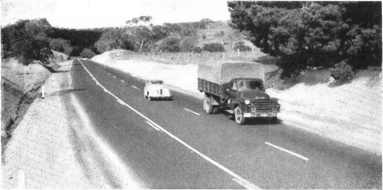
Plate 13.—Western Highway west of Pykes Creek Reservoir. Reconstruction of old, weak, tortuous section with extra up hill lane.
