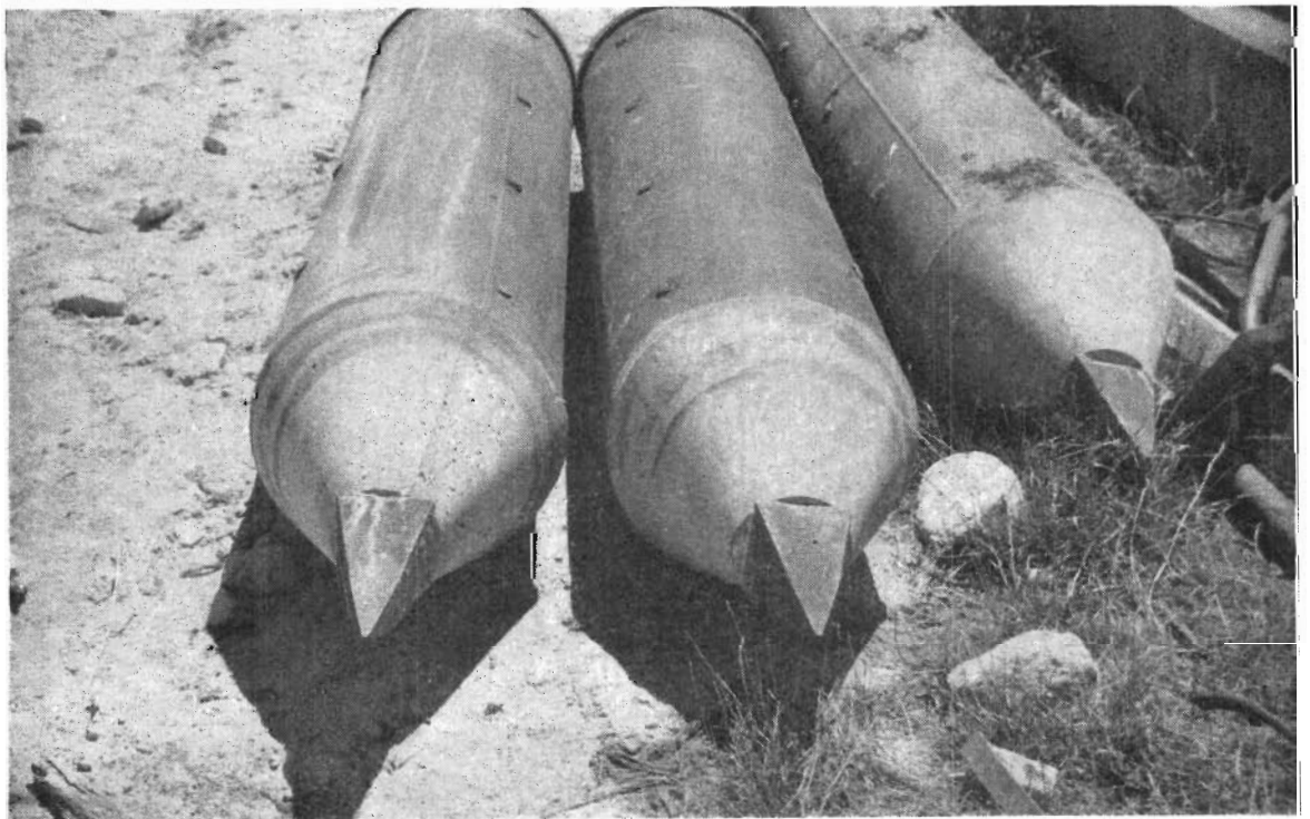
Plate 4.—Bottom section of steel tubular piles fitted with cast steel point.
