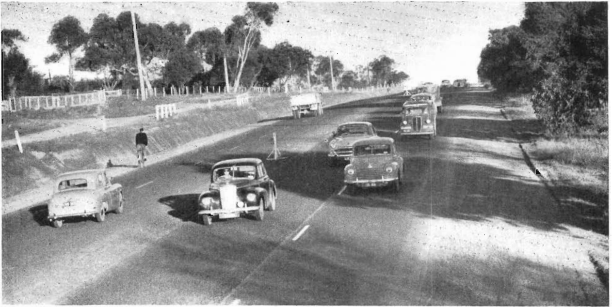
Plate 12.—Princes Highway East one mile west of Dandenong. Duplication of pavement.
