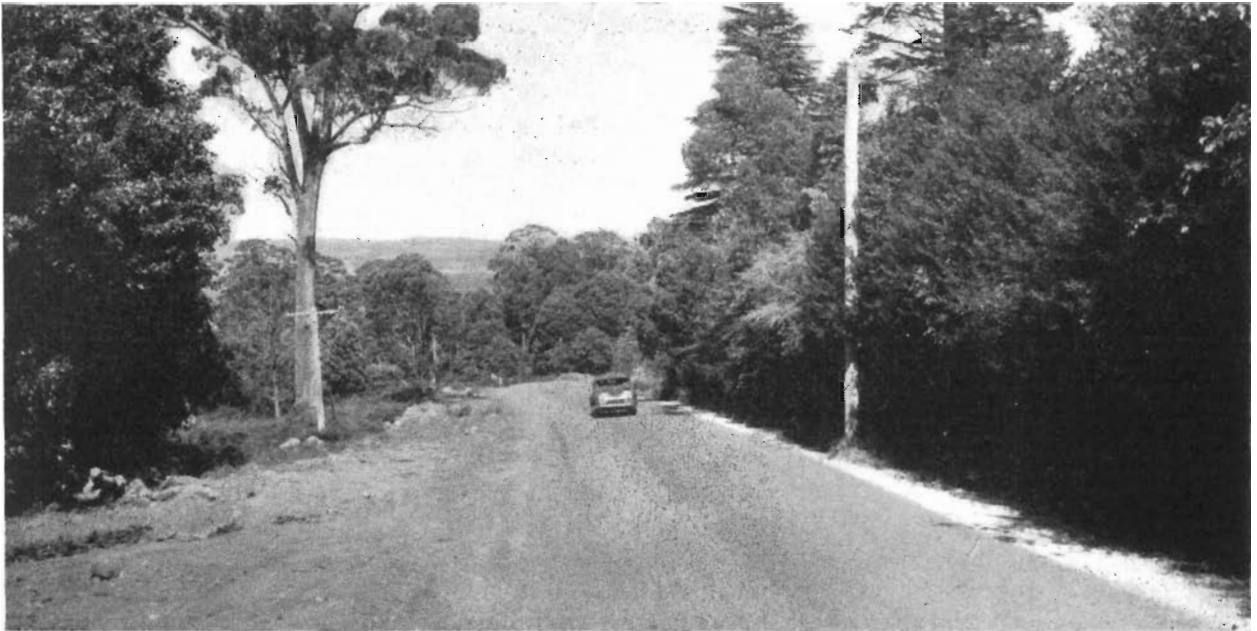
Plate 8.—Gisborne Shire—Mt. Macedon Road. Same section as in Plate 7 after reconstruction and widening.
