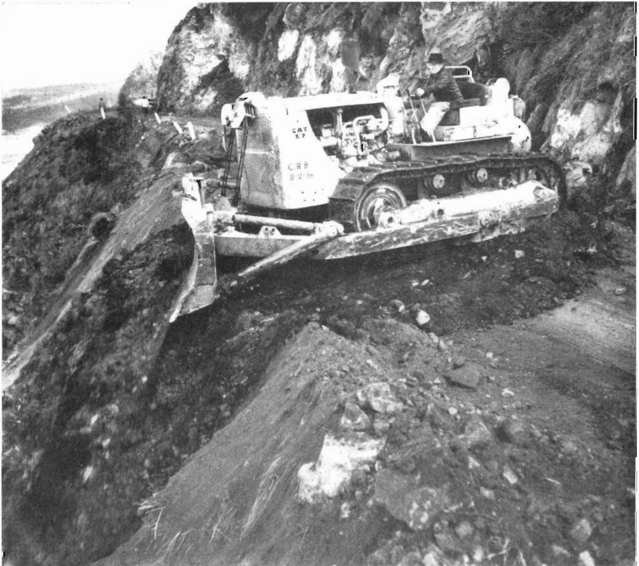
Plate 16.—Ocean Road. Widening in progress east of Wye River.
