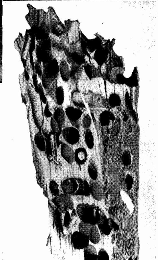
Plate No. 35.—A section of one of the piles riddled with teredo.
