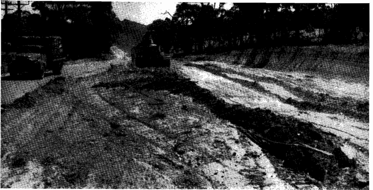
Plate No. 5.—Reconstruction in progress on Glenelg Highway east of Nintingbool.
