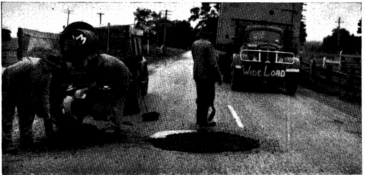
Plate No. 7.—Patching pot-hole on Hume Highway north of Glenrowan.
