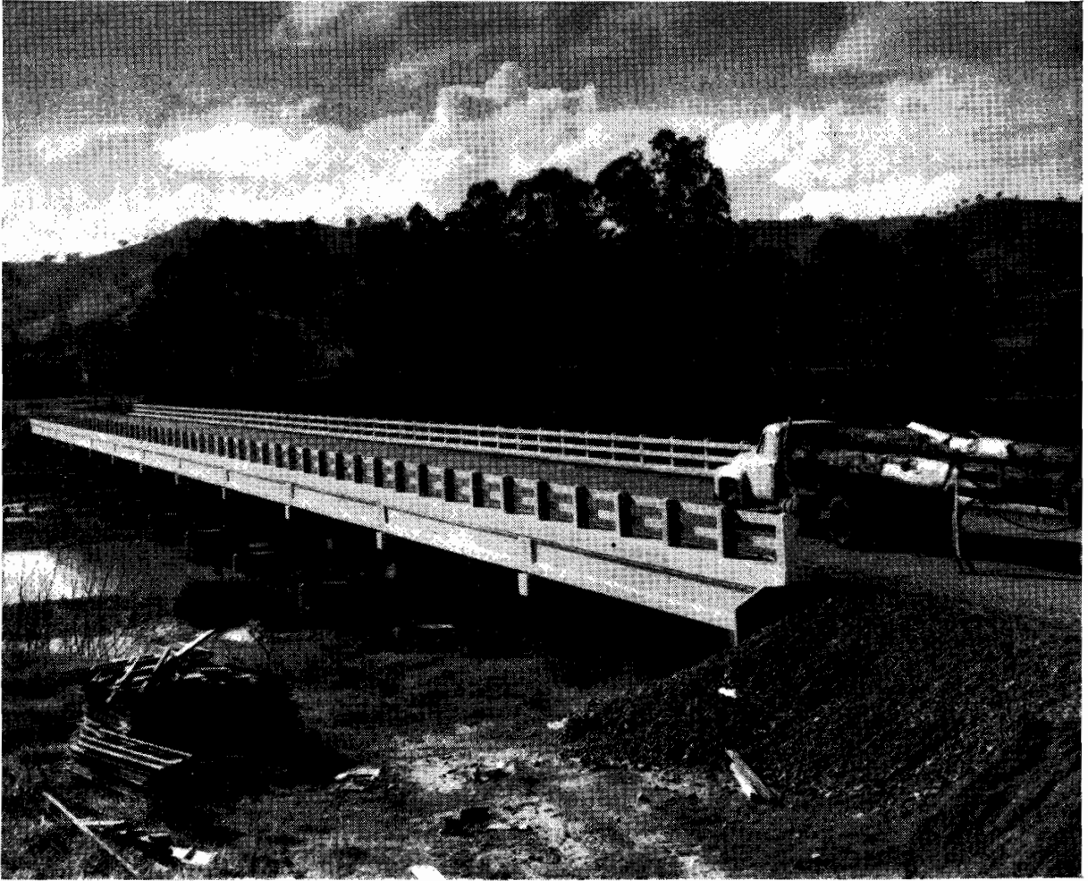
Plate No. 30.—New bridge over Goulburn River on the Upper Goulburn Road east of Alexandra.
