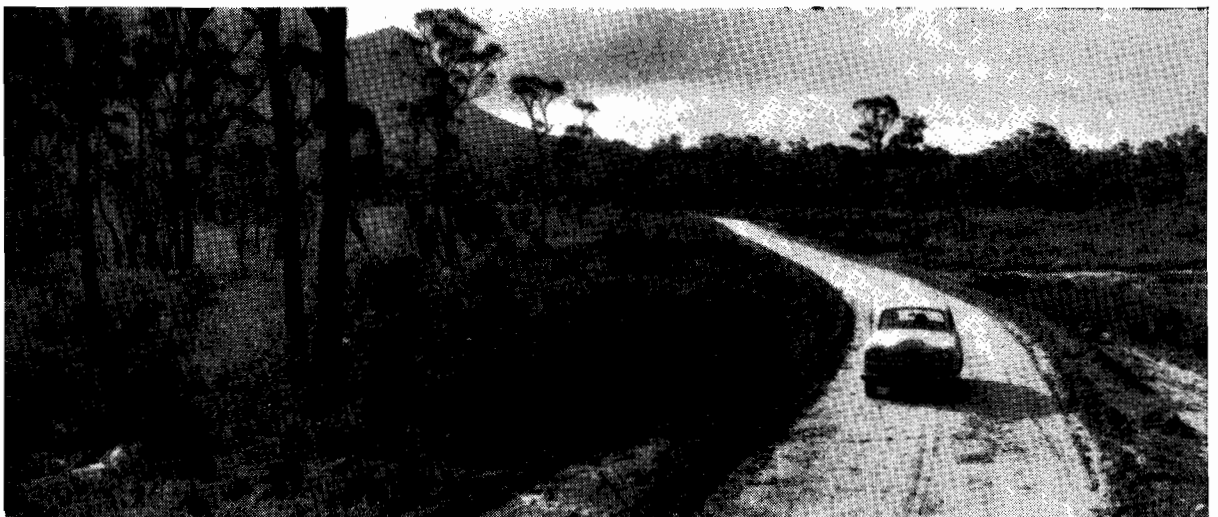
Plate No. 22.—Realigned and reconstructed section of Grampians Road approx. 6 miles west of Hall's Gap.
