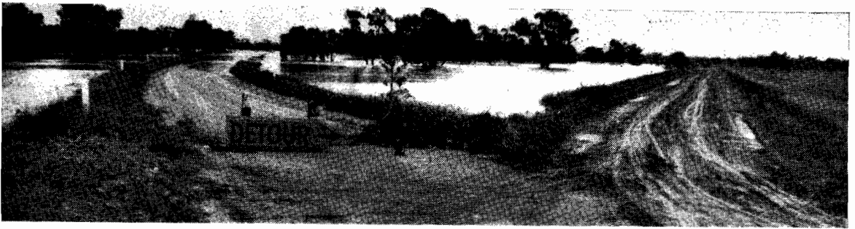
Plate No. 36.—A detour behind a levee bank at 36 miles, looking towards Swan Hill.
