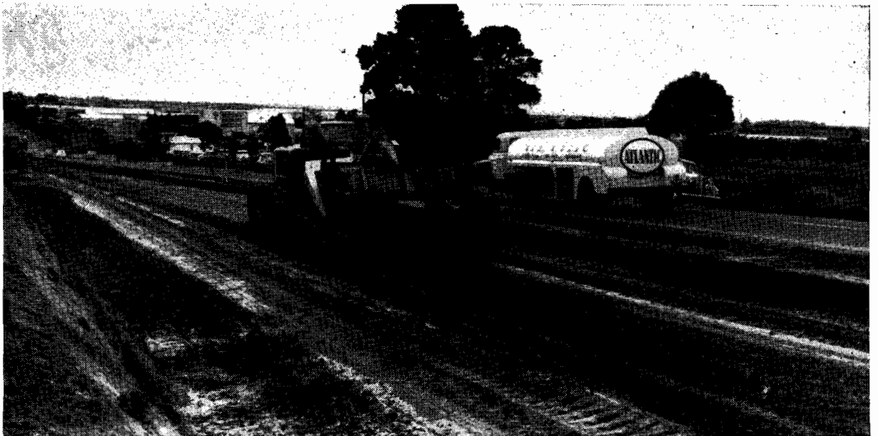
Plate No. 12.—Widening of Princes Highway East between Oakleigh and Dandenong.
