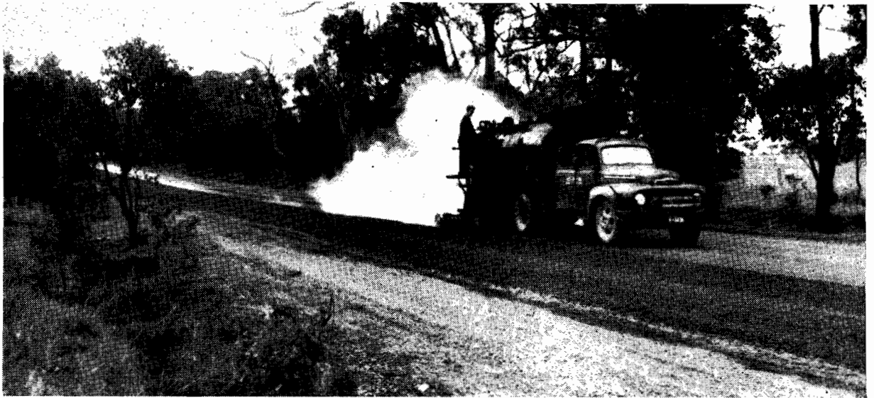
Plate No. 11.—Resealing in progress on Princes Highway East at Pakenham.
