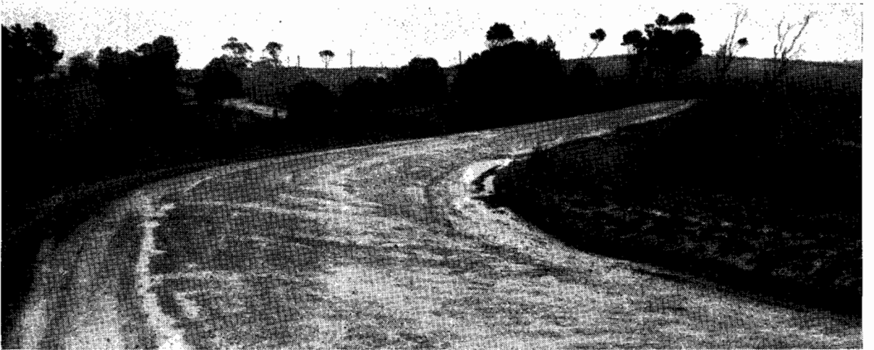
Plate No. 16.—Rough narrow twisting section of South Gippsland Highway between 67·9 and 69 miles which has been reconstructed.
