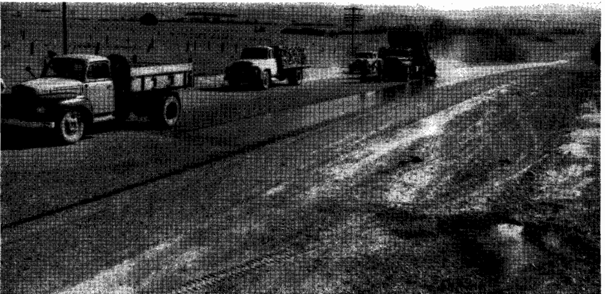
Plate No. 9.—Sealing a reconstructed and widened section of Maroondah Highway near Coldstream.
