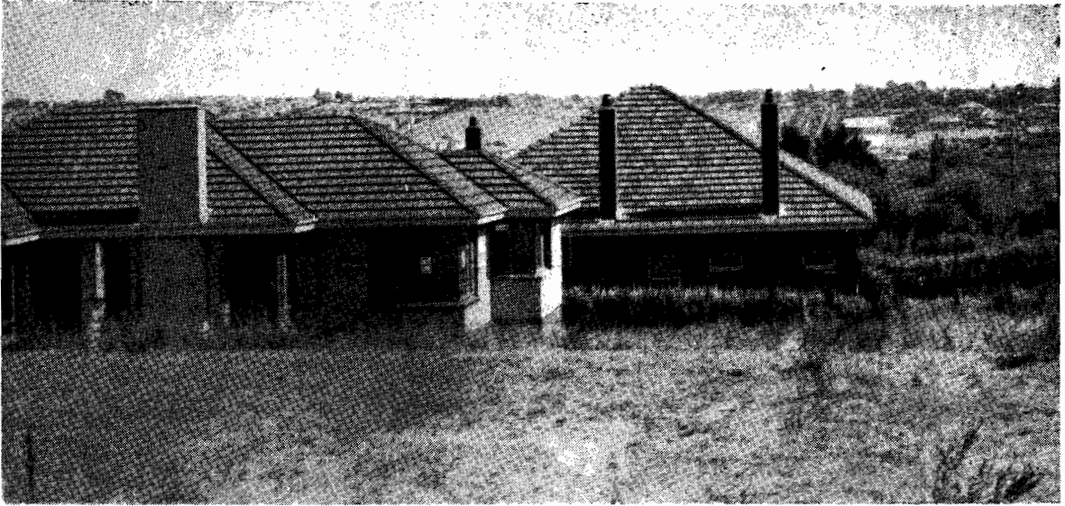
Plate No. 70.—Warrigal-road, Holmesglen, showing brick house before being moved.
