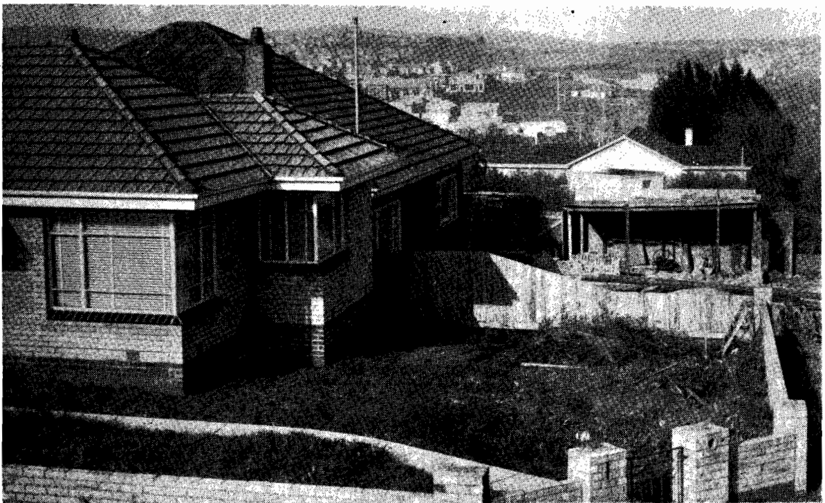
Plate No. 73.—House after removal.
