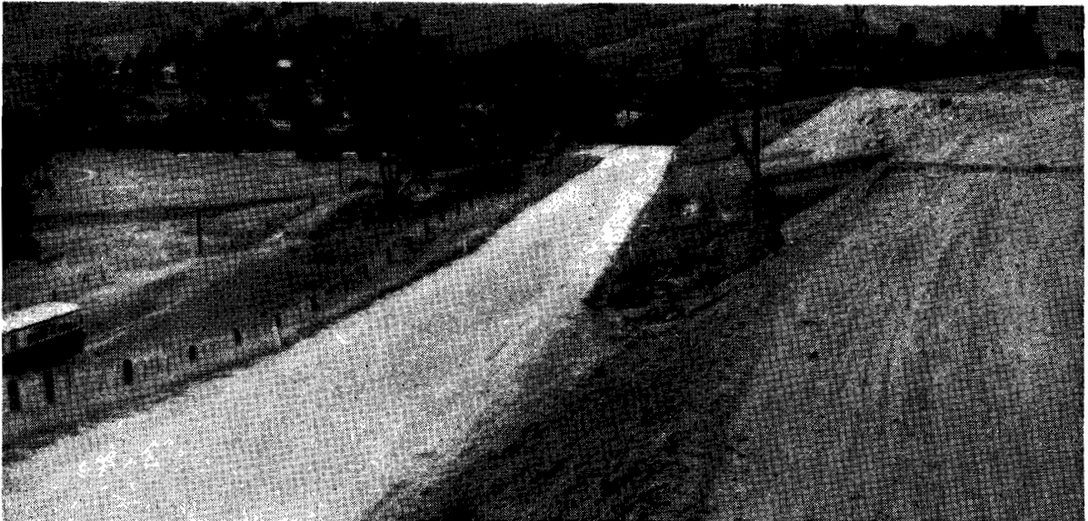
Plate No. 62.—New junction of Murray Valley and Omeo Highways at Tallangatta. The old junction will be submerged by the Hume Weir enlargement.
