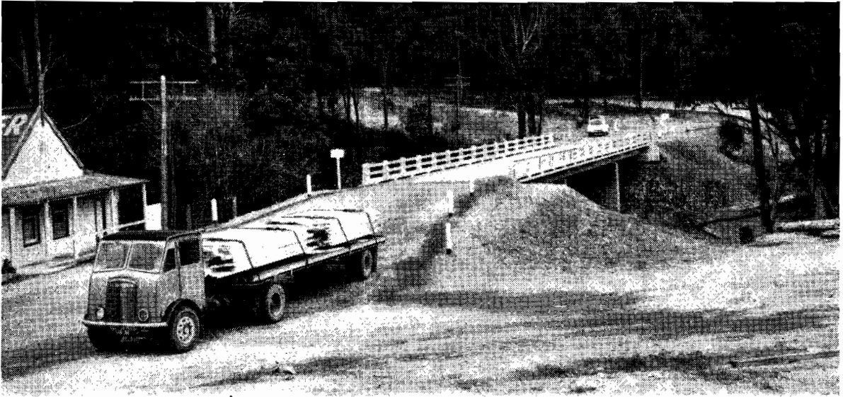
Plate No. 50.—New bridge on Walhalla Road over Tyers River at Gould.
