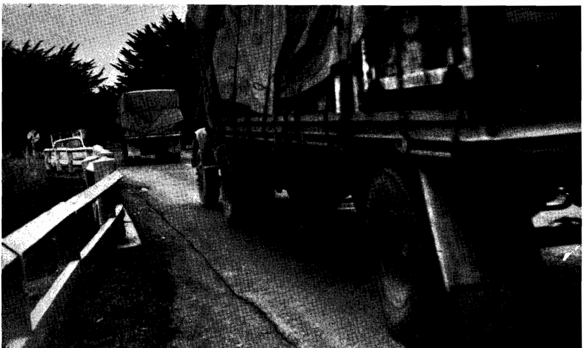
Plate No. 4.—Heavy transports on narrow bridge on Hume Highway at Kilmore, showing limited clearance.
