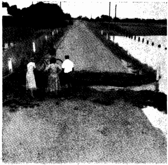
Plate No. 54.—Shepparton-Tatura Road cut by 6-ft. drain to draw floodwaters away from Tatura township.
