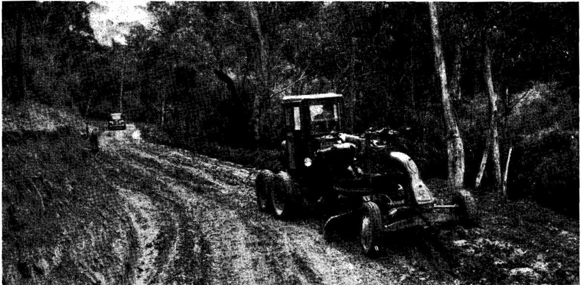
Plate No. 32.—Widening and reconstruction of the narrow Silverband Road, Grampians.
