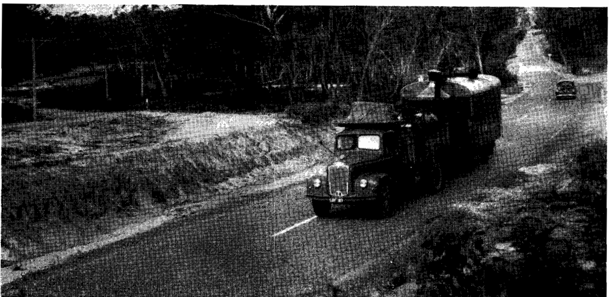
Plate No. 28.—Country Roads Board mobile kitchen on a reconstructed and re-aligned section of South Gippsland Highway, near Stradbroke.
