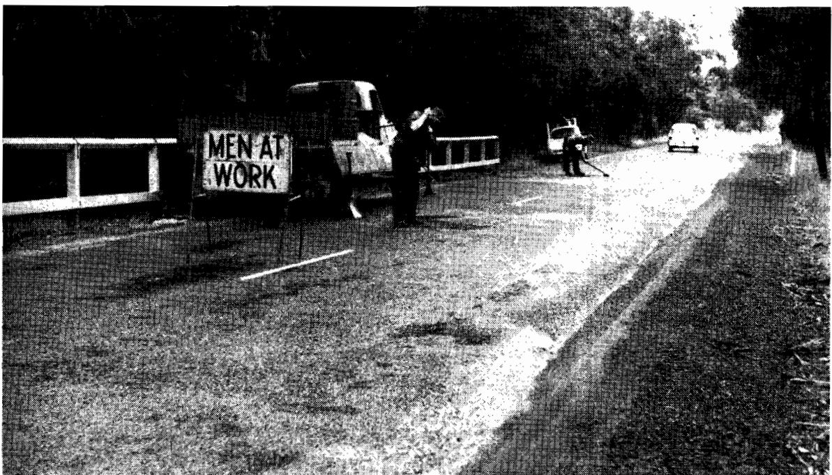
Plate No. 19.—Patching in progress on Princes Highway East, 39 miles.
