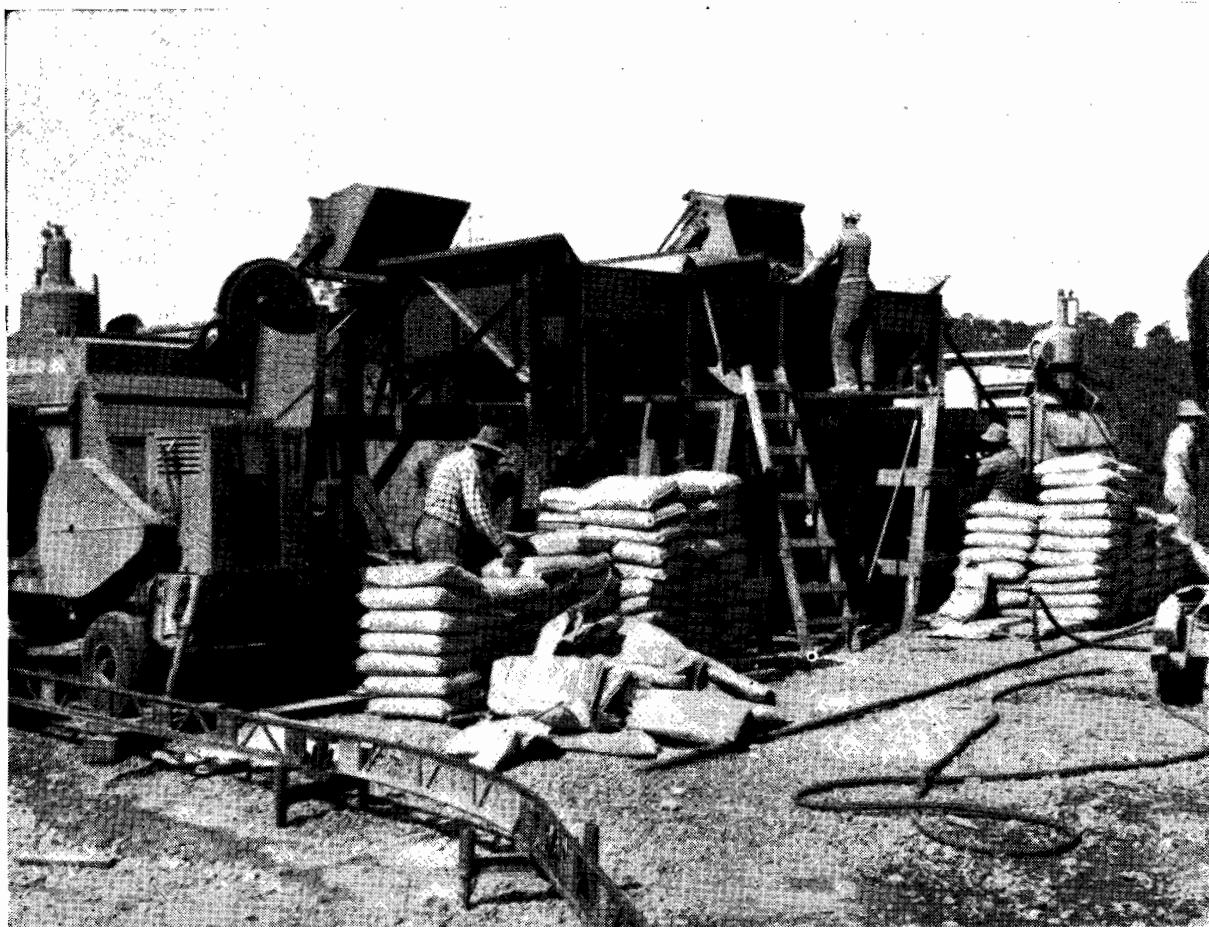
Fig. 7.—20-ton trolley weigh batcher serving two \frac{1}{2} -cub.-yd. mixers.
