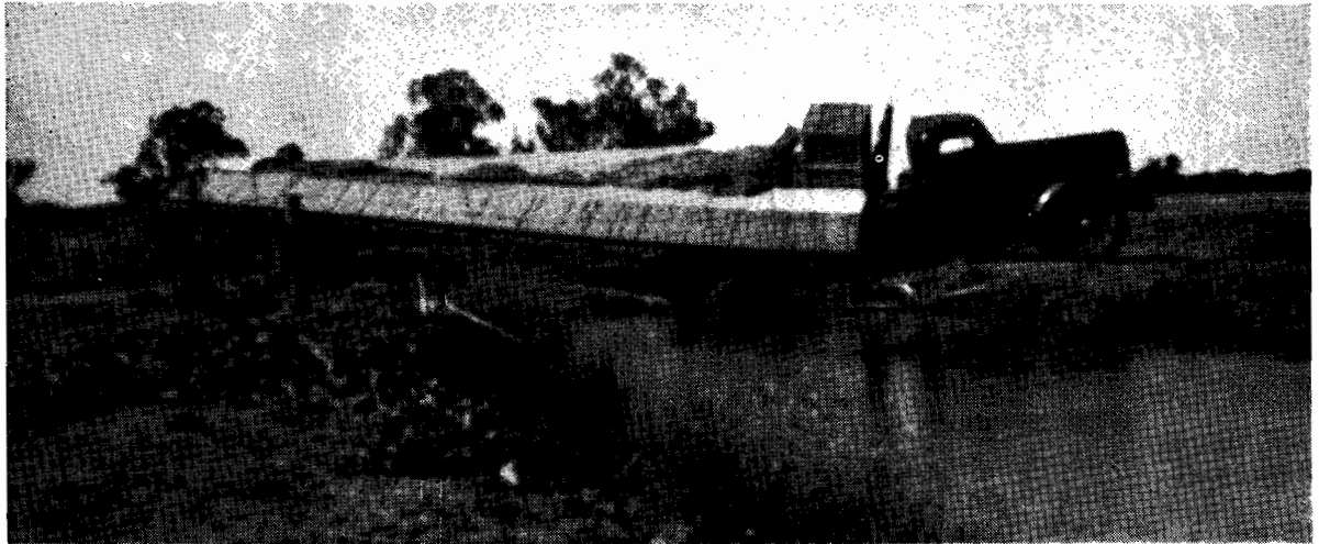
Plate No. 3.—Transport on collapsed State Rivers and Water Supply Commission bridge in Kerang Shire.
