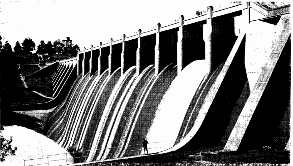
Lauriston Dam.—This concrete massive buttress dam with rockfill end embankments on the Coliban River has a total length of 800 feet and a height of 116 feet. The reservoir has a capacity of 16,000 acre-feet of water, which is reserved for the maintenance of supplies in recurrent low-rainfall periods in the Coliban system.
