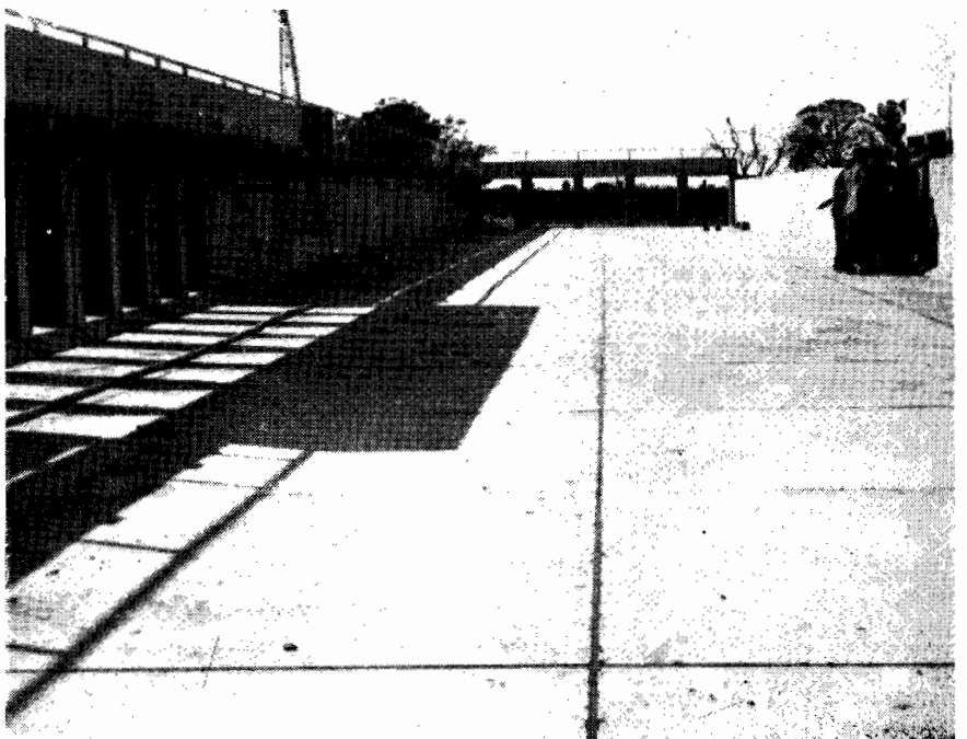
Macorna Channel Flume. —Pre-cast reinforced concrete elevated flume on the Macorna Channel at the Pyramid Creek crossing. The flume is 30 feet wide, 5 feet 3 inches deep and 223 feet long, and has a capacity of 350 cusecs. It is supported on piers and beams at 9-ft. intervals. The L-sections and slabs used in construction were pre-cast at the Central Plant Workshops, Bendigo, and transported by road to the works site.
