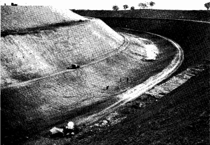
The Goulburn - Waranga Second Channel now under construction will have a capacity of 1,500 cusecs and a length of 14½ miles. Its construction involves excavation of 5,032,000 cubic yards of earth, the cut varying from 7 to 63 feet in depth and from 20 to 48 feet in bedwidth. The new channel will permit full advantage to be taken of increased water supplies from Eildon Reservoir.
