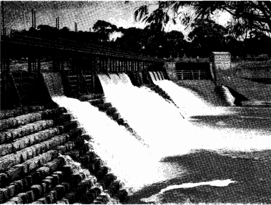
Goulburn Weir, on the Goulburn River near Nagambie, diverts water released from Eildon Reservoir to the East Goulburn Main Channel on one side of the river, and to Waranga Reservoir on the other. The weir is 550 feet long and is 57 feet in height. The structure is of mass concrete faced with granite masonry, and is fitted with flood control gates. Construction of the weir commenced in 1887 and it was thus one of the first water supply works undertaken in Victoria.
