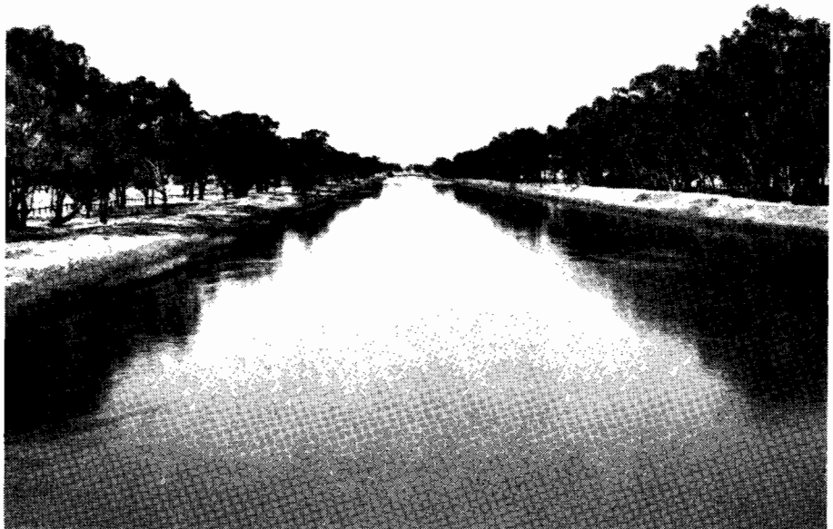
Goulburn-Waranga First Channel, between the Goulburn Weir and Waranga Reservoir, was completed in 1891. It has a capacity of 1,723 cusecs and is 23½ miles in length. Water delivered to Waranga Reservoir is distributed through the Waranga Western Main Channel to the Tongala, Stanhope, Deakin, Rochester, Dingee, Calivil, Tragowel Plains, and Boort irrigation districts.
