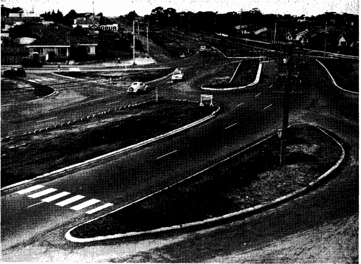
Plate No. 16.—Channelization at Corner of Nepean Highway and Warrigal Road, Mentone.
