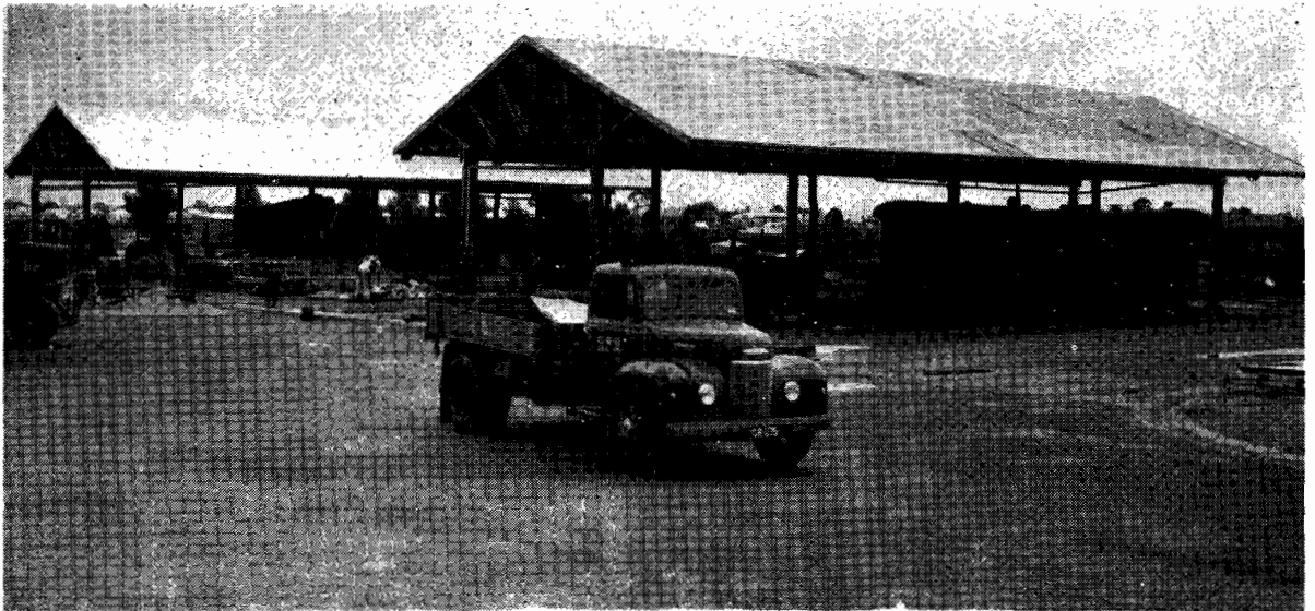
Plate No. 50.—Plant Shelters at Horsham Divisional Workshops.
