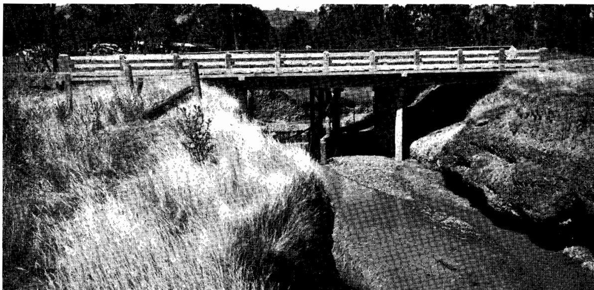
Plate No. 24.—Precast Reinforced Concrete Bridge over U.T. Creek on the Upper Goulburn Road.
