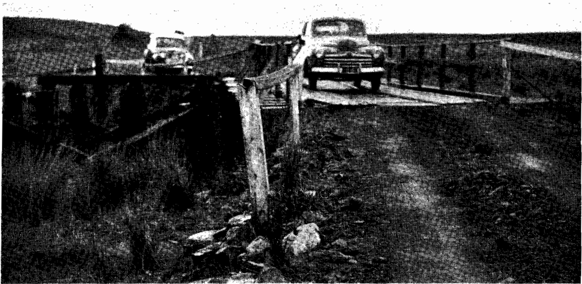
Plate No. 19.—Old Bridge and Temporary Bridge over Moyne River on Spencer Road, Shire of Belfast.
