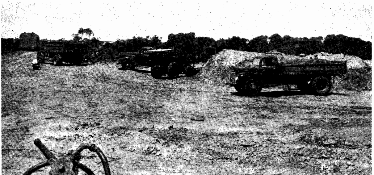
Plate No. 48.—Loading Sandy Clay for Base Course.
