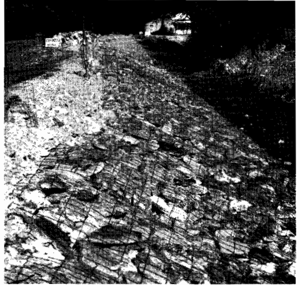
Plate No. 37.—Stone Filled Mesh Type of Bank Protection at Stringer's Creek, Walhalla.
