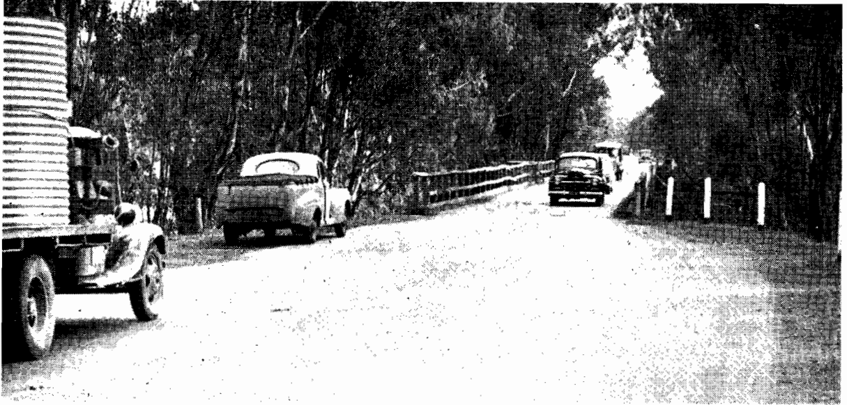
Plate No. 4.—A Narrow, Weak Bridge on the Midland Highway near Shepparton. This bridge carries heavy traffic over the Goulburn River.
