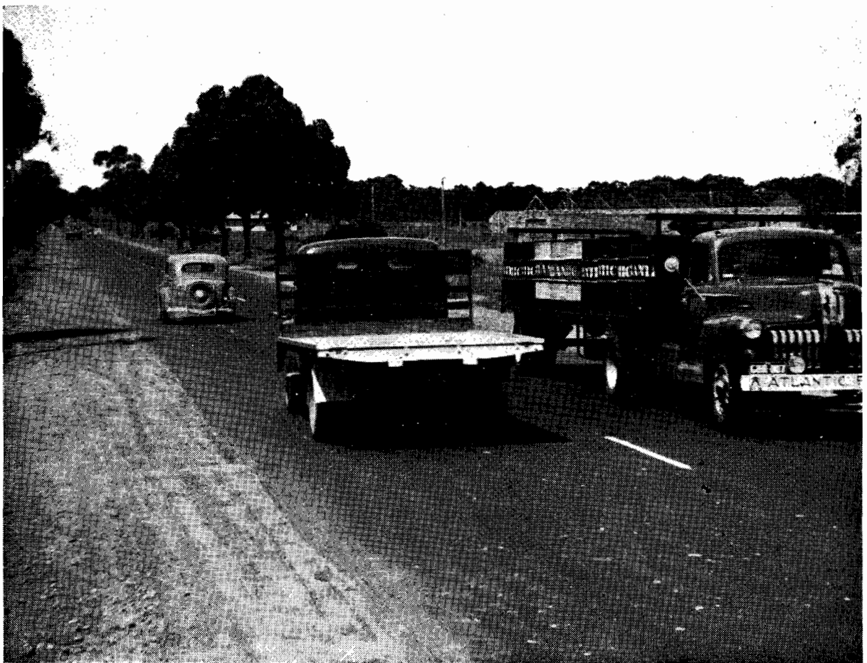
Plate No. 15.—Same Section after Widening and Resurfacing.
