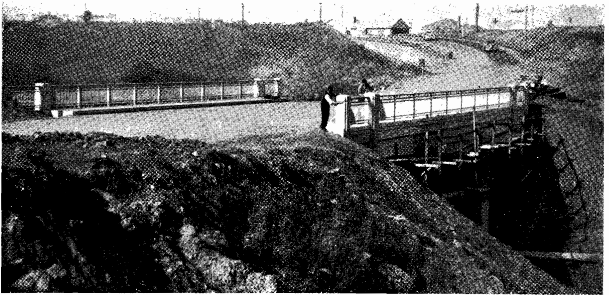
Plate No. 33.—Bridge over Darebin Creek in Bell Street, Preston.
