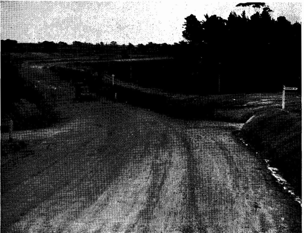
Plate No. 17.—Approaches to the New Concrete Bridge on the South Gippsland Highway at the Agnes River.
