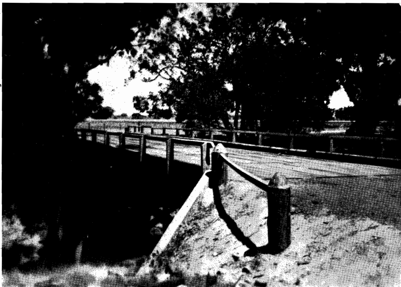
Fig. 7. Low handrails to permit passage of agricultural machinery.
