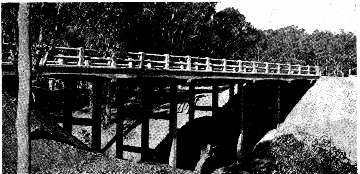
Plate No. 23.—Newly Completed Reinforced Concrete Bridge.
