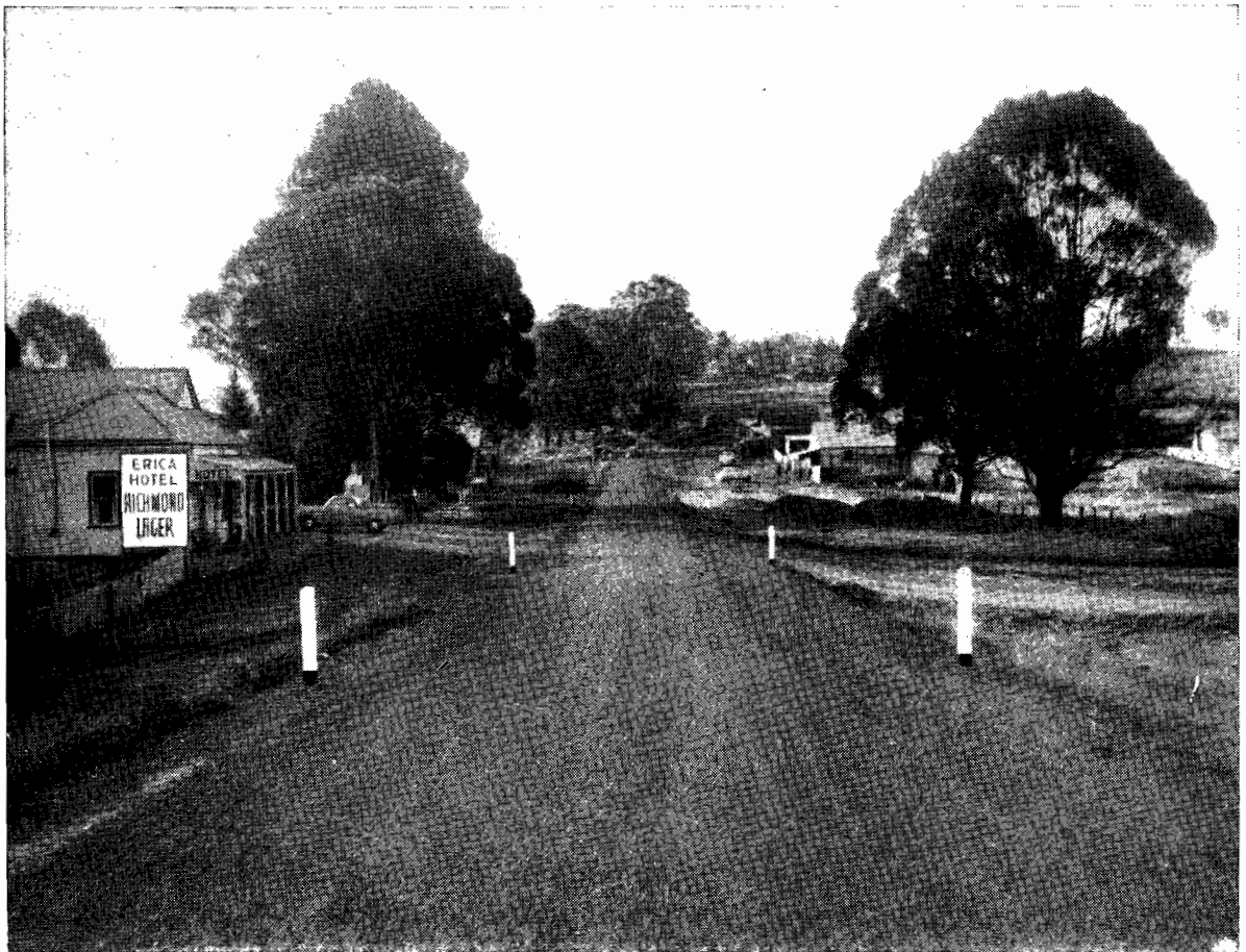
Plate No. 25.—View of completed reconstruction and sealing of Walhalla Road, Erica Township.
