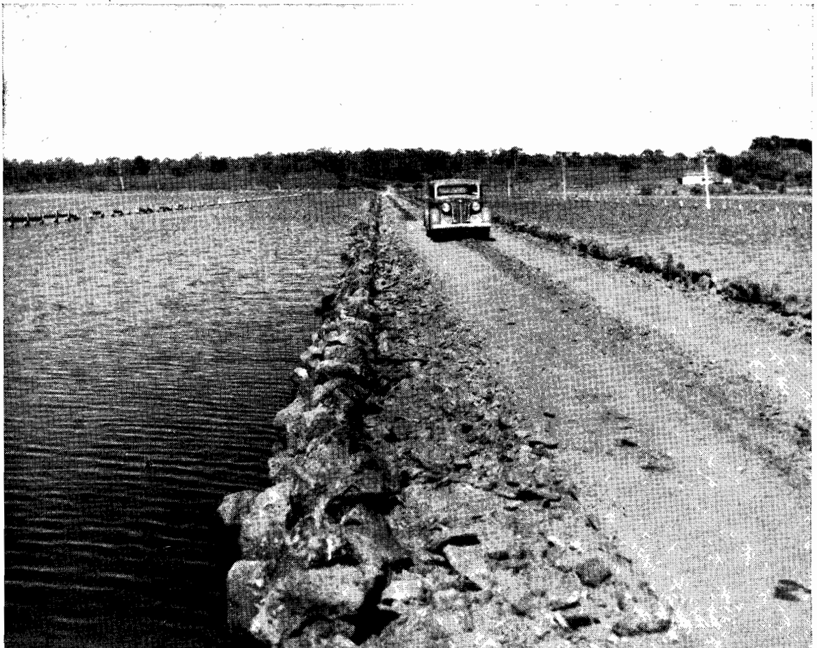
Plate No. 43.—Reconstructed causeway on Hawks Nest Road above the rising waters of Lake Corangamite.
