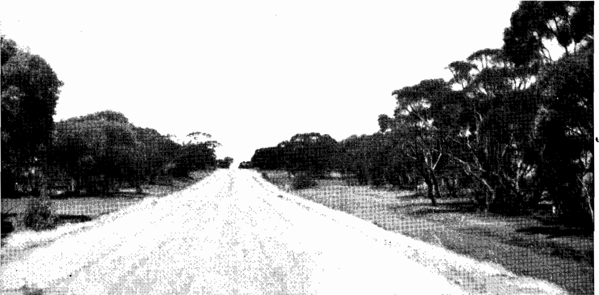
Plate No. 5.—Robinvale Road, Swan Hill Shire, section resheeted and sealed.
