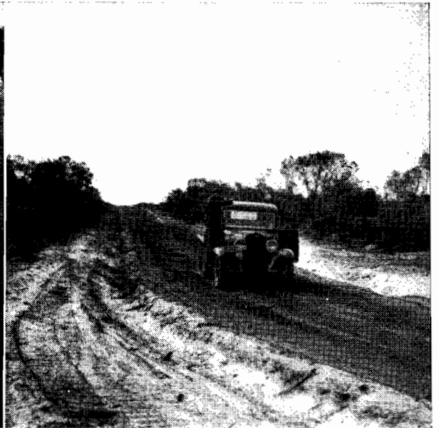
Plate No. 28.—New construction on road north from Tankerton, French Island.
