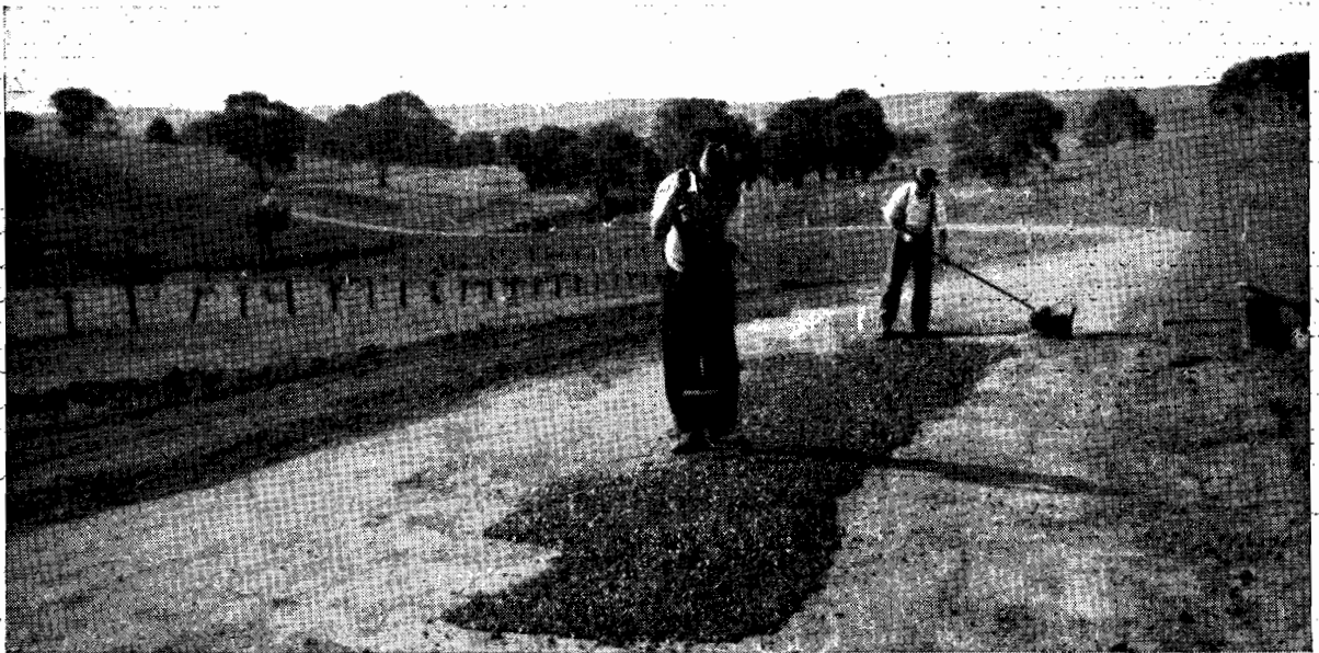
Plate No. 3.—Heavy patching on Portland-Casterton Road near Henty.
