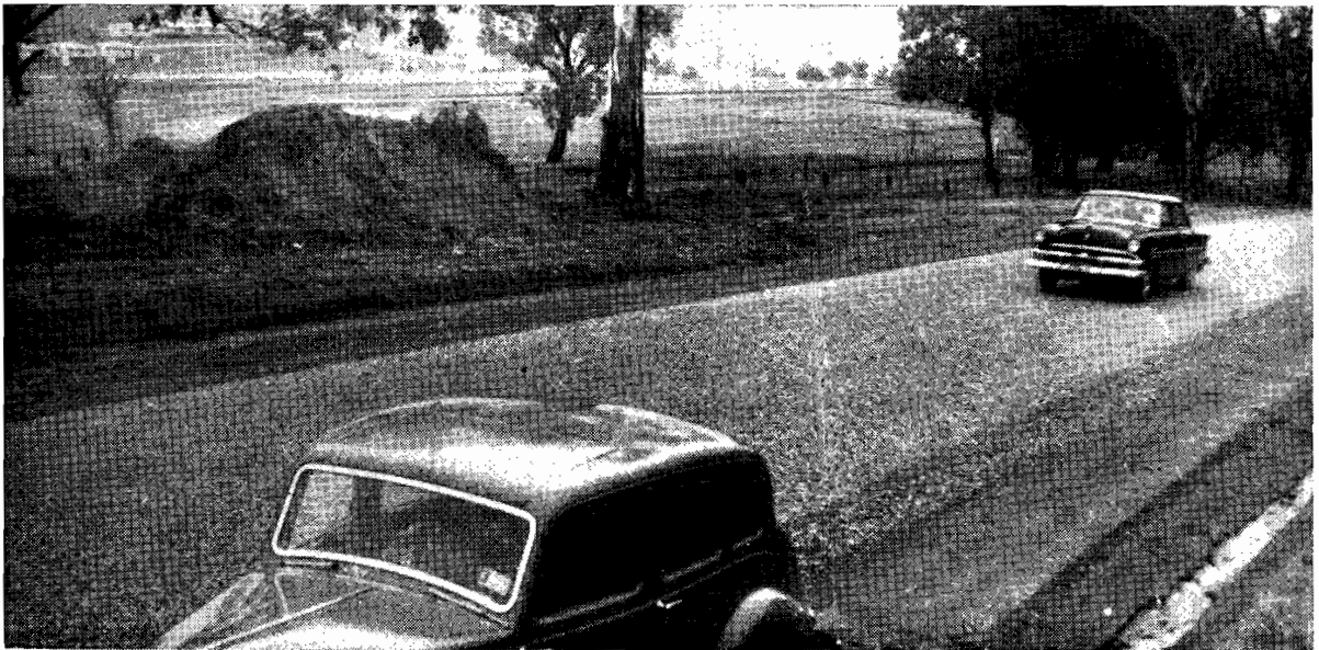
Plate No. 16.—A reconstructed and sealed section of the Murray Valley Highway at Bolga.
