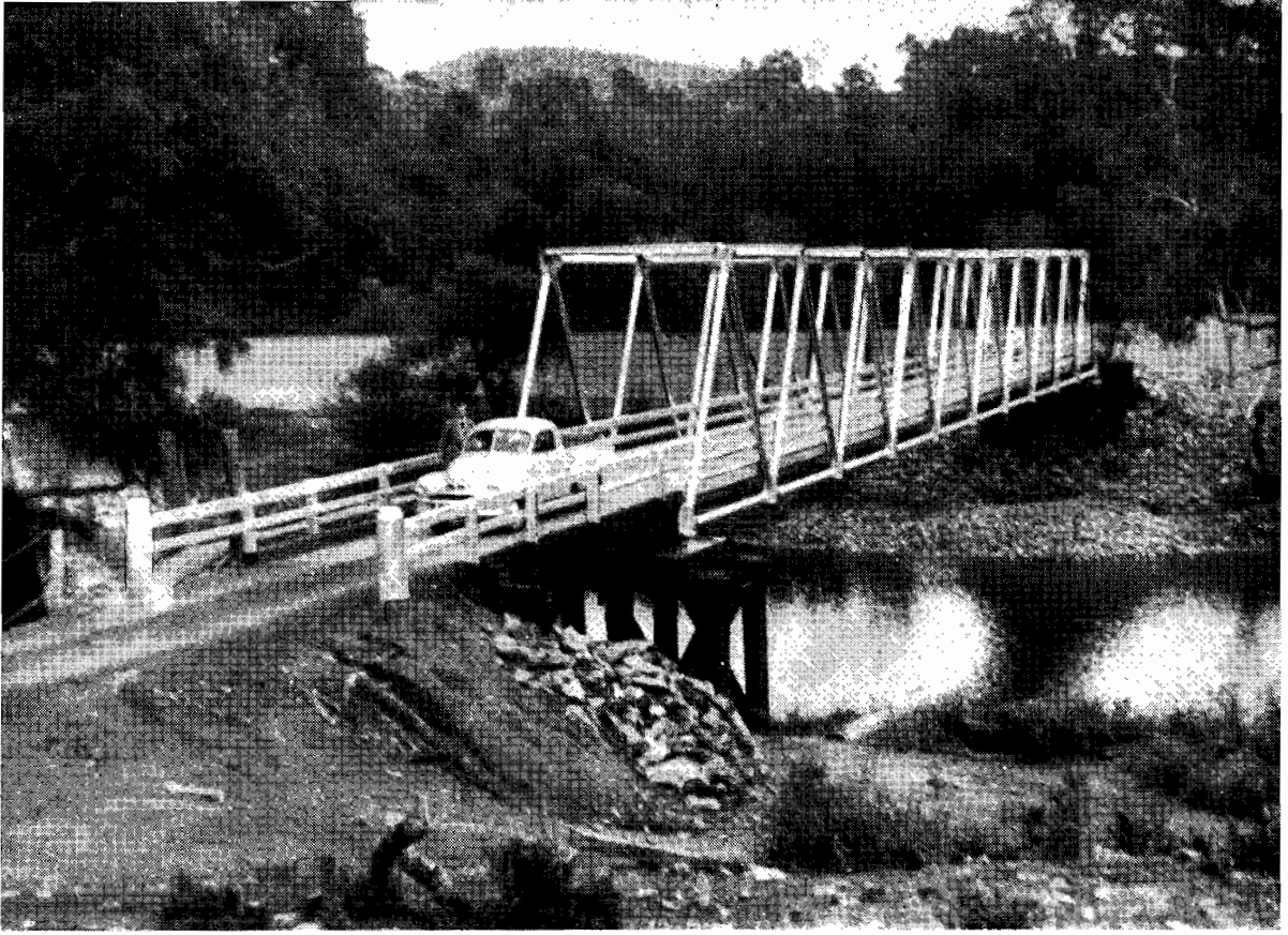
Plate No. 40.—Steel truss bridge, Crooked River Road, over Wonnangatta River.
