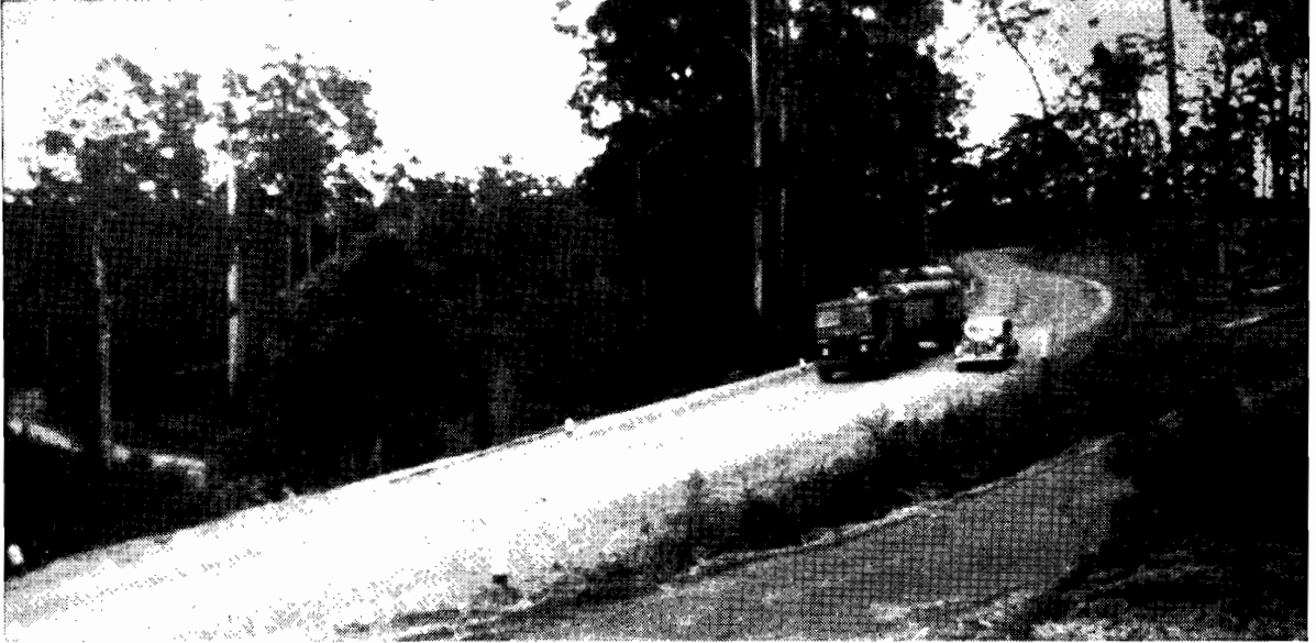
Plate No. 12.—Princes Highway East showing Mt. Raymond deviation at 245 miles.
