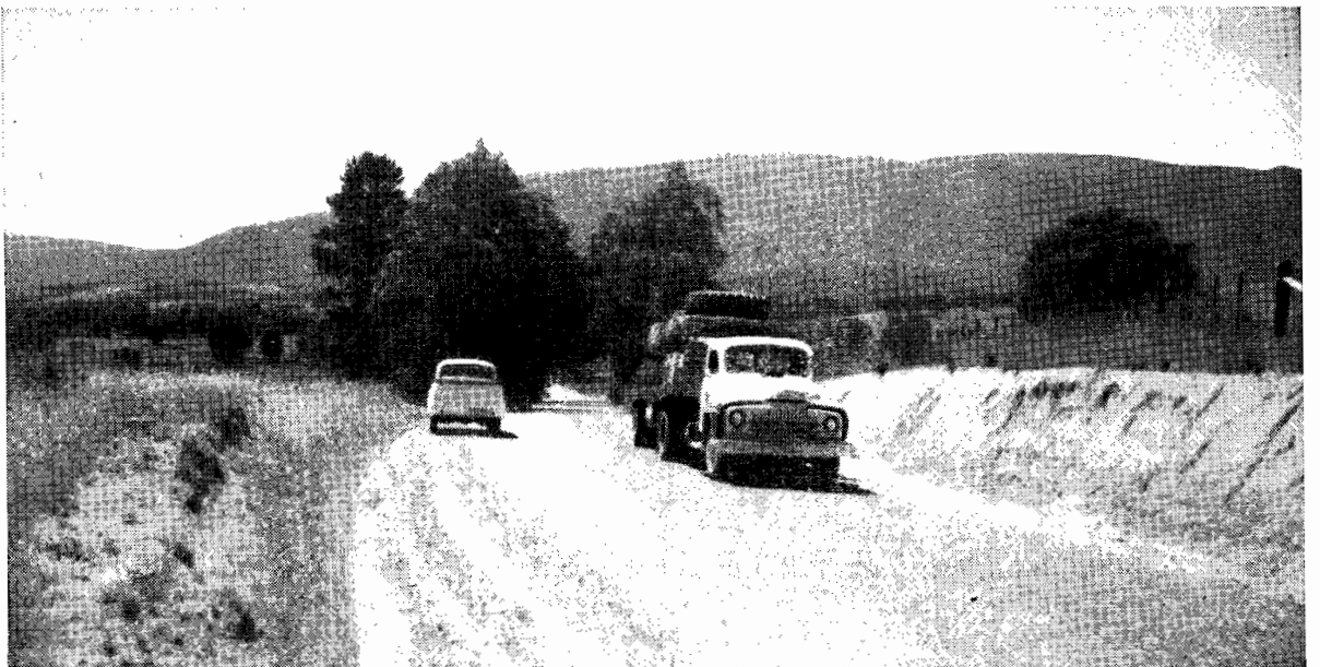
Plate No. 6.—Taggerty-Thornton Road, Alexandra Shire, section reconstructed and sealed.
