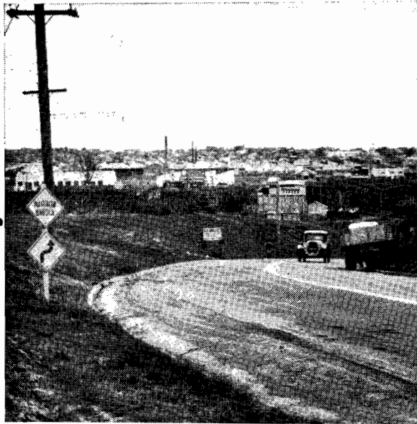
Plate No. 7.—Warning signs at old approach to bridge over Darebin Creek in Bell Street.
