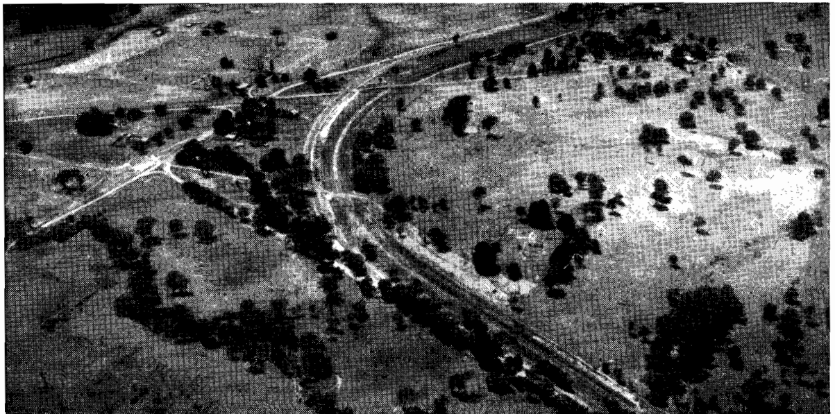
Plate No. 17.—Aerial view of reconstruction on Maroondah Highway at Merton.
