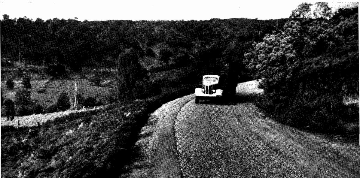
Plate No. 55.—A sheep transport on a completed section of the Longwood-Ruffy Road.
