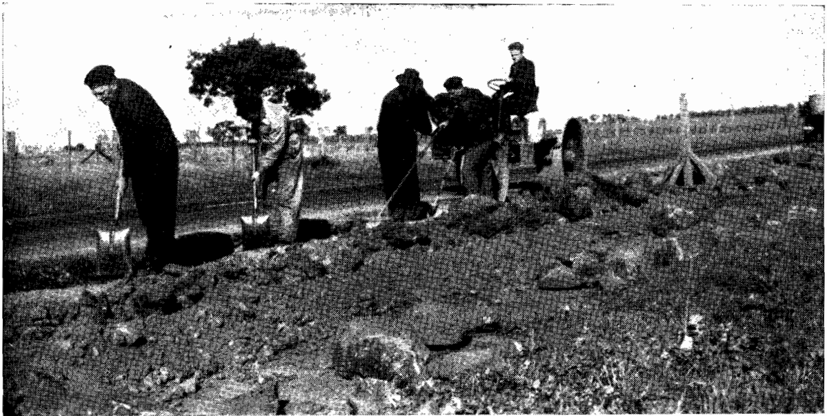
Plate No. 19.—Widening Hume Highway by 4 feet at 12 miles.
