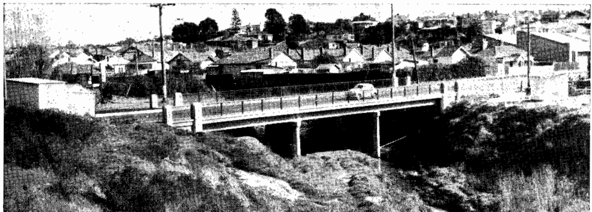
Plate No. 33.—New bridge over Moonee Ponds Creek in Albion Street.
