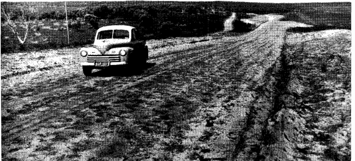
Plate No. 29.—Portland-Nelson Road, new formation approximately 7 miles west of Mt. Kincaid.
