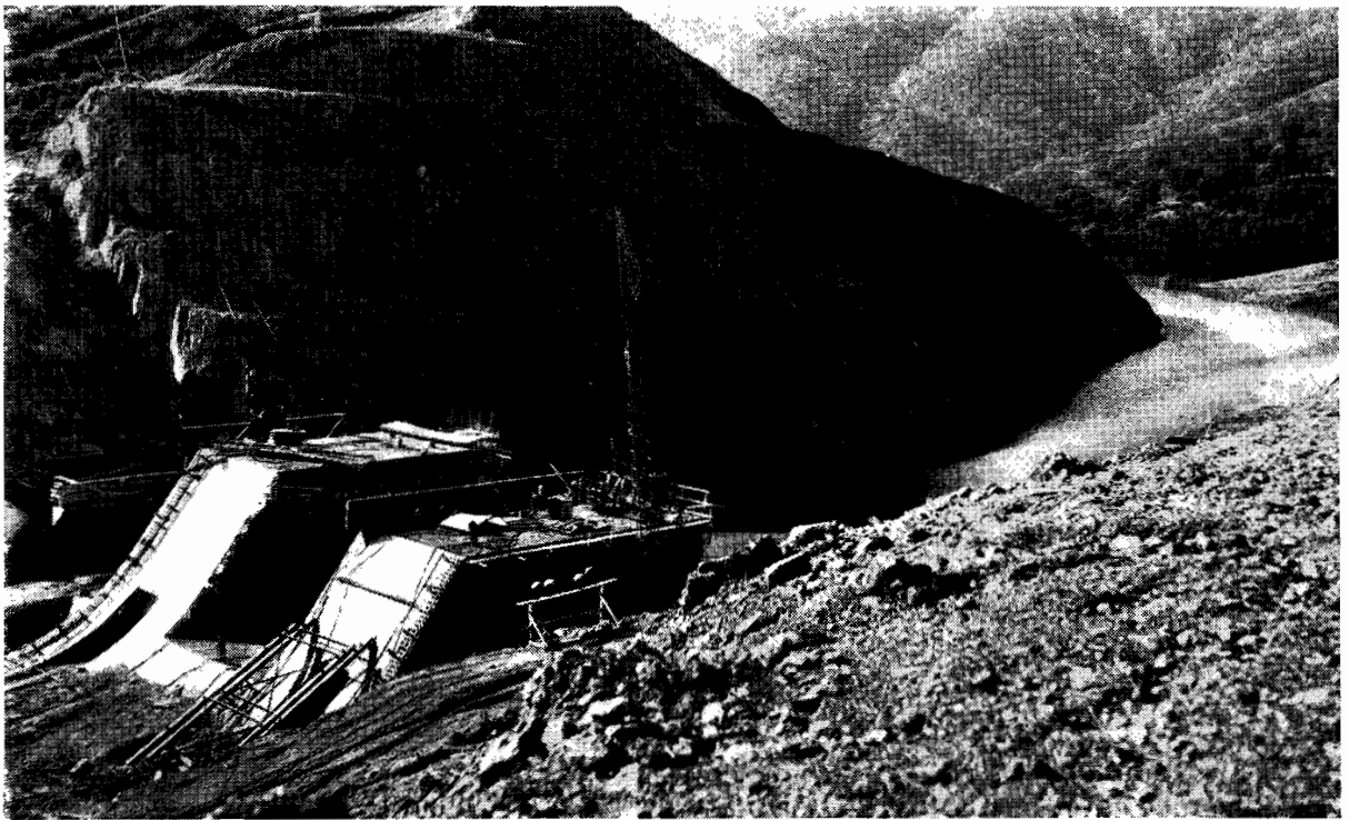
Big Eildon spillway under construction. The approach channel in the background has a depth of up to 250 feet and maximum width of 300 feet. The spillway structure in the foreground will be 215 feet wide and 100 feet thick at the base, and 120 feet high. In addition to three vertical lift steel gates, each 65 ft. 6 in. by 20 feet, two 68-in. diameter needle valves will also be installed in the structure.
