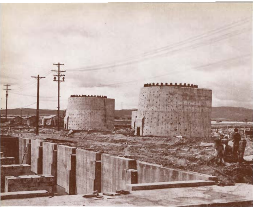
Bases for Boiler House chimneys — portion of briquette factory foundations at left.
