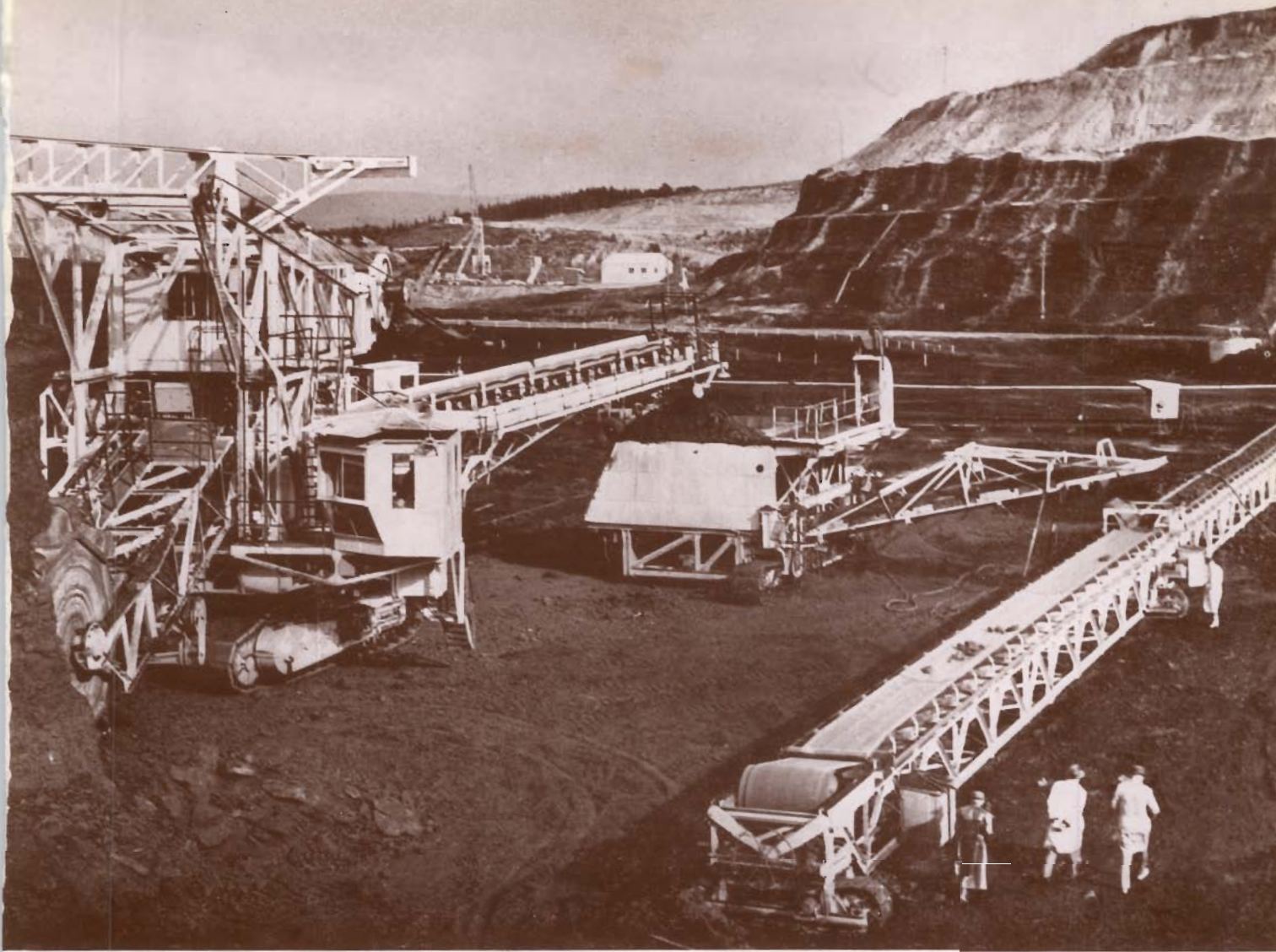
New Dredger (output 510 cubic yards coal per hour) and movable conveyors at Yallourn North Open Cut.
