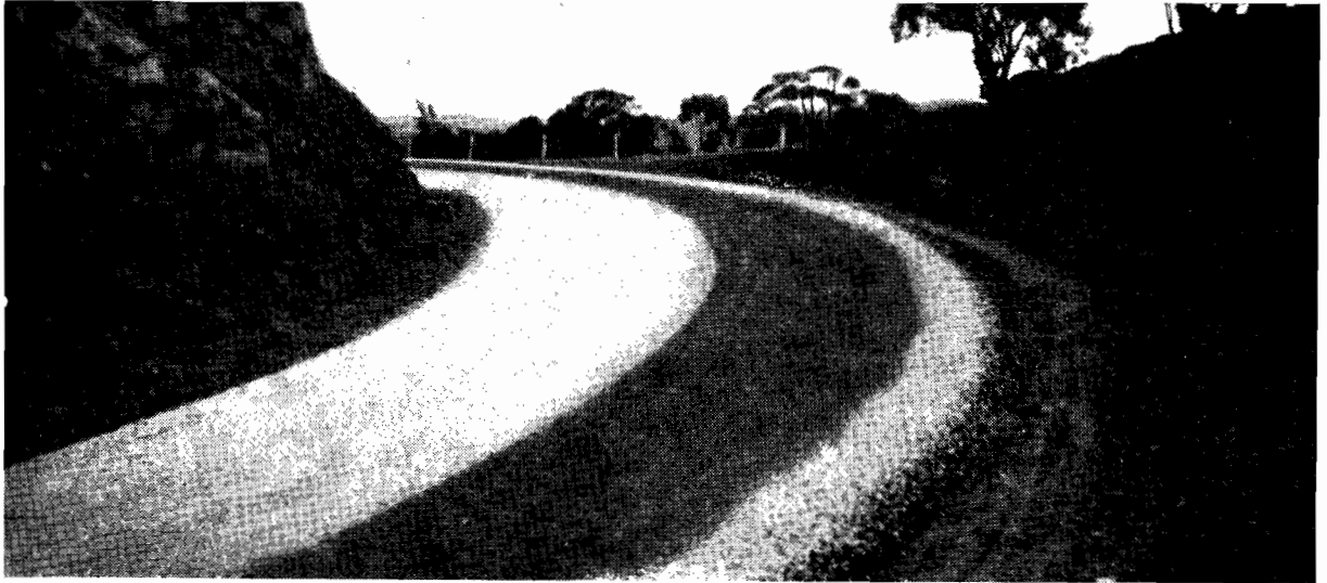
Plate No. 5.—Ararat Shire : Ararat—Halls Gap Road. Re-alignment over very steep hill (Cope's Hill) West of Ararat, where old pavement was practically worn out.
