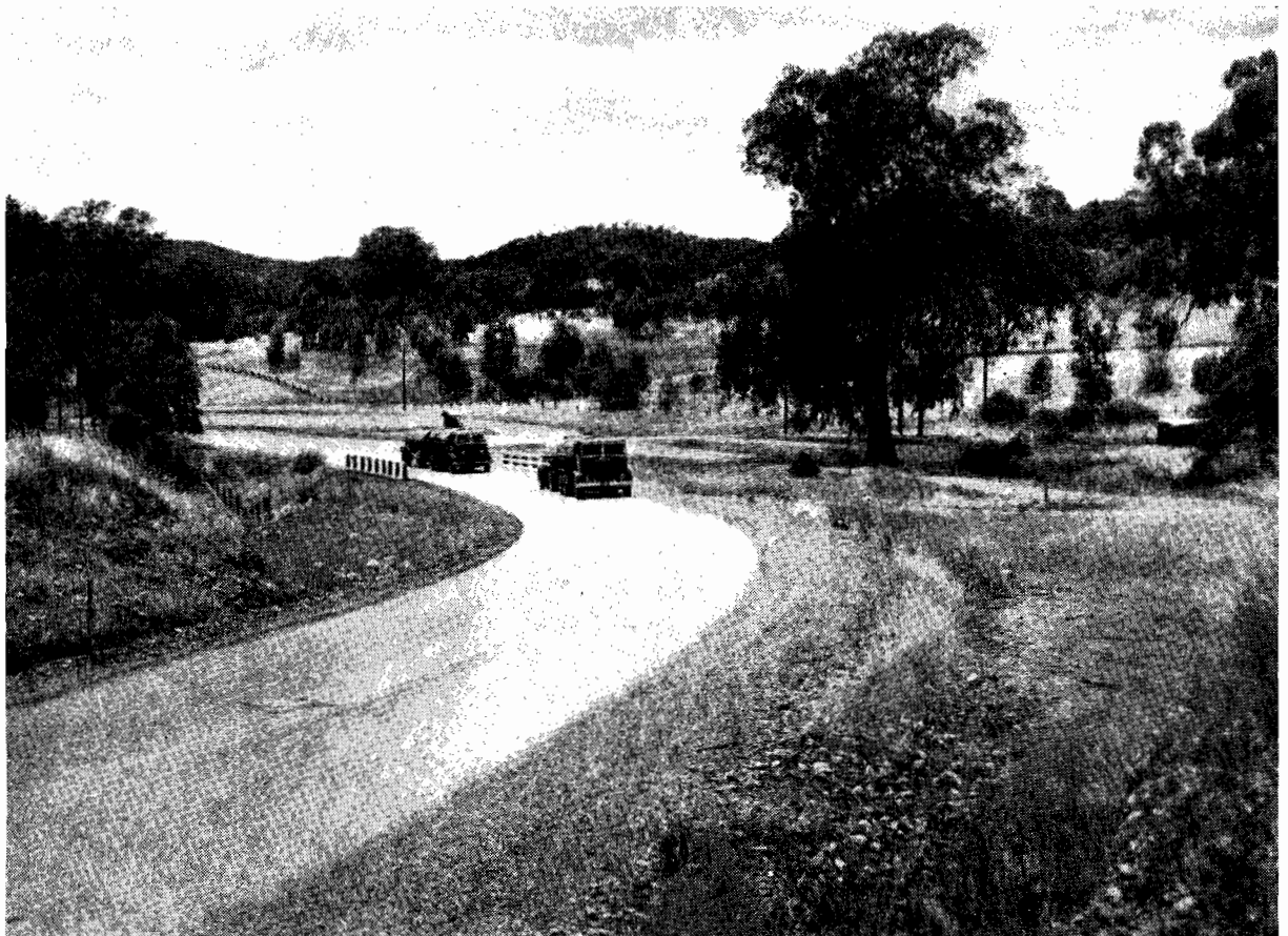
Plate No. 9.—Upper Goulburn Road. New structure replacing bridge shown above.
