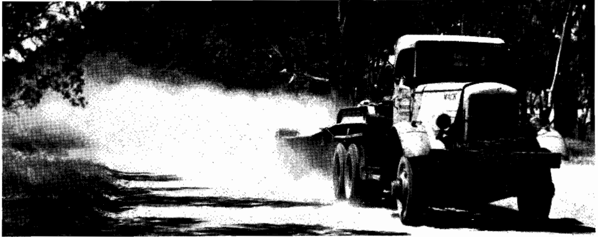
Plate No. 1.—Dust on worn out section of Pyrenees Highway near Elmhurst.
