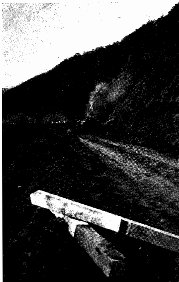
Plate No. 27.—Ocean Road. Cleaning up after landslip between Lorne and Skenes Creek.
