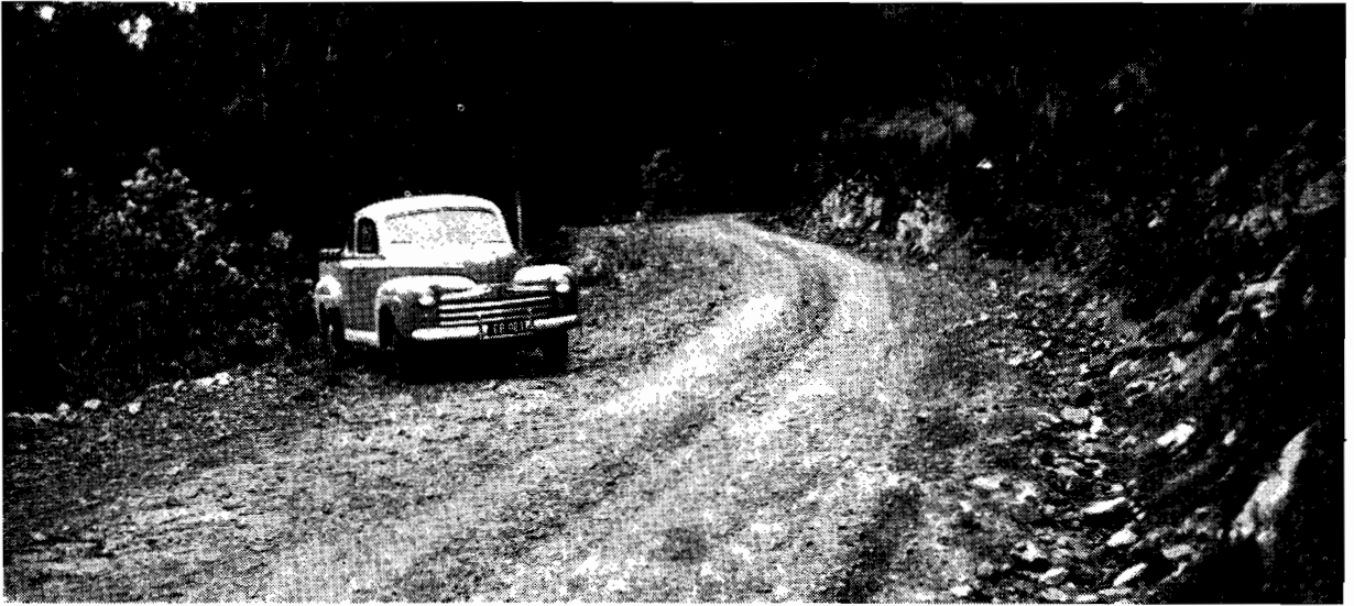
Plate No. 20.—Widened section Mt. Buller Road, providing for passing and parking.
