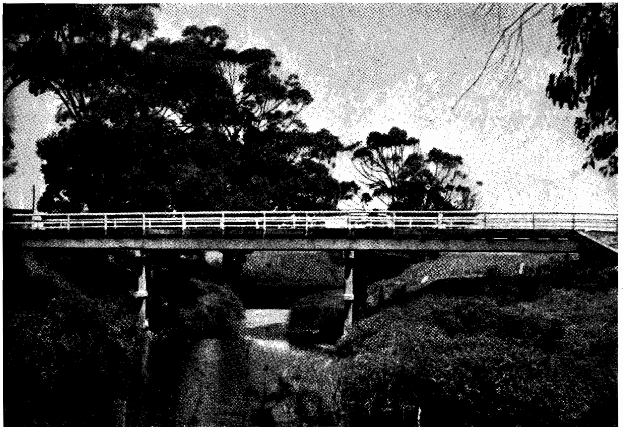
Plate No. 11.—Woorayl Shire : Nerrena Road Bridge over Tarwin River replacing worn out timber structure.
