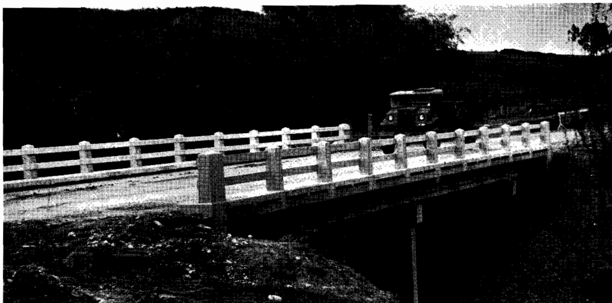
Plate No. 33.—Kiewa Valley Road. Bridge over Swamp Creek, designed for State Electricity Commission's heavy traffic.
