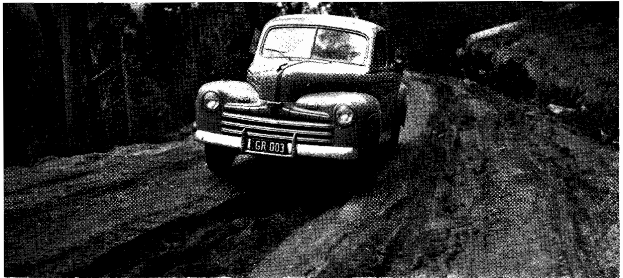
Plate No. 21.—Mt. Buller Road, ungravelled section under winter conditions.
