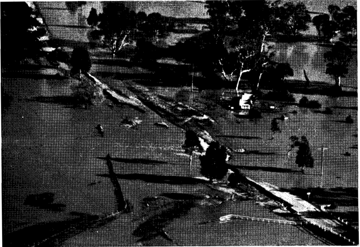
Plate No. 30.—Princes Highway East, washaway at Thompson River, Sale.
