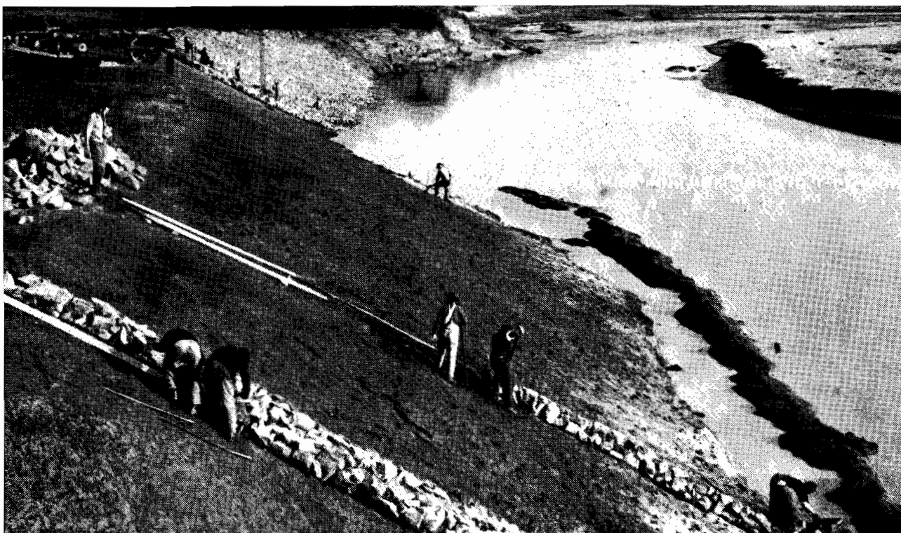
Fig. 9.—Sausages Placed in Position to Control Erosion.
