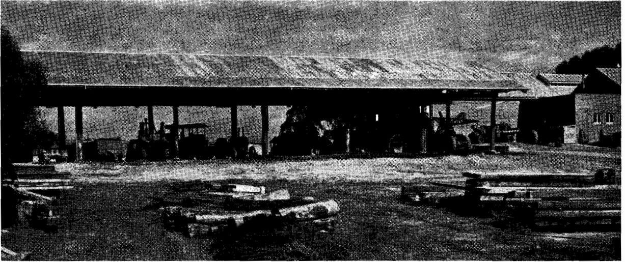
Plate No. 40.—Bendigo. Plant shelter.
