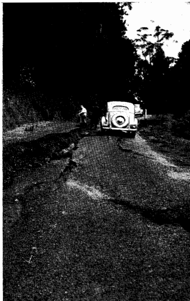
Plate No. 28.—Forrest—Apollo Bay Road. Subsidence destroying old permanent work.
