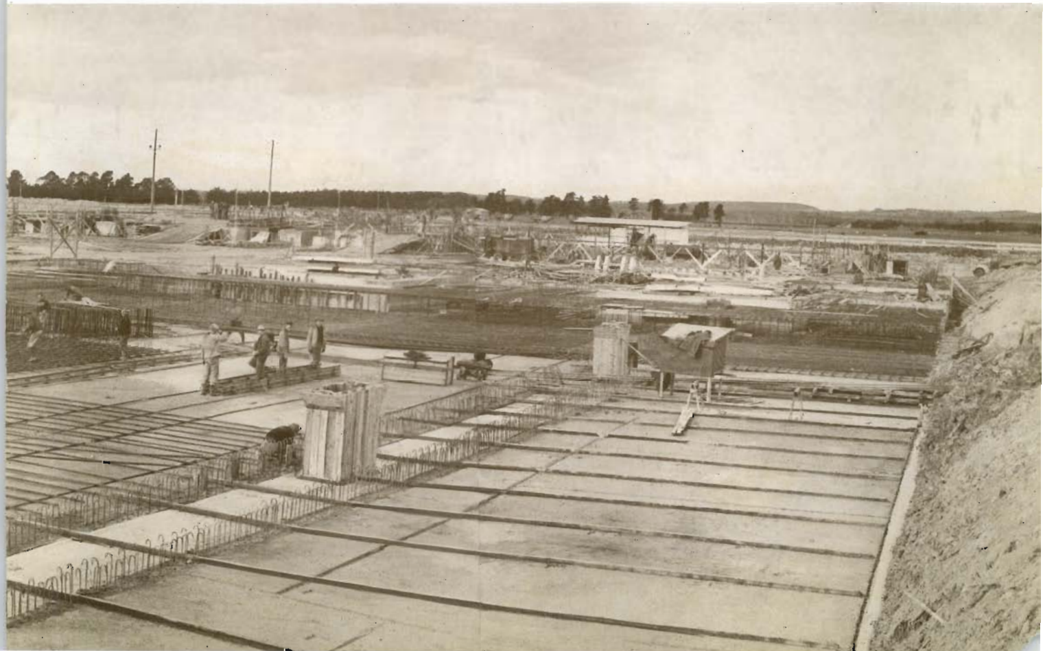
- Raft Foundations for Boiler House Building
