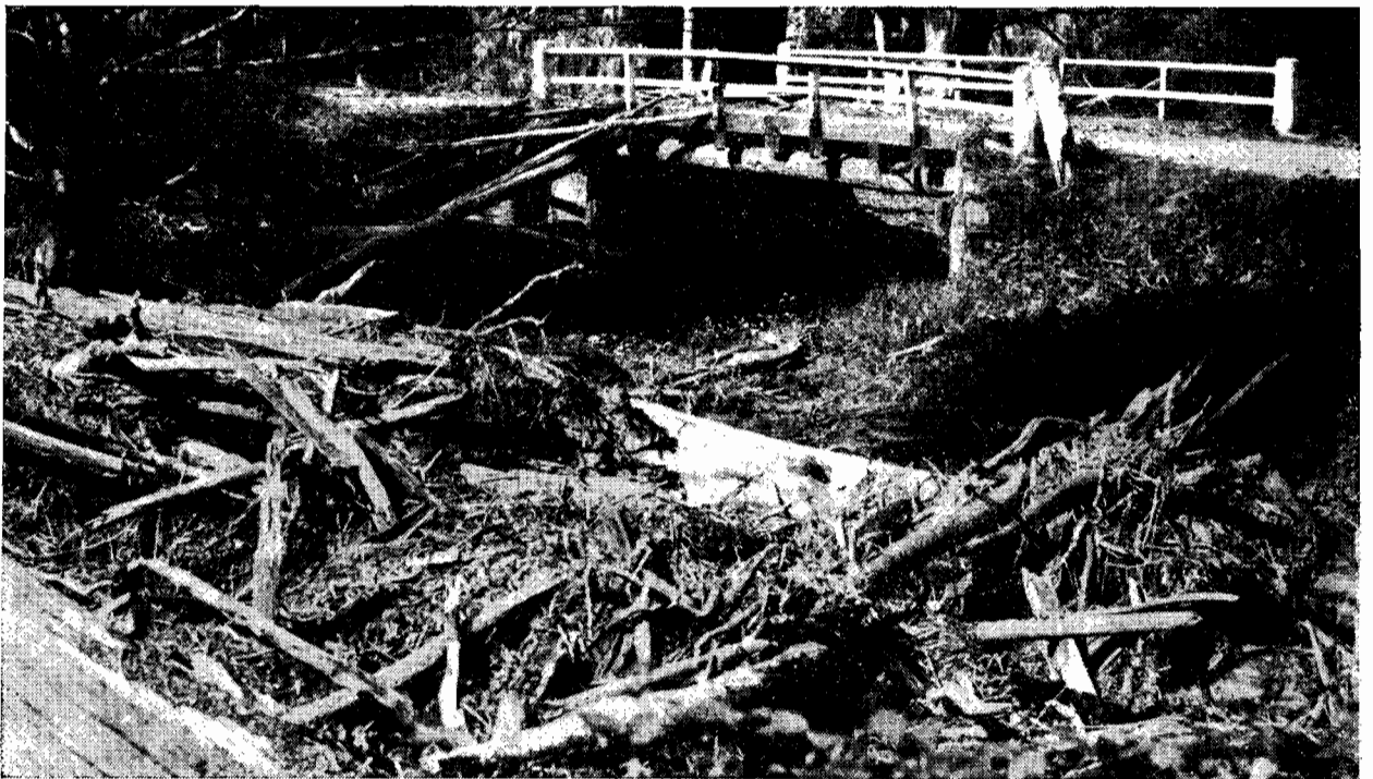
Fig. 6.—A timber bridge on the Traralgon Creek Road provided with a floodway. This was the only structure to survive the flood in this section.
