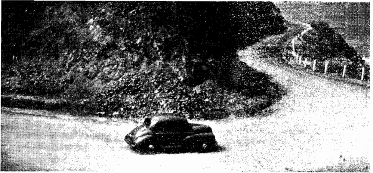
Plate No. 18.—A corner of the Ocean Road between Eastern View and Lorne, which has been widened for safety.
