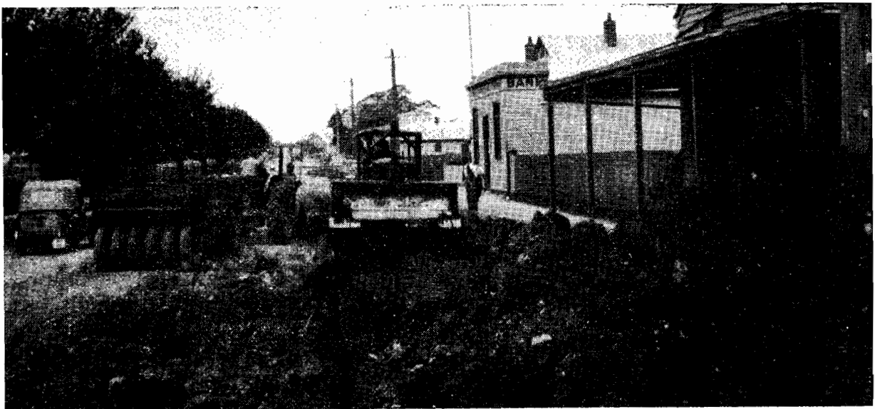
Plate No. 57.—Repairing the failed section of the Princes Highway East at Yarragon where the poor quality sub-grades were removed. Granitic sand was used for back filling to a depth of as much as 5 feet.
