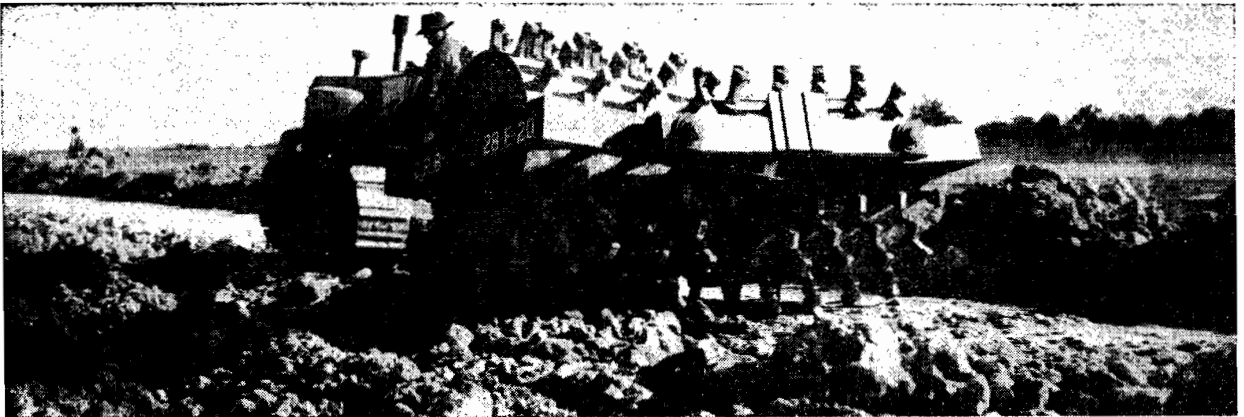
Plate No. 49.—A sheep's foot roller at work on the Loddon Valley Highway south of Kerang, compacting soft sandstone.
