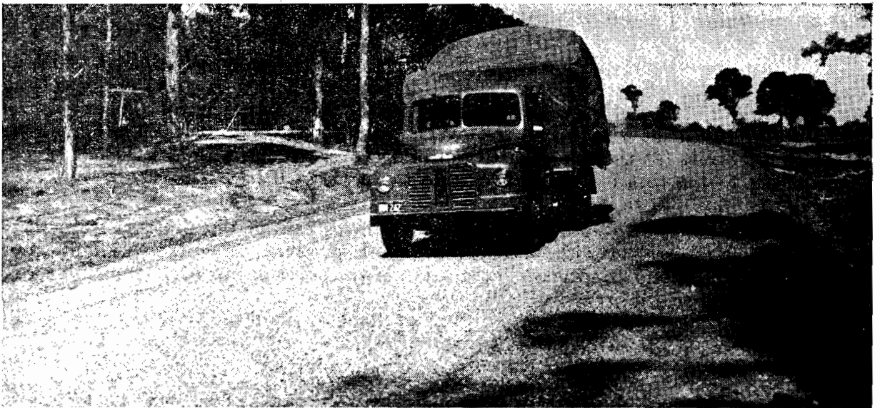
Plate No. 1.—Reconstruction and Sealing of the Omeo Highway near Bruthen.
