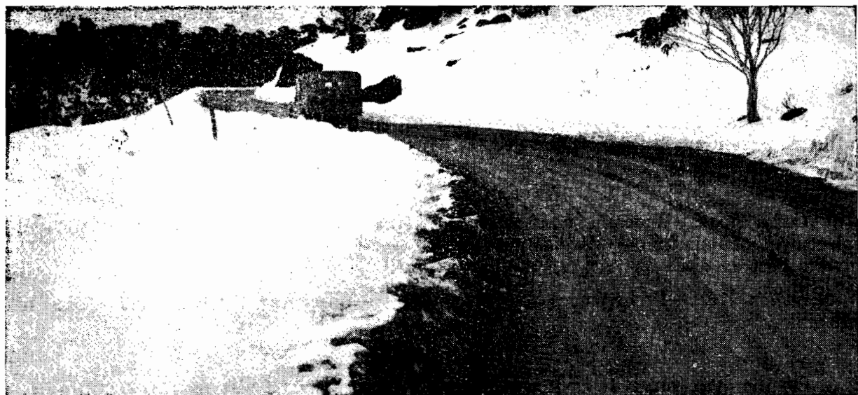
Plate No. 17.—A section of the Mt. Buffalo Tourists' Road near Mt. Buffalo Chalet, reconstructed after failure.
