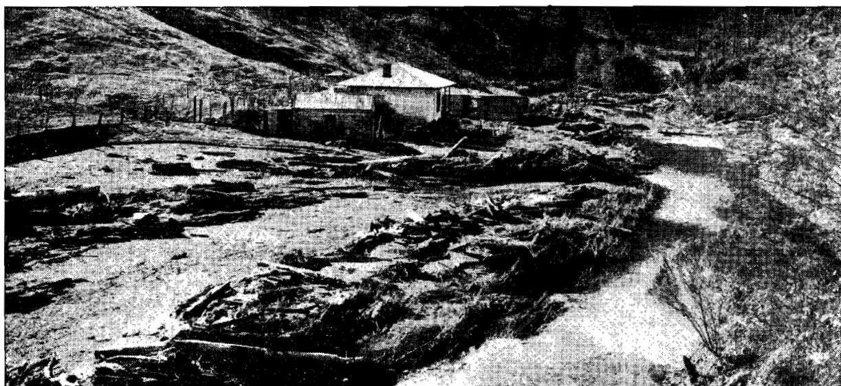
Plate No. 24.—Eight bridges across the Traralgon Creek were destroyed as a result of the 21-inch fall of rain at Balook at the head of the Catchment Area in February, 1951. The photograph above shows the debris just below Caldwell's Bridge.
