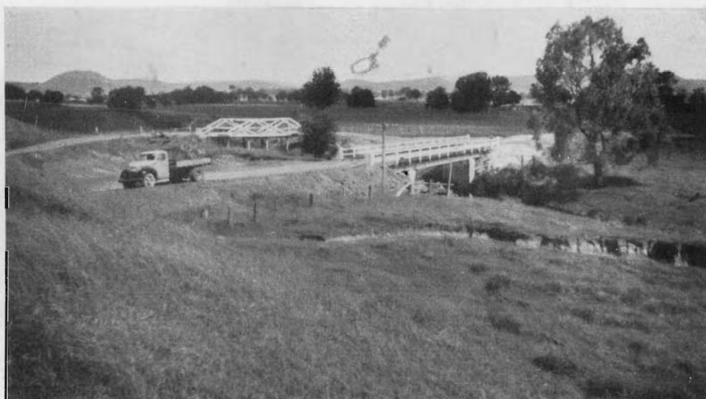
11. Benalla Shire. Mollyullah-Tatong Road. New bridge over Ryan's Creek.
