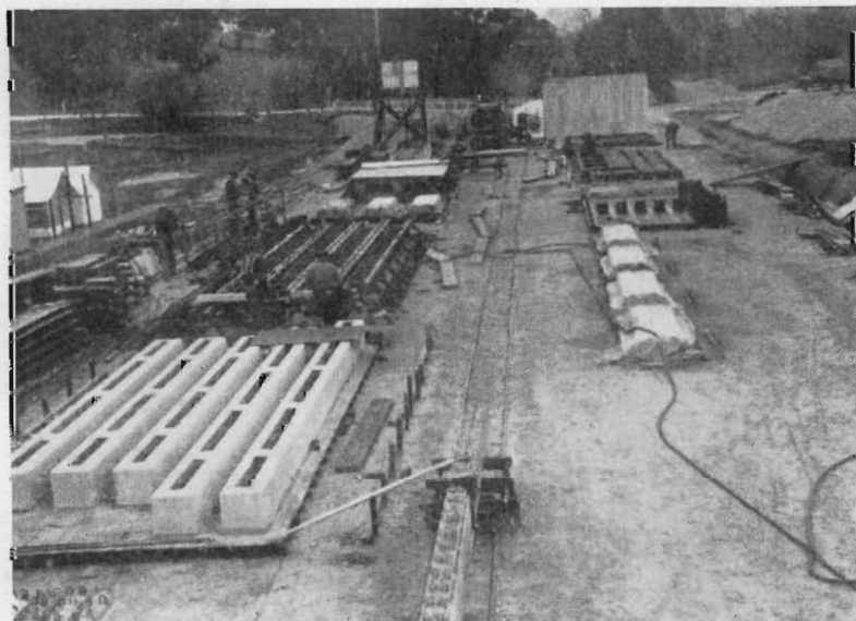
36. Kiewa Valley Road. General view of reinforced concrete bridge casting depot.
