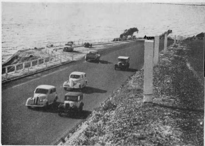
3. Nepean Highway. Completed pavement at Oliver's Hill.
