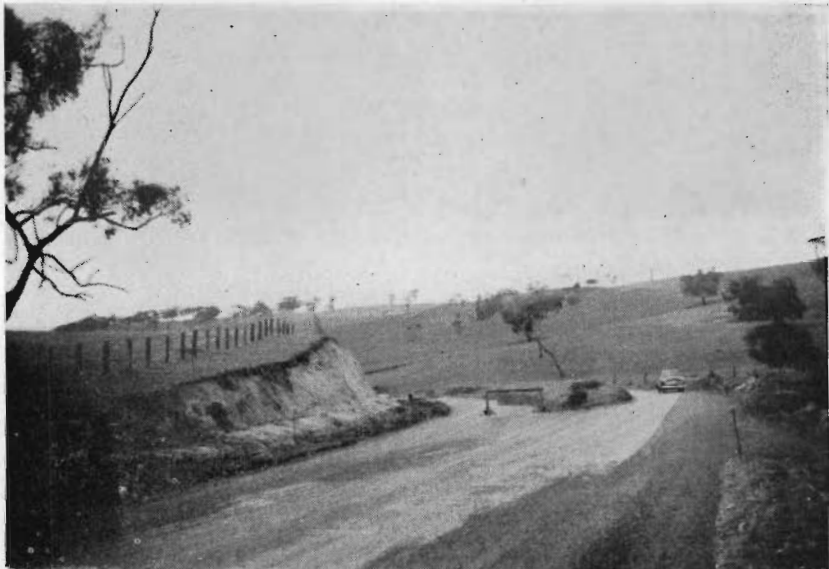
5. Western Highway. Reconstruction work in progress between Bacchus Marsh and Myrniong.
