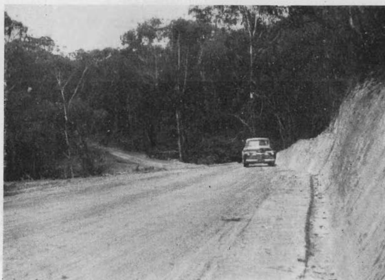
10. Lockhart's Gap Road. Section shown in plate No. 7 after reconstruction.
