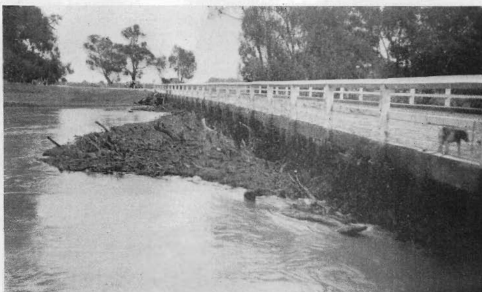
25. Goornong - Colbinabbin Road. Debris at Ferguson's Bridge over Campaspe River after flood in October, 1949.
