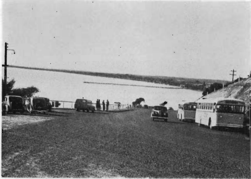
4. Nepean Highway. Completed pavement at Oliver's Hill.
