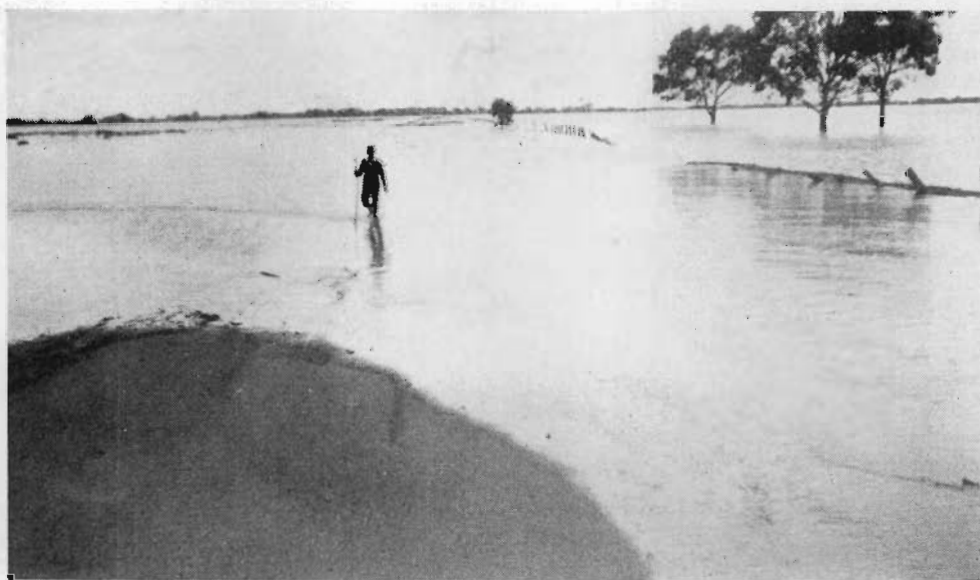
24. Midland Highway. Flooded section at Wallinjoc Swamp, approximately 5 miles west of Stanhope—March, 1950.
