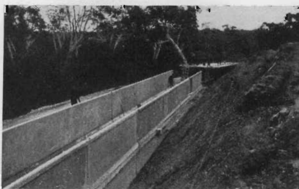
Reinforced concrete bench flume on Rocklands Outlet Channel. The flume is 10 feet wide and 6 feet high.
