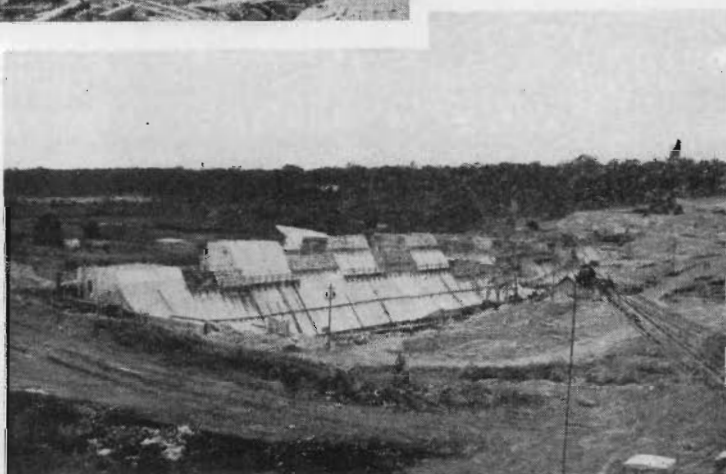
Above.—Rocklands Dam.—General view of progress at stage when top of concrete had reached a level 25 feet below crest of spillway.
