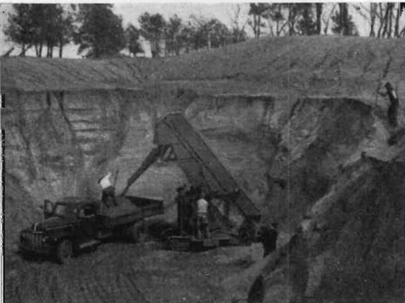
3. Murray Valley Irrigation District.—Loading sand for use in channel structures.
