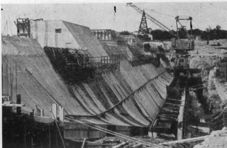
At left.—Rocklands Dam.—Looking along downstream face of dam. Six-ton portal crane for handling formwork at right.
