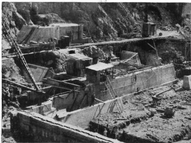
Foundations for Clover Dam taking shape.
