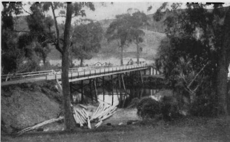
Plate No. 4. New Bridge over Macalister River at Licola.
