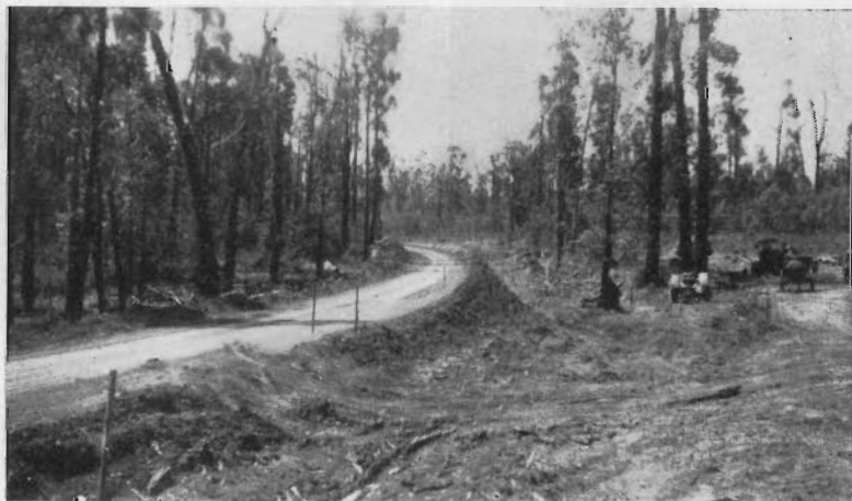
Plate No. 1. Reconstruction of Princes Highway East near Cabbage Tree.
