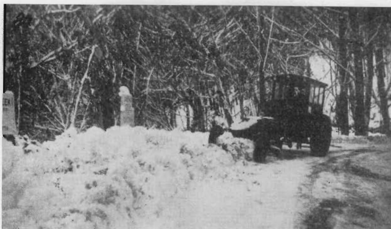
Plate No. 14. Omeo Highway. Snow clearing with light power grader.
