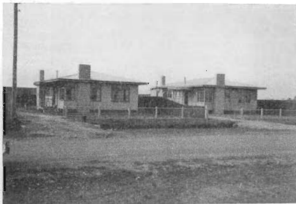
Plate No. 18. Prefabricated houses at Horsham depot.
