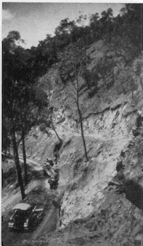
Plate No. 11. Warburton-Woods Point Road. Widening in progress near Muddy Creek.
