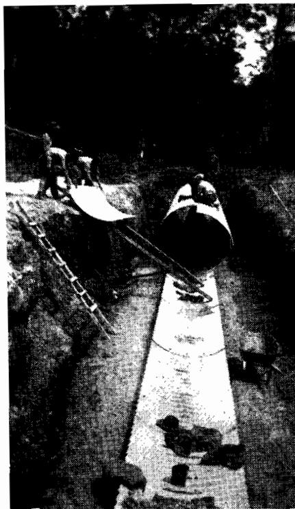
Plate No. 3.—Installation of 75-in. multi-plate culvert at McDonald's Creek.
