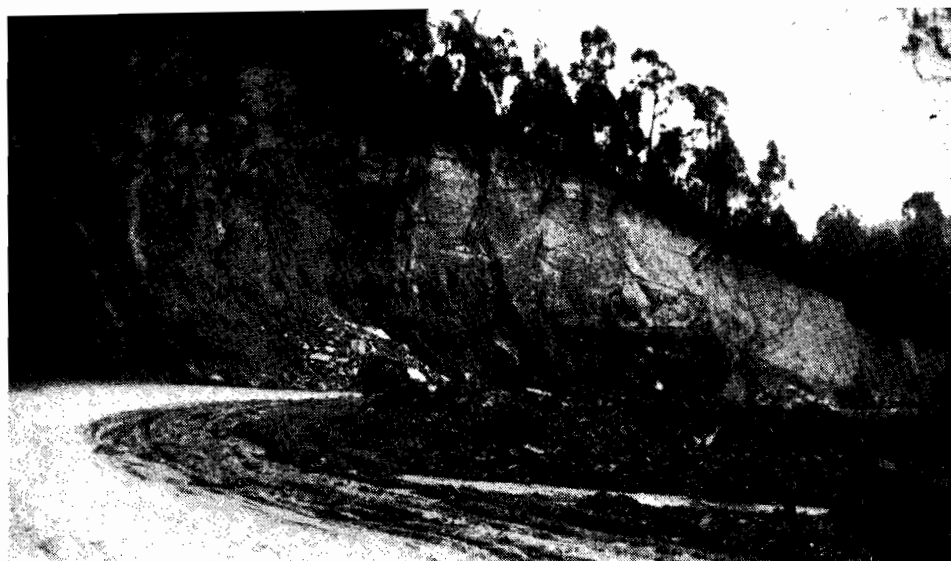
Plate No. 4.—Widening on a curve previously 15 feet formation with river on one side.
