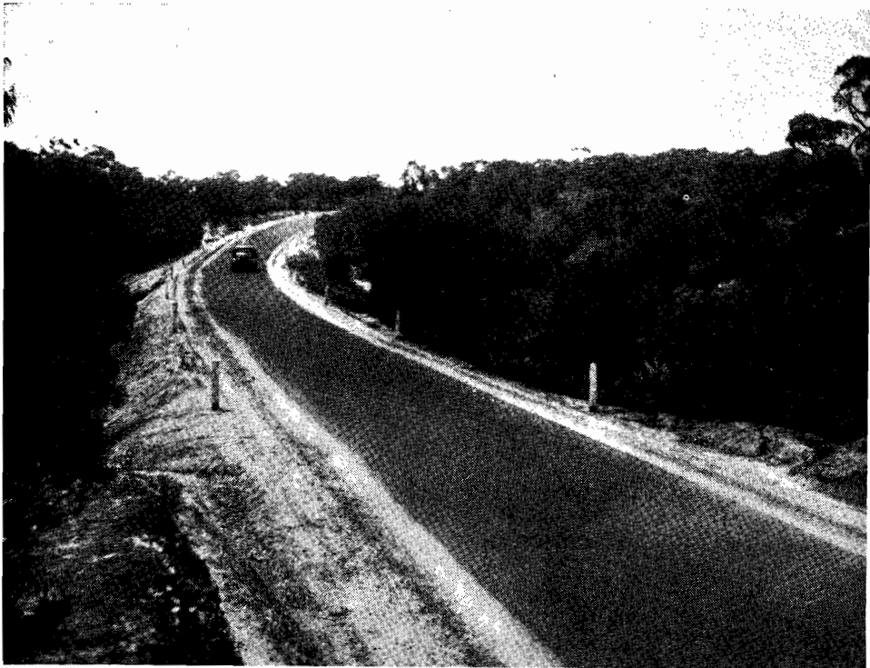
Plates Nos. 5 and 6.—Bass Highway—completed sections north of Grantville.
