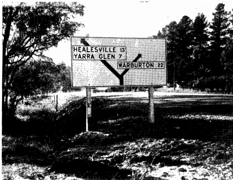
PLATE NO. 12.—Maroondah Highway. Advanced direction sign near Lilydale.
