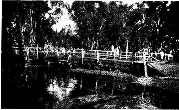
PLATE No. 20.—Grampians Road. Old bridge over Mokepilly Creek.
