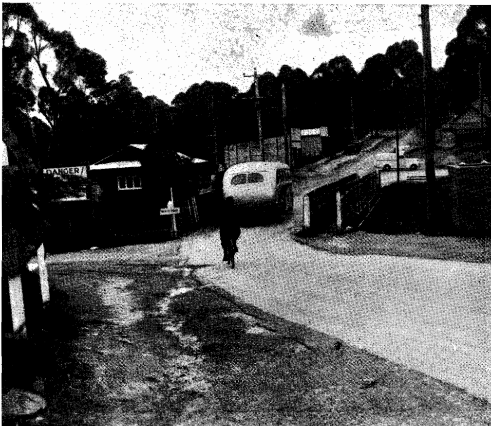
Plate No. 8.—Bridge over railway at Belgrave.
