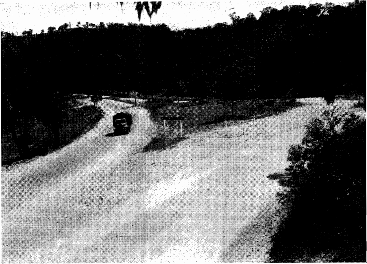
Plate No. 1.—New junction of Main Healesville and Warburton Roads near Lilydale (old junction on right).
