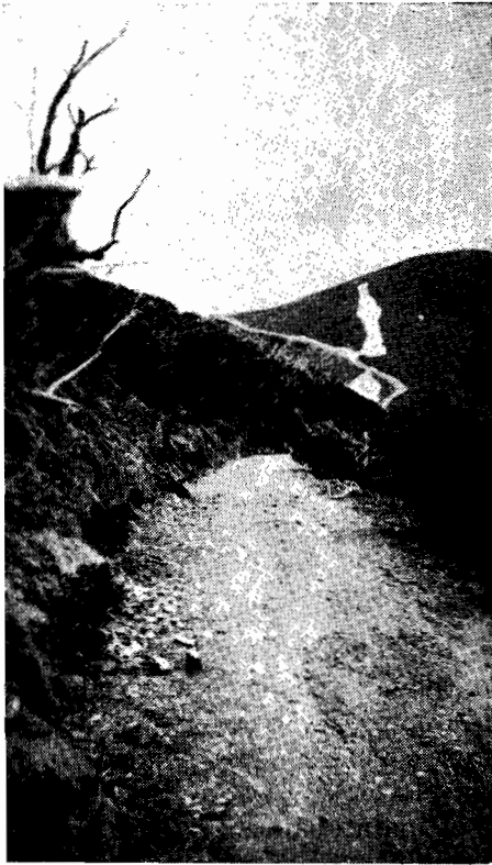
Plate No. 2.—Alpine Road near Mount Hotham—unwidened section.
