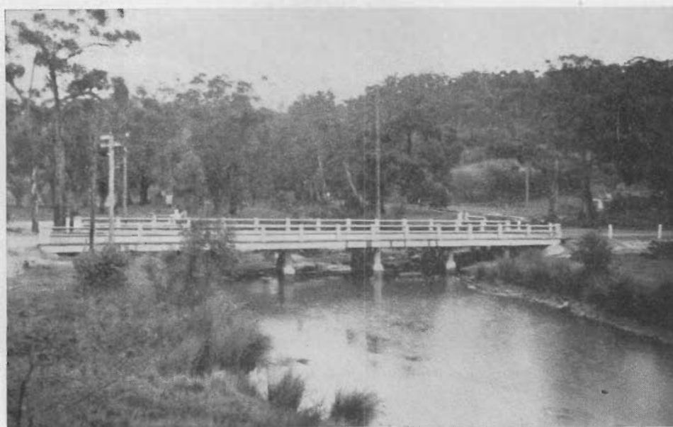
PLATE 5.—New bridge over Erskine River on Ocean Road at Lorne.
