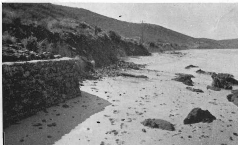
PLATE 4.—Sea wall at Eastern View, and site for extension.
