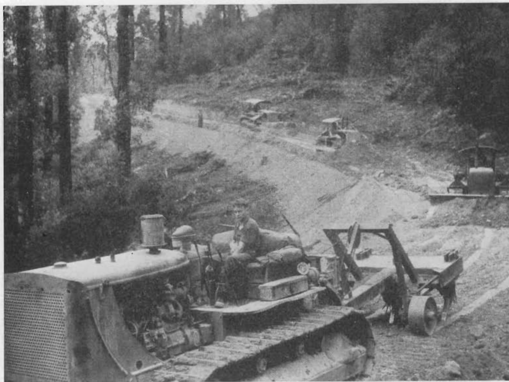
PLATE 8.—Work in progress on Reefton Spur Road.
