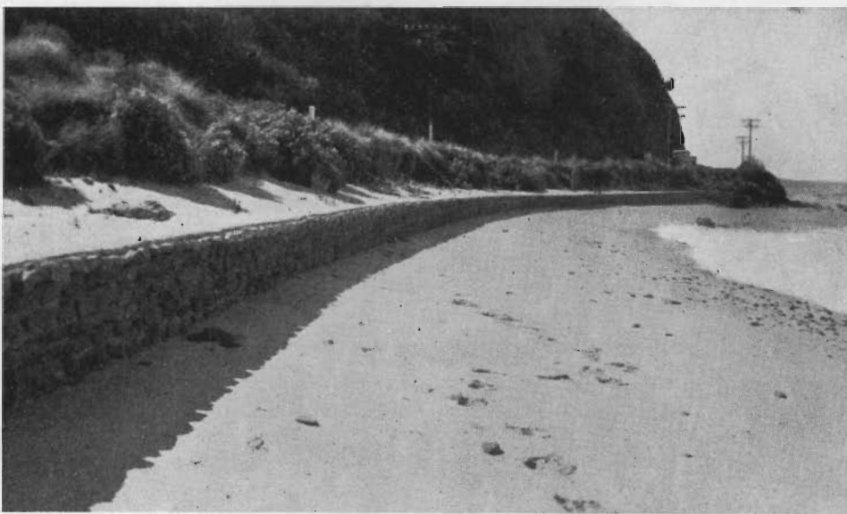
PLATES 1 and 2.—Sea wall constructed at Cathedral Rock, Lorne.
