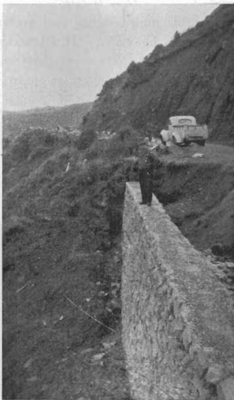
PLATE 3.—Section of completed wall before placing of filling.
