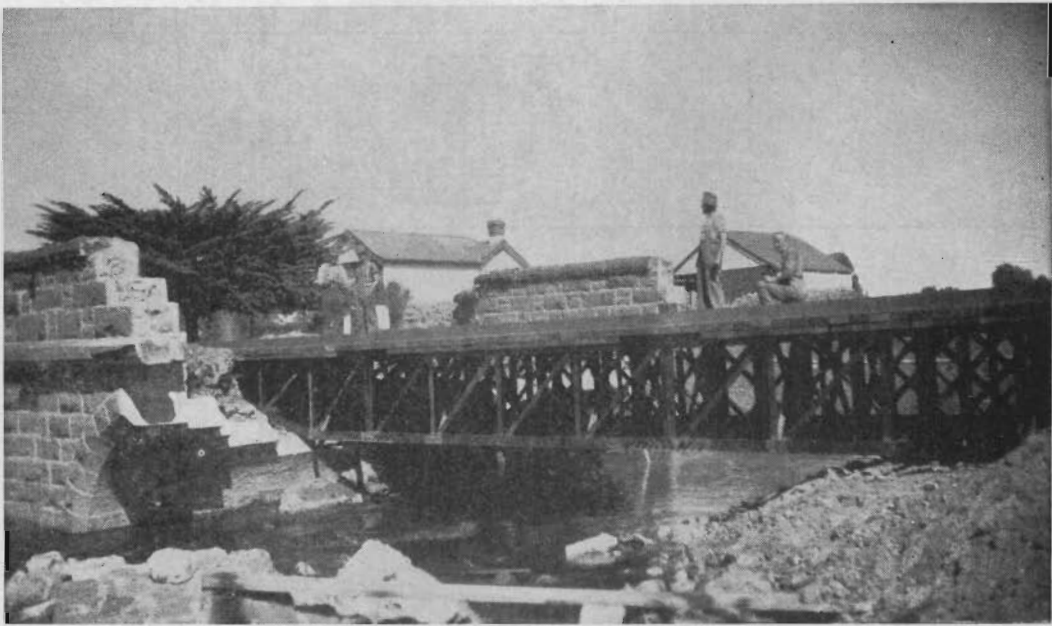
FIG. 2.—Temporary bridge over Main Drain at Port Fairy.
